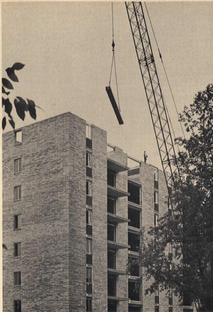
Eight story apartment uses Hi-Stress Deck on masonry bearing walls.
