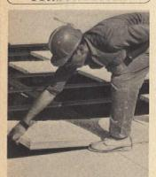
Perlite lightens roof panels. High strength and low density of reinforced concrete roof slabs made with perlite aggregate are said to offer good insulating and acoustical properties. "Tuflon" panels, 2' x 4' or 24" x 32" in varying thicknesses, provide an interior surface that may be painted or left exposed; top side has smooth surface ready for conventional roofing. Illinois Brick Co., 228 N. La Salle St., Chicago, Ill. 60601.
