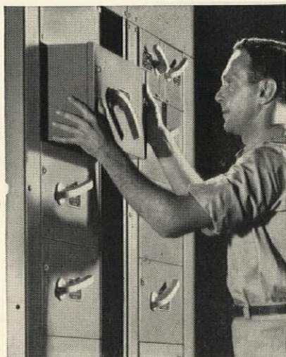
Individual switch units, even whole sections, can be added or changed as requirements dictate.
