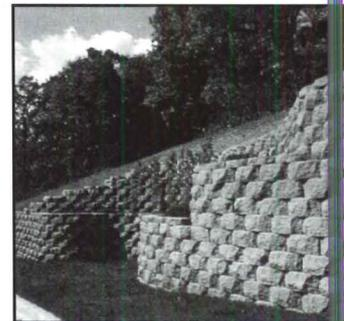
**Retaining walls** may be specified in three sizes, with different face patterns and angles, and in a variety of colors. Standard units weigh about 94 pounds. Keystone.
