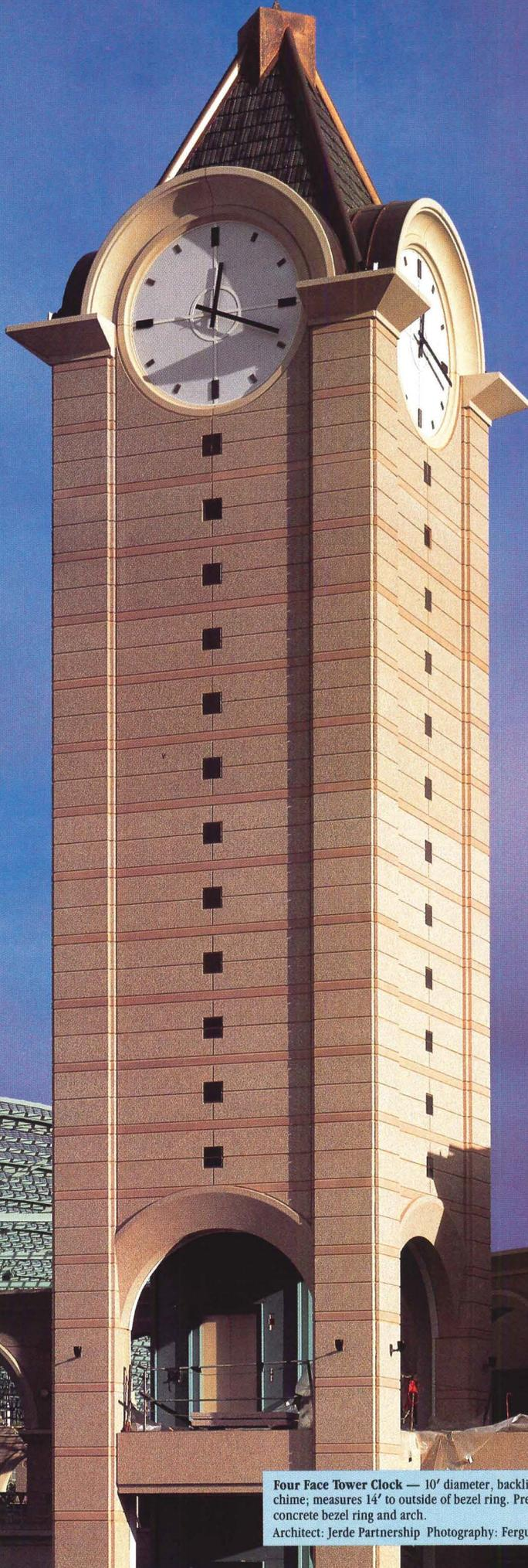
**Four Face Tower Clock** — 10' diameter, backlit dials; Westminster chime; measures 14' to outside of bezel ring. Pre-fabricated resinous concrete bezel ring and arch.
