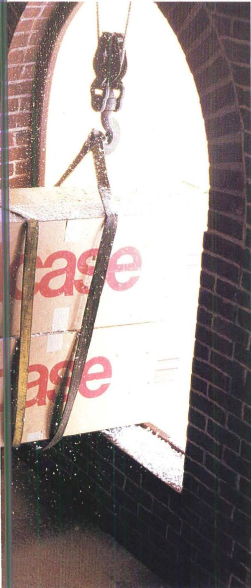
The best approach, they decided, was to jury-rig an outside elevator. They took out a third-story bay window. Built a scaffold. And rolled a giant crane over from Kodak. Steelcase’s deliveries were coordinated so that as furniture arrived, it was unloaded, hoisted up to the scaffold, and moved in through the window.
