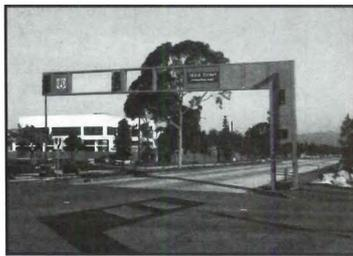
**Lighting and traffic control** modules are finished in Nickclad® and are supported by two heavy-wall rectangular legs joined by steel cross-braces. The demountable units have provisions for telephone booths, emergency call boxes, litter containers, parking meters, pedestrian push buttons, and traffic controller cabinets. Urbanco.
