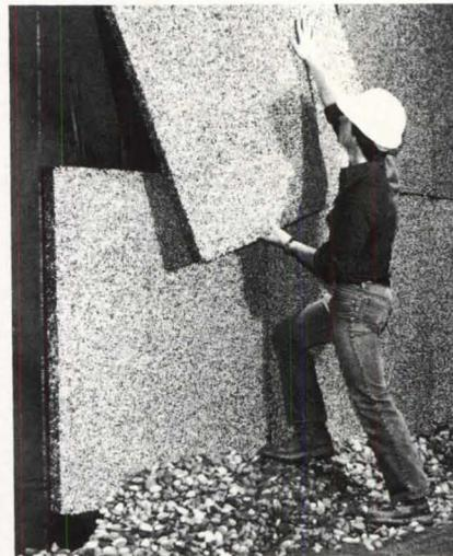
New GeoTech Drainage Board relieves the problems and expense of gravel fills below grade. Economical Drainage Board eliminates hydrostatic pressure by ensuring groundwater drainage. It enhances the integrity of the waterproofing system, provides thermal insulation up to R-3.5 per inch, and protects the structure from backfill damage.
