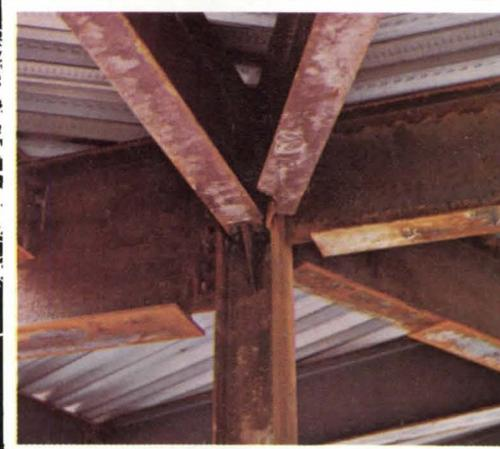
Although many of the connections were skewed, no difficulty was encountered during the fabrication or erection of the frame.
