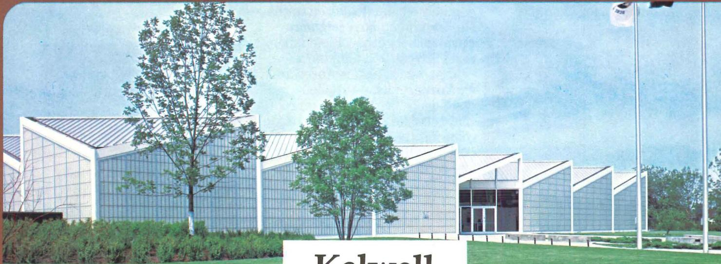
KALWALL® SYSTEMS . . . are BOTH **LIGHT TRANSMITTING** — light transmission range 3% to 83% — AND **INSULATED** — U-Factors .40, .24, .15, and even .06 — WITH **SHADING COEFFICIENTS** from .85 to less than .06! They weigh only 1½ pounds per square foot, and are only 2¾ inches thick. They transmit natural, diffused sunlight; and keep heated (and cooled) air in.
