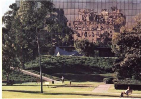
CNA Park Place is sheathed in nearly 146,000 square feet of PPG's *Solarban*<sup>®</sup> 480 *Twindow*<sup>®</sup> Insulating Glass. Its neutral gray reflectivity provides the unifying effect that makes this building a unique visual success. Its performance characteristics offset the higher cost by contributing to savings in heating and air conditioning equipment and operating costs. It is a building material ideally suited to the sunny climate and moderate building densities of Los Angeles.
