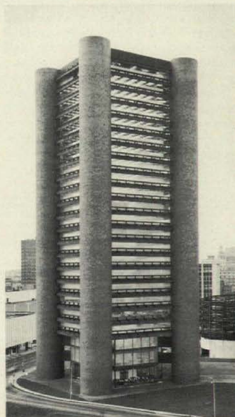
Weathering steel girders, slung horizontally between the towers and diagonally to connect with the central core, support floor beams and horizontal sun grilles.
