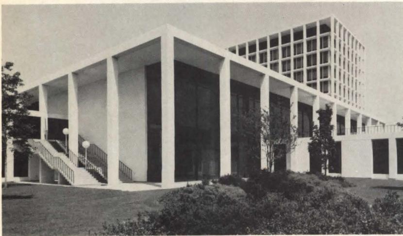
Two-story precast load-bearing panels of Pozzolith concrete in the departmental buildings (foreground) each measure 10' 6" wide and 27' 0" high. Each weighs 10 tons. Single-story panels in the administration building (background) are 5' 3" x 13' 6" and are non-load-bearing.
