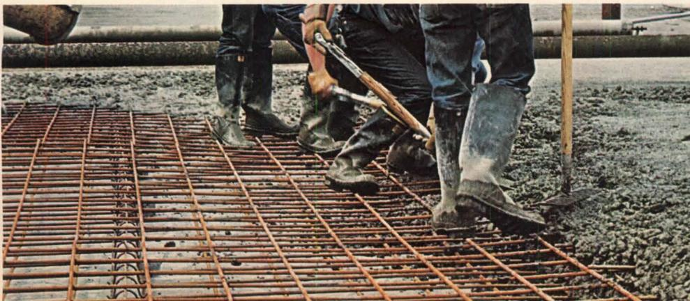
Keyweld concrete reinforcement fits the space and the specifications—in one layer or two—in sheets or rolls. There's a minimum of waste and cutting time—and practically no engineering supervision needed.
