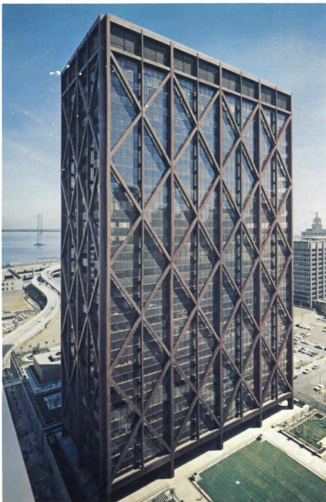
24-story Alcoa Building, San Francisco. Steel diagonal bracing, together with vertical hangers and only twelve exterior columns, form a sophisticated system for resisting seismic forces. Floors, column-free except for the service core, are suspended within the clad steel frame. Architect: Skidmore, Owings and Merrill.
