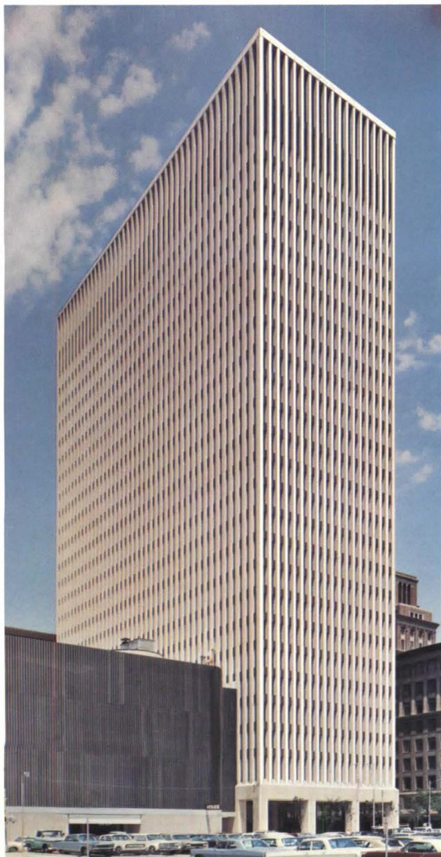
28-story Houston Natural Gas Building. ASTM A572 steel used in columns and beams for economy. Architect: Lloyd Morgan and Jones, A.I.A.
