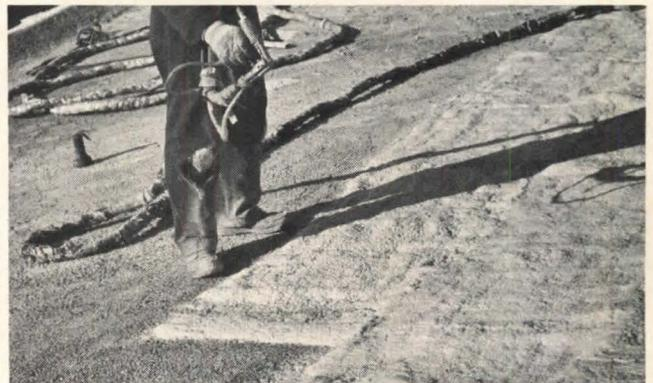
The 1" layer of urethane was applied to 98,000 sq ft by 3-man crew. Foam was later sealant-coated for added durability.
