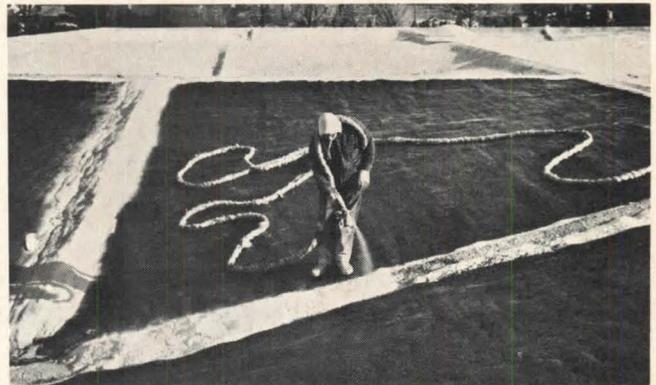
Good resistance of rigid urethane to thermal stress was critical factor in sealing expansion joints between parabolic shell sections on roof.
