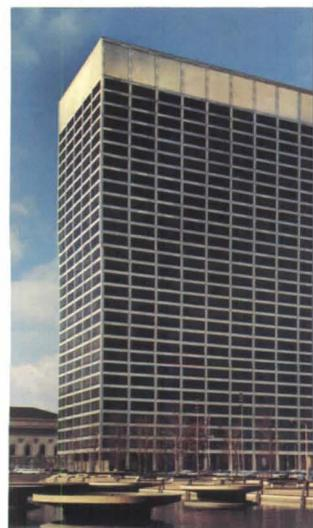
32-story Federal Office Building, Cleveland (at right). Columns in lower 9 stories are high-strength A441 steel to maintain same column dimension the full height of the building. Cellular floor system provides interior flexibility. Architects: Outcalt, Guenther, Rode & Bonebrake; Schafer, Flynn & van Dijk; Dalton-Dalton Associates.
