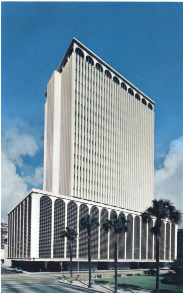
22-story Exchange National Bank Building, Tampa. Redesign in ASTM A572 steel (grades 50 and 55) saved \$45,000. Floor framing in office tower section is designed compositely with the slab. Architect: Harry A. MacEwen, A.I.A.
