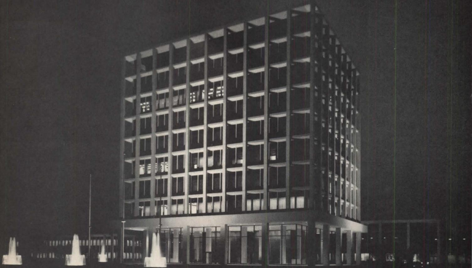
The face of Allstate Plaza is precast concrete panels of Indiana limestone aggregate. Sandblasting creates an interesting texture compatible with the rural surrounds. All precast and cast-in-place concrete contained Pozzolith admixture.
