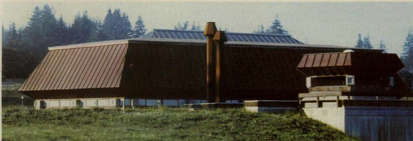
New Field House, University of California at Santa Cruz. Copper encloses the terminal chords of the two-way steel truss that spans the large main area of the building. Repetition of copper above an open stairway unites the design. The unusually prominent drip created at the eave gives strong definition to the roof.
