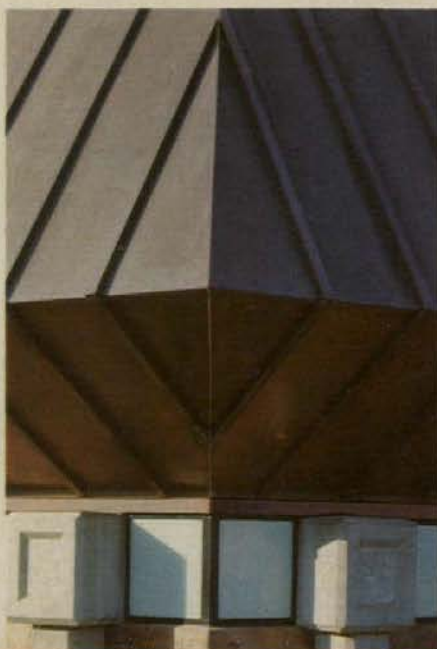
New Field House, University of California at Santa Cruz. Copper encloses the terminal chords of the two-way steel truss that spans the large main area of the building. Repetition of copper above an open stairway unites the design. The unusually prominent drip created at the eave gives strong definition to the roof.
