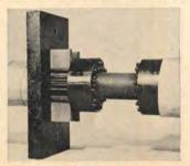
Here two tendons have been coupled. In final stage the ends and threads are mastic coated and covered with a sleeve.
