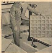
All-steel floor system for rooms requiring underfloor access and plenums comprises 2' x 2' standard panels and adjustable-height pedestals. A stringer system for increasing lateral stability is also manufactured. Brochure contains cutaway views, installation details and specifications. 8 pages. Tate Engineering, Inc., 516 S. Eutaw St., Baltimore, Md. 21201.
