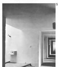
of concrete block. Cavity is foam-plasticfilled and window frames are stained softwood. Concrete toplights are doubleglazed. Interior finishes are simple: ceilings are plastered and painted white; walls are blockwork painted white; doors are painted orange, blue, or yellow; joinery is either left natural or stained. Ceiling of the library is timber-lined.
