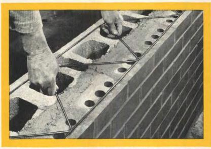
Dur-O-waL brand is the original masonry wall reinforcement with the truss design—for plain, composite and cavity walls. For added versatility and economy in masonry walls, use Dur-O-waL in lieu of brick headers, as approved by building codes. Send for your free copy of the new Sweet's Catalogue. Dur-O-waL, P.O. Box 150, Cedar Rapids, Iowa.
