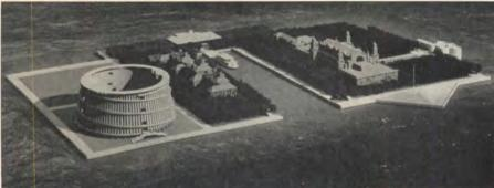
The cone will be spiraled within and without by 8-ft-wide ramps ascending to viewing platforms at various points of the structure. Johnson hopes to have plaques bearing the names of the immigrants who entered the U.S. through Ellis Island mounted between the vertical, prestressed concrete ribs of the building. A 100-ft-diameter pool will be located at the interior of the great court.
