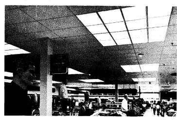
Westinghouse Frameless Mainliners fit flush with ceiling. Mainliners are fully gasketed to prevent light leak, have integral cantilever hangers to simplify installation. Shown in J. C. Penney store, Pittsburgh, Mainliners give bright, nonglare light, help display merchandise to best advantage.
