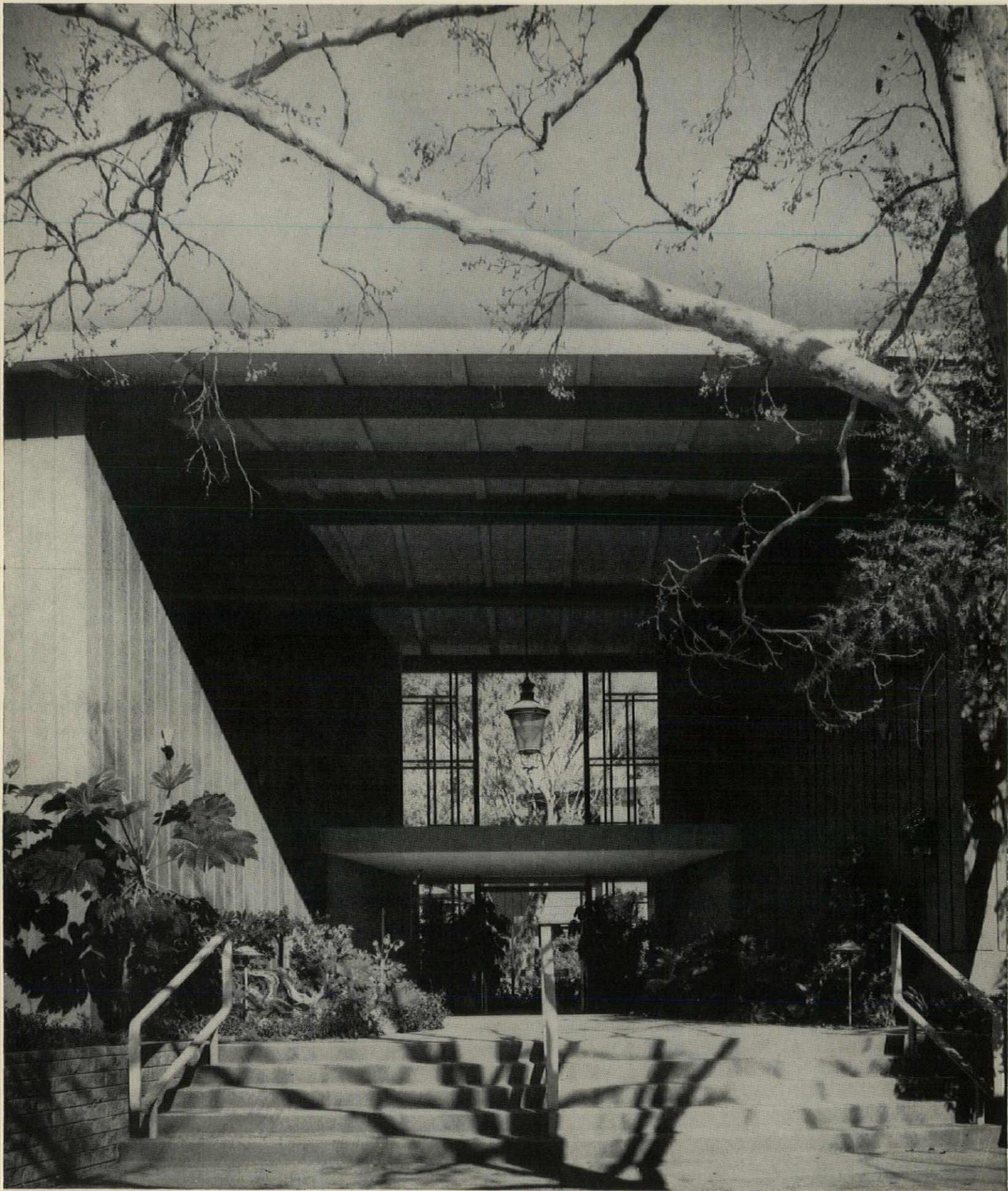
A glass-walled entrance framed with vertically channeled siding and a plank-and-beam overhead creates an imposing approach to the interior court of the Bay Tree Apartments. This extraordinary 7-unit, 2-story design is located in Los Gatos, California. Architect: Fred Marburg.
