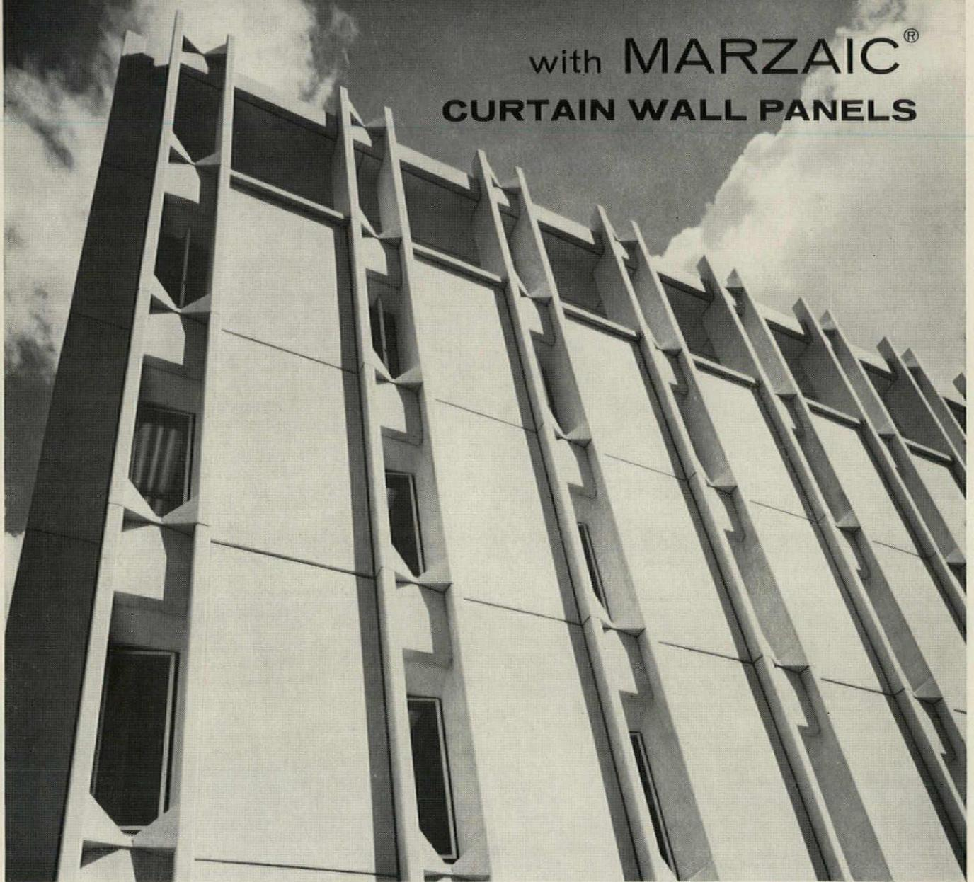
The exciting new design of the Leader Federal Savings and Loan Association Building has made it a center of attraction in Memphis. This new structure has gained recognition from all parts of the country as a pioneer in the trend toward frame type wall panel construction. Martin Marietta's frame type, Marzaic curtain wall panels have significantly contributed to the beauty of this building. The exterior surfaces of
