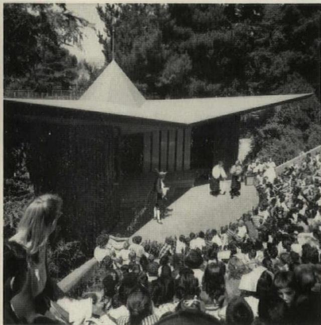
THIS INGENUOUS STAR-SHAPED ROOF demonstrates the remarkable structural forms that can be achieved with plywood. Deceptively simple, the design bears more resemblance to airplane wings than a conventional roof, with interacting plywood and lightweight lumber members forming skeleton and structural skin.
