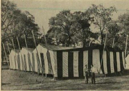
fabric made of "Acrilan" acrylic fiber. This solution-dyed fiber is watertight, colorfast, weather resistant, and resistant to stains, mildew, and moths. Manufactured by Glen Raven Mills, Glen Raven, N. C., the fabric's color is "locked in" by having it added while fiber is still in the liquid state. Other properties are dimensional stability, rapidity of drying, durability, pleasing feel to the touch, and resistance to chemicals and acids. Chemstrand Corp., 350 Fifth Ave., New York 1, N. Y.
