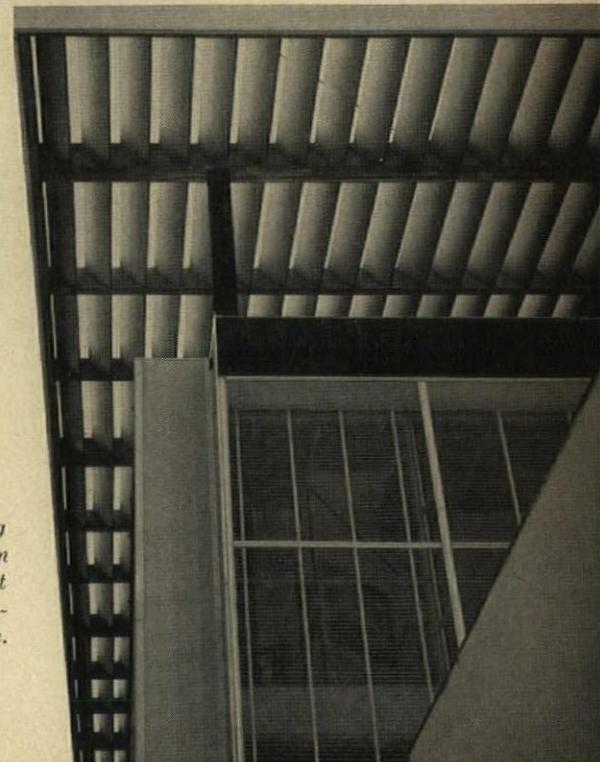
*Each elevation is different, having been designed for its orientation and special problems. Critical west wall has two sheets of glass separated by a 3' ventilated air space.*
