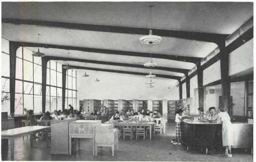
*The library, with space for 10,000 volumes, is in a wing at the rear of the administration building. The bordering landscaped patio is used for outdoor reading. Framed in welded-steel bents, the building has ceiling-height windows along the north wall; a narrow, lowered window band occurs at the ceiling line on the south wall.*
