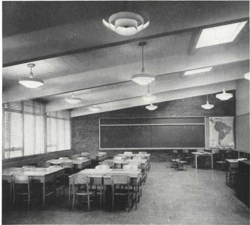
*Acoustical ceiling tile between exposed roof beams handles the sound problem very well. Tinted chalkboards get strong diffused light from roof bubbles. Note how windows rise between roof beams, to the ceiling. Classroom coat rack, in front of sinks (below), can be wheeled around and used as a screen.*
