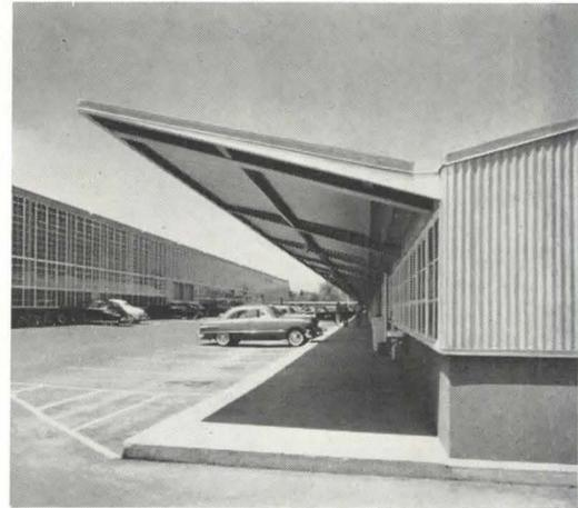
*The bold forms of the buildings are a neat translation of familiar industrial elements. In shop areas, the roof line of the shallow wing section shown above continues on up to the 26-ft height of the tall north walls. In this latter case, an intermediate skylight brings interior light to the low portion.*
