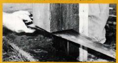
10" rotted bottoms of these load-bearing columns.
