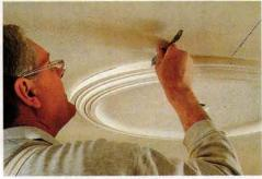
Apply plaster to seams with a paint brush as you might caulk around wood mouldings.
