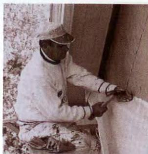
**When the paint fails, installing new canvas and rosin paper is the only solution.**
