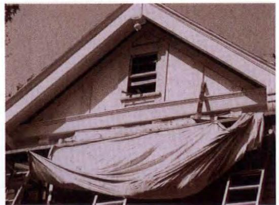
**Top:** To prevent costly mistakes, cut out windows after the canvas has been stretched over most of the gable. **Middle:** Completely tacked into place, the canvas is heavily coated with primer. **Bottom:** Once the canvas is dry, install the rakeboards to tighten it and then follow with the wood trim.
