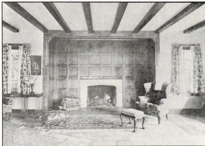
A living room in the English mode: Dark oak woodwork contrasts with the light value of trowel-finished plaster.
