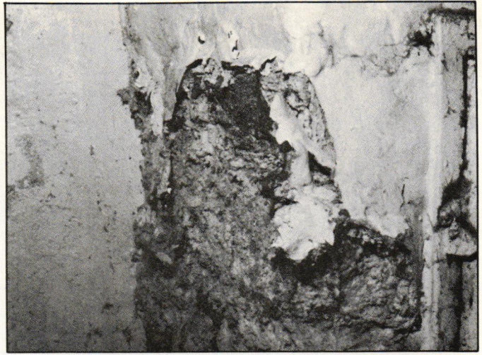
This is how the other side of the wall pictured at left looks. Paint is peeling, and efflorescence is spreading.
