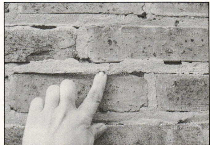
Differential expansion and contraction rates have this portland-rich mortar popping out -- and damaging the bricks in the process.
