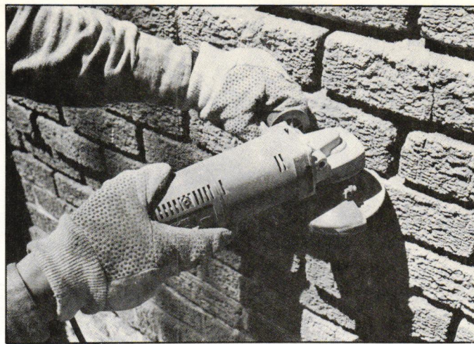
If you use a power grinder, use it on horizontal joints only. You're sure to damage the brick if you try it on the vertical ones.
