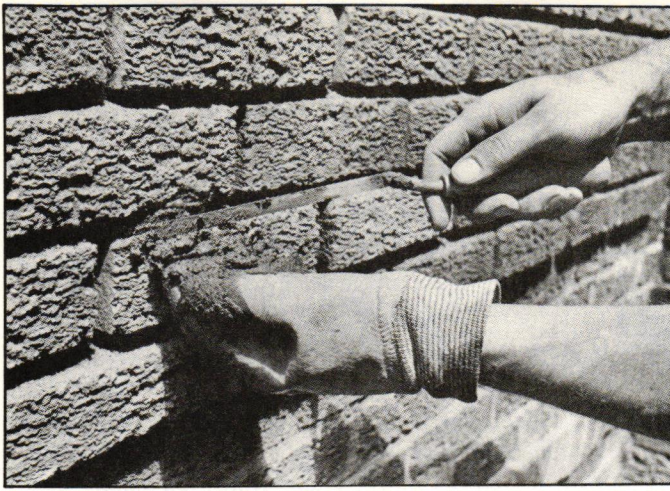
Pressing the new mortar into place. Press firmly to fill the joint completely without creating voids or air pockets.
