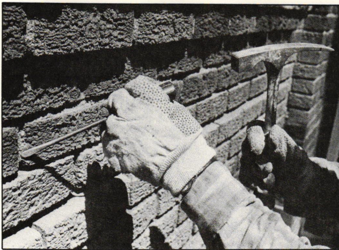
Knocking the old mortar out manually is your best bet. It's time consuming, but you're less likely to damage the brick.
