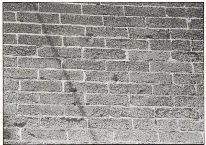
An eave overhangs this wall just a few courses above the top of the photo. The blasted bricks most exposed are "rotting" fastest.
