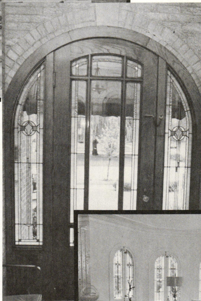
A close-up of the entry door shows a predominant muntin detail and the brick arch.
