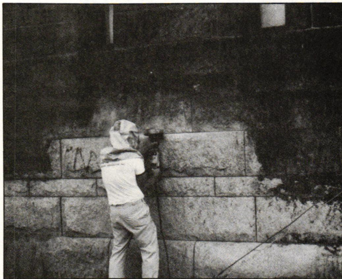
Power grinding the joints of this stone wall is grueling work. It requires steady hands and a lot of muscle.
