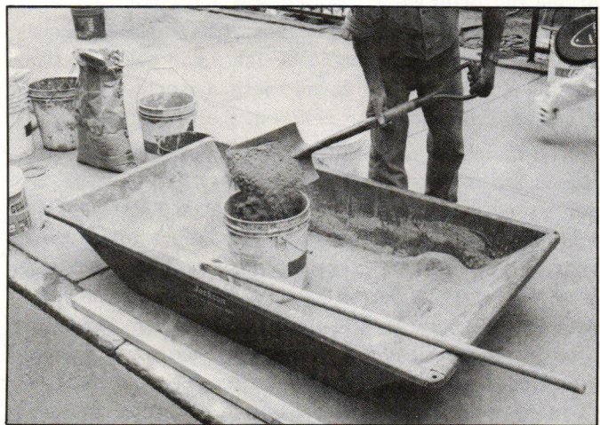
Finding the right aggregate is the only tough part in preparing the new mortar. Actually mixing it takes only minutes.
