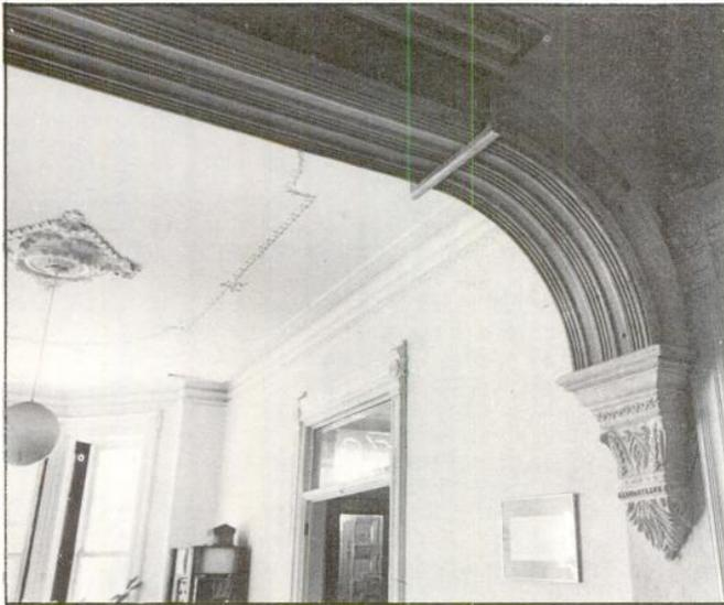
Evidence pointed to a plasterwork arch between the front and back parlors. Bill reconstructed the arch in wood with plaster corbels.
