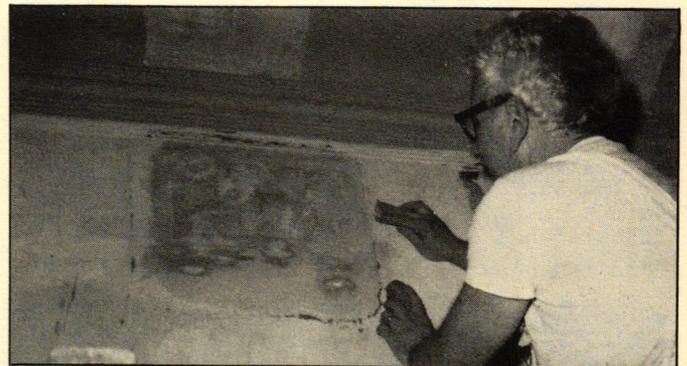
Howard Zucker, of Rambusch, has uncovered enough of the lotus flower design in the frieze to make a stencil. After removing 5 or 6 layers of paint with paint remover, until a trace of pattern appears, he then sands with very fine wet and dry sandpaper.
