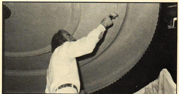
Jim Geraghty is priming the ceiling. The stencils have already been made and are ready to be applied. The tan paint is a few shades darker than the final coat will be—the way to prime when painting with colored paint.
