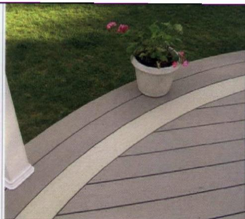
From 20 feet away, AZEK's cellular composite could be mistaken for wood with a semi-transparent stain.
