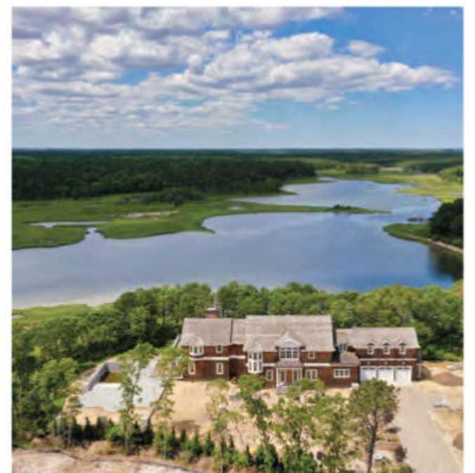
Nearing completion, private dock, Cotuit $10.5M Robert B. Kinlin 508.648.2739
