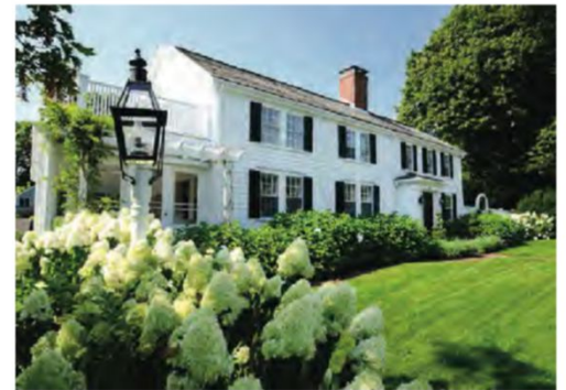
DUXBURY, MA. Water views! No detail spared! Decorator restored five bedroom Antique Colonial with private master suite offering 30' deck views. Open living with French doors to screened porch. Cherry study with fireplace and custom details. $1,649,000
