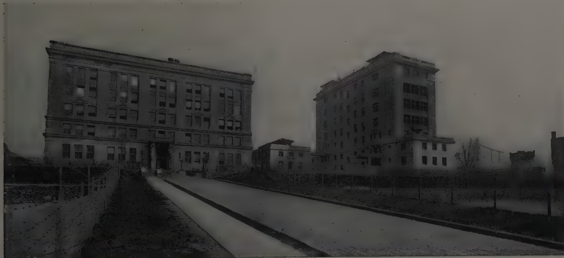
GENERAL VIEW, ROCKEFELLER INSTITUTE FOR MEDICAL RESEARCH YORK & SAWYER, ARCHITECTS
