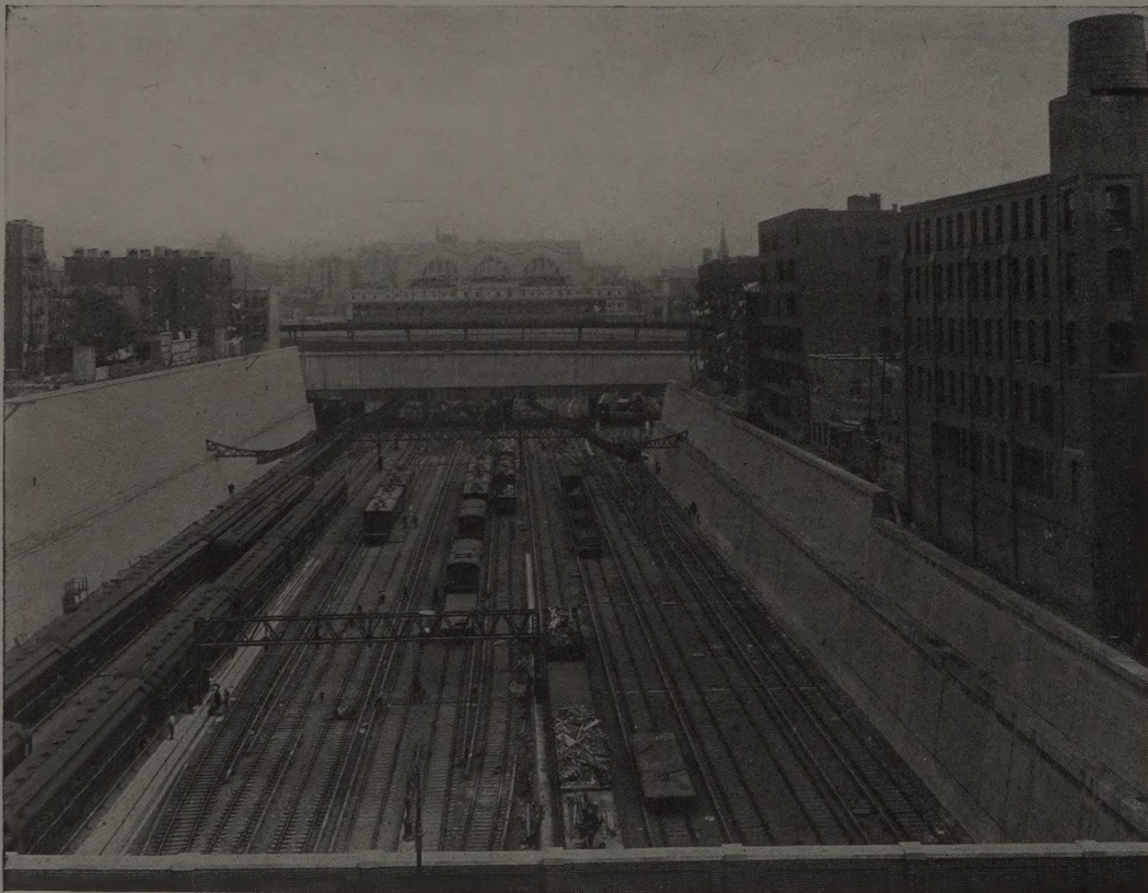
TRACKS, WITH STATION IN THE DISTANCE
