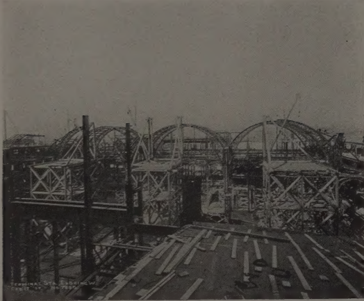
CONCOURSE ROOF, DURING CONSTRUCTION LOOKING WEST
