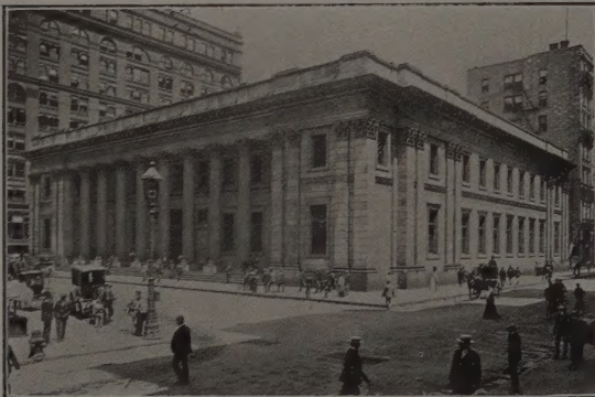
D. H. BURNHAM & CO., ARCHITECTS ILLINOIS TRUST AND SAVINGS BANK, CHICAGO, ILL.
