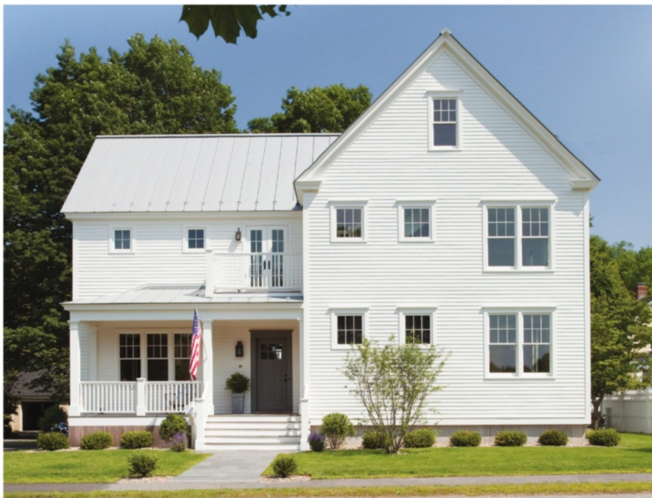
A simple farmhouse sits in a suburban area in Massachusetts.
