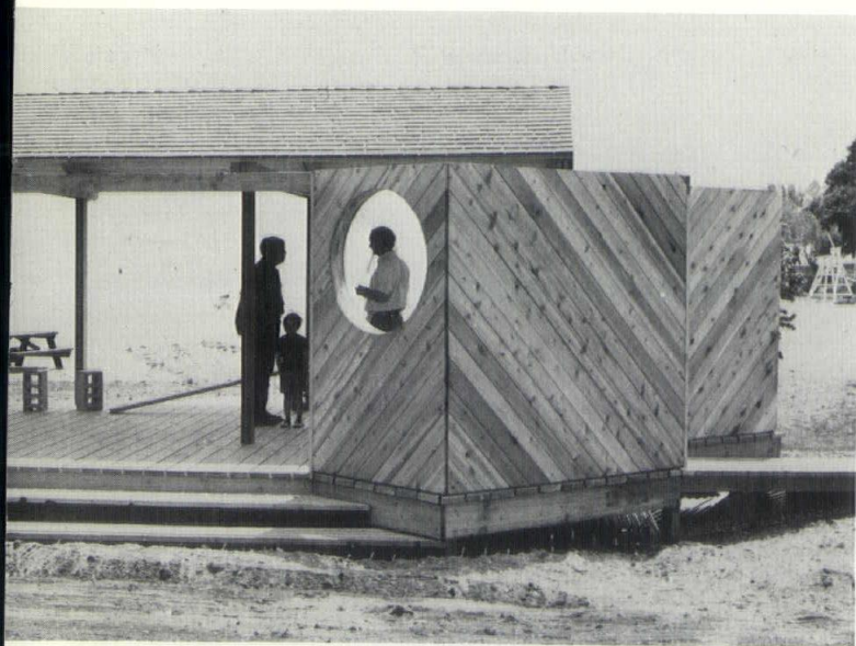
The pavilion, open to the view but designed to protect the beachgoer from sun and wind, stands on the eastern back corner of Jacob's Beach, and the service building, with insets for such "necessities" as vending machines and lifeguard apparatus stands opposite on the western corner.
