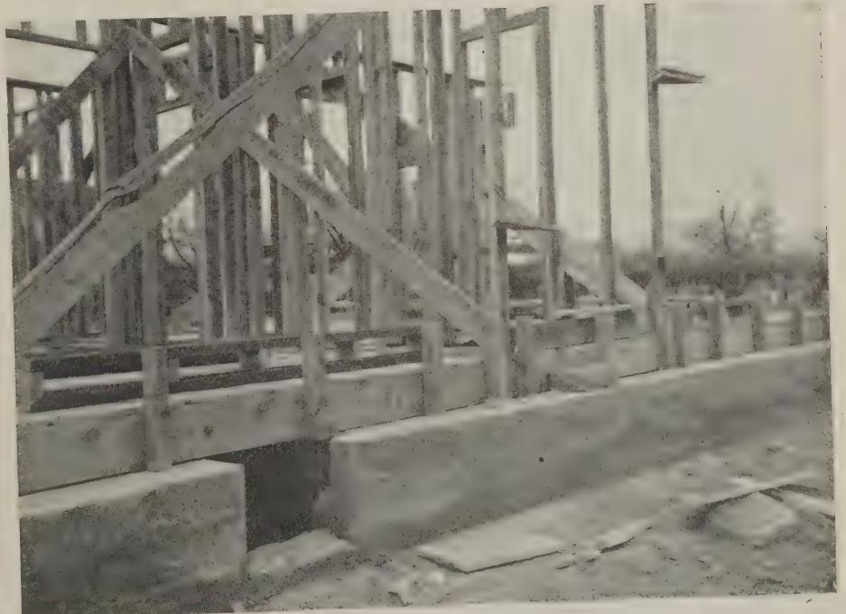
Fig. 12—A "close-up" of the framing shown in Fig. 2. The wings projecting from the stud at the extreme right fit into the wall and serve to hold the partition
