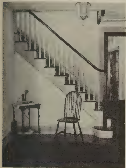
Combination stair, accessible from both front and rear of house
