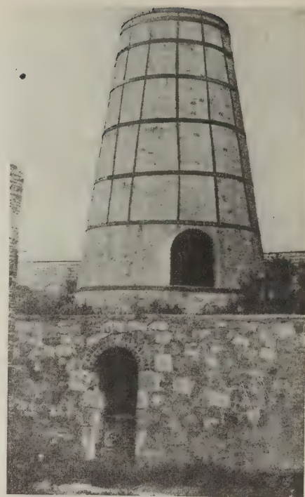
Kiln made by Joseph Aspdin, the British inventor of portland cement
