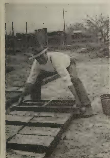
Fig. 7—Lifting the mold from the mass of clay
