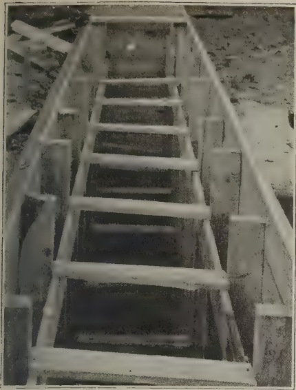
Inside formwork in place
