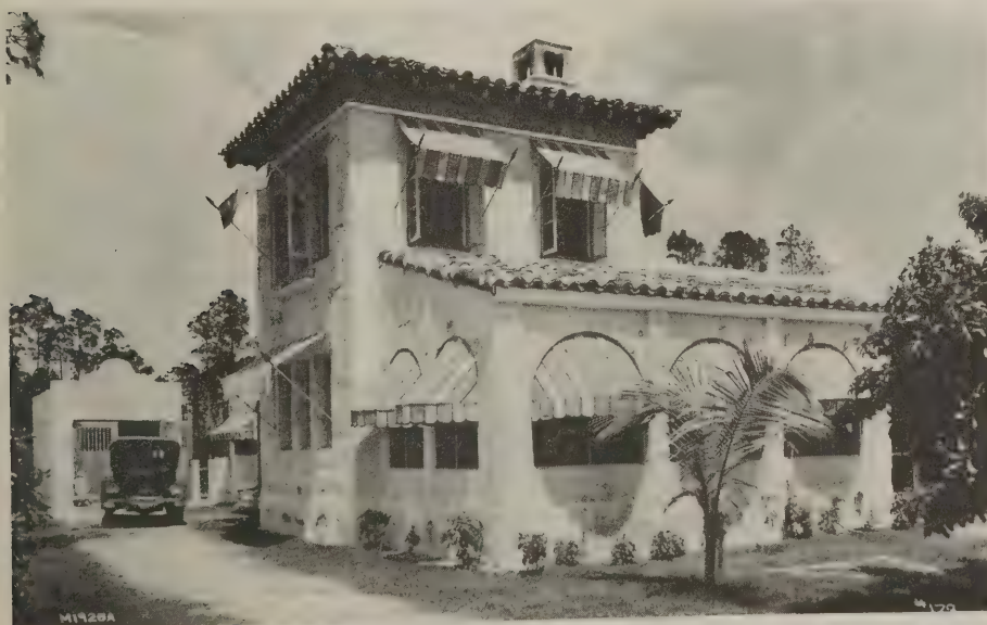
Patches of brickwork, only partially covered with stucco, show through in this wall. Note the decorative frieze of colored stucco under the cornice
