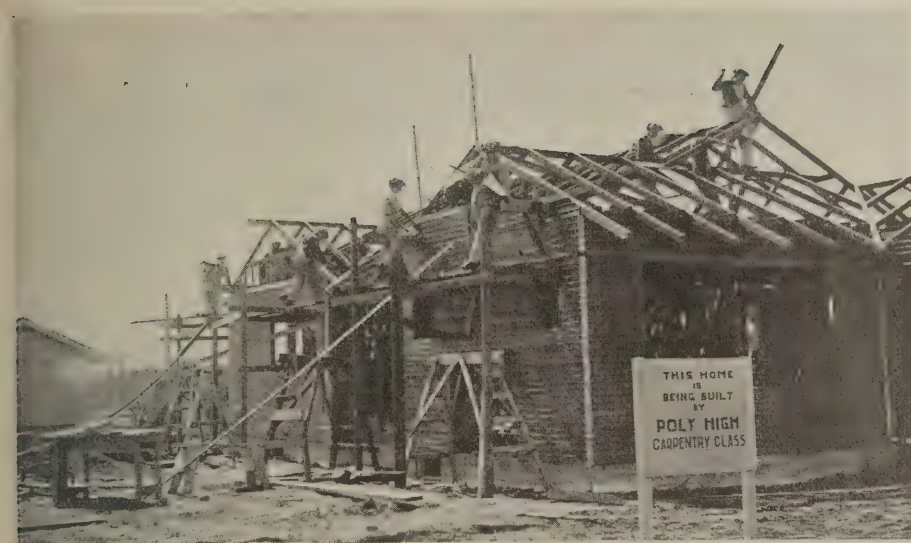
Framing a roof is good practical experience for any boy
