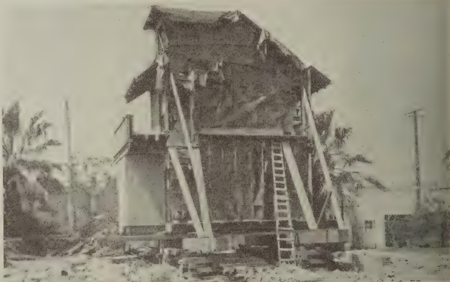
A view of the second section. This section was so high in proportion to its width that there was danger of its tipping unless it was properly supported. In order to brace it and prevent it from toppling over, the beams upon which it was carried were made extra long and joists run from the extremities of the beams to points on the house, thus holding it securely
