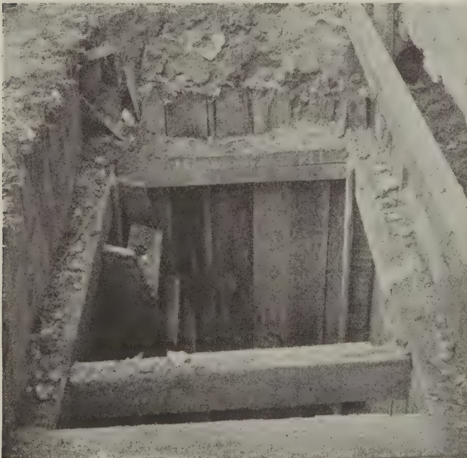
View of one end of the well. Notice how the wale timbers keep the sheet piling from caving in
