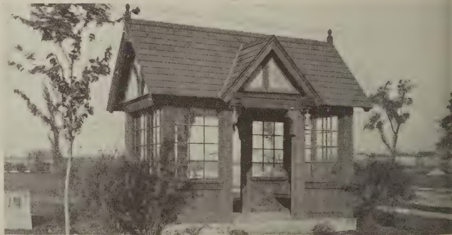
People waiting for the trolley cars find shelter in this little building, whose design is reminiscent of old English half-timber garden houses
