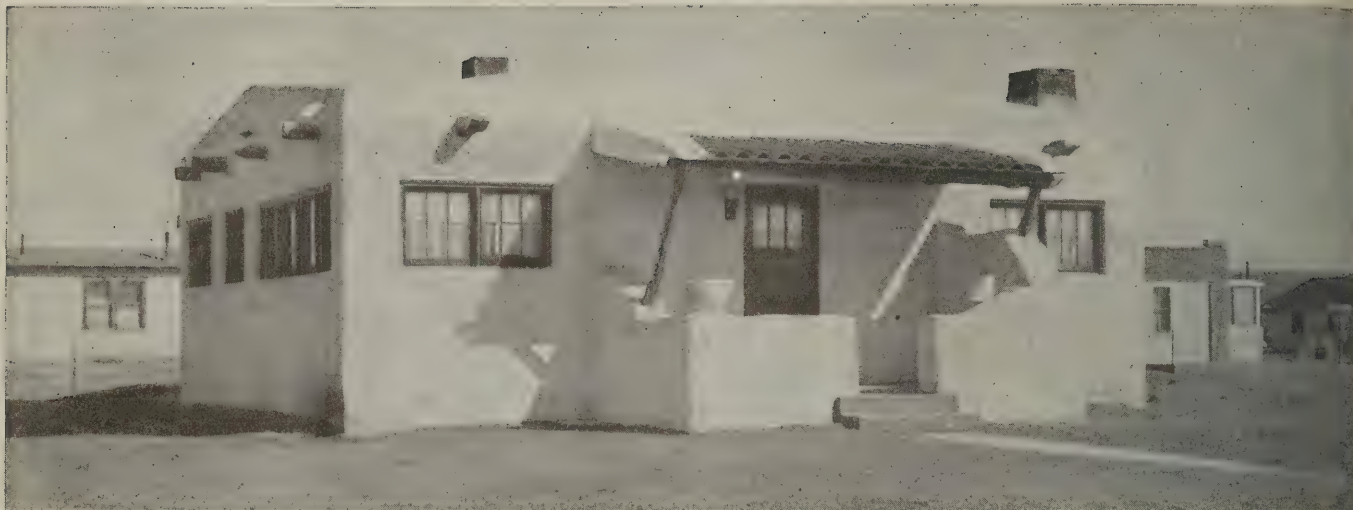
Fig. 1—Here is a type of construction that is literally of the soil
