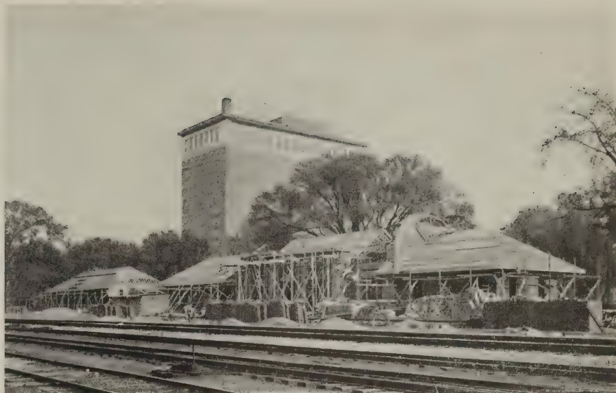
Fig. 4—View showing station under construction
