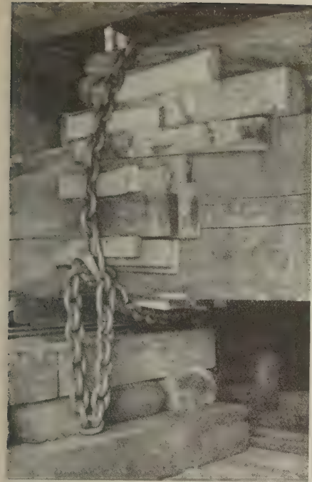
The separators, used to prevent lateral movement of the longitudinal timbers, were firmly chained to the 16x16s which carried the entire load, and the chains were tightened by driving wedges between the chain and the timber
