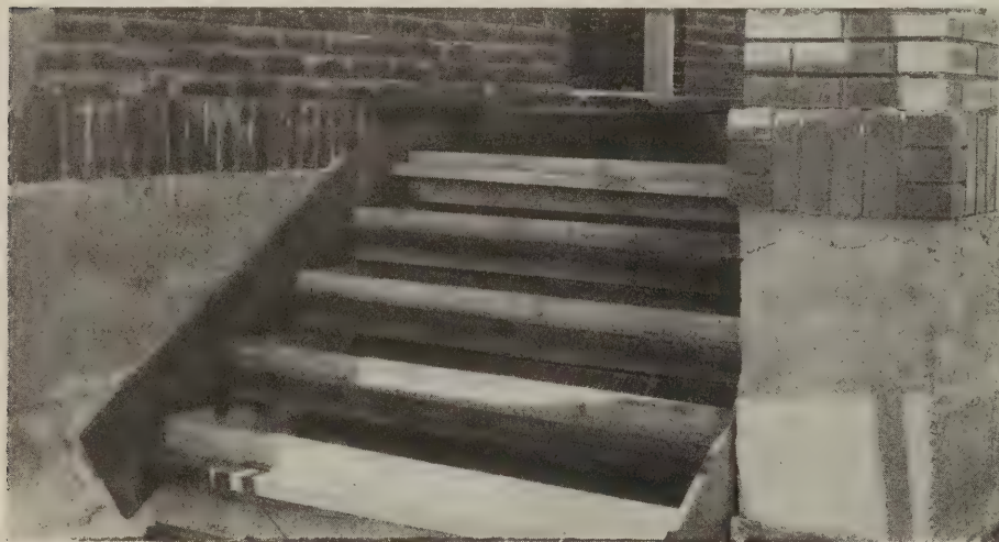
It is not necessary to cut expensive stringer forms for these concrete steps
