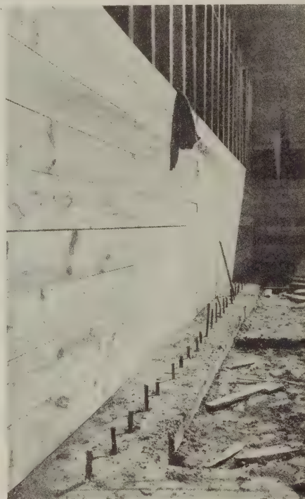
These rods sticking up above the foundation form a base to which the reinforcement rods in the wall may be wired to hold them in place
