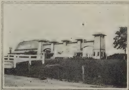
Main entrance. Ramp guard rail at left for tunnel under interurban tracks
