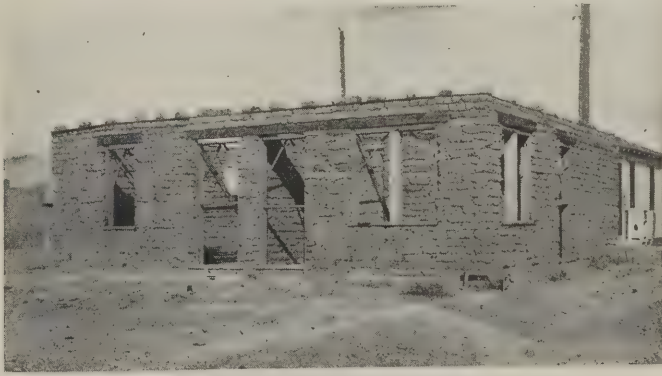
Fig. 3—An adobe house with walls erected. Note weather protection at top course
