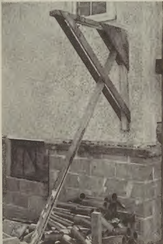
Detail of bracket and method of support
