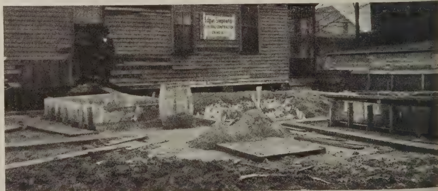
This shows how part of the excavation has been utilized to provide a storage space for mortar
