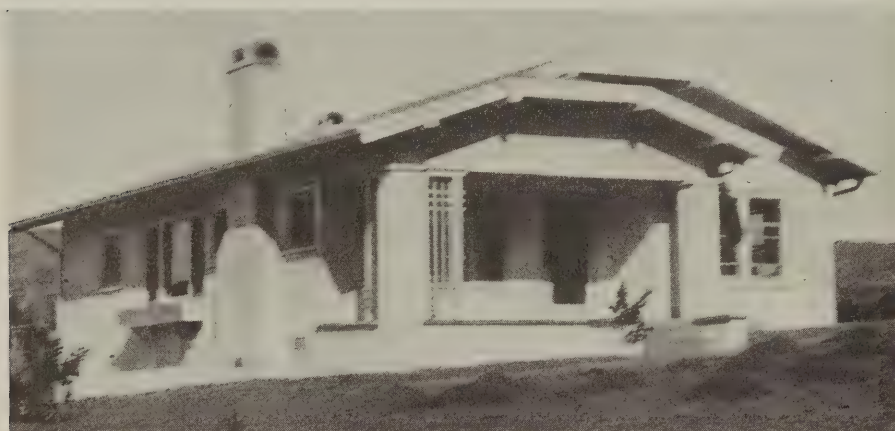
Home of A. N. Phillips at El Cajon, California, built according to the method described in this article
