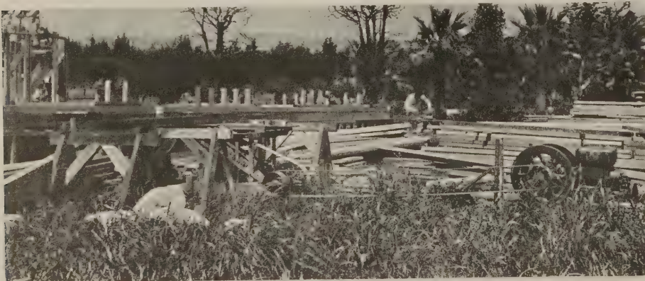
A general view of the plant showing saw, table, and engine
