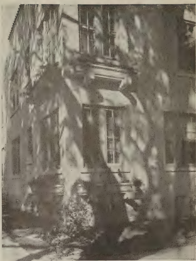
Detail at corner
