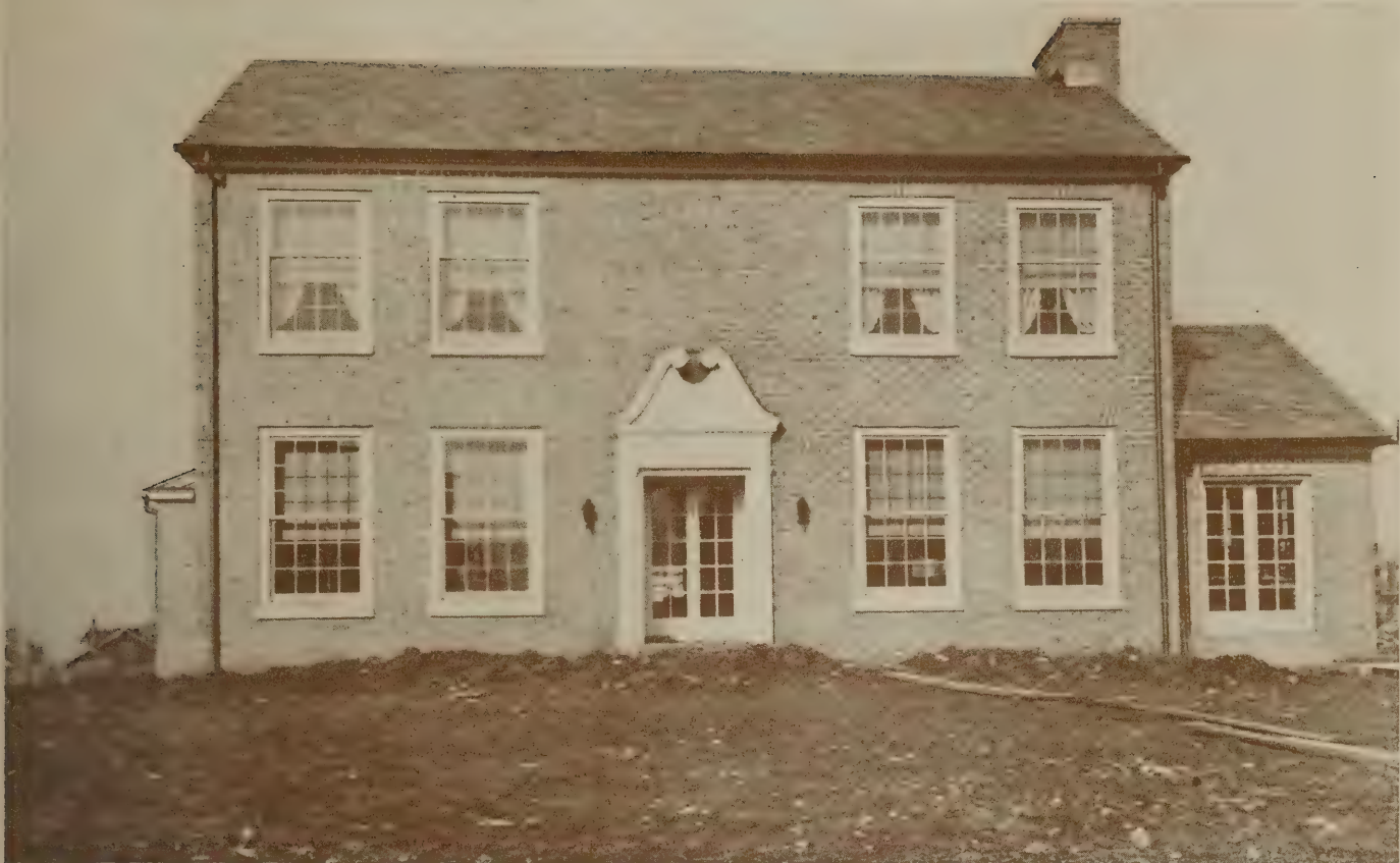
The use of French doors at the entrance is unusual but pleasing
