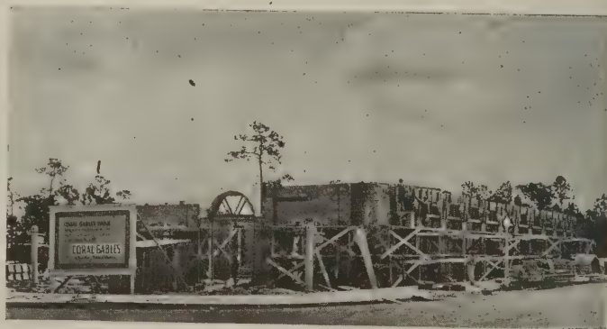
The Coral Gables Bank and Post Office under construction
