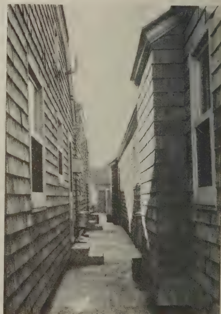
View between buildings. The cement floor is carried from wall to wall
