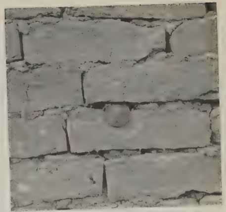
Fig. 10—Bolt used for holding partition. Notice that the adobe thru which it passes has been chipped so that the bolt head will be covered by the stucco
