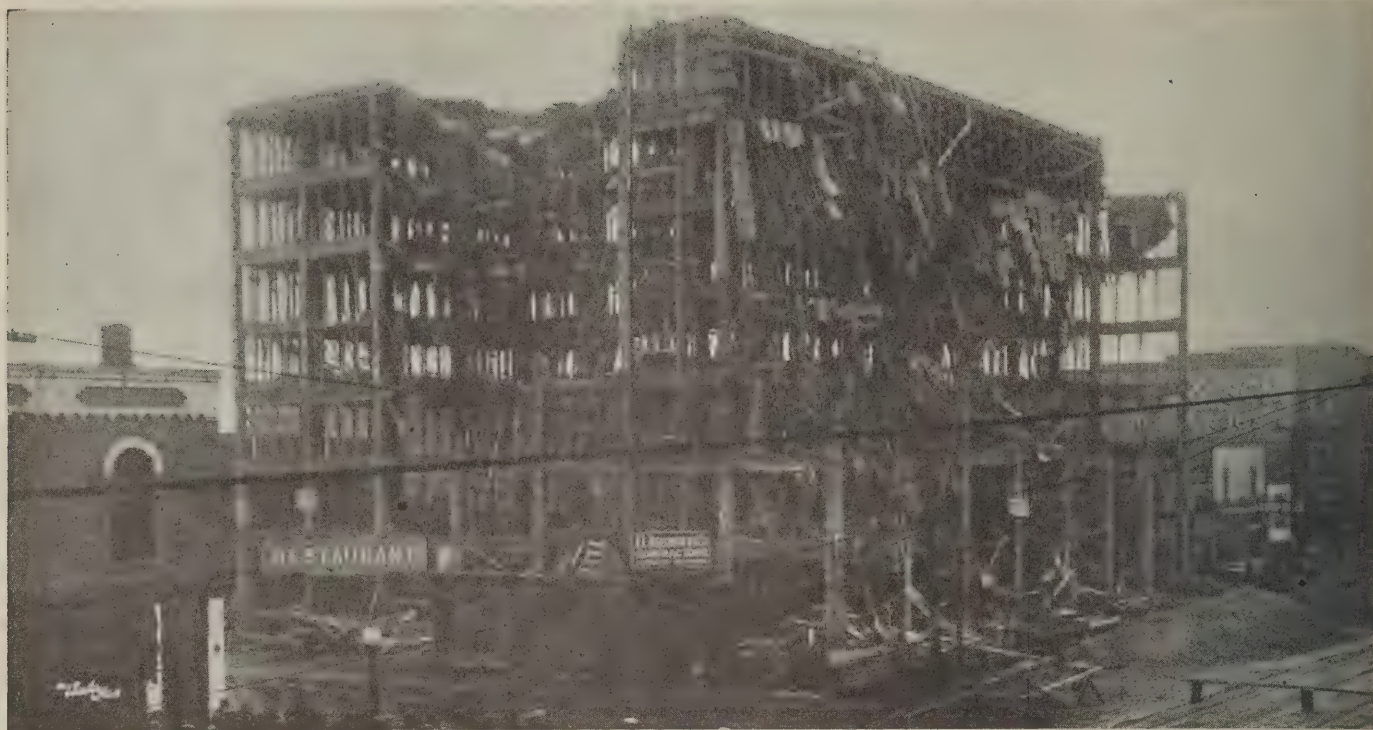
Fig. 1. This photograph was taken about fourteen hours after the collapse started. Notice the concrete hanging by the reinforcing on the upper floors
