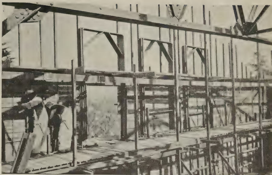
View of the top of the scaffolding showing false frames set in place to allow for window opening
