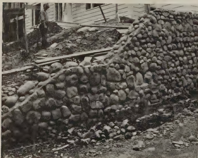
Face of wall
