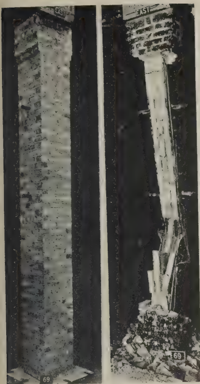
Brick protection before and after tests
