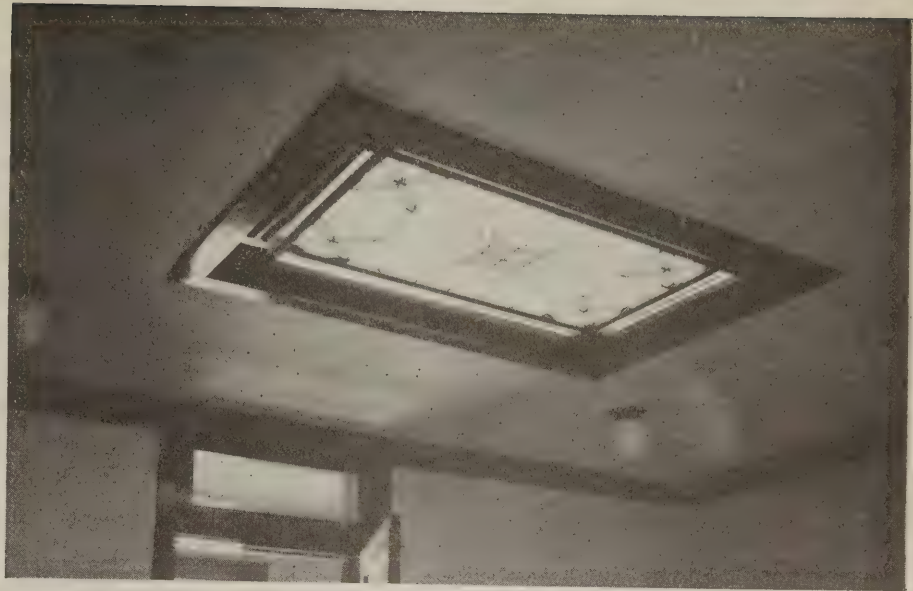
This is a view of the underside of the skylights which provide light for the office reception rooms
