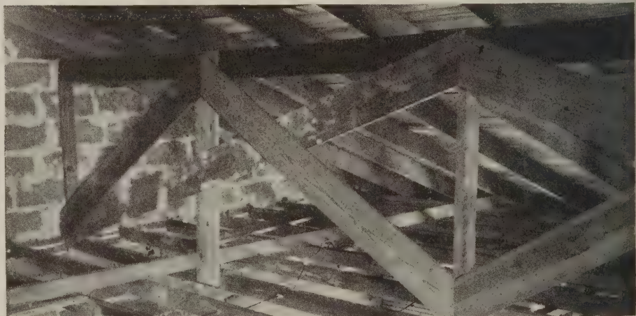
This truss was used to help support a roof where the rafters were of exceedingly long span. The truss was placed at the mid-point of the rafters
