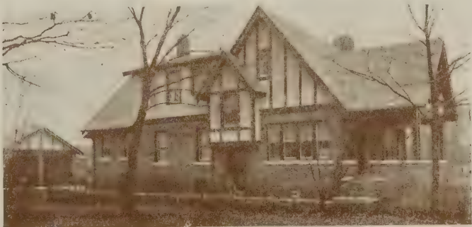
Rear view, showing the sun room, the stairway projection, and the dormer that provides windows for the bathroom and rear bedroom
