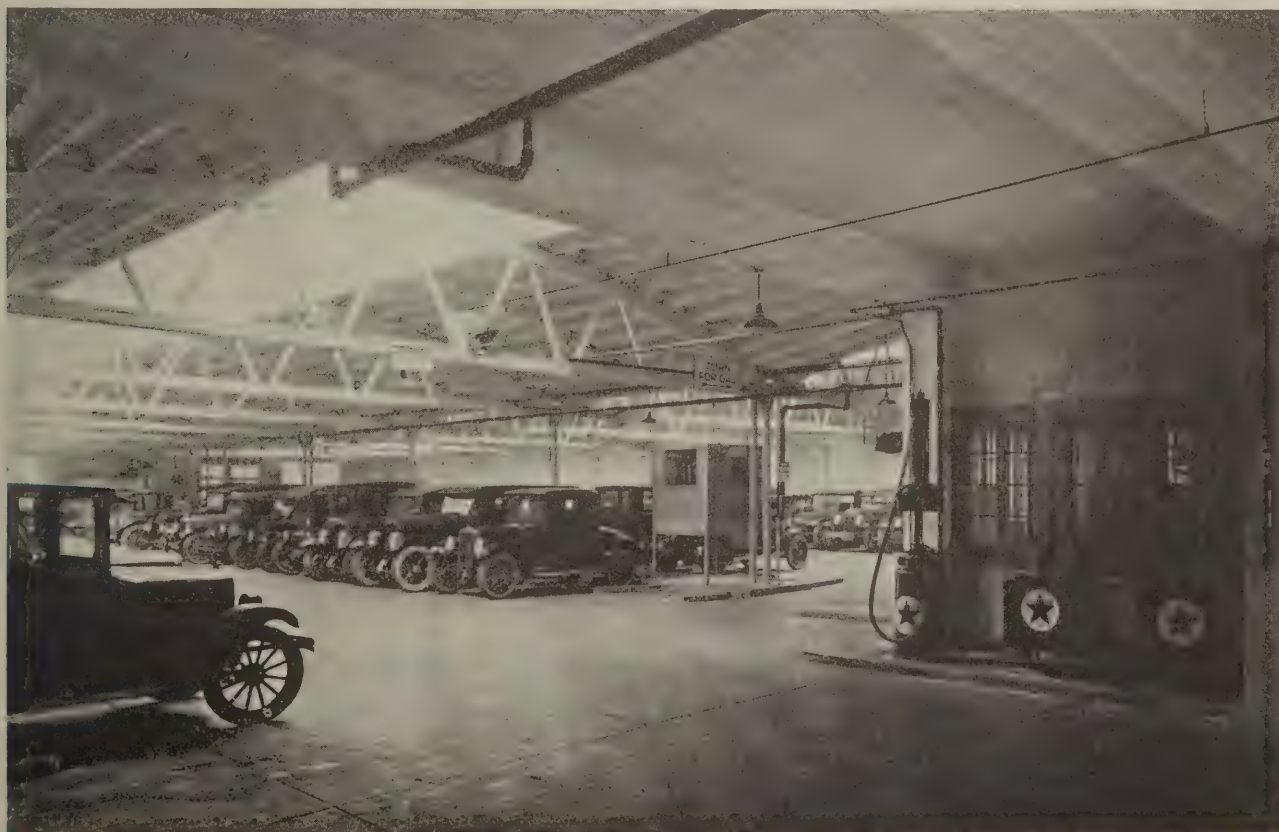
The car stalls are divided by concrete curbs and they slope to the rear so that cars may coast into position
