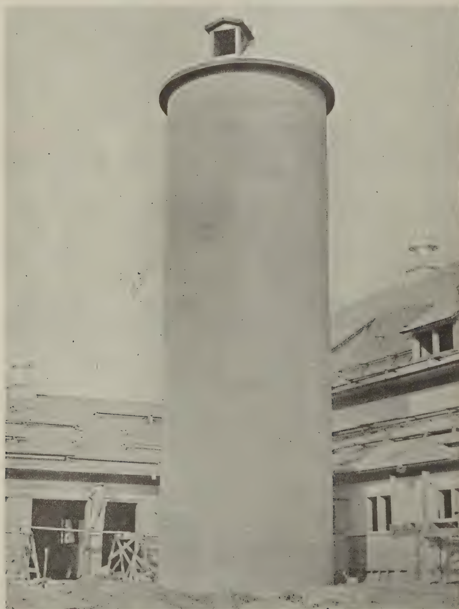
A monolithic reinforced-concrete silo on the farm. The opening at the top is where the silage is taken in
