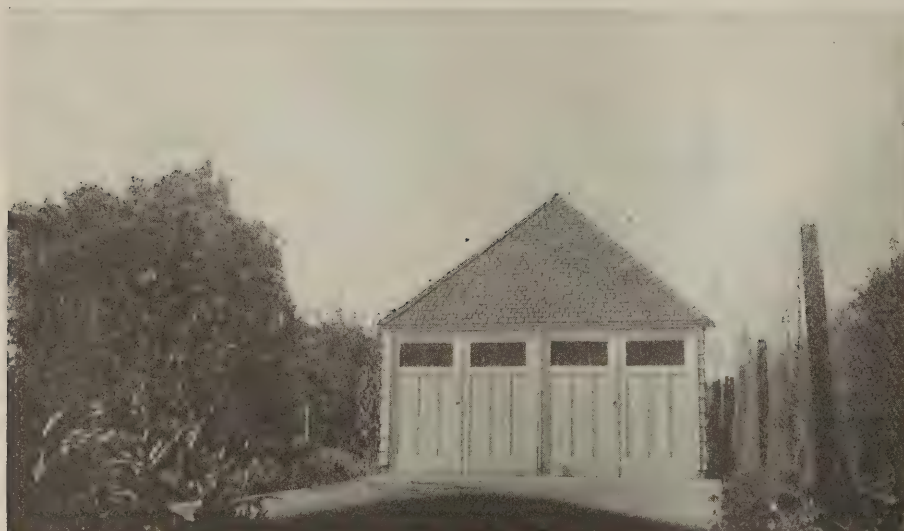
In this detached garage, the designer, Ernest Irving Freese of Los Angeles, has used a high pitched roof and clapboarded walls, conforming to the treatment of the house, and thus bringing the two into relation
