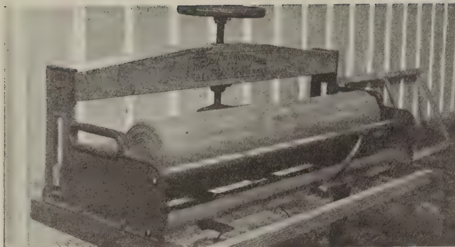
Front and rear views of a screen wire stretcher manufactured and sold by J. E. Donaho, of Milton, Iowa
