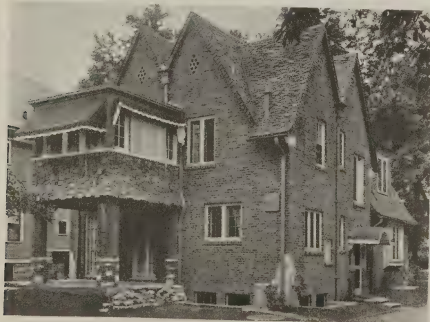
A view of the rear showing the added porch
