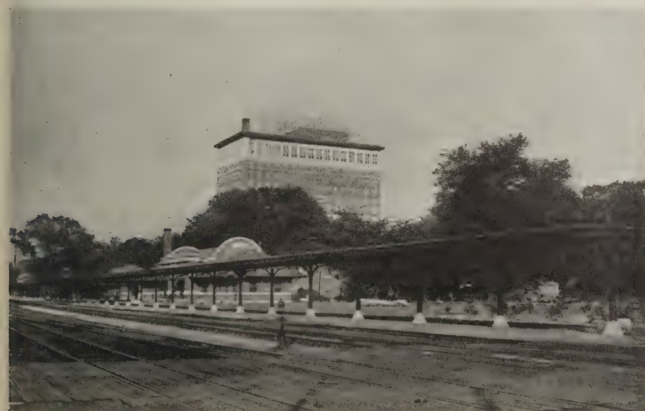
Fig. 5—View showing platform canopy
