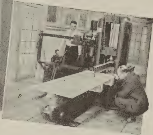
Laminex doors being tested for strength of panels in 200,000 pound Olsen testing machine.
