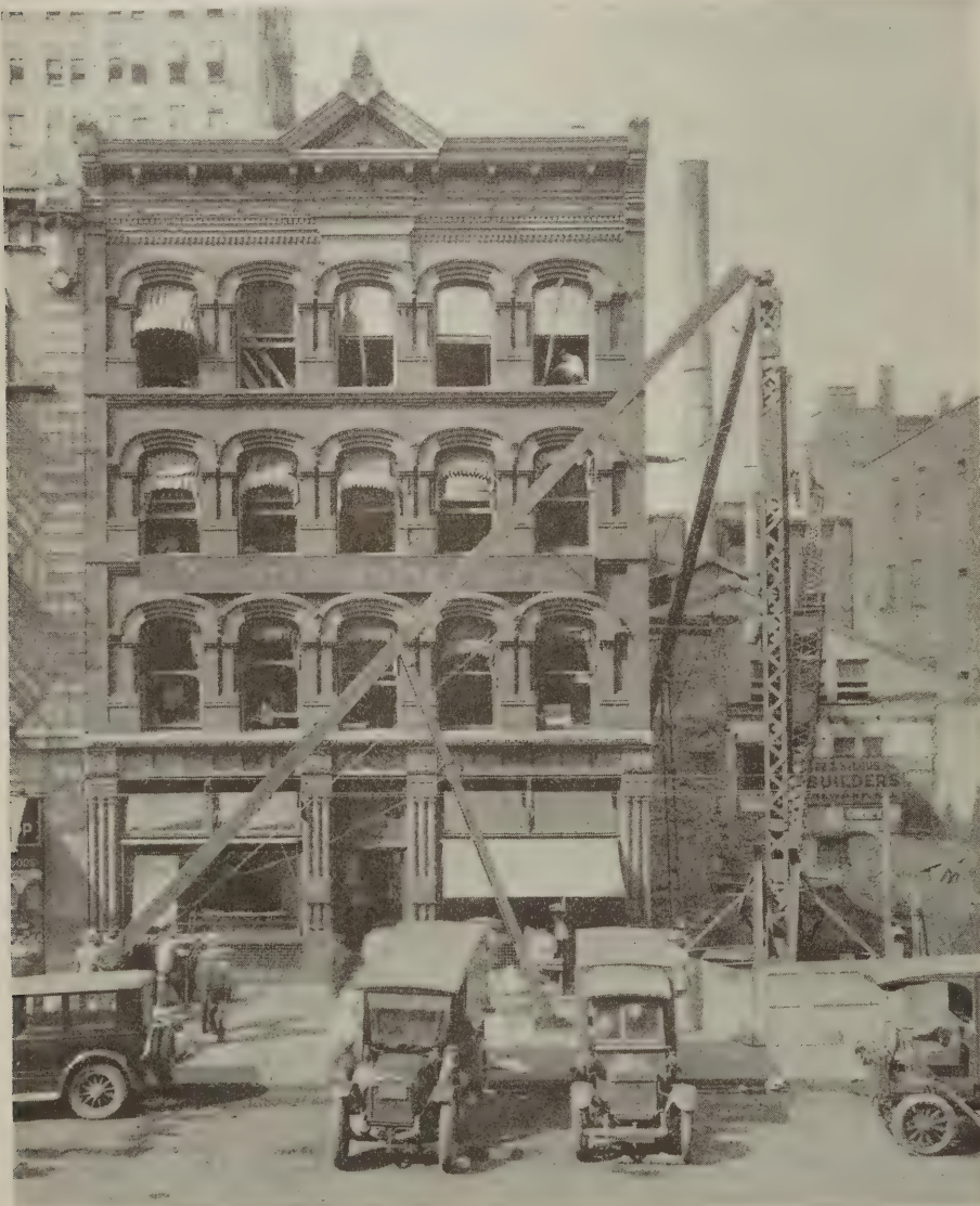
A general view of the job. Notice that the derrick leg across the face of the building is so arranged that the entrance is unobstructed
