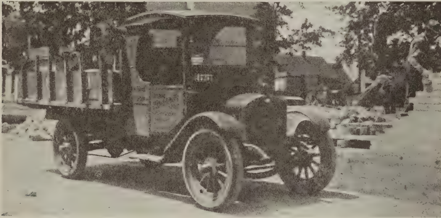
Fig. 1—A "general purpose" contractor's truck, having a body with removable sides, which permits hauling bulky concrete forms
