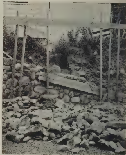
Formwork for face of wall
