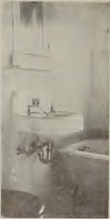
Tub enclosure and floor are of magnesite cement
