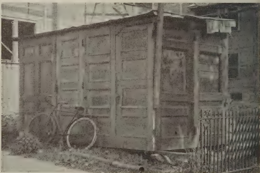
These old doors are nailed together to make a contractor's shanty, thus saving the lumber which would be required for this purpose
