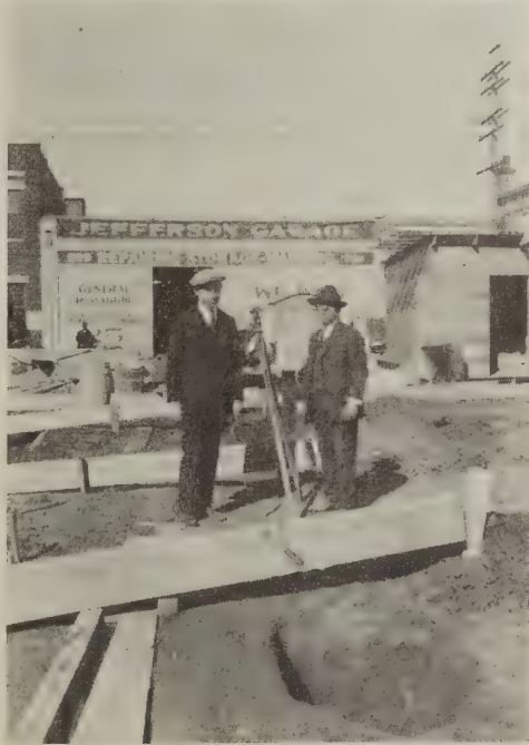
Singer (left) on the level with W. A. Rogers of Rogers & O'Rourke, builders, of Dallas
