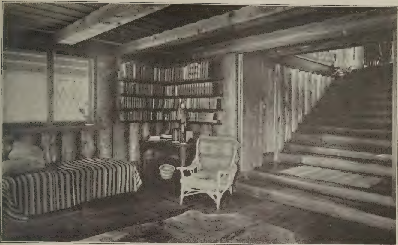
The main stair, leading from the living room to the corridor above, is built up of solid logs, roughly hewn to form steps. Note the full-framed construction of the ceilings with heavy timberwork left exposed
