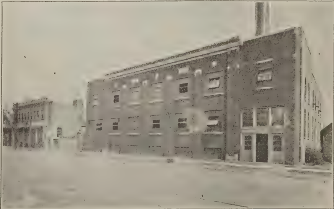
An electric power station helps to swell the total
