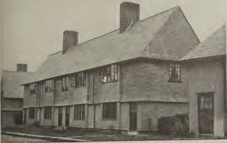
Upper story of slate, broken by stucco panels
