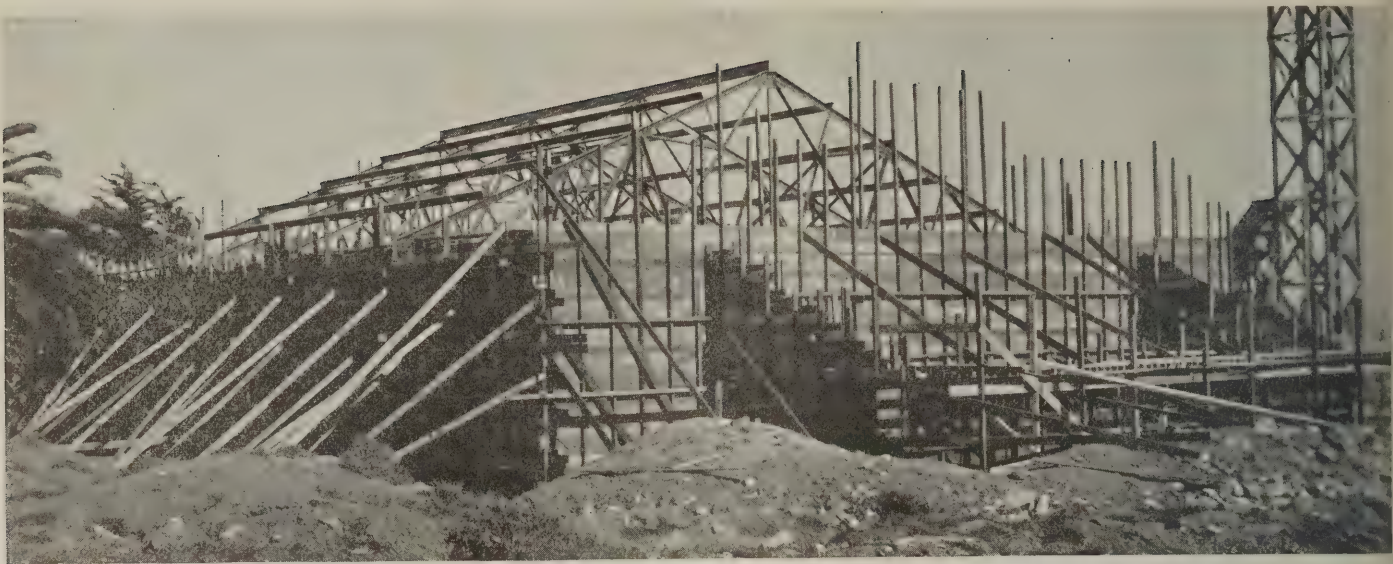
A general view of the job showing forms in place for the walls
