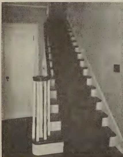
A straight flight. Open rail at bottom, closed in near top
