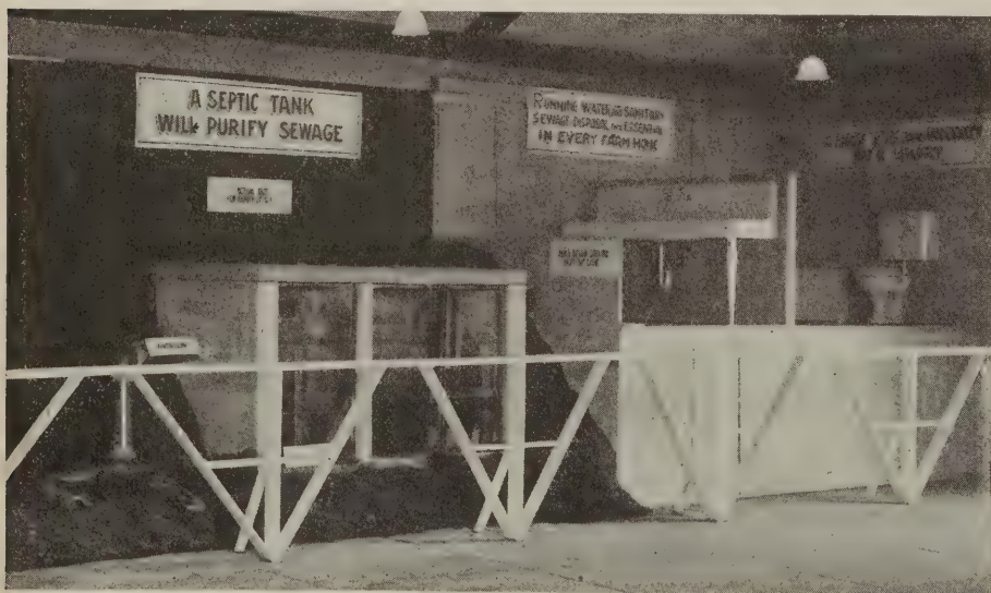
An exhibit of a septic tank showing the two chambers, tile distribution system and the siphon. The sides of this tank are of glass so that the action of the tank may be watched
