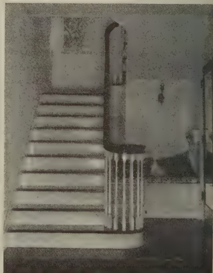
Stair with starting volute and continuous handrail
