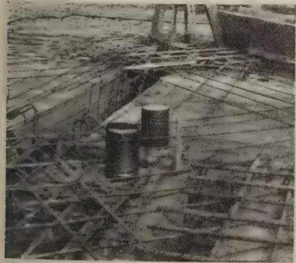
Fig. 5—Ordinary stovepipe used to form openings in floor slabs
