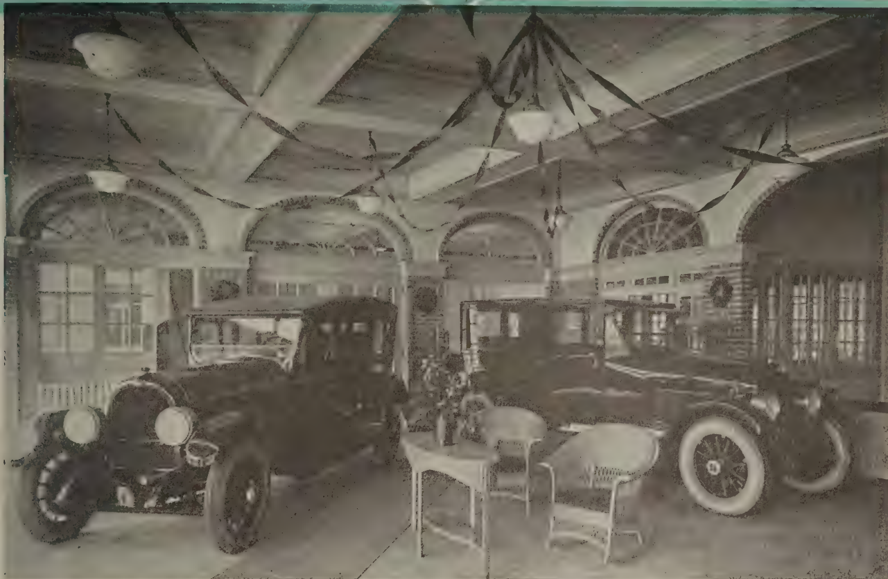
The walls of the display room are glazed so that the displays may be viewed from either without or within the building
