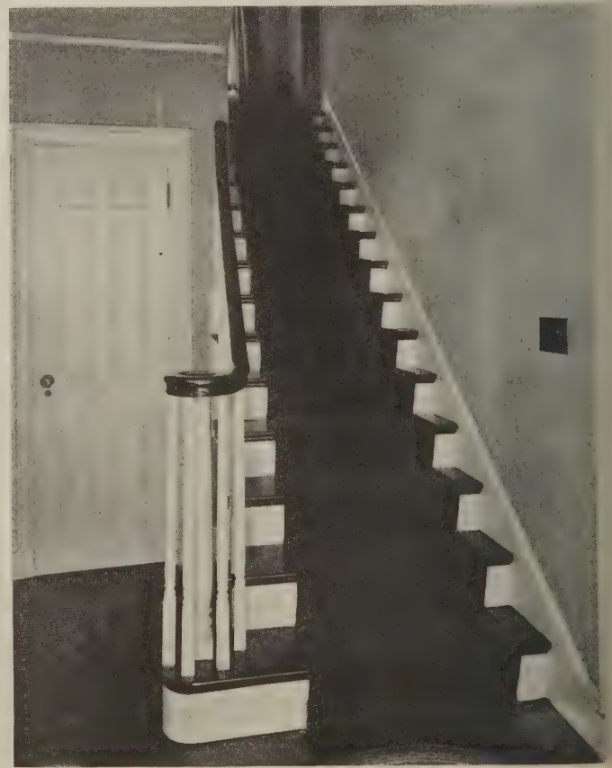
This is a straight flight stair, partially enclosed between walls
