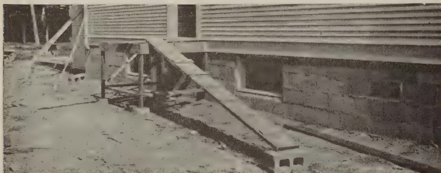
This plank walk cannot slip and cause the injury of a workman
