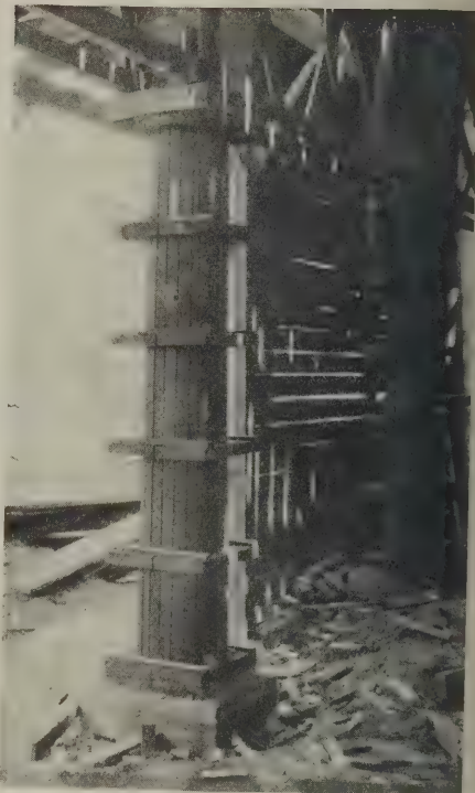
The collars hold the long pieces together
