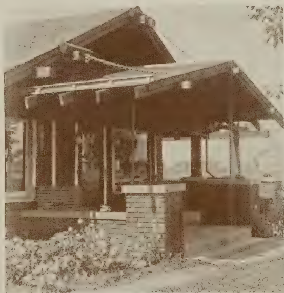
Detail of front porch. The use of iron posts avoids the heavy appearance of oversized wood members
