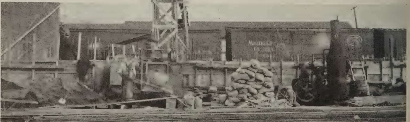
Fig. 3—The materials are grouped so that there is no confusion when charging the mixer
