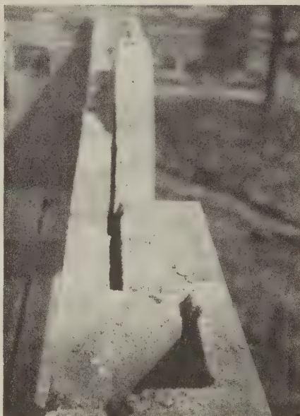
View of the double walls under construction, showing continuous air space. The decorative facing is plainly visible on the units in the outer wall
