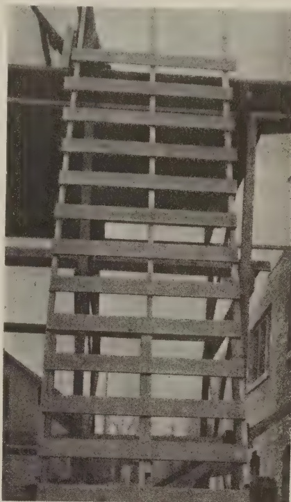
By means of this ladder two men can be accommodated at the same time
