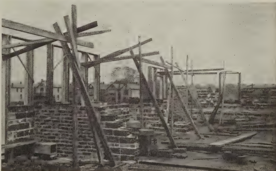
Window frame bracing that does not block the job, but assures well-plumbed frames, which make sash fitting easy. Notice the bracing system which seems to be very carefully and logically worked out. Notice also that plenty of working space is provided between the braces so that little interference is given the bricklayers who may be working on the wall
