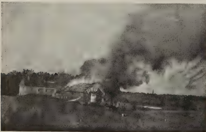
This farm house was rodded but the barn was not. Lightning struck the barn. The ensuing fire destroyed the house as well as the barn. Lightning rod protection must be complete to be effective
