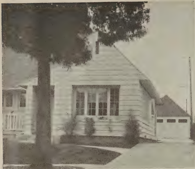
Flower boxes are built-in beneath the deeply recessed windows
