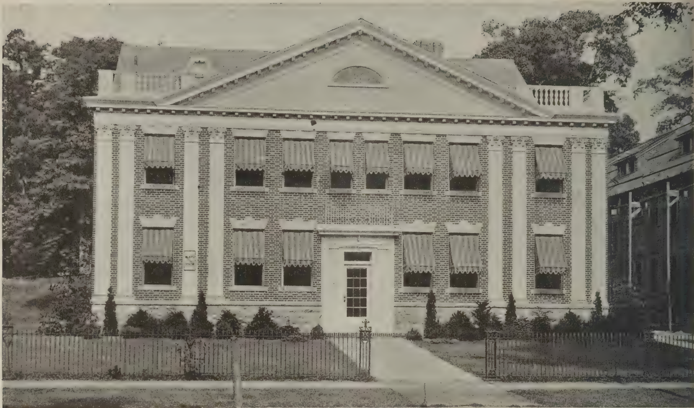
Remodeled apartment building in New Haven, Connecticut. Jacob Weinstein, New Haven, Architect
