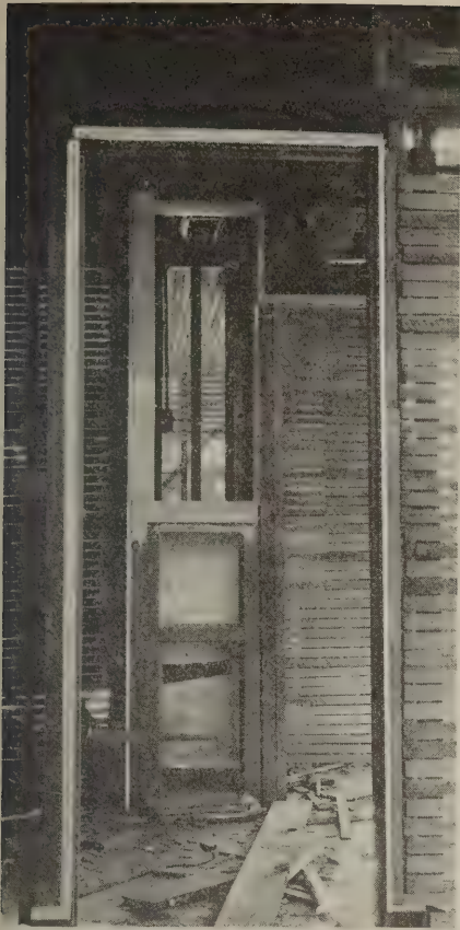
Showing galvanized iron plaster stop around a door opening
