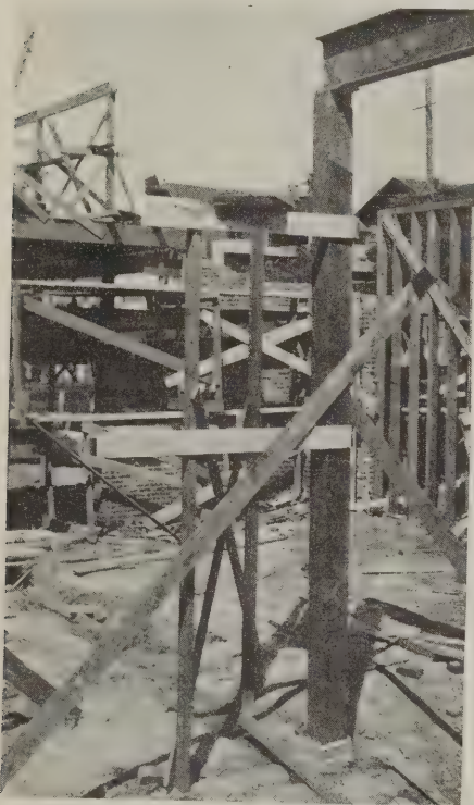
This platform gives the steelworker a place to stand
