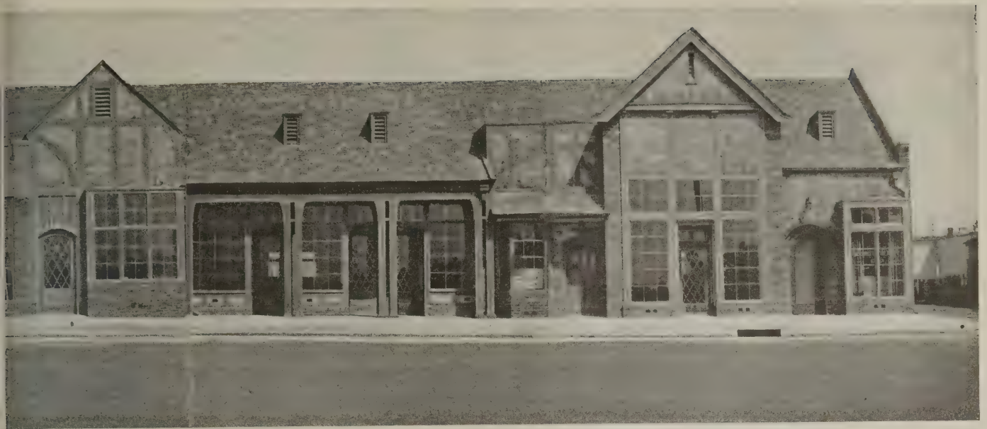
A view showing seven stores forming the right-hand portion of the group
