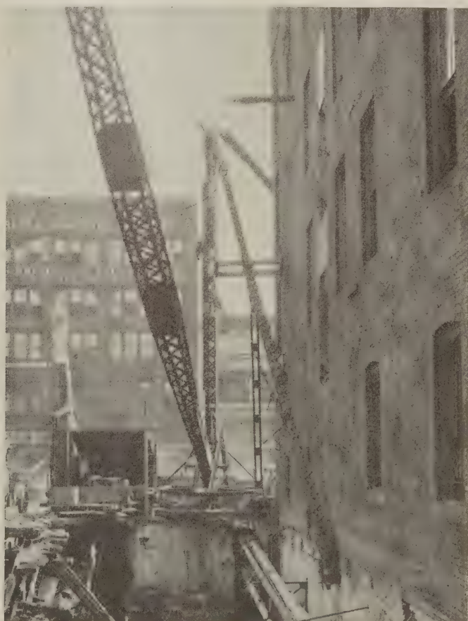
View of the derrick and power plant. The leg extending into the excavation is fastened to a pin fixed in the wall
