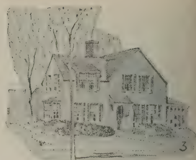
Fig. 3—Completely altered by a wing at the left and a sun parlor at the right
