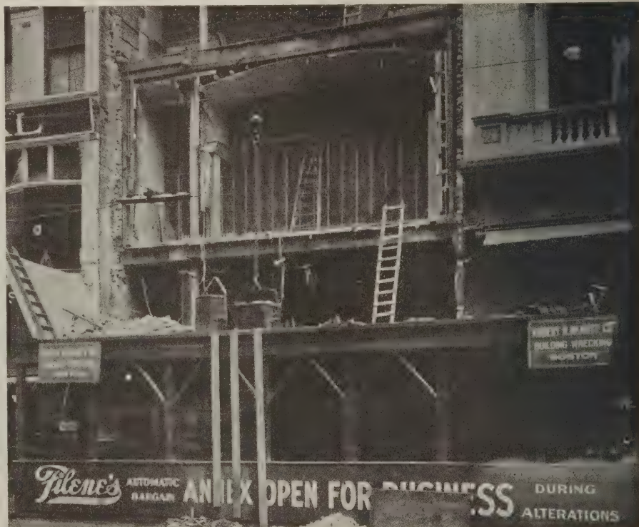
Temporary partitions were built in a short distance from the front wall before the work was started
