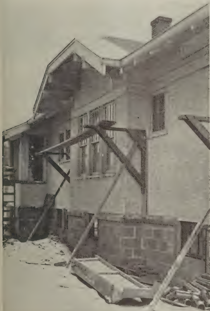
Scaffold support for finished walls
