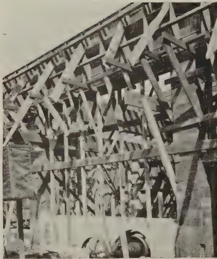
Close-up of formwork. The parapet is braced by diagonals attached to the shores
