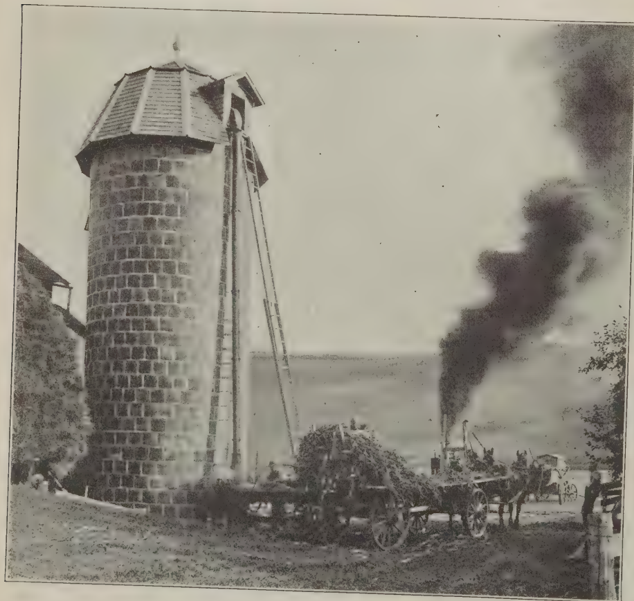
Fig. 1—A hollow tile silo on a farm
