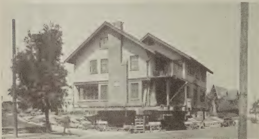
Here is the first section of the house partly moved off the lot. When left to stand over night it was not considered safe enough to leave the house without any support except the rollers so it was braced by building up cribbing at each end of the longitudinal beams, setting a couple of screw jacks on top of the cribbing and tightening up on the jacks to make the cribbing take part of the load. In the morning when the moving was ready to begin, the jacks and cribbing were taken down
