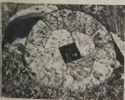
In the early days the rock for portland cement was ground between crude millstones
