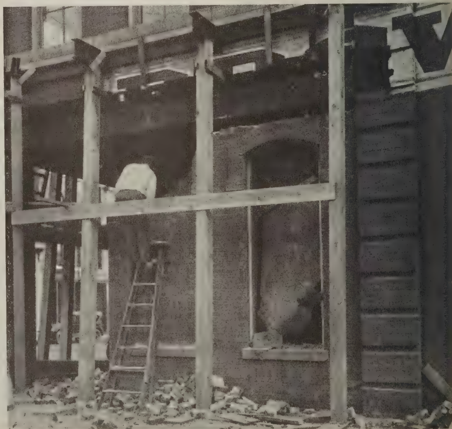
View showing method of supporting stone sill from I-beam
