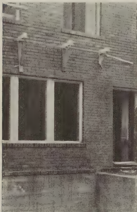
This illustration shows the reinforced-concrete flower box supports in place, and the brackets used to hold them until they are strong enough to sustain themselves. Notice the bracing used to prevent shifting of the brackets
