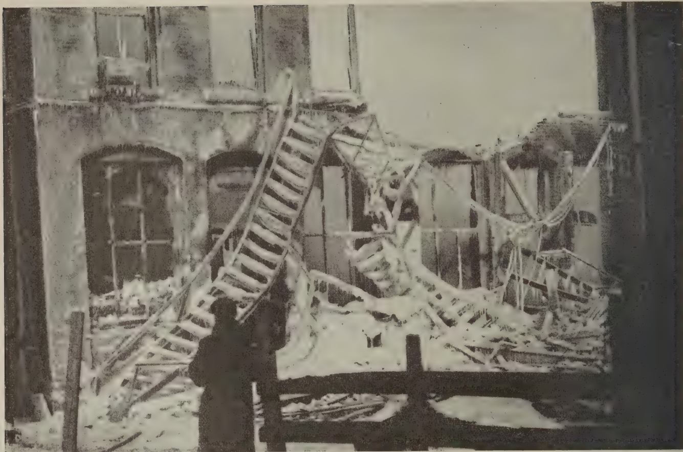
Eleven people were killed in this recent Montpelier, Vermont, fire. Note the condition of the fire escape
