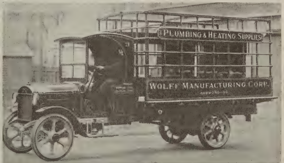
Fig. 5—High stake body suitable for light bulky materials such as frames, crated materials, etc.
