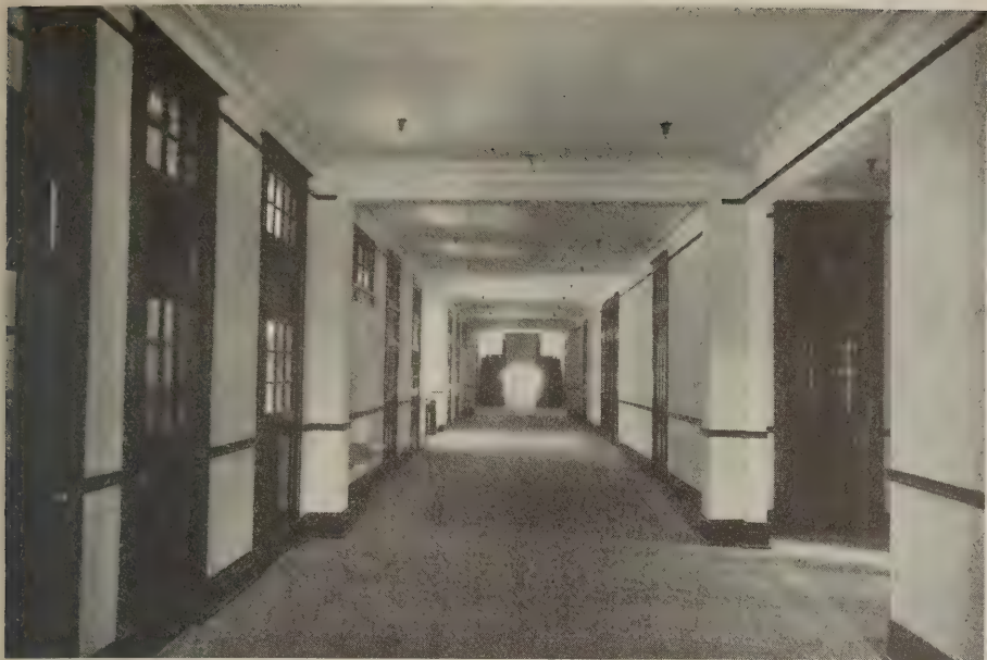
Fig. 5—There is no danger of fire panic in this wide, sprinkler-protected corridor
