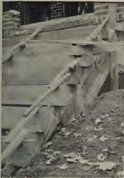
The riser forms were nailed to ears projecting from the stringers
