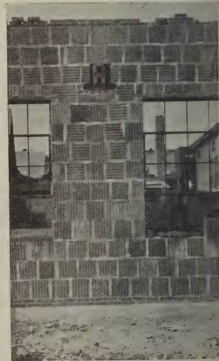
The other side wall is entirely built-up with only the truss seat left open
