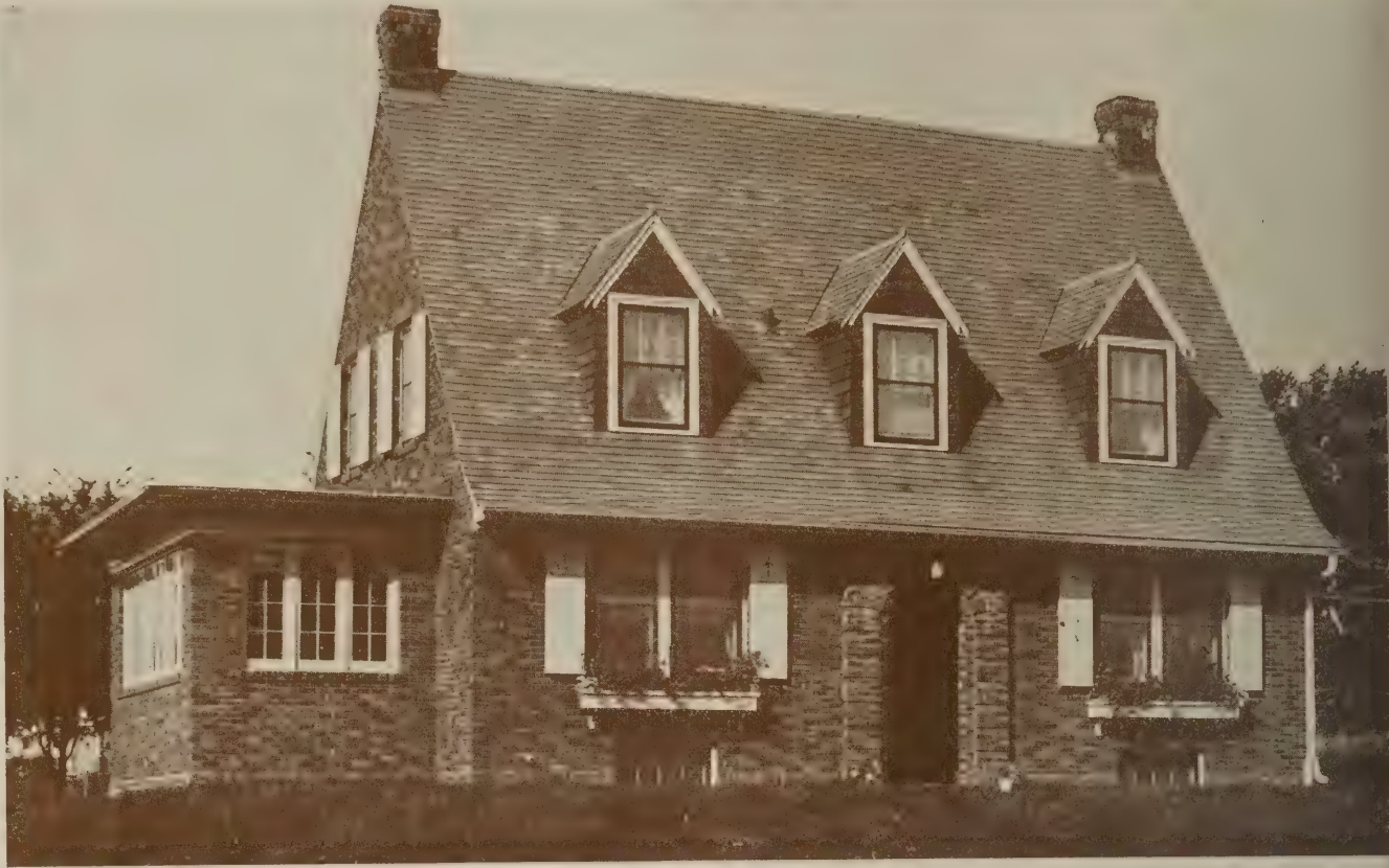
Face Brick and Stained Shingles Are Effectively Combined in This Little House in Iowa City, Iowa
