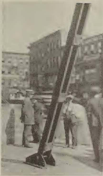
The stiff-leg brace is fastened to falsework built below the sidewalk. The legs are fixed in the same manner
