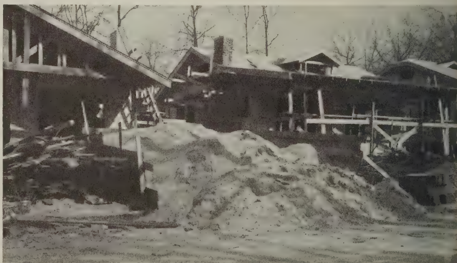
These few planks thrown together form retaining walls which confine the sand and keep it from spreading. This makes possible the dumping of a large amount of sand in a small area, a necessity where the working space is small
