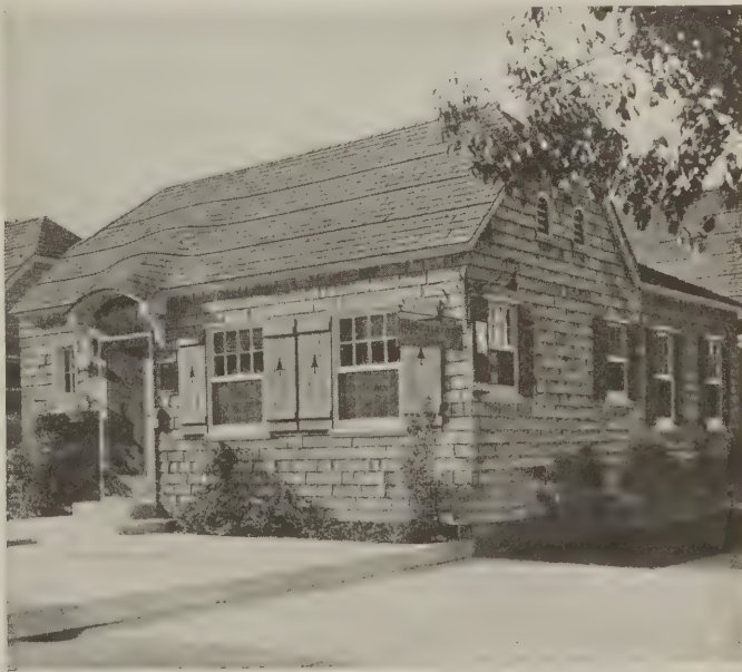
One of the buildings on the street front. The sign is not painted, the letters being cut in the wood
