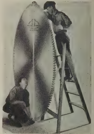
This saw, of the largest size ever made, is 108 inches in diameter and weighs 795 pounds. It was made by Henry Disston & Sons, Inc.
