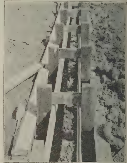
Top view showing shape of forms
