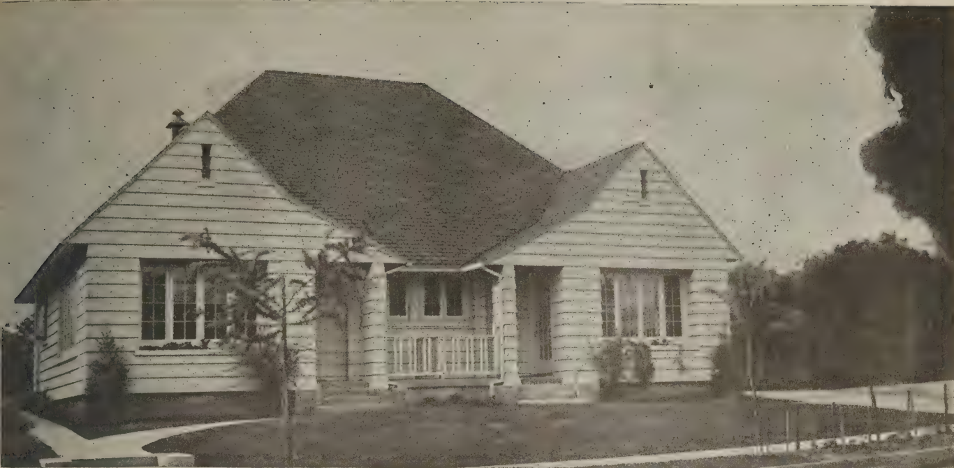
Duplex house of Mrs. Lucy E. Sellers, Alhambra, California. Ernest Irving Freese, Architect, 4675 Hollywood Boulevard, Los Angeles
