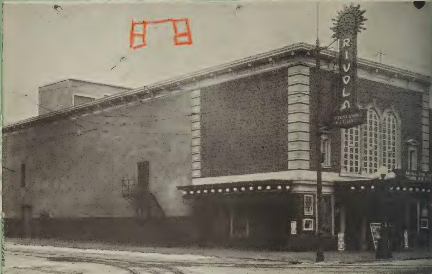
Rivola moving picture theater, Oskaloosa, Iowa. Vorse, Kraetsch & Kraetsch, architects. The building is an old remodeled store, with new fronts on both streets
