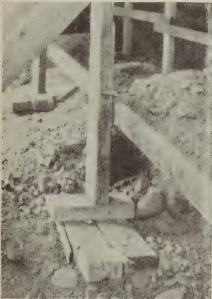
The two pieces which rest directly on the ground provide for the distribution of the load over a large area of ground and the folding wedges upon which the vertical support is set permits leveling of the formwork above
