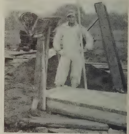
This hod rest is nailed to the side of the mortar box
