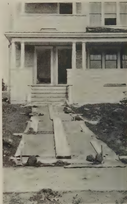
A small amount of ordinary building paper and a few plank will protect a fresh-laid walk against damage by rain. The cost of this protection is small
