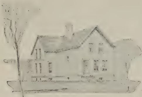
Fig. 1—Cottage type of house before remodeling
