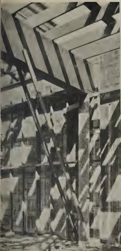
Method of supporting girders temporarily
