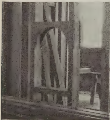
This simple framing is all that is necessary to install a wall niche for a telephone
