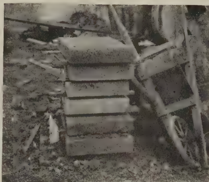
Wood strips are used between each of these pieces of stone
