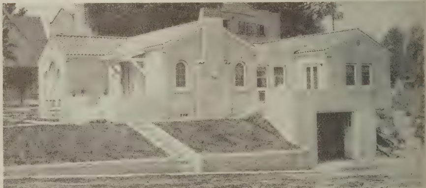
Built on a sloping street, it was possible to incorporate the garage beneath the house
