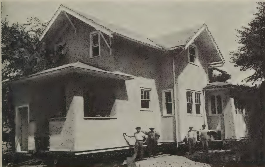
Rear view of the main section of the building as it was being set on its new foundation. It was pulled into the lot rear-end first
