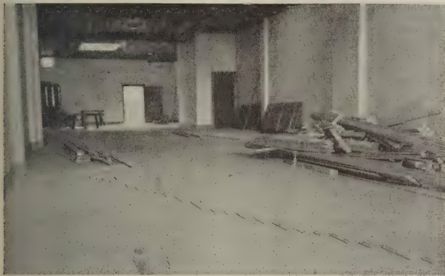
Notice the broken joints in this flooring enabling the carpenters to use up the smaller pieces. This method of laying floors provides for building up the full width of the floor soon after the laying is begun. Thus the floor is wedged tightly and is not liable to loosen up if left overnight, as might be the case if the flooring were laid in sections parallel to the walls
