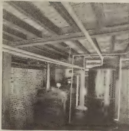
View of boiler room. Note steel joist construction
