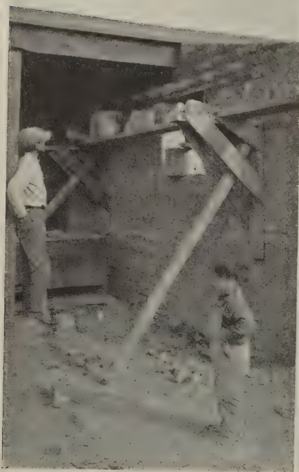
Fig. 6—Native scaffolding. The pole is not fastened in the ground but its pointed end keeps it from slipping
