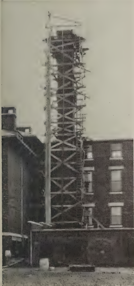
The built-up scaffold
