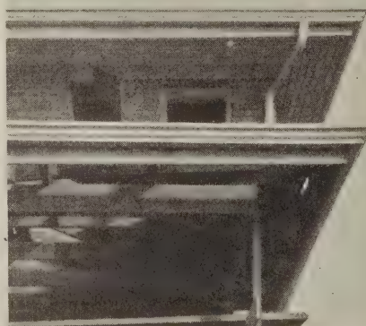
This is a view of the gutter from below. Notice the nice, clean-looking job, and the fact that the hangers do not show
