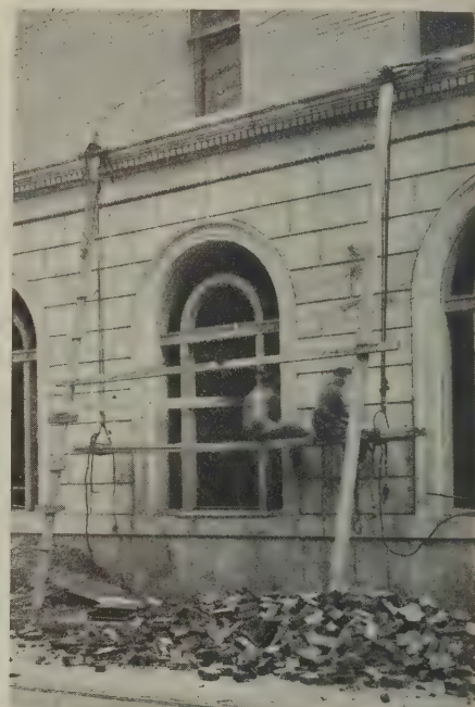
This type of scaffold can be used only for the base of the wall
