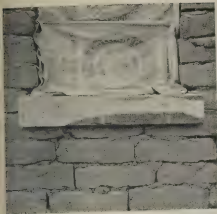
Fig. 8—Formwork for concrete sill. The cement sacks were used to block the window opening
