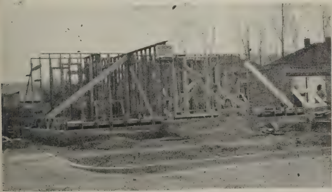
Fig. 2—The start of an adobe house. The partitions are erected before the walls
