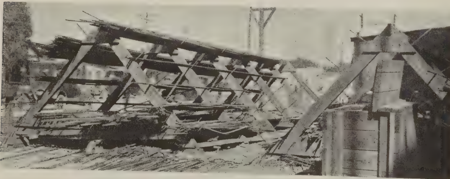
This rack for holding reinforcing rods may be easily dismantled and moved from job to job
