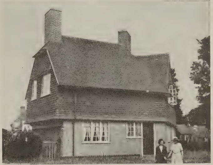
At the end of this house, the upper story projects considerably beyond the lower story and the overhang is carried on a stucco cove springing from the lower wall
