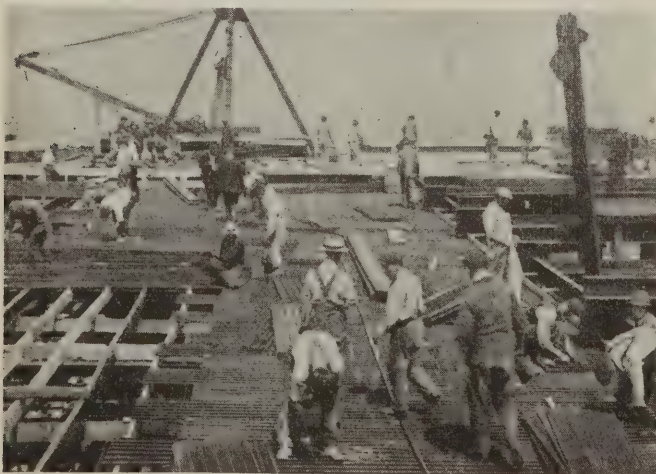
How skyscrapers were erected way back in 1924
