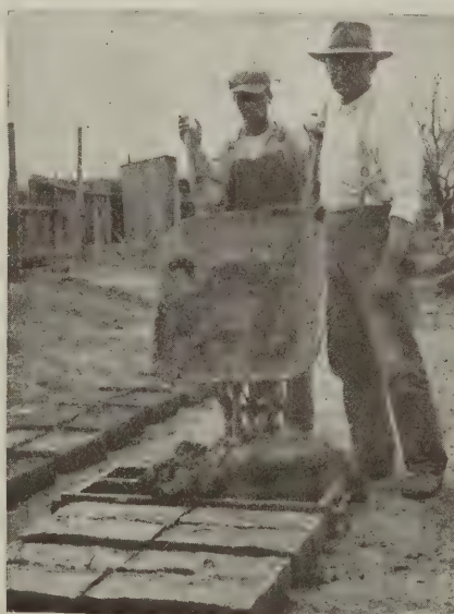
Fig. 3—Dumping the mixed clay into the mold
