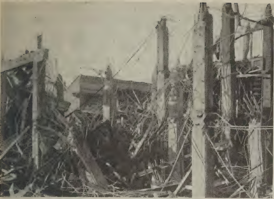
Fig. 4. Close-up view of the collapsed structure. Notice that the concrete has broken entirely away from the reinforcing rods
