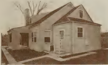
Rear view from the garage
