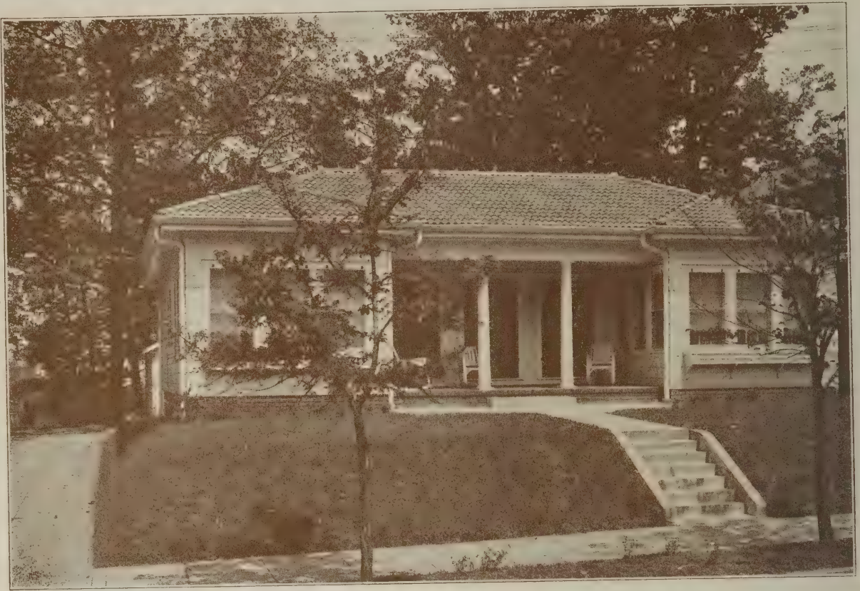
The home of John D. Chichester. Designed and built by Chichester Brothers, Birmingham, Alabama
