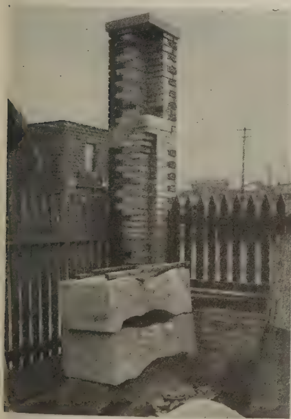
One of the corner piers. Note that it is arranged to carry beams in two directions
