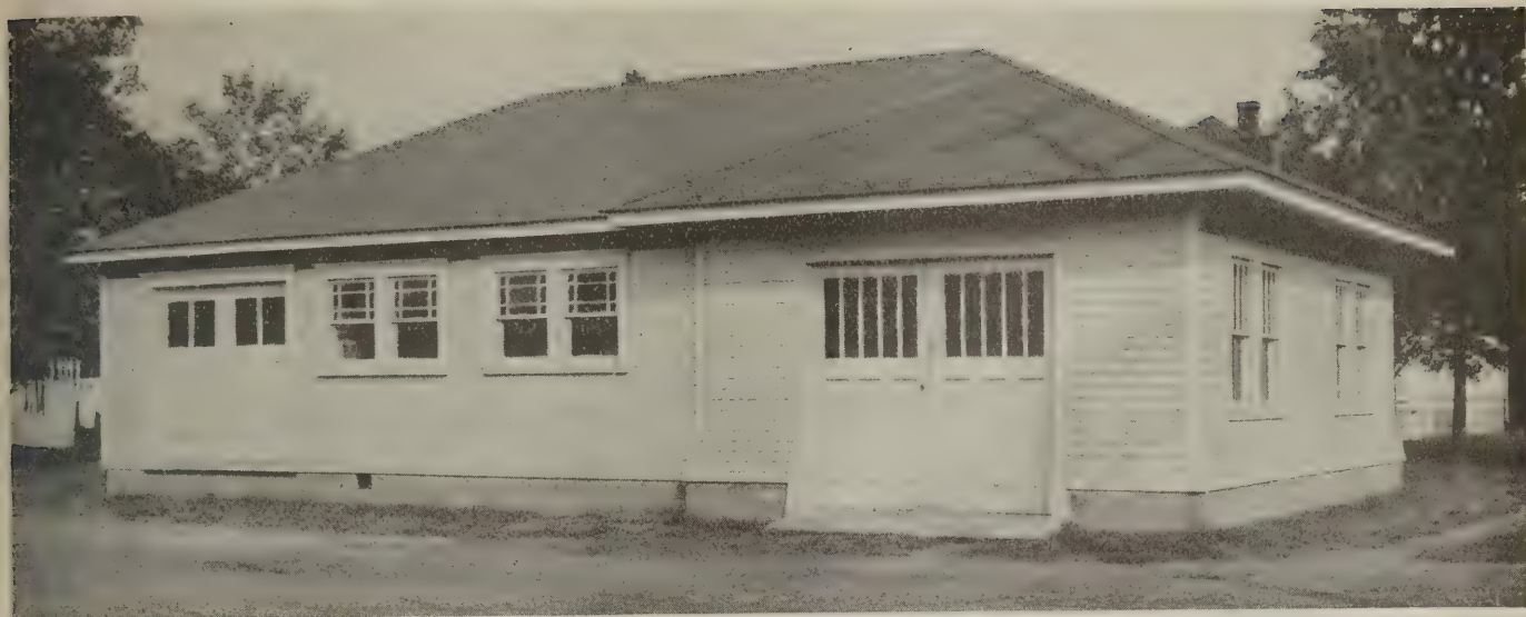
This looks a little different from the ordinary contractor's mill, doesn't it? The doors at one end are raised above the grade to make loading and unloading easier, and at the other end provision has been made for caring for a motor truck
