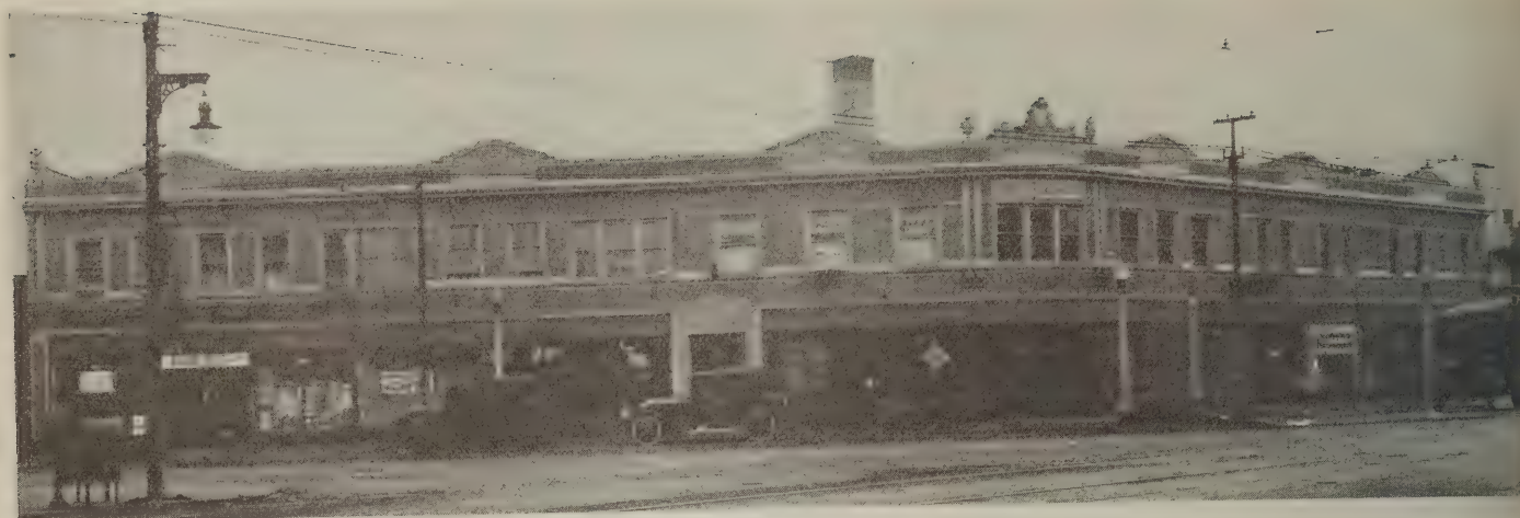
View showing elevations on both streets. Note the absence of posts in the corner entrance
