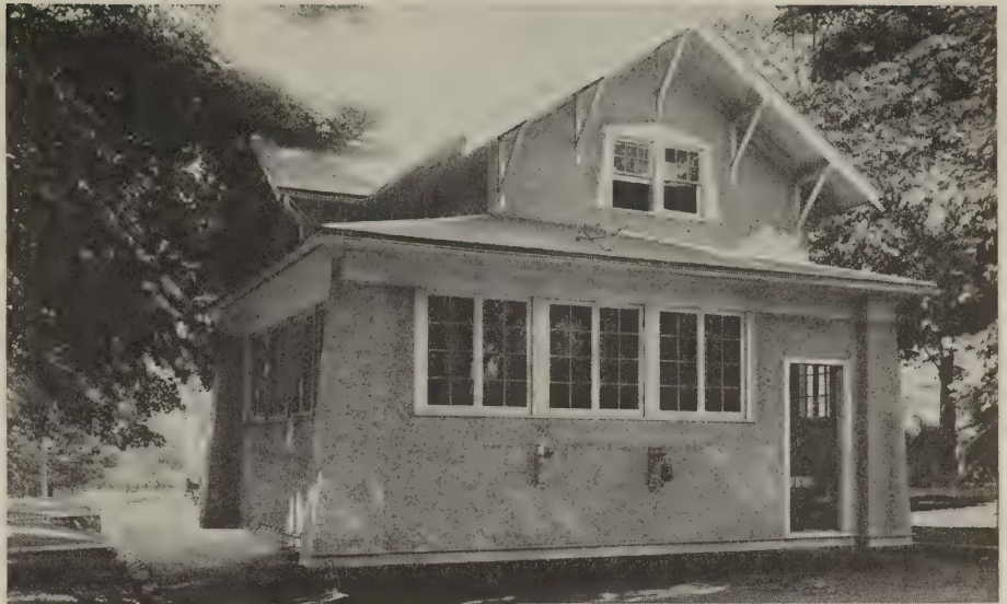
Front view of the main section of the building as it was being towed through the street. Heavy, wide-tread trucks were used
