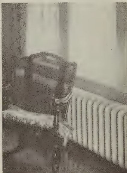
Behold the innocent radiator—paint it one way and heat is lost; paint it another and heat transmission is increased
