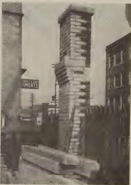
One of the intermediate piers. The stone plate above where the brick are corbelled out is the base for a steel beam
