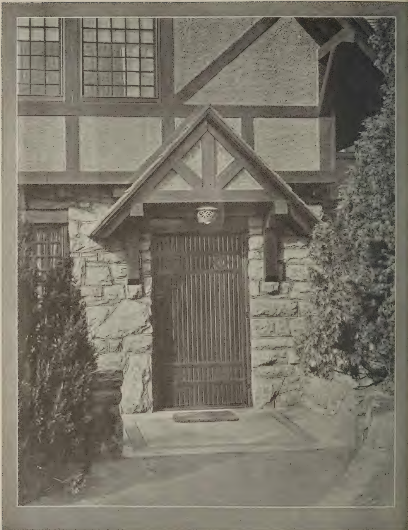
The Japanesque character of the design is well marked in the entrance. The rough stonework, the bronze lantern, the brass inserts in the stucco panels of the hood, the iron door hardware and the small panes of glass in the windows, all are reminiscent of Japan
