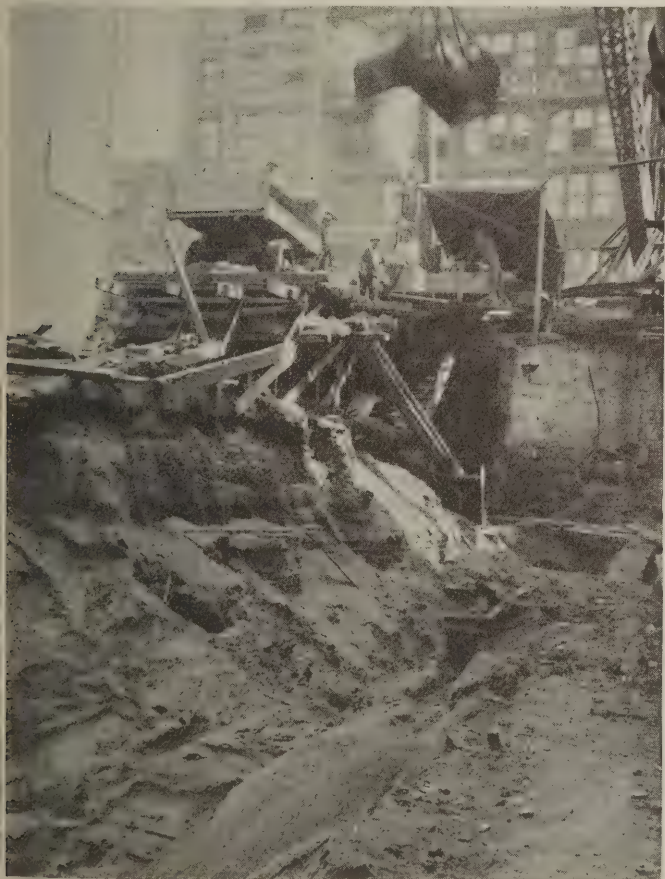
Illustration showing how trucks were loaded. The runway extends only part way into the excavation
