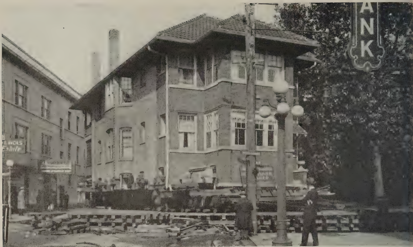
Illustration showing the house being turned
