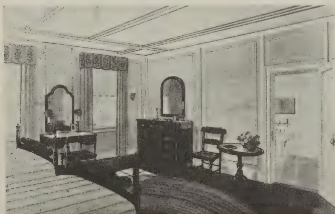
A bedroom paneled with wallboard. Wallboard tiling is seen in the bathroom
