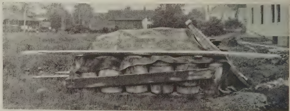
Planks are used to hold down the tarpaulin. They are set in rope loops running through the tarpaulin eyes
