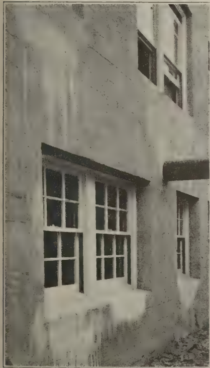
The court walls are of plain unfinished concrete allowing form marks to show
