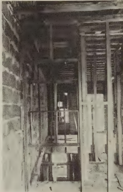
This is a front view of the closet. Notice that the steps appear as a series of shelves
