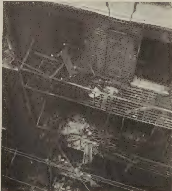
Flames came out these windows in the early stages of the New York tenement fire and rendered the escape useless. Fourteen people killed
