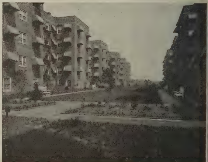
A view looking into a garden court in the rear of the buildings
