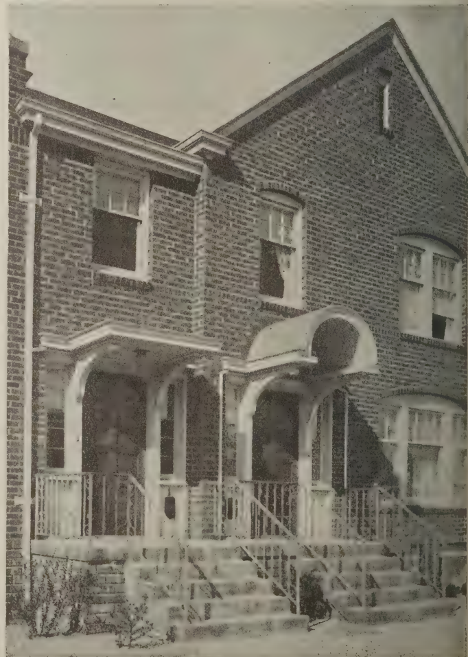
The entrances are dignified by the use of wrought-iron railings
