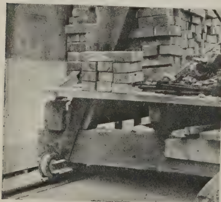
Wheels at base of derrick
