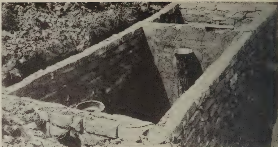
A brick septic tank, being built from the plans on the preceding page, for a family of eight. The walls are laid up with cement, lime mortar plastered on the inside. A concrete top and bottom was used. The cover was reinforced by one-quarter inch bars spaced about eight inches apart, both ways. The tank has no siphon but discharges directly into an agricultural tile line. The tank was constructed under the supervision of the author of this article. It stood a temperature of seventeen degrees below zero before being covered with earth
