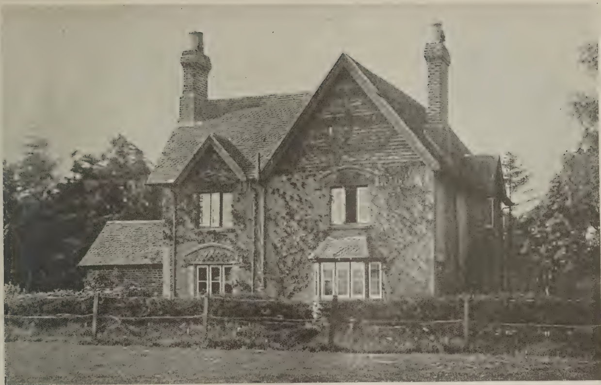
The courses of shaped tiles in the roof of this old house are repeated in the gables, thus relieving the plain surface
