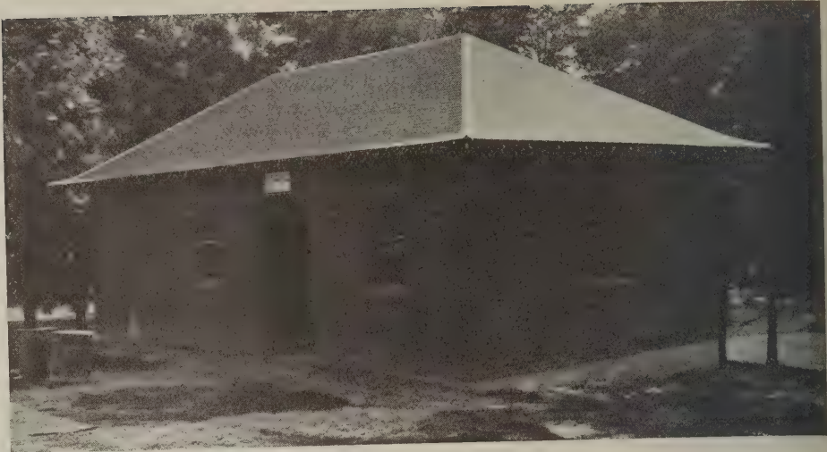
Open during the entire touring season, this little building in one of the parks in Keokuk, Iowa, spells hospitality in all capitals to the tired, disheveled tourist. It is a gift of the local Lions Club and was designed and built by Fred C. Johnson
