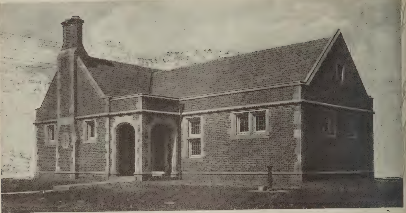
This building is located near institutional buildings built of a reddish brown stone. The bricks were selected with great care to match the color of the stone
