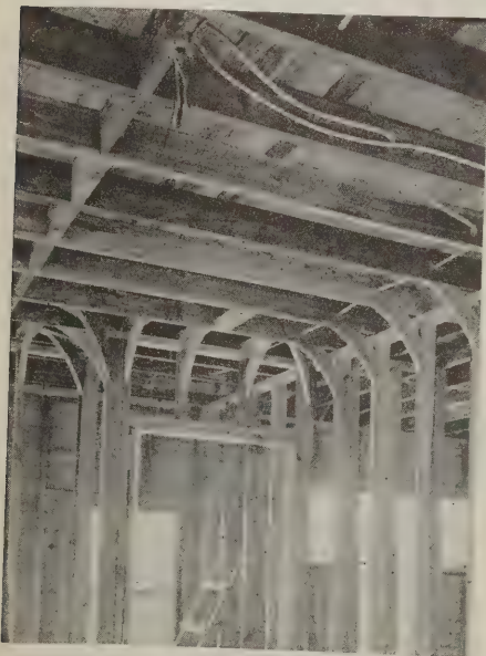
Cove pieces in place at the junction of wall and ceiling
