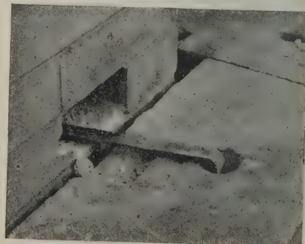
Wall tie used to hold stone veneer
