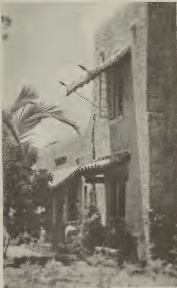
The October National Builder will be full of pictures like this
