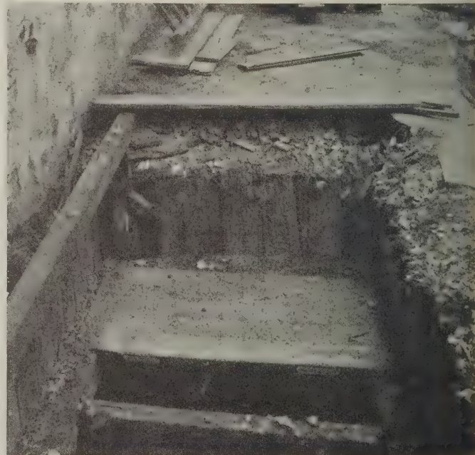
View of the other end of the well. Here is shown the top platform to which the excavated material is shoveled from below
