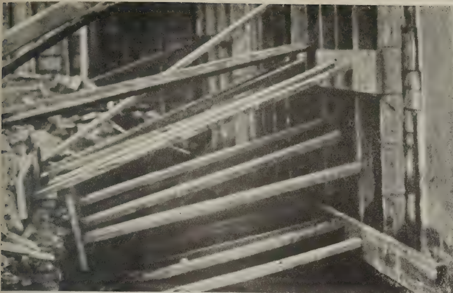
Concrete foundation formwork. Notice the water at the bottom of the picture
