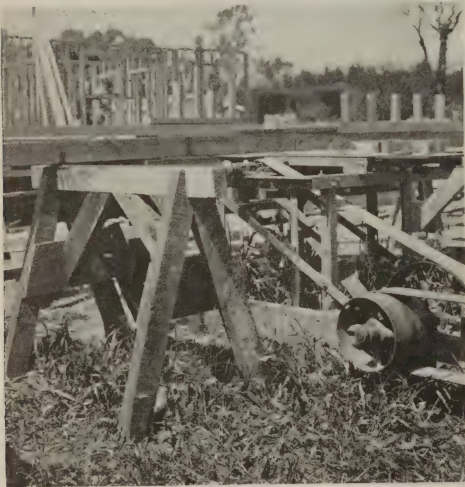
Close-up of the saw showing construction details for the horses. Notice that they are fastened to stakes, thus holding them firmly
