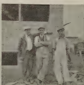
On the Job With J. Johnson and Son, Mal- den, Massachusetts
