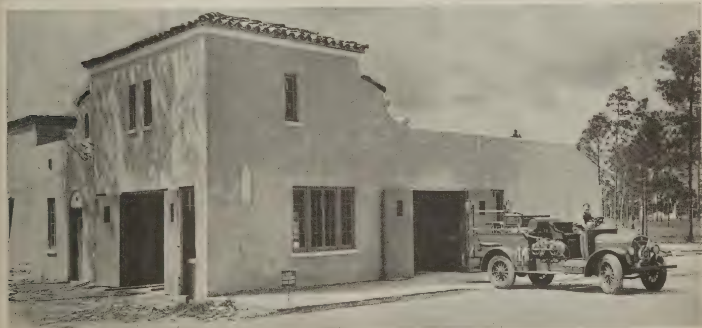
The fire department quarters is an important feature of the business section
