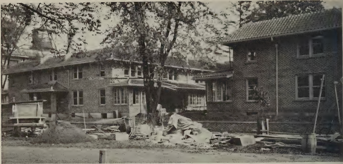
A general view of the job. The building is set up off the street grade and a retaining wall built at the sidewalk to carry the terrace
