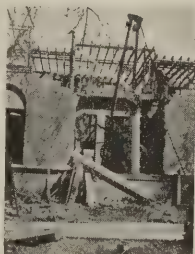
Stone columns are lifted by mechanical power
