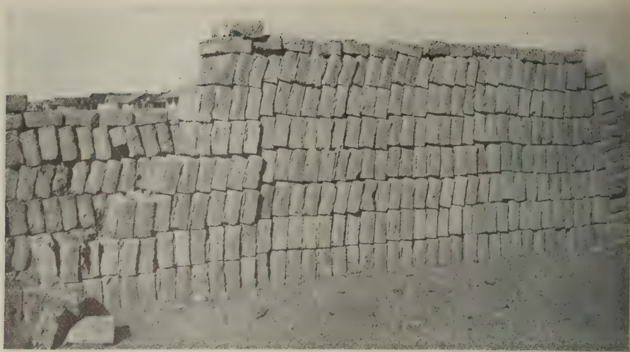
Fig. 11—The cured adobe brick are stacked as shown here
