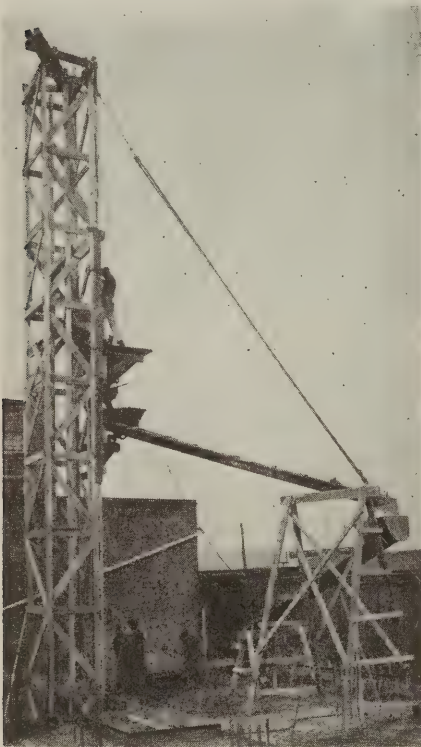
Fig. 1—Boom chute supported near end by tall scaffolding similar to an ordinary "horse"
