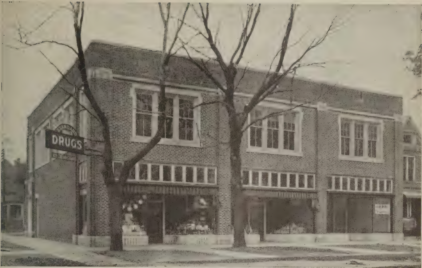
A small building, free from pretence, yet dignified and interesting
