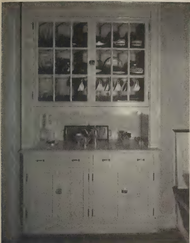
This is an example of poorly-selected hardware. It is conspicuous and crude for a sideboard, where it might pass for use on a kitchen dresser. Compare it with the hardware on the sideboard on the right
