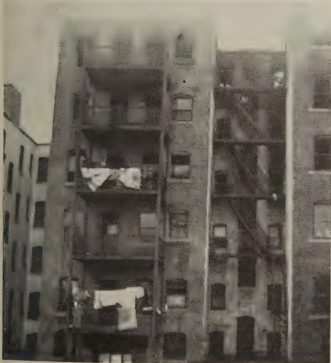
Rear view of apartment house in Boston after the fire in which eight lives were lost. Escape was made impossible by flames issuing from window openings
