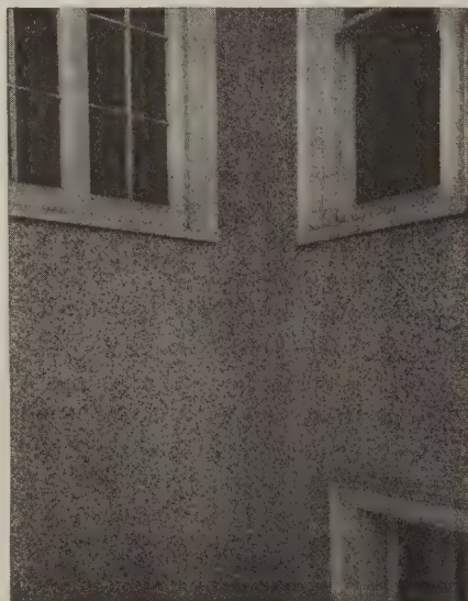
An interior wall corner, a likely place for a crack, yet no crack is to be seen
