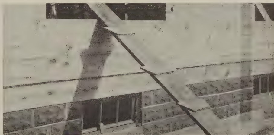
View of plank with extended cleats
