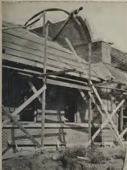
Fig. 3—Templet used in forming curve
