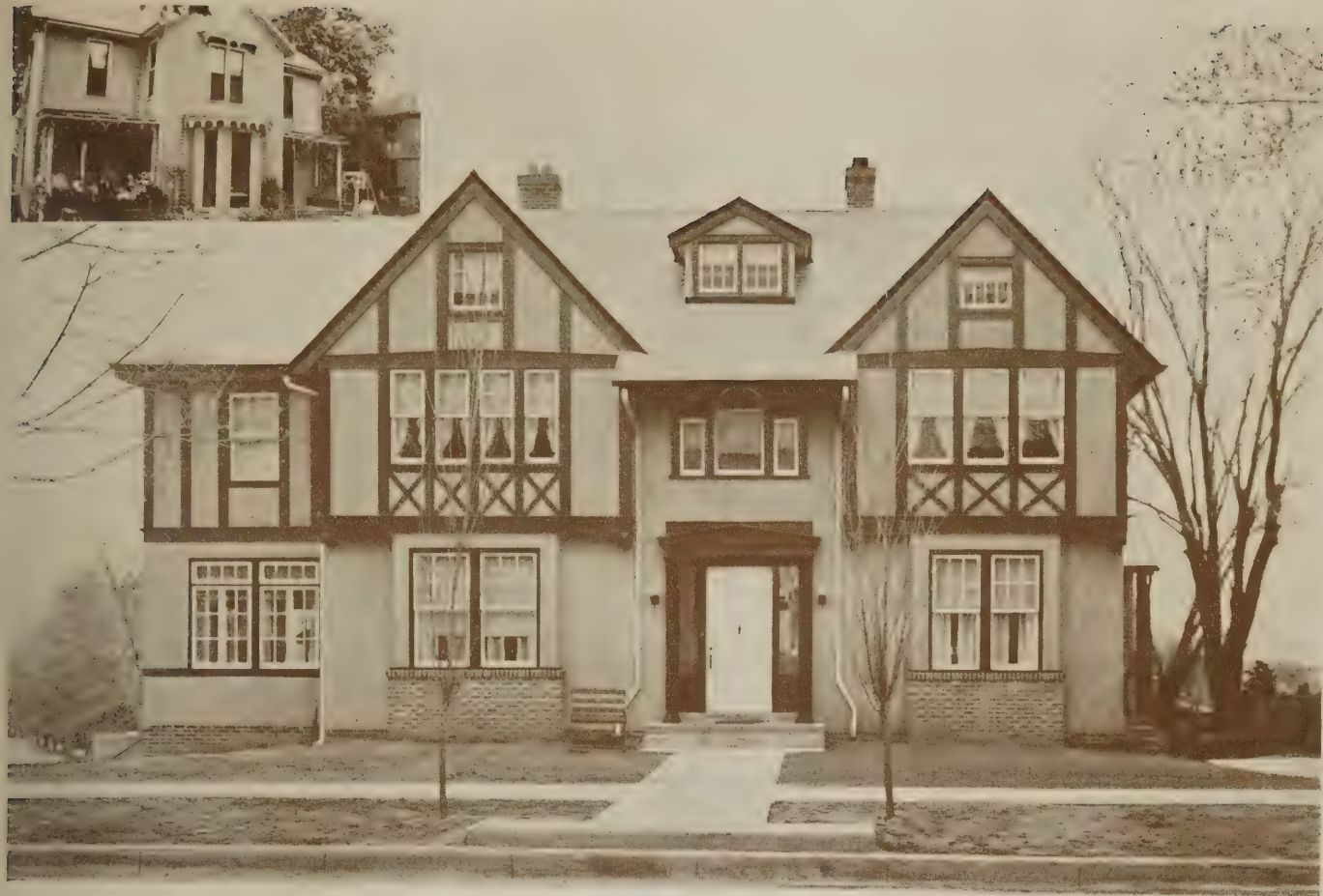
In the upper left-hand corner is how the old house looked before it was renewed and enlarged as shown above. Frank Weber, owner; J. W. Young, contractor, Keokuk, Iowa
