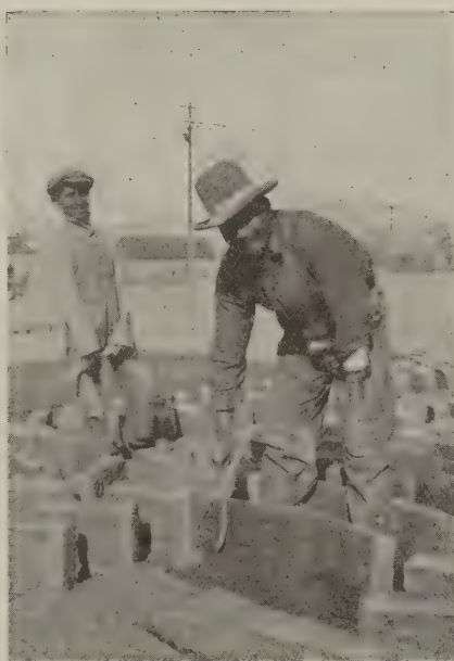
Fig. 8—Scraping off the dust from the bottom of the bricks
