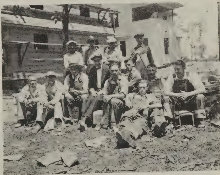
On the job at Rochester, New York, with the building crew of Geo. Wegman's Sons Co.
