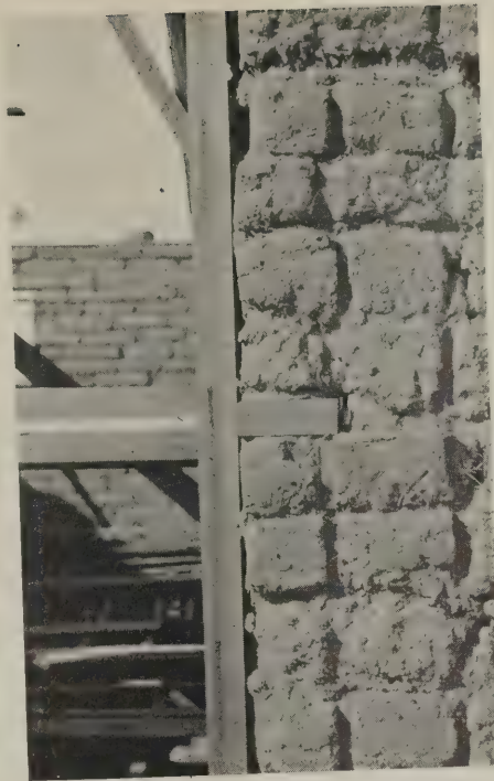
Fig. 9—Jamb block for holding door frame
