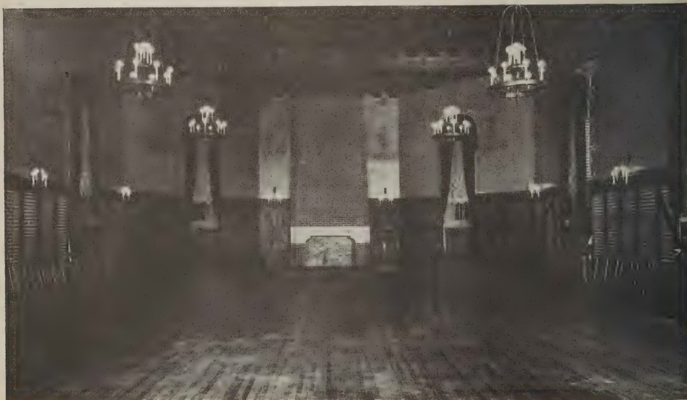
The ballroom is treated after the manner of the Great Halls of the Tudor period. The ceiling is of dark stained wood supported by a series of heavy timbered beams. The fireplace is a prominent feature and an important means of ventilation
