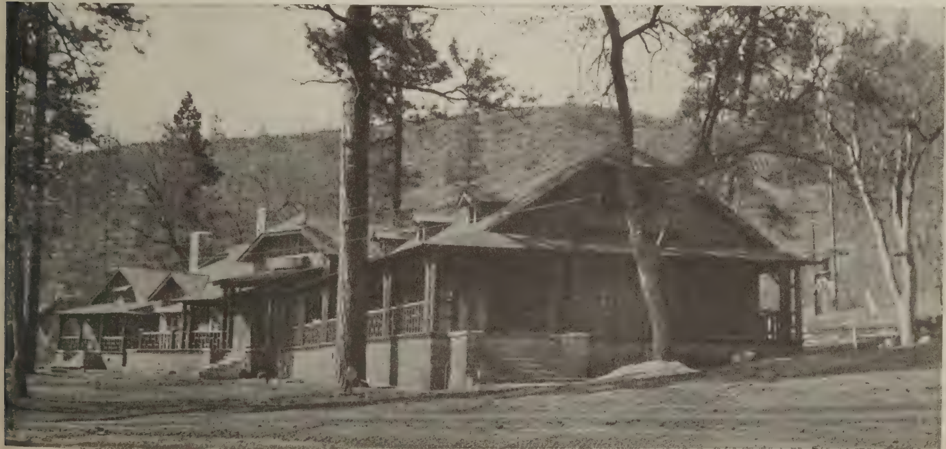
Cedar logs were used for the porch posts and the walls are covered with split cedar shakes
