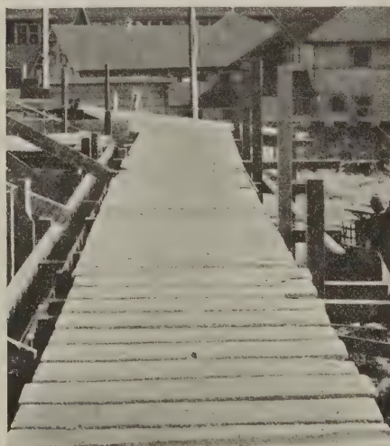
Detail of runway
