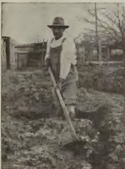
Fig. 2—Mixing the adobe clay with straw and water
