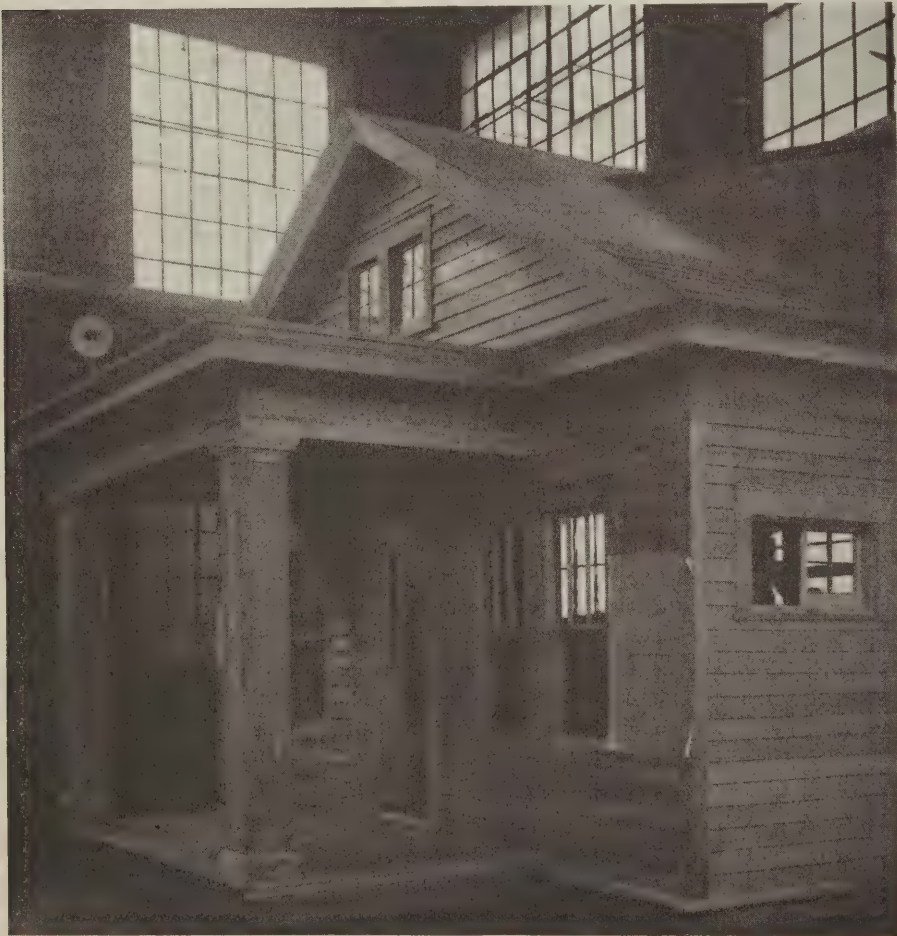
Outdoor building in an ideal climate. Class has nearly completed structure
