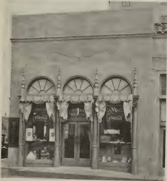
A detail of one of the corner stores
