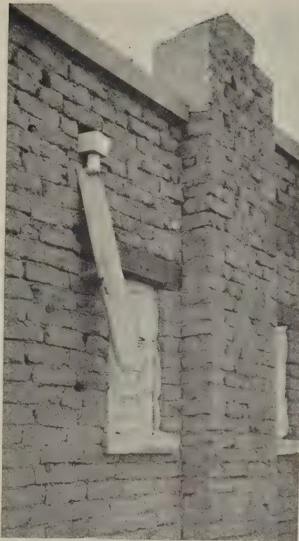
Fig. 5—Water is led away from the wall until the downspout is placed
