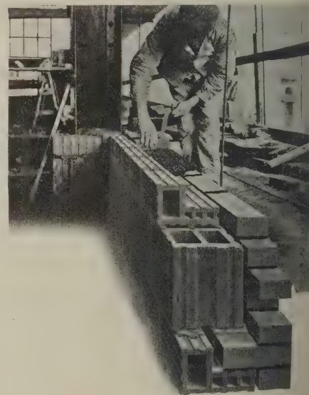
Showing how Natco header backer tile is employed to back up a stone wall
