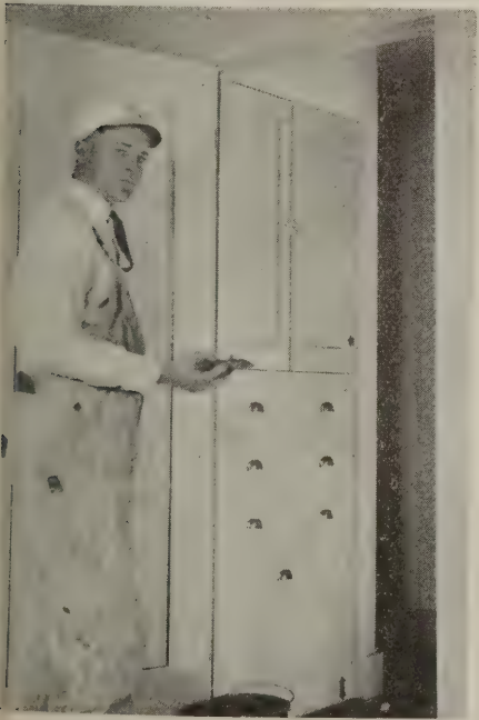
L. H. Pickens finishing up the galvanized plaster stop
