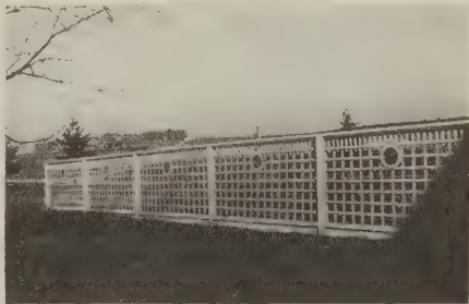
Fig. 5—Fence to screen railroad
