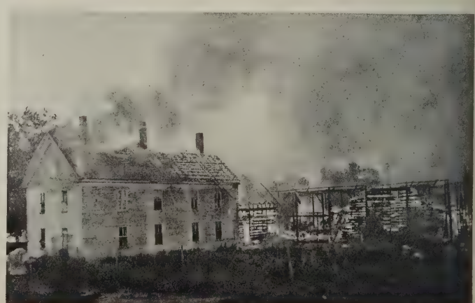
This farm house was rodded but the barn was not. Lightning struck the barn. The ensuing fire destroyed the house as well as the barn. Lightning rod protection must be complete to be effective
