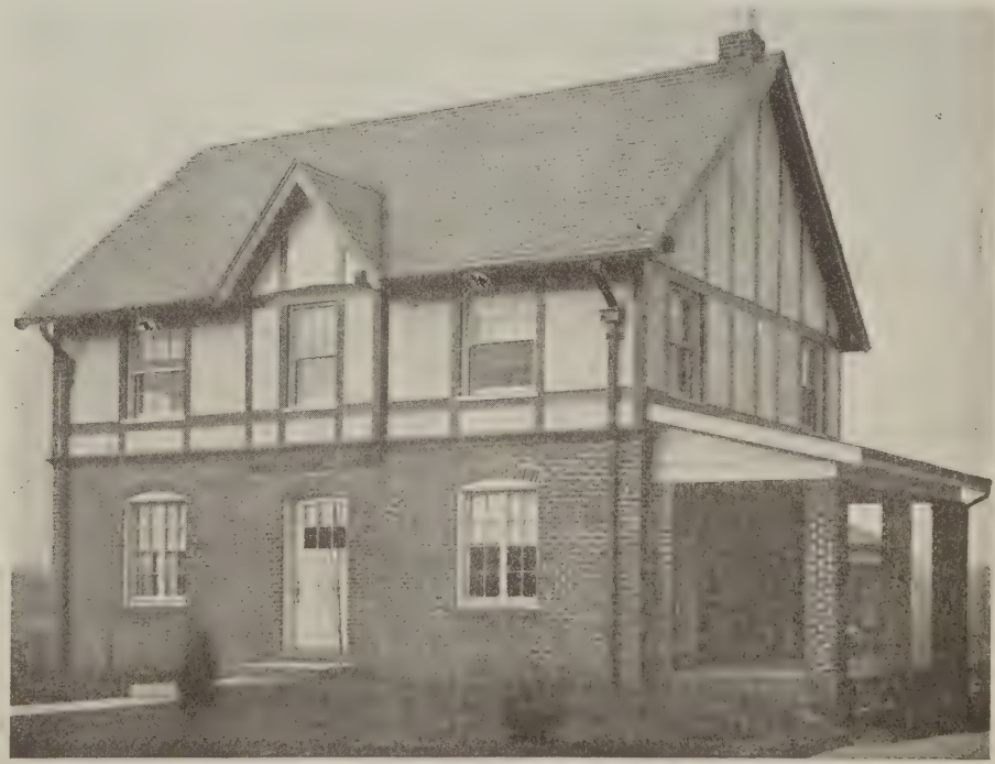
Building No. 3 on lot No. 5, a seven-room brick-and-stucco house with seven major rooms and attached garage. This house is on a 55-foot lot
