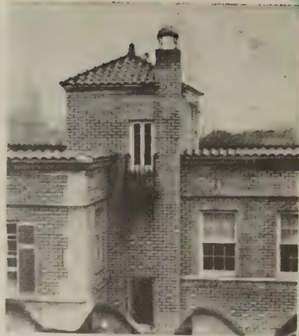
View showing elevator pent-house. It is an attractive feature of the building instead of an eye-sore as is often the case
