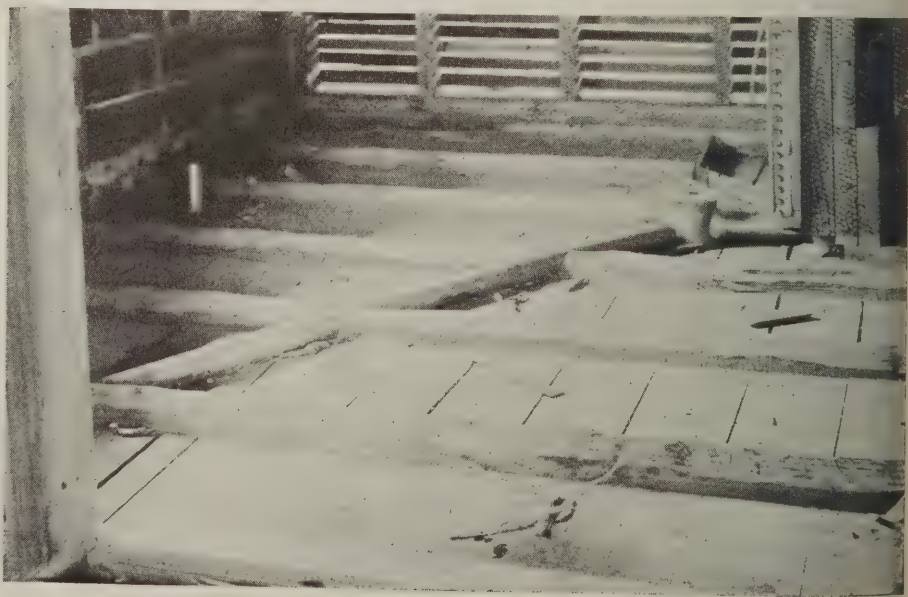
Notice that the edges of the joists are trimmed to a V shape
