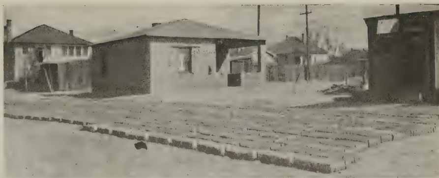
Fig. 5—Adobe brick set out to dry in the sun after being molded
