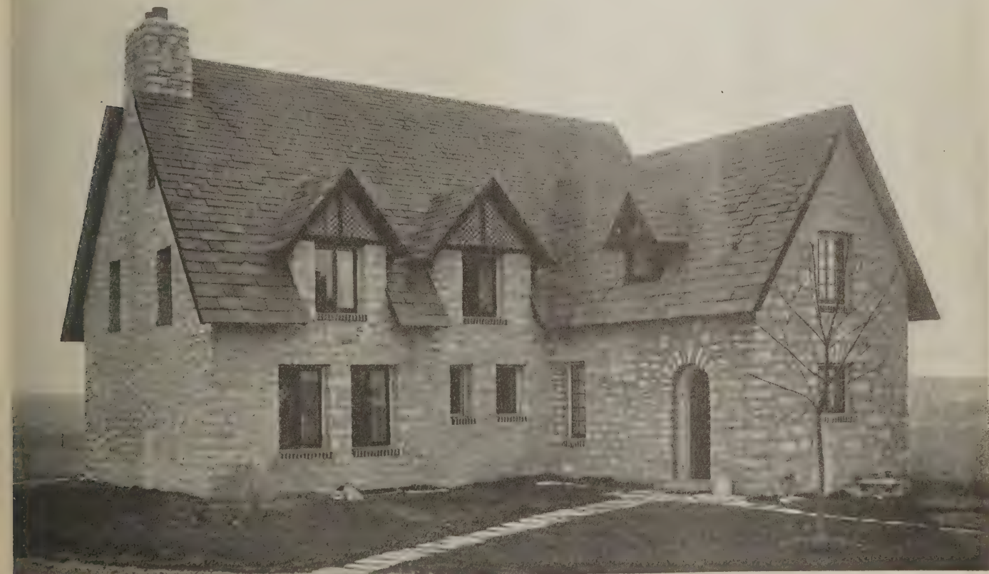
Rear view showing the kitchen wing
