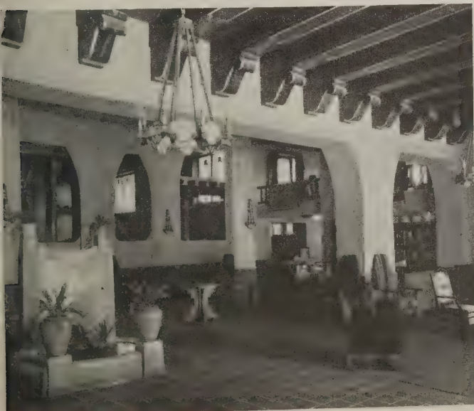
A corner of the main lobby
