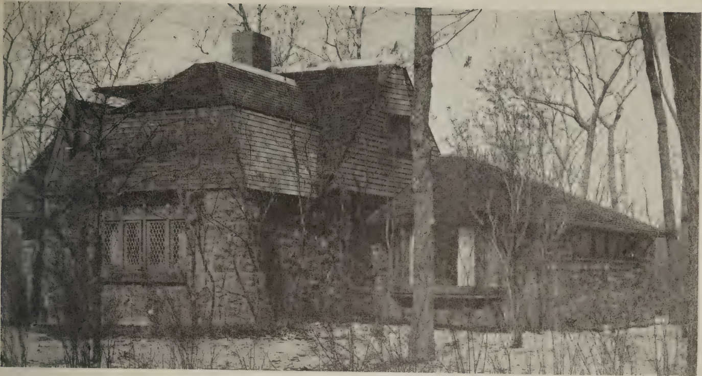
The walls are of rough stonework, with shingled roof and gables. The sheet metal ridge cresting is interesting
