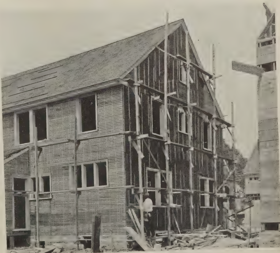
Illustration showing scaffolding in place
