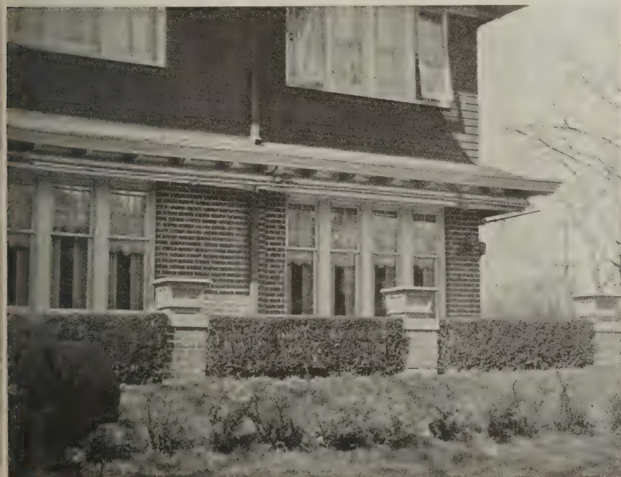
Brick piers with a hedge between form a terrace enclosure
