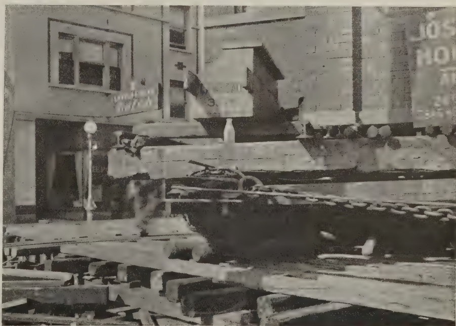
A view at a corner. Note that the tool box is set on the building and so carried along with it
