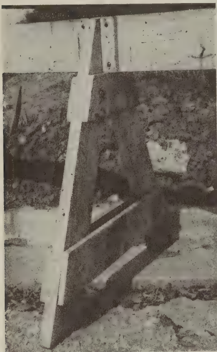
One of the bar supports
