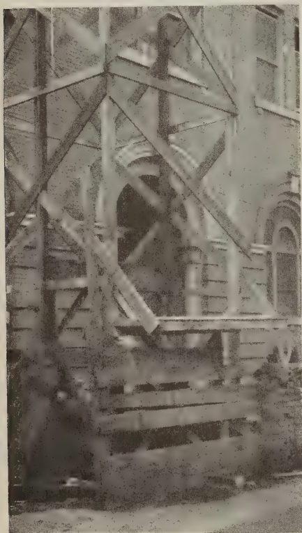
This platform attached to the tower permits unloading from the wagon directly to the hoist and saves the labor required to rehandle the materials
