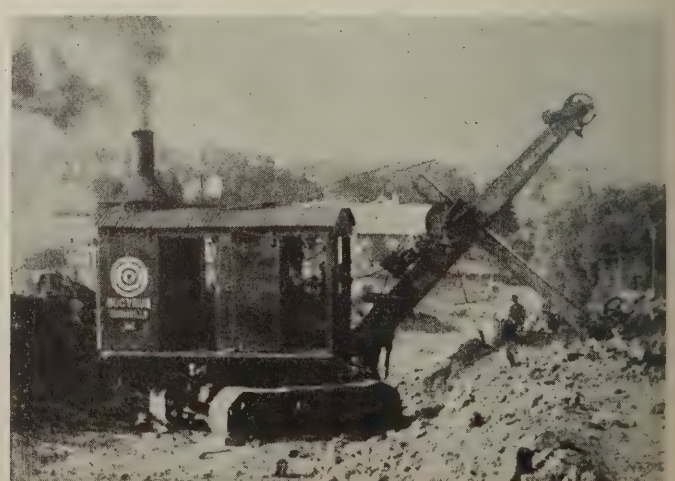
Excavating for a big Twentieth Century building
