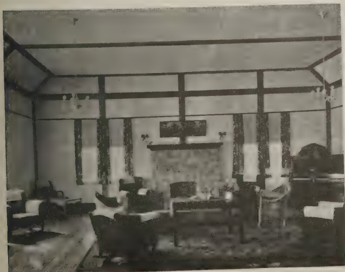
Stone fireplaces are provided at the ends of the assembly room
