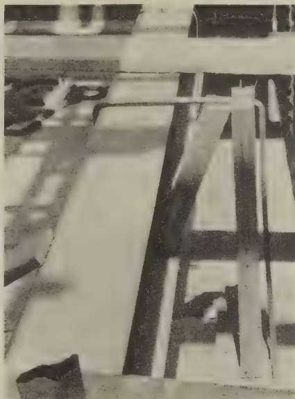
Fig. 4—Photographic illustration of steel-rod loop above roof
