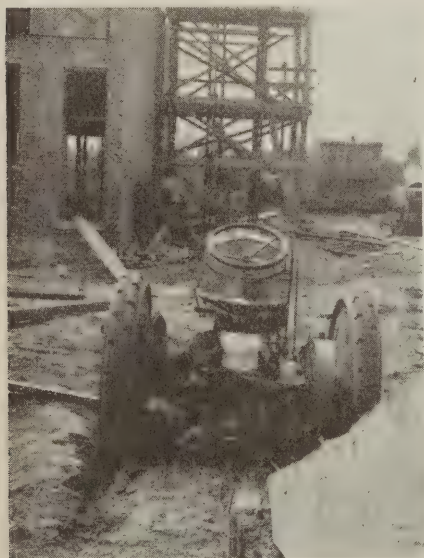
Combination hoist and tractor on the job in Chicago
