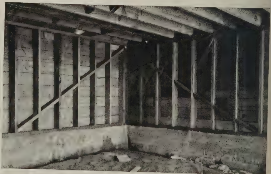
2x4 bridging used for bracing a wall corner
