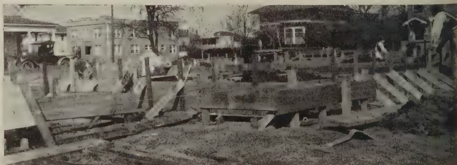
Illustrations showing the forms in place. Note how the braces are nailed to the cleats
