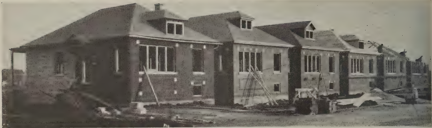
Here is the first group of bungalows almost completed. Compare this with the bleak view on the next page
