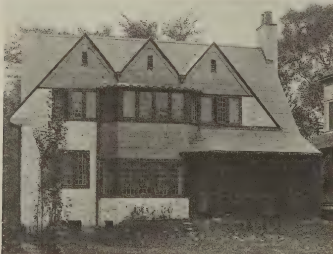
At the rear of the house, the upper portion of the bay and the gables are slated. The woodwork is stained and the gutters are painted black
