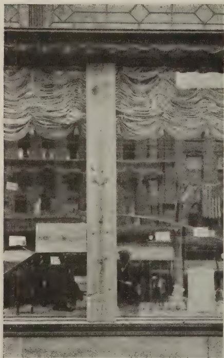
An emergency method of holding a broken plate
