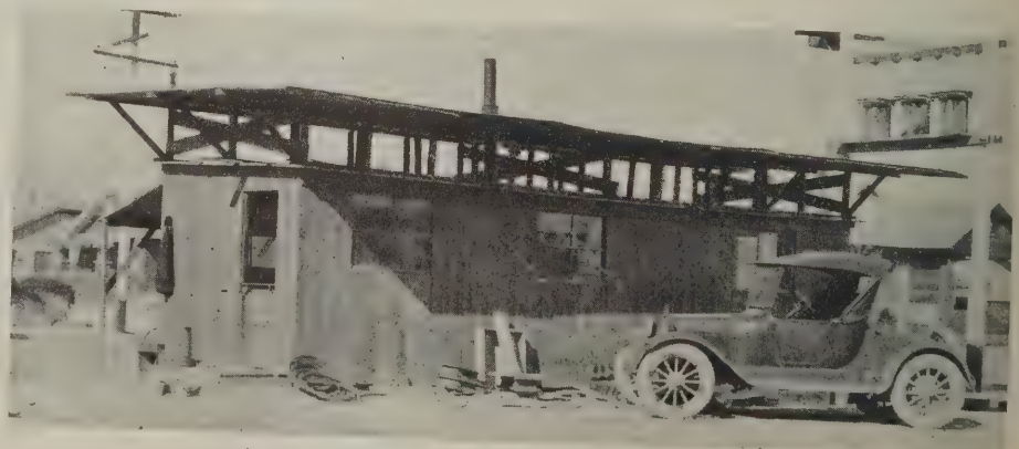
The double roof helped considerably to keep this shack cool in the summer time
