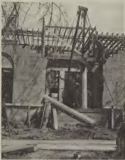
General view of building under construction, showing solid concrete columns, weighing one ton each, being raised into place
