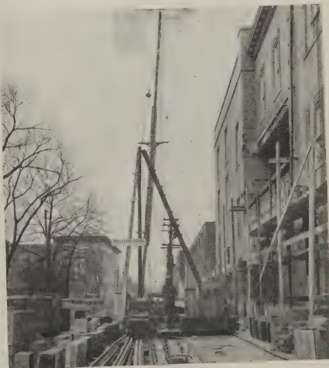
View of the stiff-leg derrick used to hoist stone
