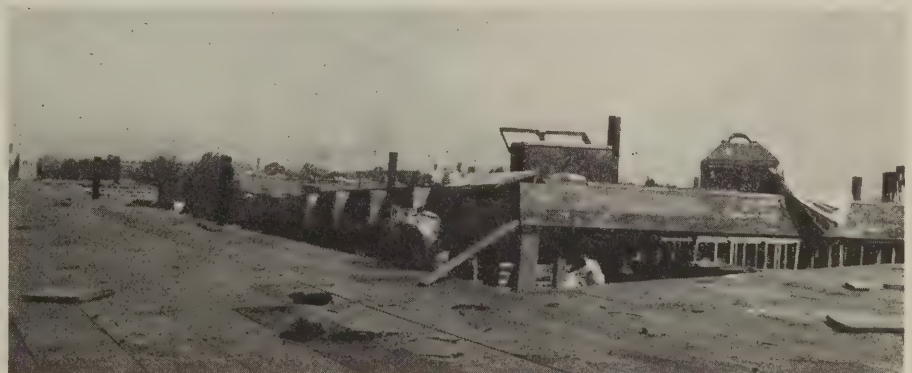
Notice the blue print box on the roof
