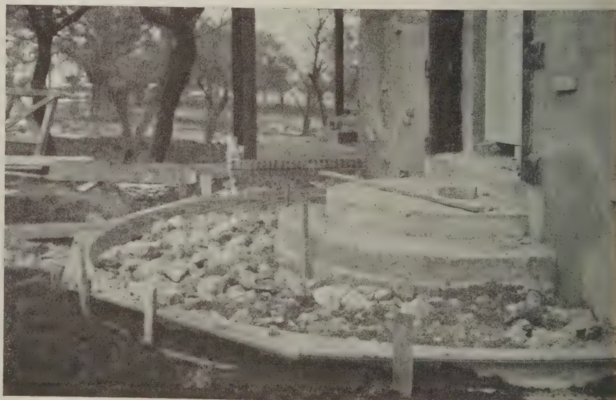
This carefully placed formwork is bound to result in a true curve. The horizontal templet is cut to a given radius and its purpose is to brace the piece of siding shown bent to the curve
