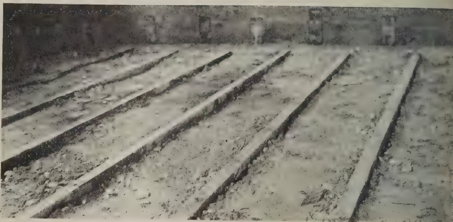
Sleepers set in the concrete floor
