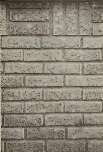
The tools described below can be used to produce a wall like this
