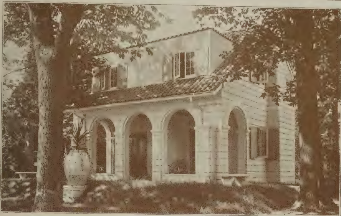
Home of James Roy Allen, Wilmette, Illinois. James Roy Allen, architect, Fine Arts Building, Chicago
