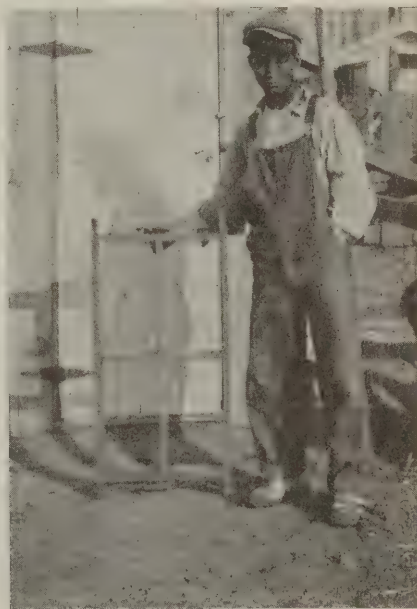
Fig. 9—A typical adobe mold and molder
