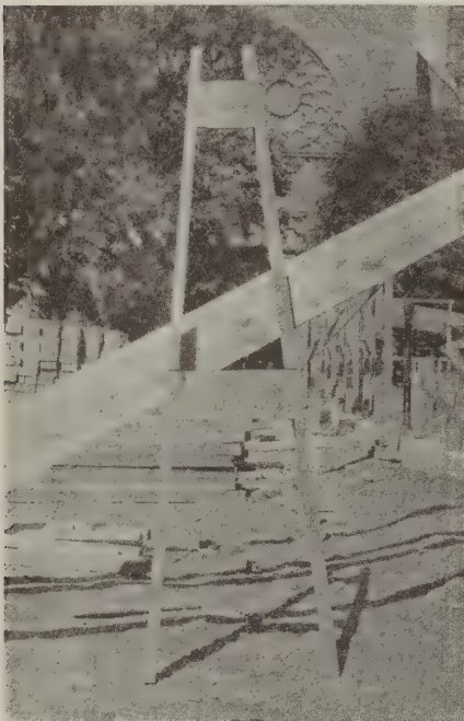
Front view of putlog support. No lateral bracing is necessary because the slanting legs act as braces
