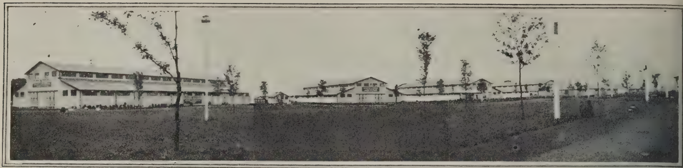
Women's Building, Horticulture and Agriculture, Fine Arts, and Automobile and Tractor Buildings. The amusements and swimming pool are in the right background
