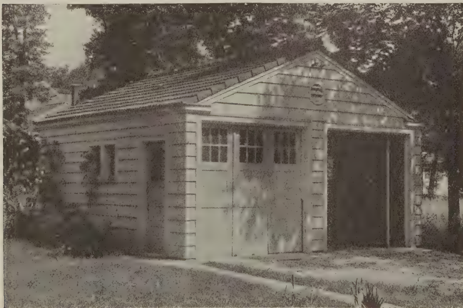
The doors are glazed with wire glass to reduce broken panes
