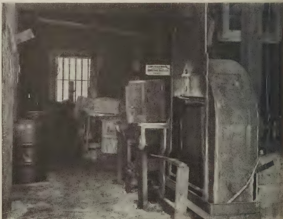
The shingle staining plant of the Industrial Sales Company
