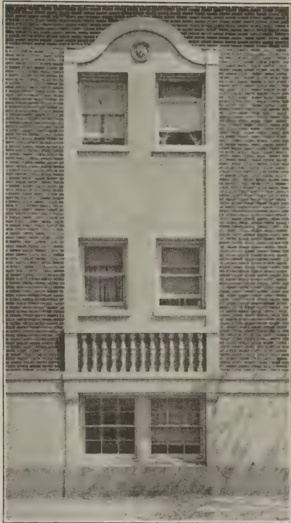
Stucco, contrasting brick and cast cement form interesting panels
