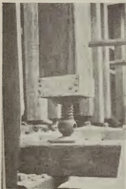
Nails driven into the under side of the shore at the drum flange and bent over the drum serve as a precaution against the flange rotating. The rotation of the drum flange may result in a loosening of the entire shoring system, hence it is well to take some step to prevent it
