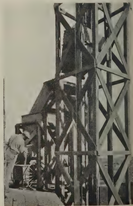
View at top of tower
