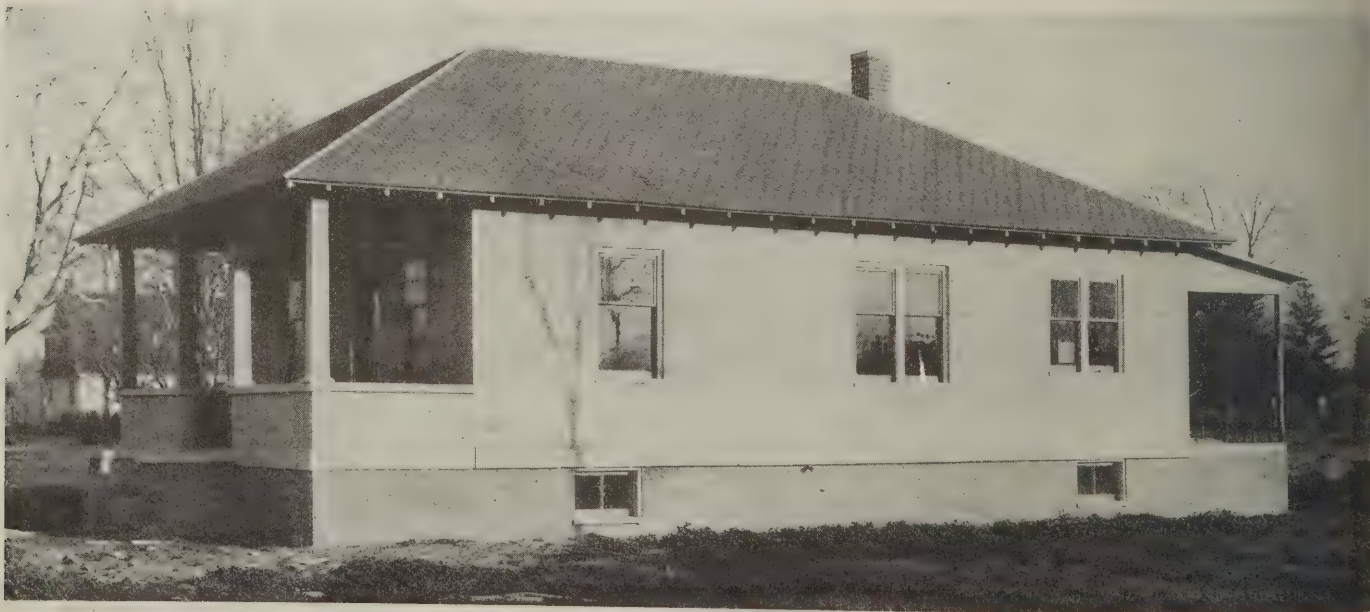
This house, built at Holland, Michigan, is a good example of how a building, though low in cost, may nevertheless be attractive in design
