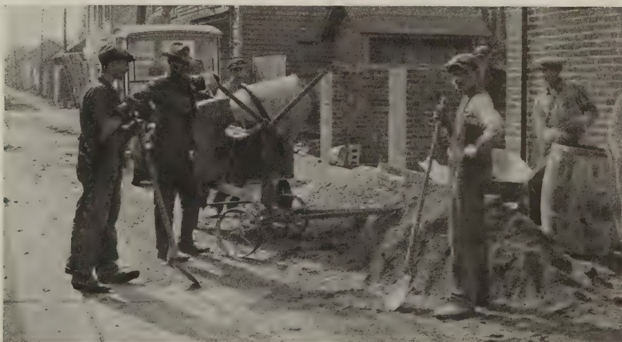
The aggregates for the mixer were dumped directly adjacent to it so that no wheeling was required
