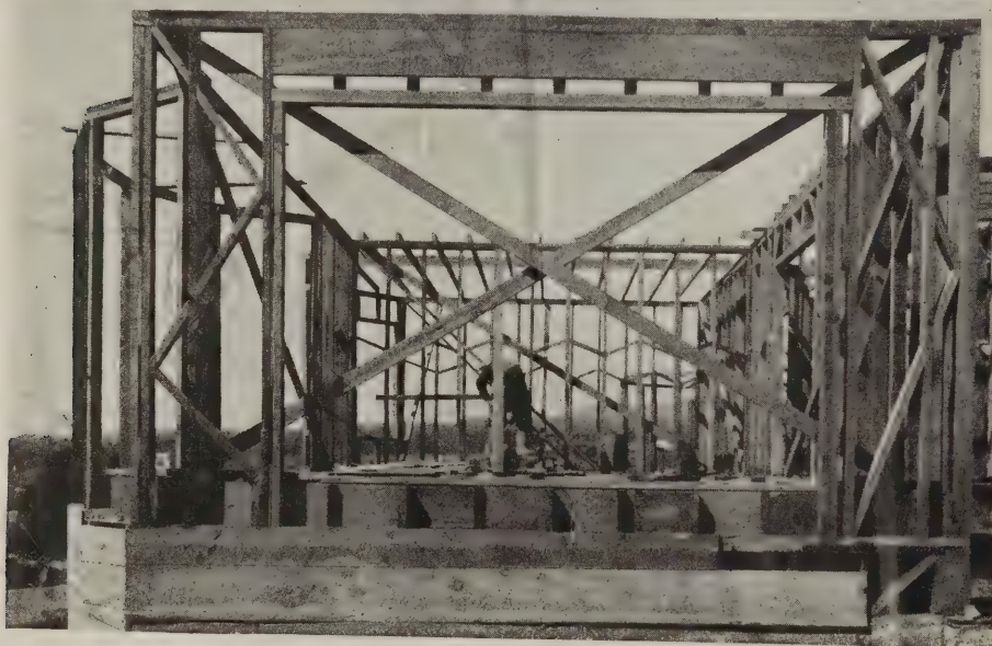
The bracing and heavy lintel help to strengthen the wall
