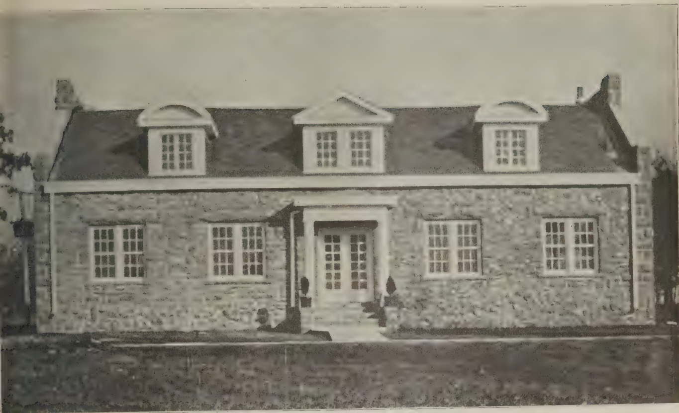
Hospital for Girls' Vocational School, Tullahoma, Tennessee. C. K. Colley, Architect, Nashville
