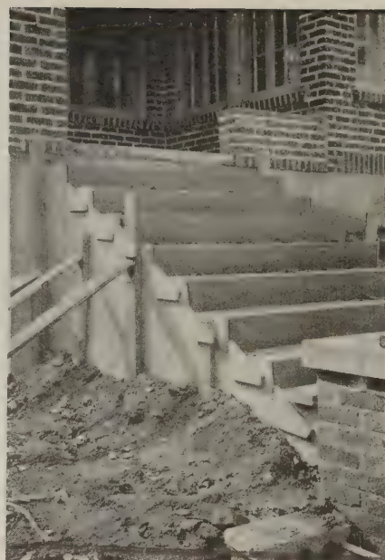
After use they were tacked to the stringer forms to prevent their being lost
