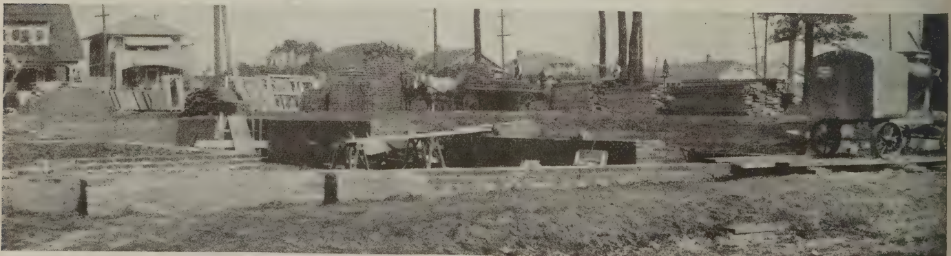
A view of the $140,000 apartment building under construction. This building was sold under the co-operative plan, each apartment being purchased by a different individual. All apartments were sold before the job was started
