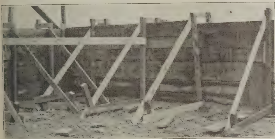
View of the formwork. Note its simple construction and also the method of bracing the corner
