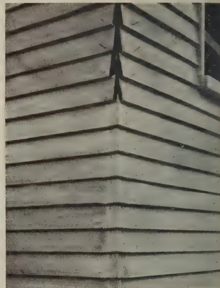
The siding is only tacked at the corners until the tin corner-pieces are placed
