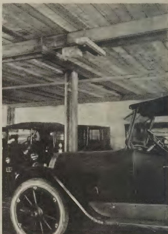
Fig. 2—View of interior showing wood shore removed and roof girders held in suspended seat
