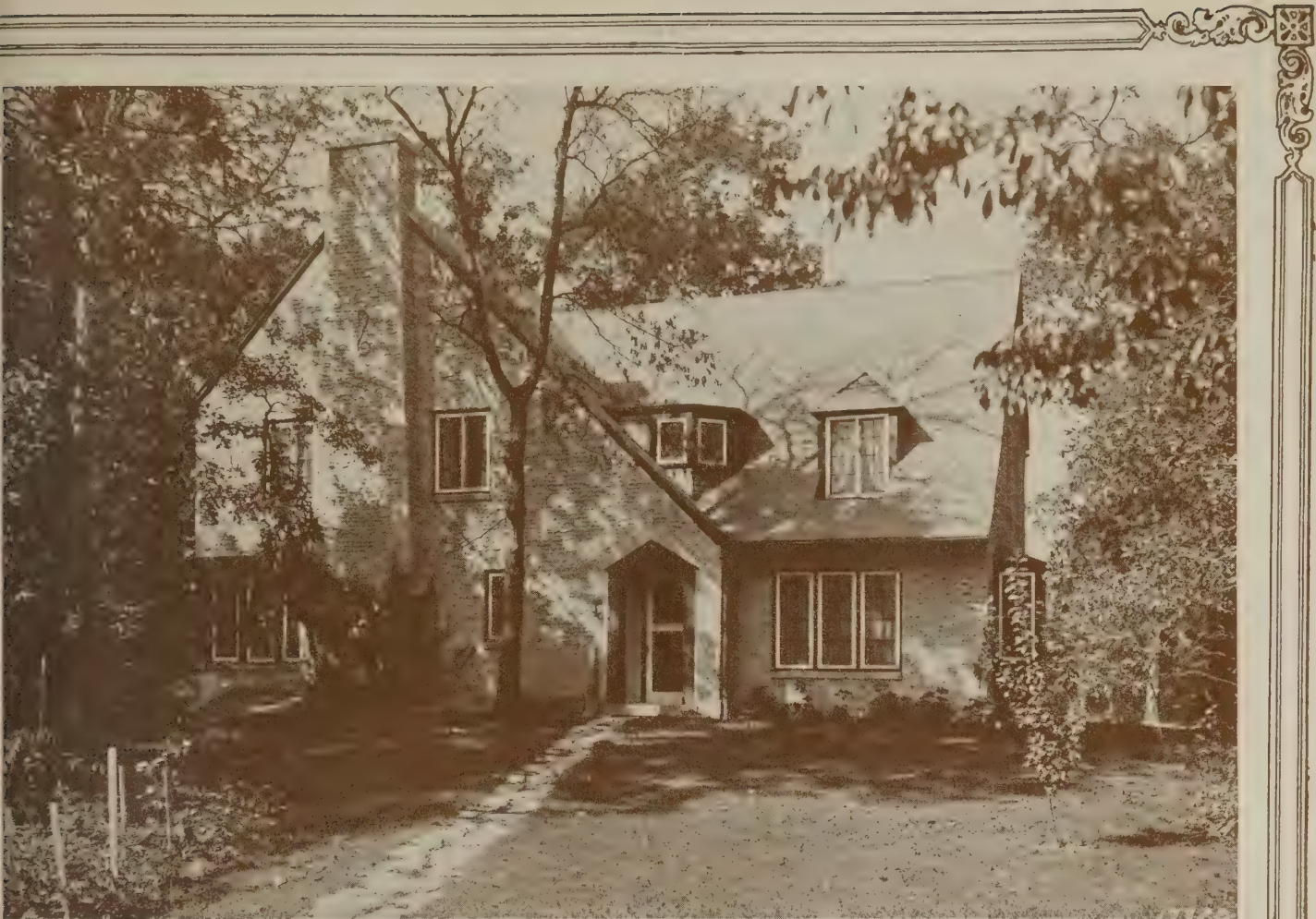
Built of Common Brick, with Rough Mortar Joints
