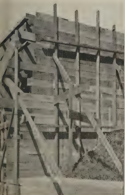
Formwork for the side wall
