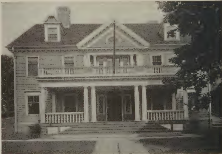
View of the old residence before remodeling
