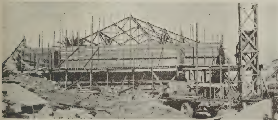
The truck in the foreground furnished the power for operating the hoist
