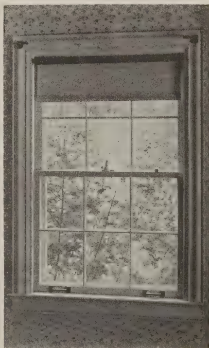
Sash lifts of this sort work better than the old thumb lift placed in the middle of the bottom rail. They equalize the strain on the sash. The sash fasteners draw the sash firmly together
