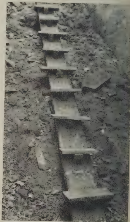
One plank and a few scraps make this stairway
