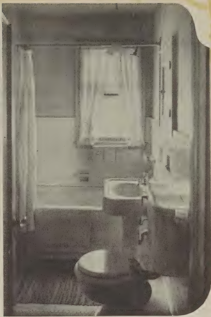
Left: The oil burner and the hot water heating plant. Note the water heater in the background. The oil burner was connected with the sewer when the house was built. Right: Tiled walls and floors, with built-in soap dishes, showers, standard tubs and pedestal lavatories, are found in the bathrooms
