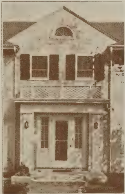
Detail of the entrance
