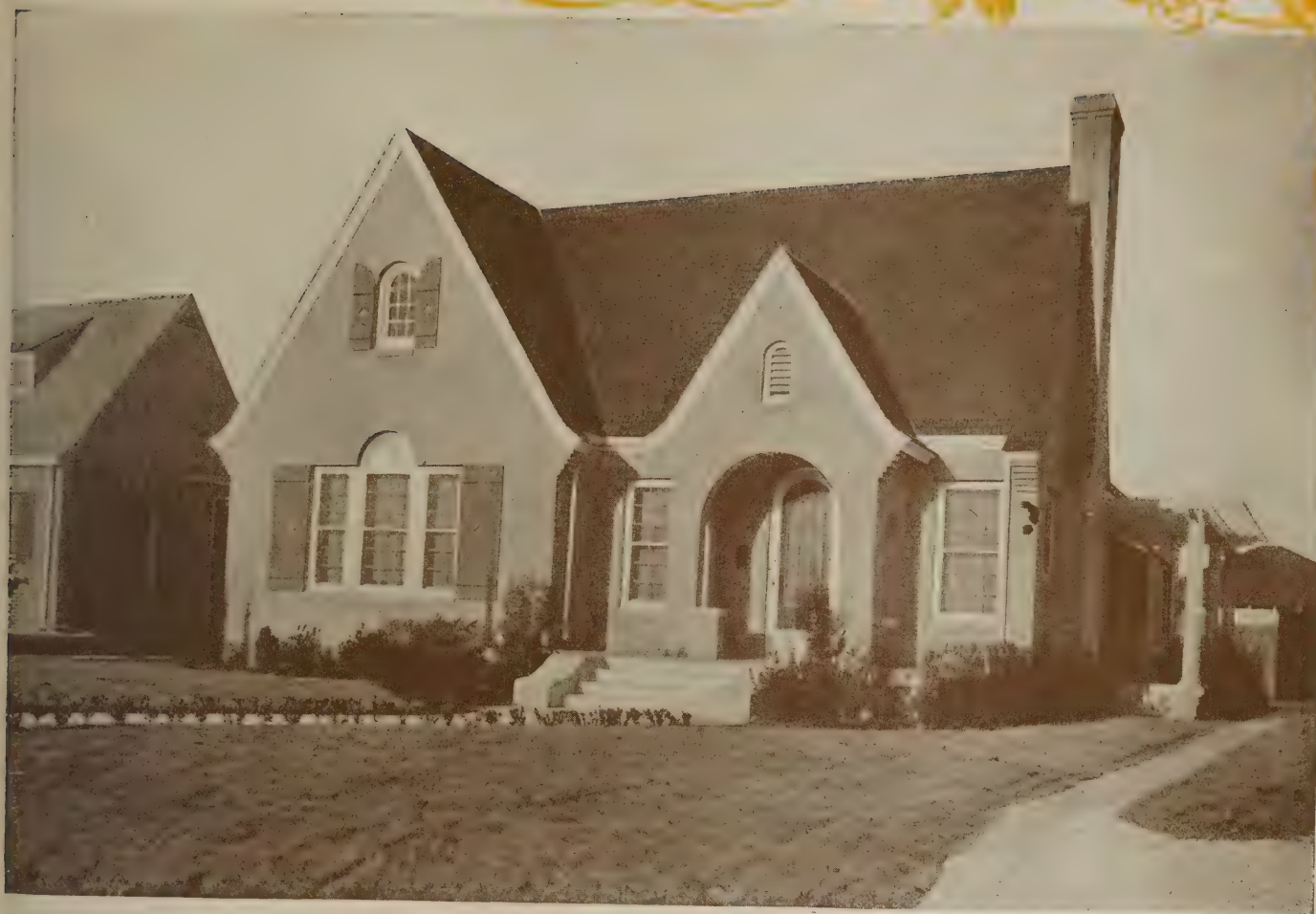
Repeating the lines of the main gable makes this entrance harmonious
