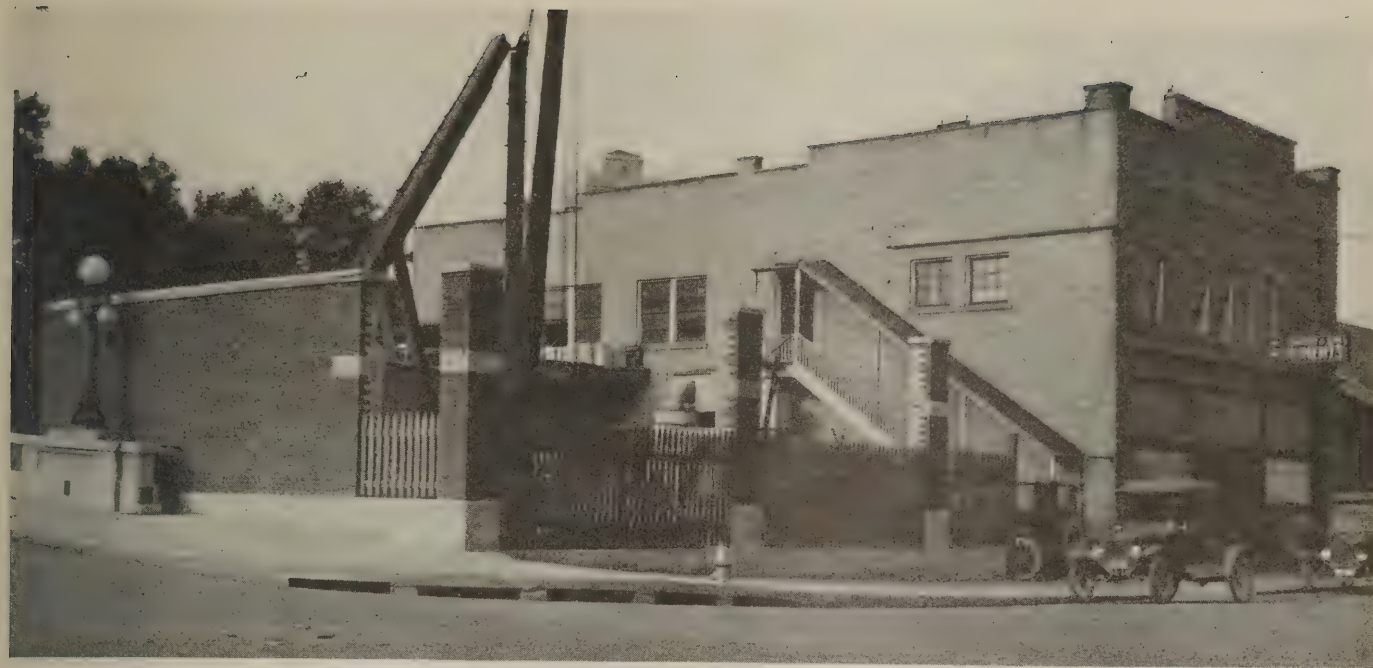
This is a view of the existing building and the stone-yard alongside. The stone-yard has been so constructed that when the wood part is removed the brick wall and piers can be utilized as a part of the store building to be erected
