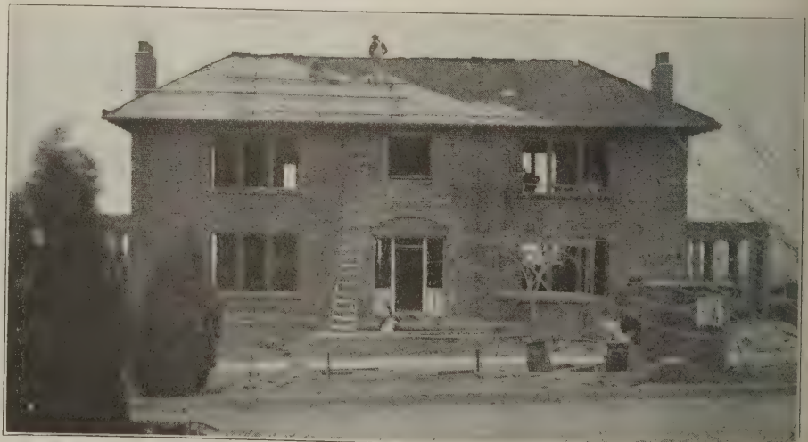
View showing workmen on roof. Note the absolute freedom from restraint provided by this scaffold
