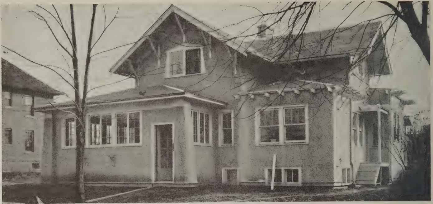
This is the stucco house, which was moved without cracking the stucco, as it stands in its new location. The light vertical streak near the center of the building is where the two sections into which the house was cut were joined after moving
