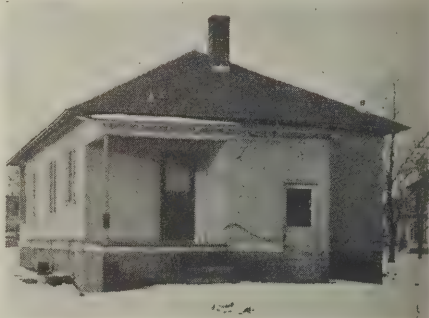
Rear view showing enclosed porch
