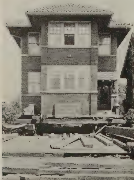
This view shows the house in place on its new foundation
