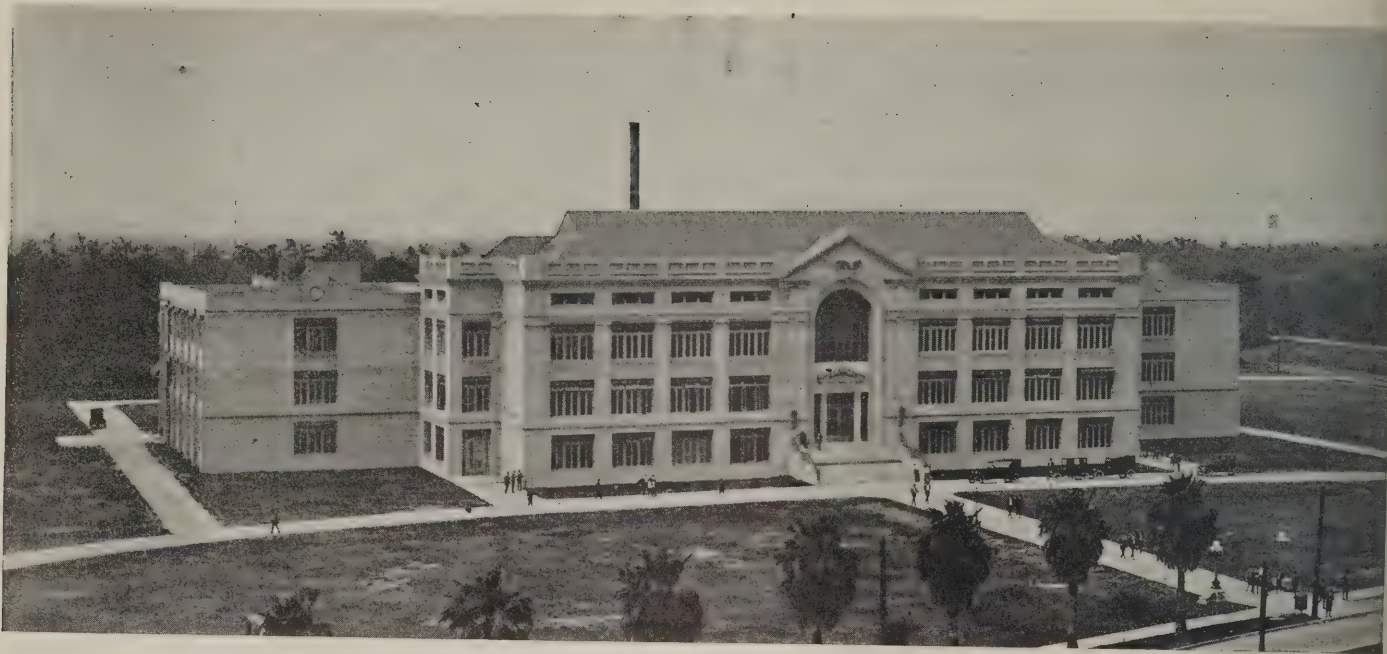
The Isaac Delgado Central Trades School, New Orleans, Louisiana
