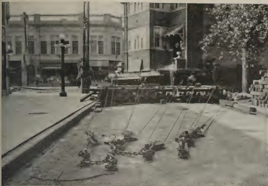
Since no means of holding the load line pulley was available they were fastened to stakes driven into the pavement
