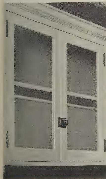
Cupboard latches are to be had in a number of finishes—brass, oxidized copper, black japanned. They should be as small as consistent with the size of the door. Notice the placing of these
