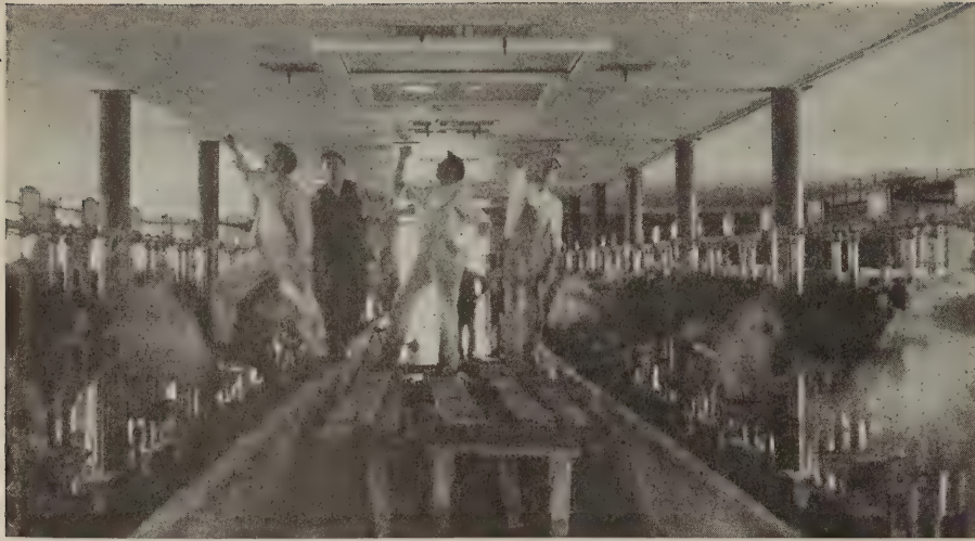
"Asbestone Everlasting" magnesite stucco being applied to the ceiling of a dairy barn
