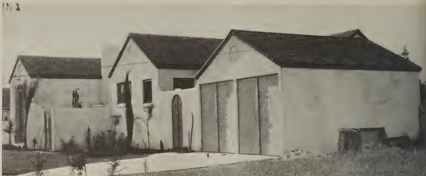
From the standpoint of appearance, the doors are the weak point in most garage designs. In the above group, however, the garage doors, with their carved astragals, are made attractive features
