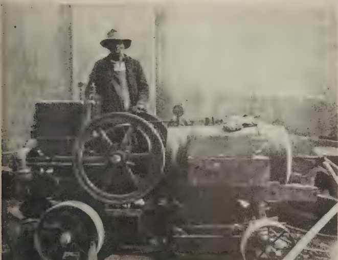
Air compressor used to furnish power for the air drills
