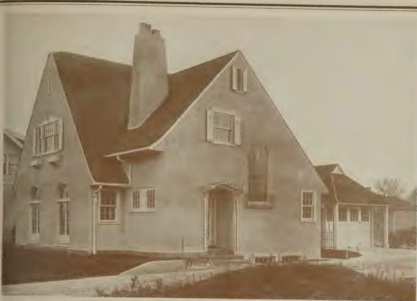
The decorative window at the stair landing is an important feature of the design
