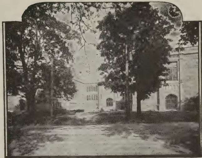
Roscoe Conkling School Building, Utica, N. Y. Kinne and Frank, Mayro Bldg., Utica, N. Y., Architects
