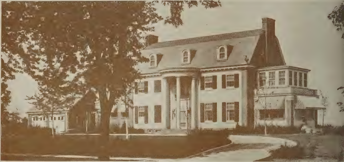
The west facade showing the house as it is viewed from the street. The entrance portico, with columns of two-story height, is a distinctive feature
