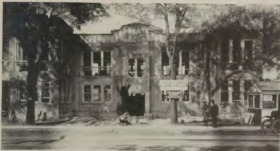
Charlton Apartment Building. Started November 12, 1921. Progress as of November 21, 1921
