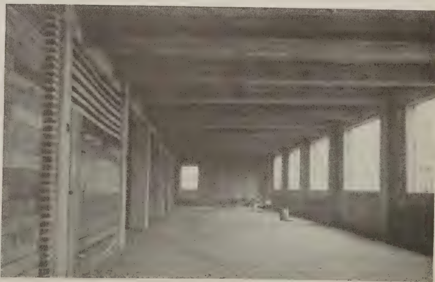
Finished room, showing that columns and girders "line up"
