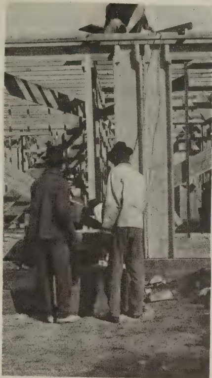
Placing concrete uprights in position
