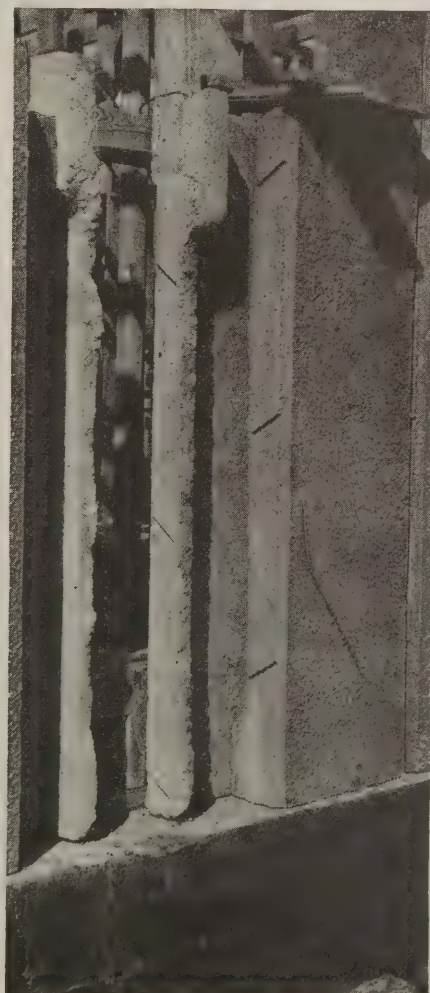
Near view of slabs in place
