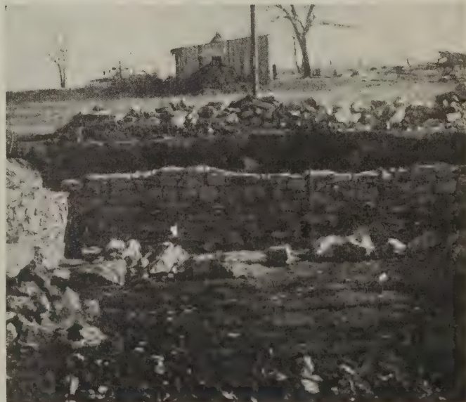
Cellar walls are invariably built of rough ashlar laid in cement mortar
