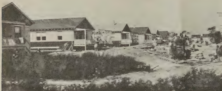
Other views of the bungalow development
