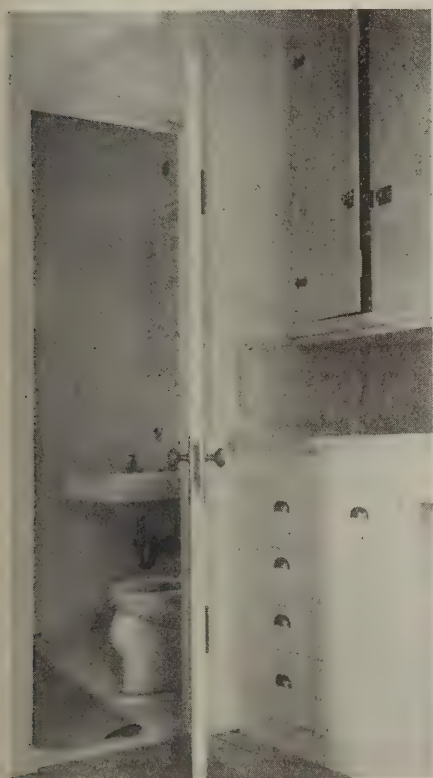
Fig. 22—Magnesite floor laid in bathroom and magnesite drain-board in kitchen sink. The sink is in combination with cupboard, flour-bin and drawers
