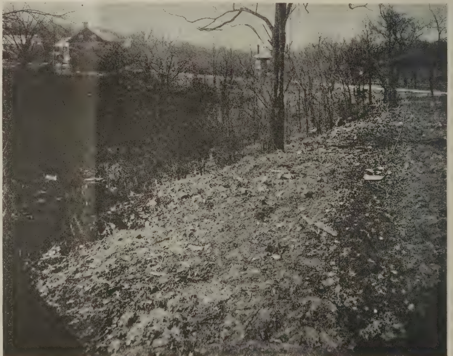
The building site used for the Forest Glen Apartments
