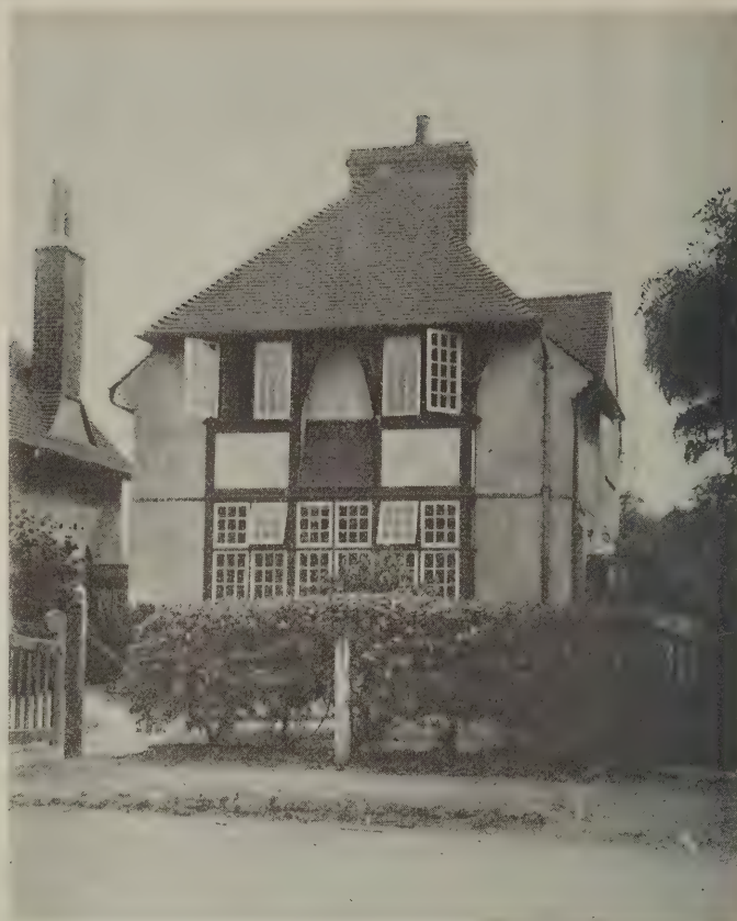
Timber framed and stucco filling for a small house The window in the front projects about 18 inches
