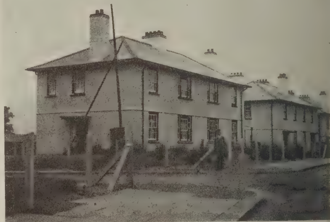
Six-apartment double houses built with brick and stucco. Slate roofs
