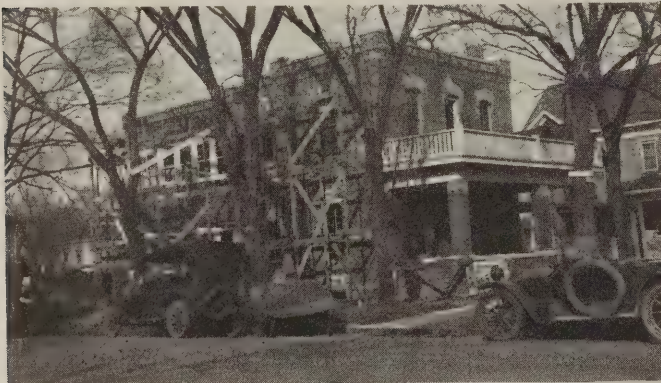
Old brick house, Topeka, being made over into two-apartment building
