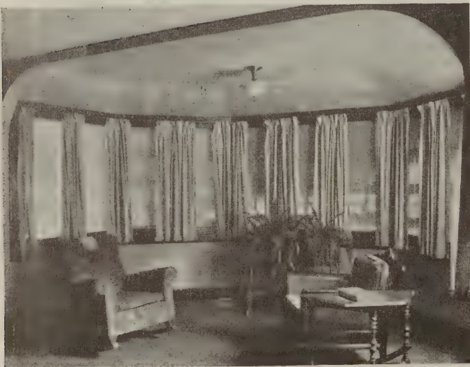
The sun parlor at the front of the house is an alcove off the living room. Notice its plaster arch and the domed ceiling. The drawn shades hide the windows, which are all small-paned casements, opening outward
