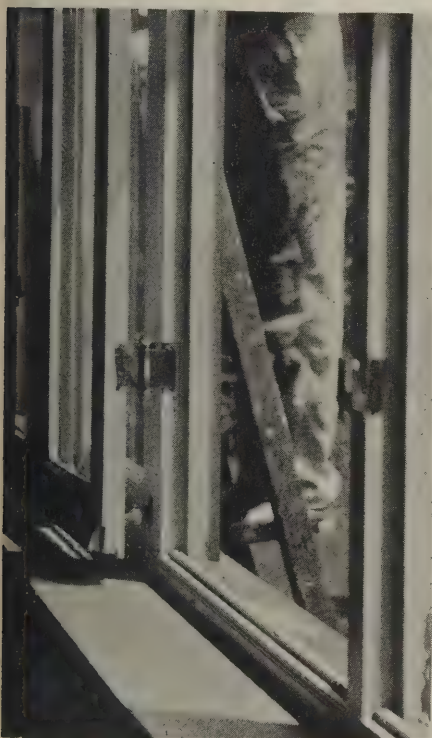
These hinges permit opening of the windows without removing the curtain rods
