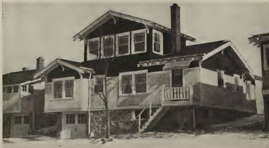
Back view of 5716 Locust street
