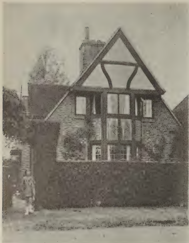
Timber framed bay window with brick filling and stucco gable
