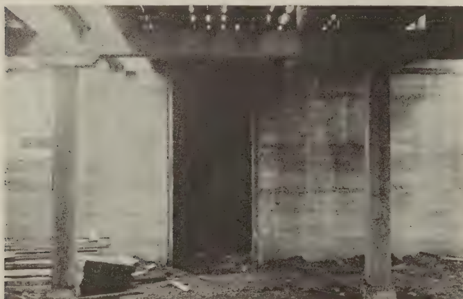
Post and floor construction in Naperville barn and entrance to vault under driveway
