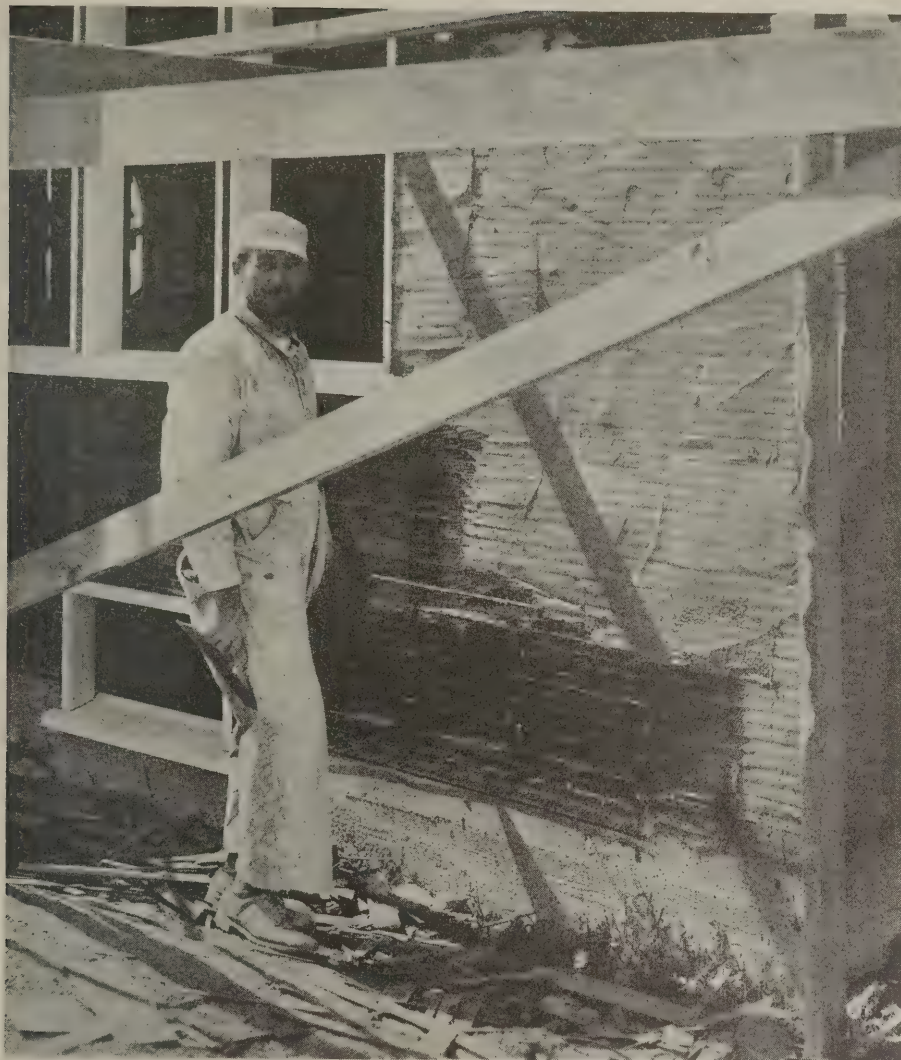
Showing metal lath with first coat of plaster
