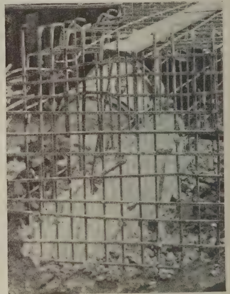
Half to three-quarter inch reinforcing rods on 8 in. centers were rapidly cut with the concave chisels on the paving breaker
