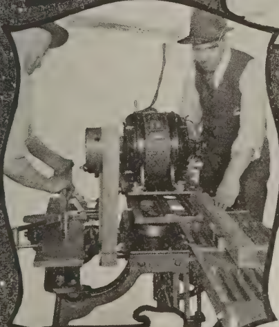
Ripping and Jointing
