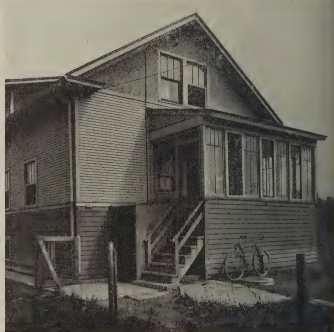
This rather unattractive rear porch was improved at a small expense
