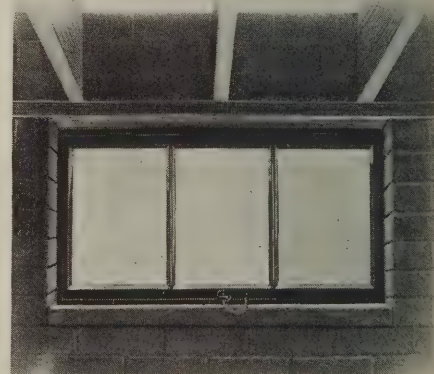
Steel basement window
