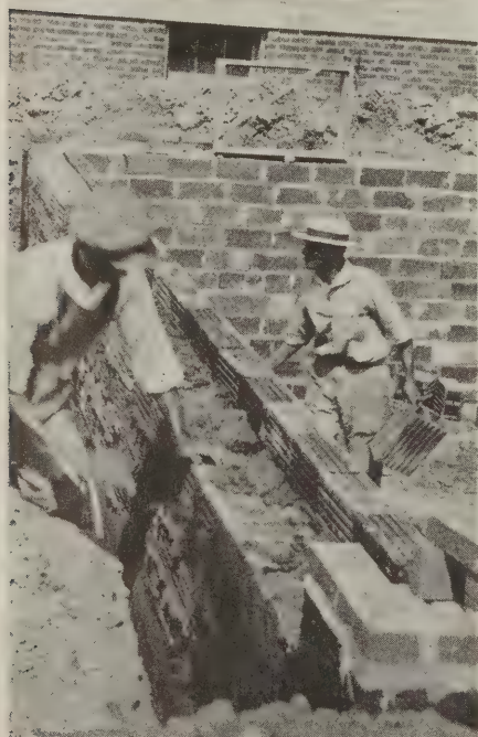
Method of laying hollow-tile cellar walls in Cleveland, Ohio
