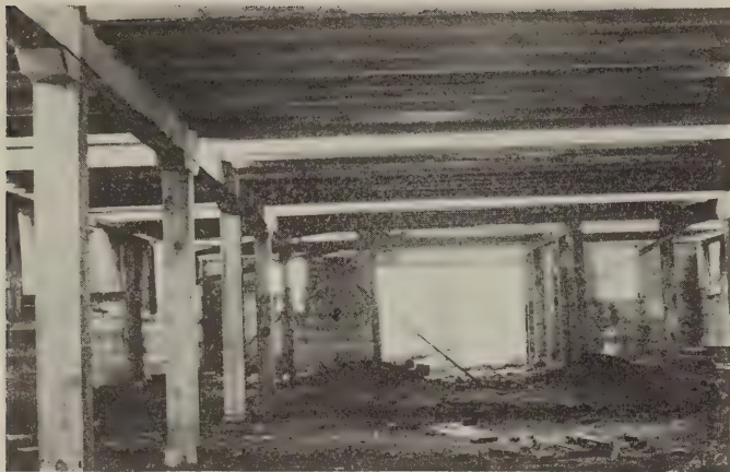
Basement view during construction
