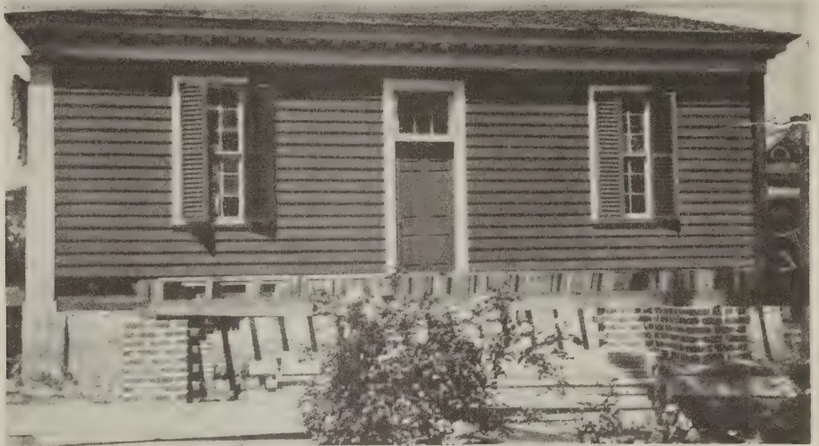
A 125-year-old building still worth all it cost
