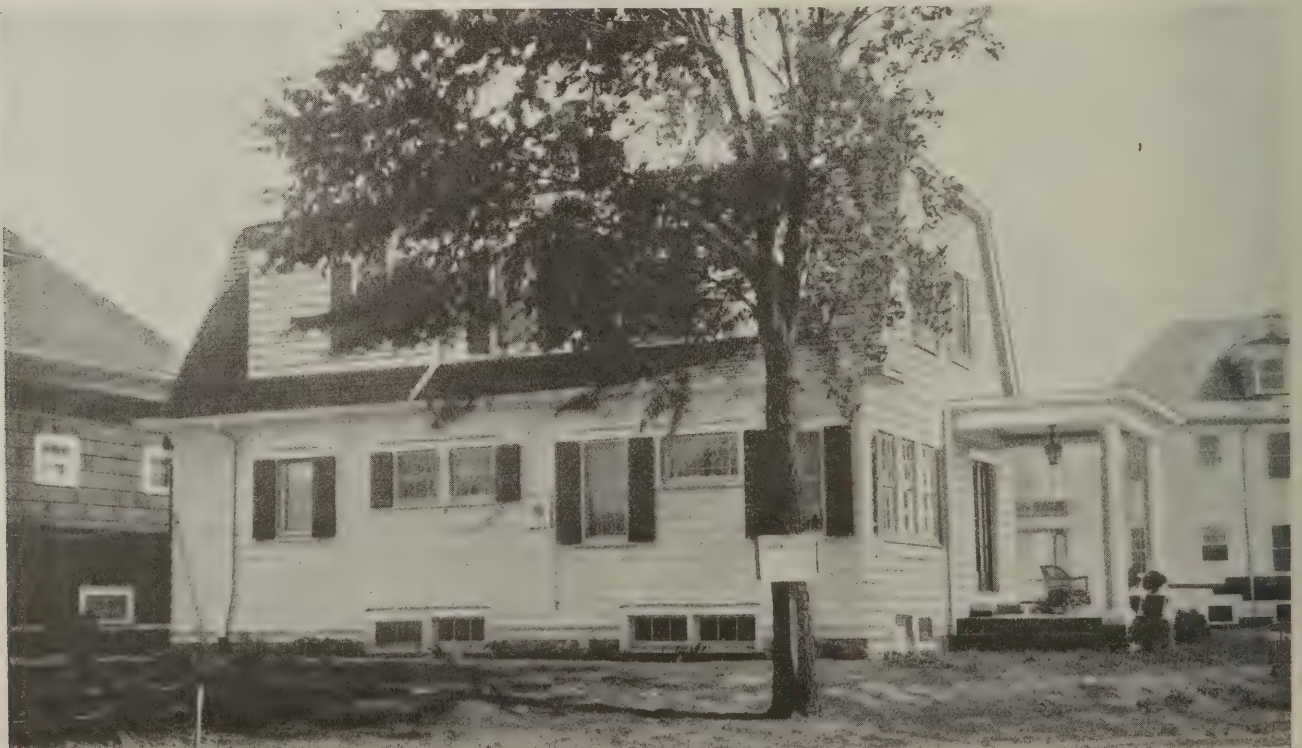
Model electrically equipped home, Buffalo, N. Y. See another elevation in Style Sheet, page 36
