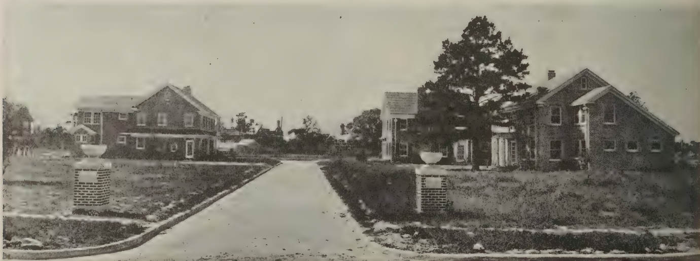
A community development in Houston, Texas
