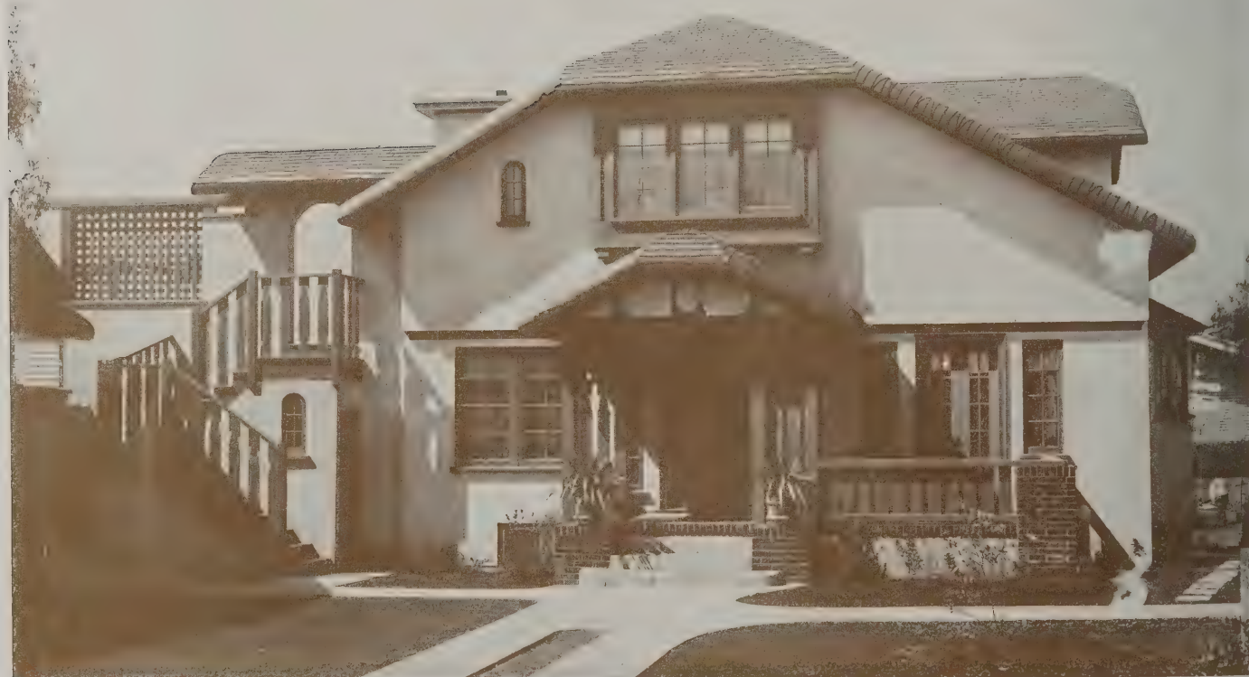
A two-story bungalow in Southern California
