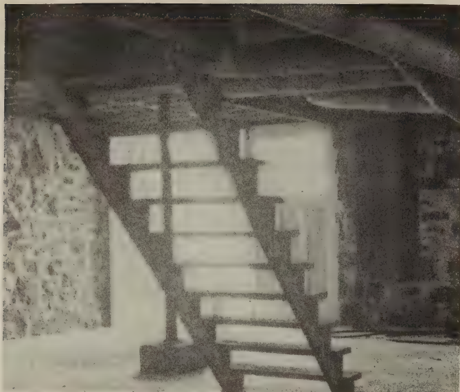
Cellar-garage detail showing clothes chute and entrance
