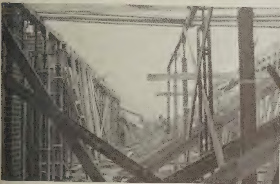
Forms for roof in place, showing special type of shoring
