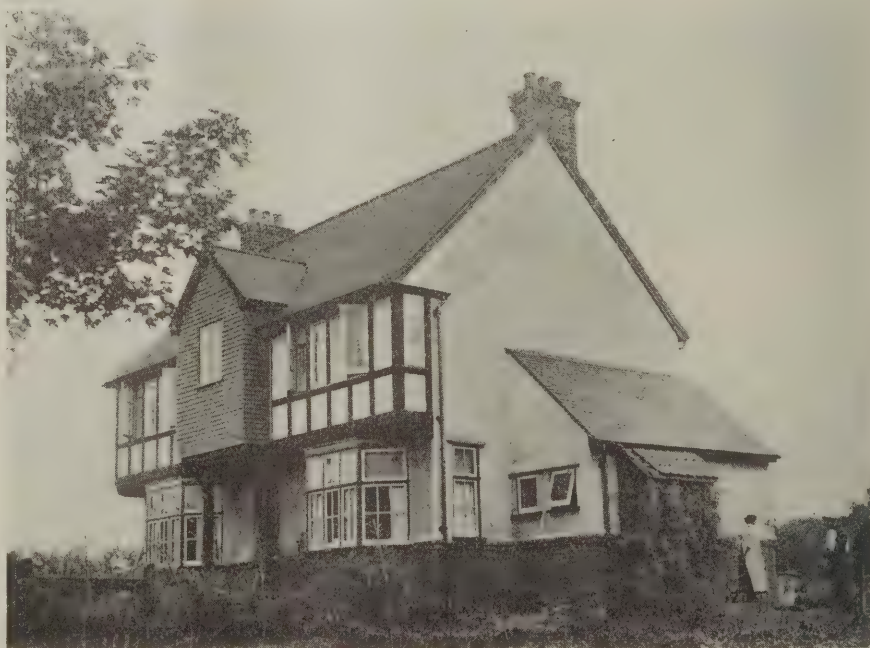
Timber framed and stucco wall of upper floor. Note how the timber framing projects over the bay window of the ground floor
