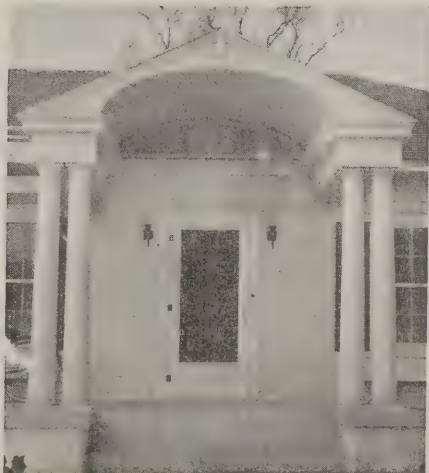
Detail of entrance, House No. 127, page 36. All house numbers are of tile, blue figures on a white ground
