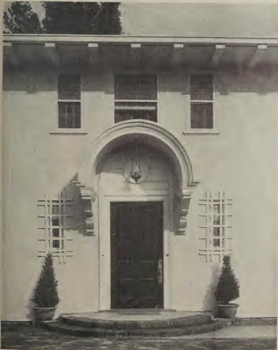
Fig. 2—Entrance to a stucco house
