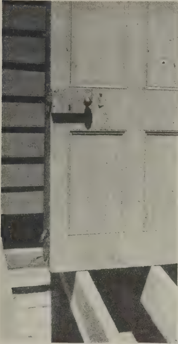
Home-made doors and colonial hand-made hardware
