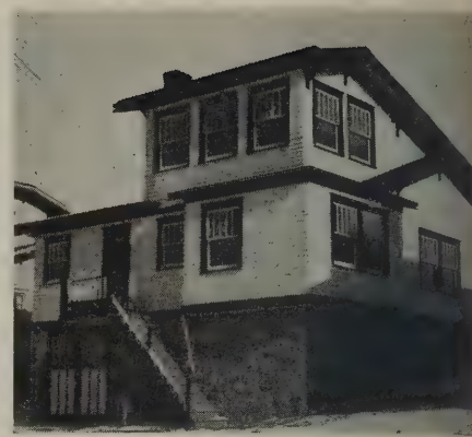
Back view of 5708 Locust street
