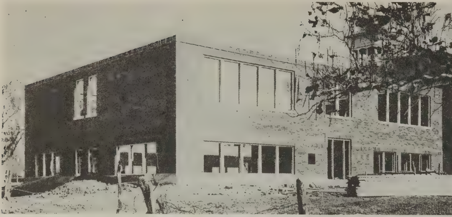
Progress photograph, November, 1921—Rear
