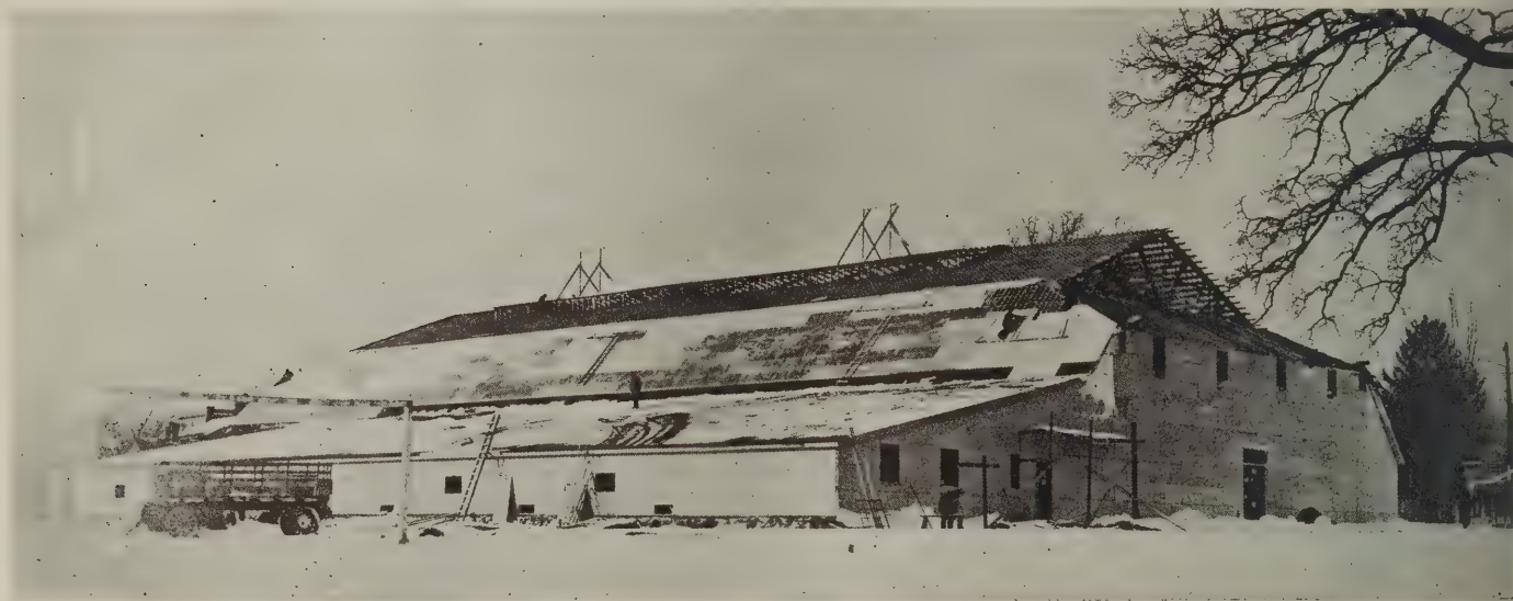
Arena at Paris, Ont., Canada—Wood frame, and plaster board and stucco
