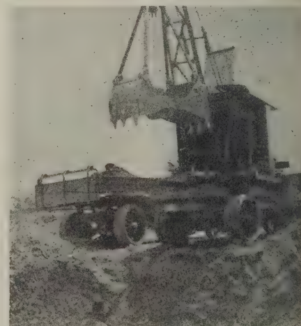
Motor-truck crane dropping the clam-shell bucket to get a grip in hard material
