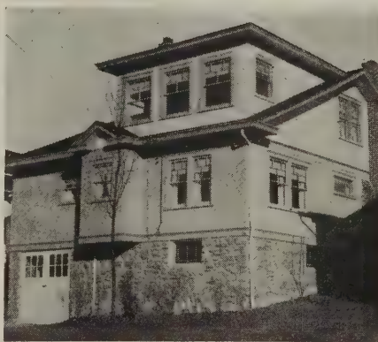
Back view of 5712 Locust street
