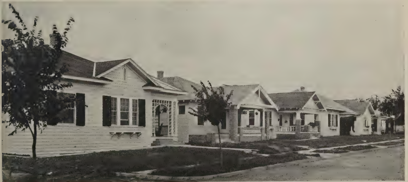
Another view of Eckert houses on Dumont street
