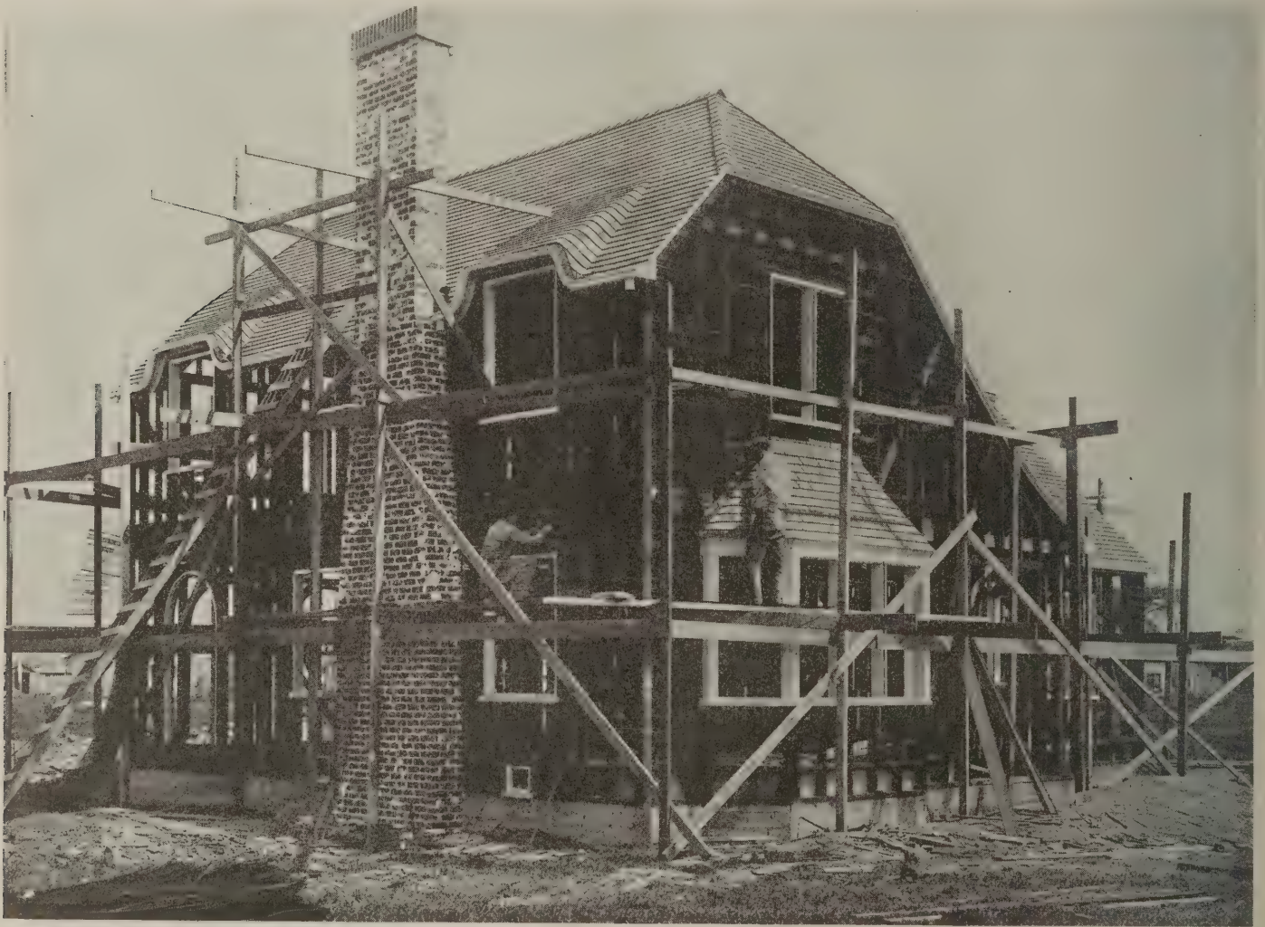
Residence in Stockton, Calif., showing application of metal lath direct to studs without sheathing boards. Hurtzig & Orcutt, general contractors; Perry Bros., plastering contractors
