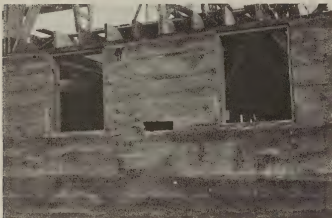
Provision for ventilation in concrete foundation walls
