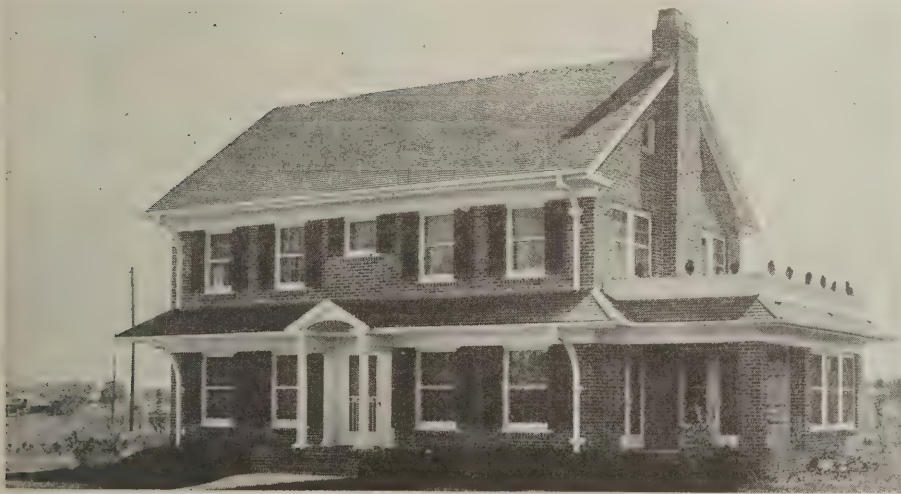
R. W. Henderson residence—one of the community development houses
