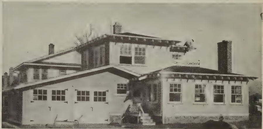
Back view of 5730 Locust street
