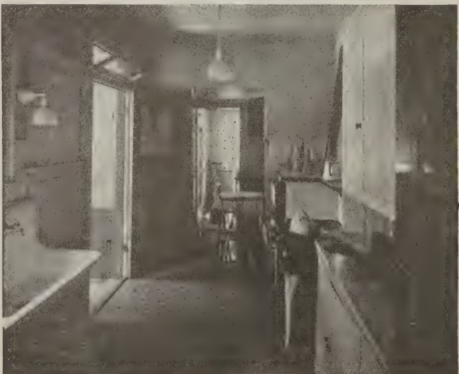
The kitchen of the stucco bungalow is conveniently arranged. A small drop-leaf table in the jog in the wall serves as a breakfast alcove
