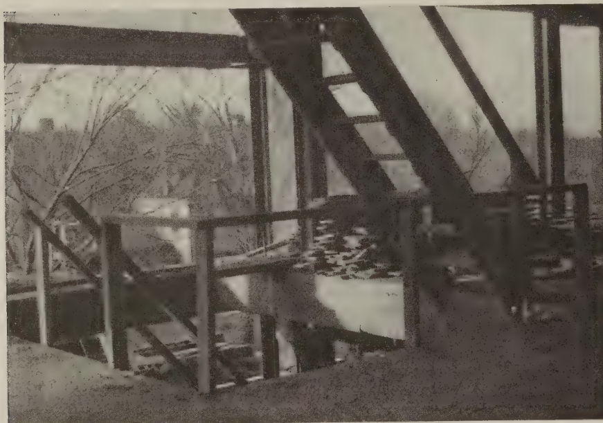
Stair wells and stairs for insuring safety and efficiency of workmen
