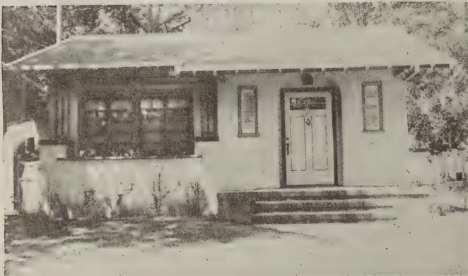
Front view showing detail of entrance
