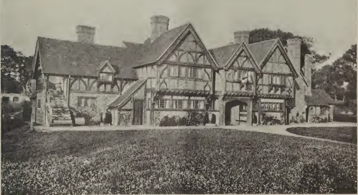
House in Hampshire. Timber framing with brick work filled into the panels
