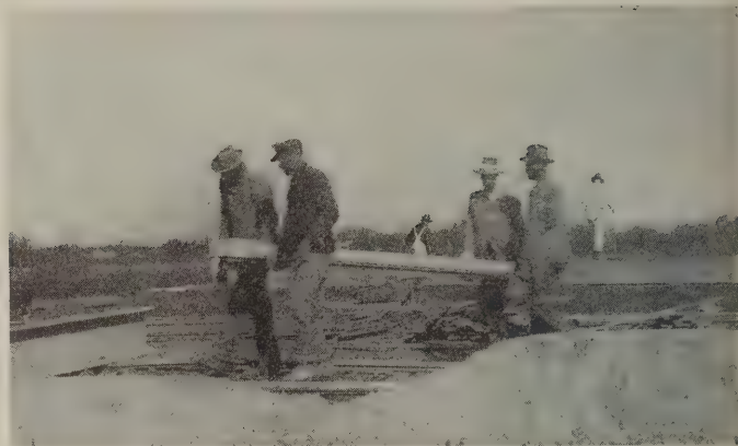
Stacking the concrete lumber on the job
