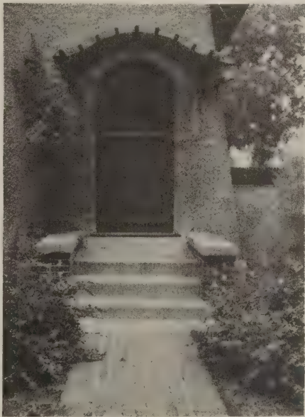
Doorway to house No. 6, page 35. An open trellis is above it. Note the hinges that extend across the entire width of the door
