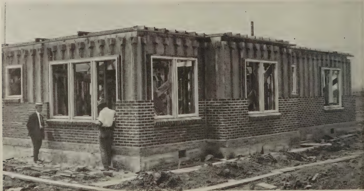
Concrete bungalow with brick veneer
