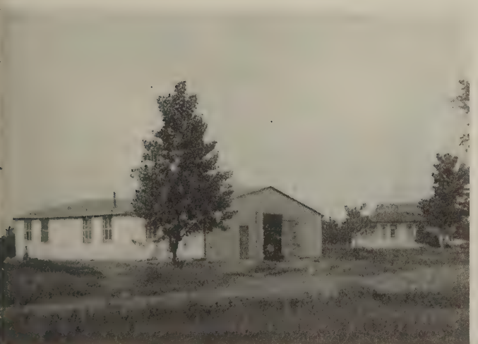
Because of the scale on which the Jos. E. Jones Co. are building, they have erected this temporary warehouse on the property to take care of the large quantities of materials that are delivered and in which to do special work
