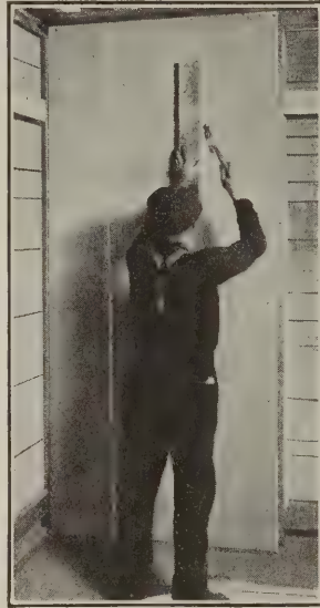
Fig. 4—Applying the wallboard over the fasteners, using a piece of 2x4 with rounded corners to avoid marring the panel. A few blows of the hammer on the 2x4 placed on the wallboard over the fastener clinches the prongs in the board and leaves a smooth, unbroken surface
