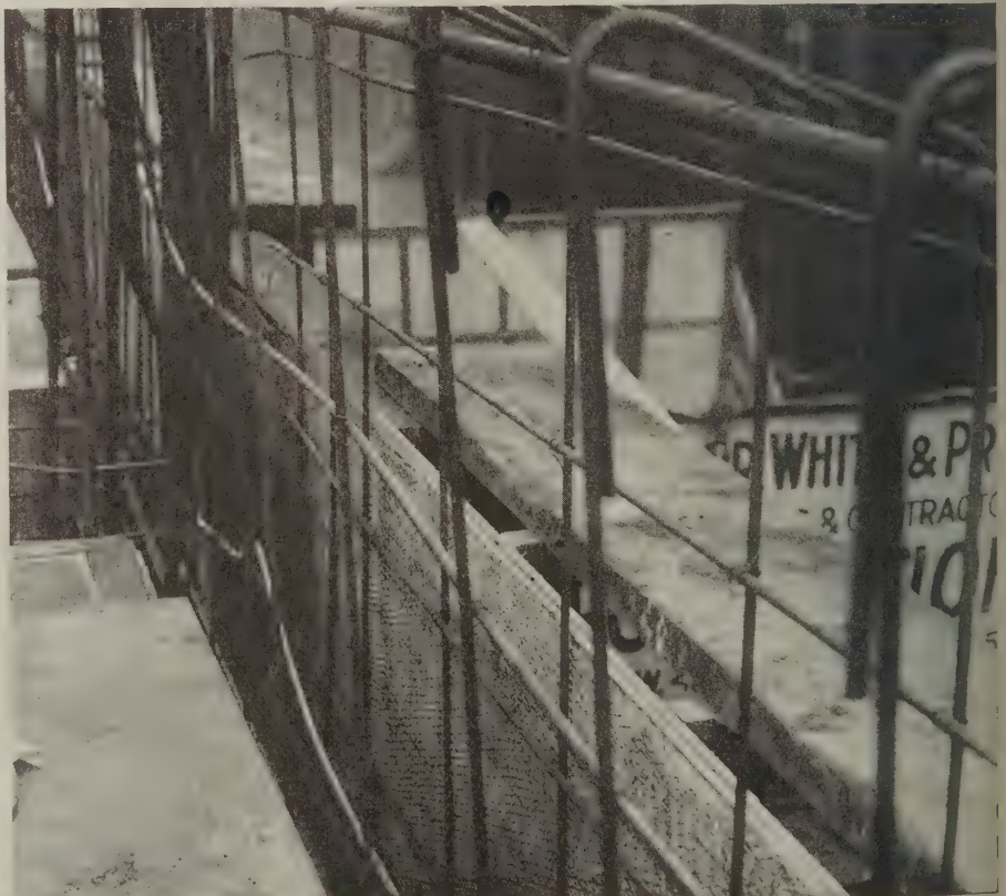
Ready for pouring the special facing concrete. Note expanded metal attached to reinforcement
