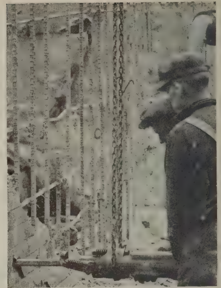
The "paving breaker" can be operated by one man but two men and other aids, such as the improvised chain support, expedite the work
