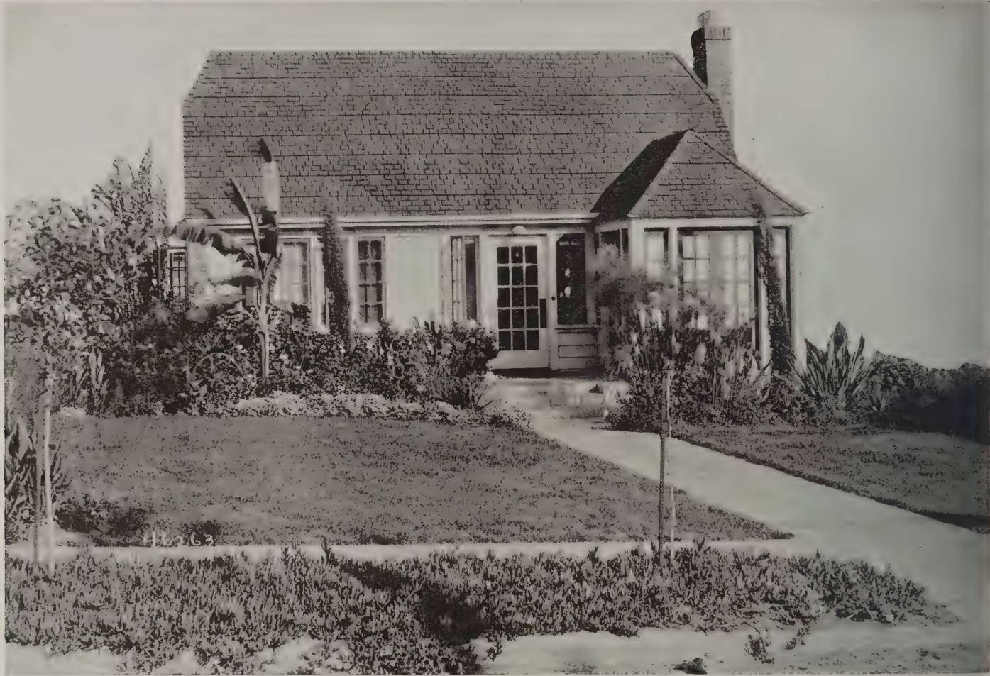
A high-roofed bungalow in California—the higher the cooler
