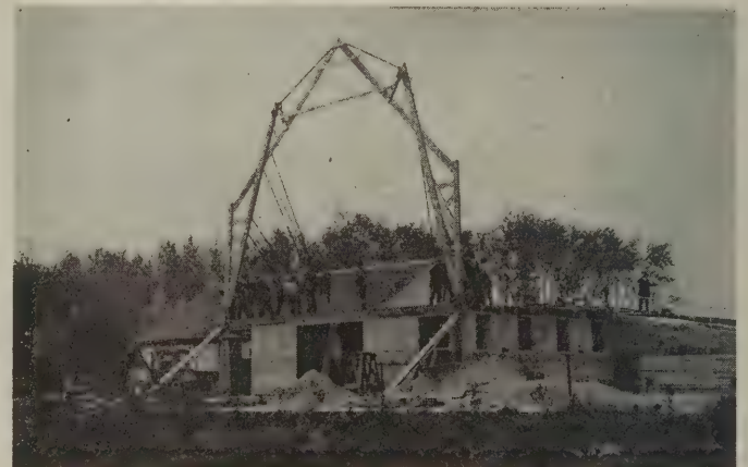
Preliminary plumbing of first bent
