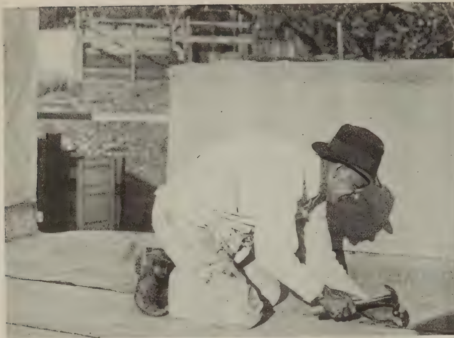
Fig. 16—Laying the waterproof deck of heavy roofing paper over garage. Underneath is caulked with pitch. Magnesite floor may be installed later
