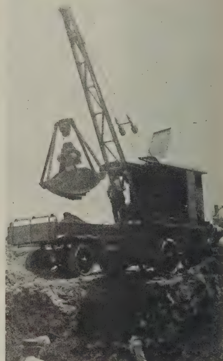
Motor-truck crane for cellar excavation, Cleveland, Ohio
