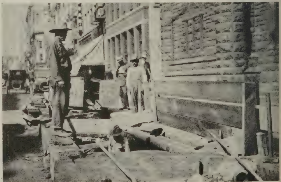
Illustrating a satisfactory method of protecting an excavation from being flooded. The pipe extends across the hole and is sufficient to carry all water that may flow along the gutter without interfering with the work or permitting water to back up
