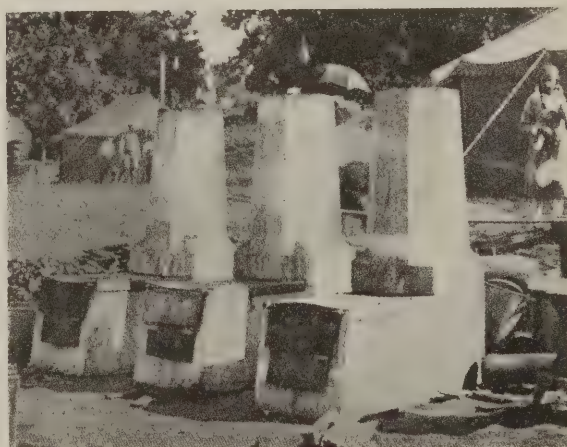
Fig. 6—Small concrete cook stoves arranged around a concrete chimney afford convenient means for preparing meals. Concrete block may be substituted for poured concrete in the construction of these stoves, if desired
