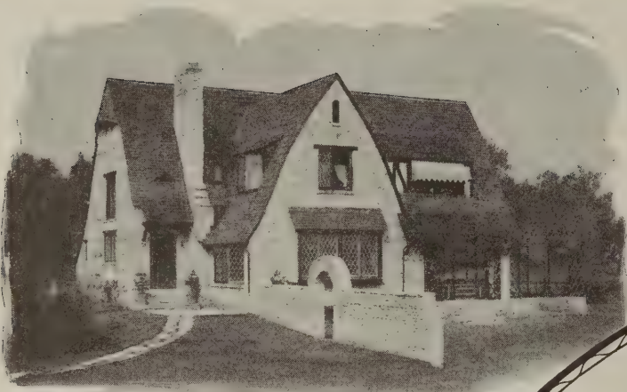
Residence of S. S. Beman, Winnetka, Ill. Celotex used for in- sulation on all walls, under ex- terior finish and under roof rafters.
