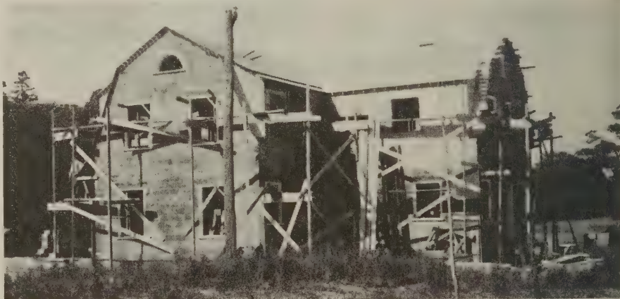
House made from coal-ash concrete
