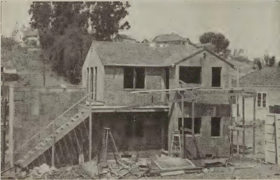
Fig. 7—Rear view of building showing button lath and wire reinforcing in place
