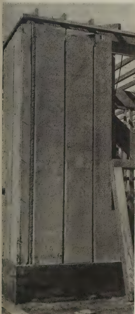
Corner with slabs in place
