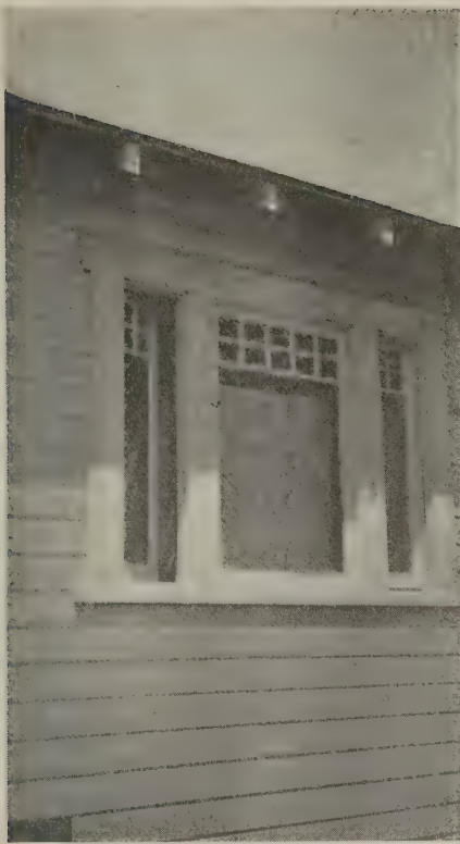
The window before being screened
