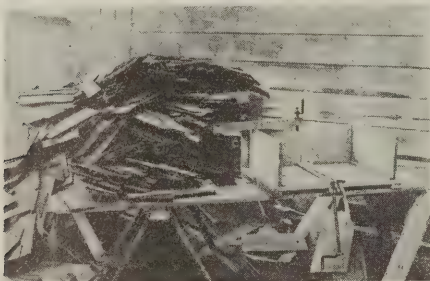
Typical pile of broken shingle bundles
