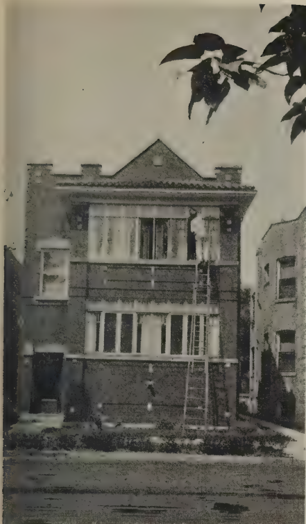
Enclosing these porches adds one room to each flat
