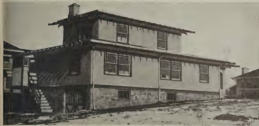
Back view of 5702 Locust street
