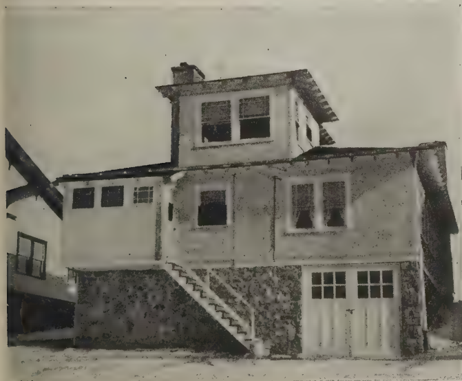
Back view of 5710 Locust street
