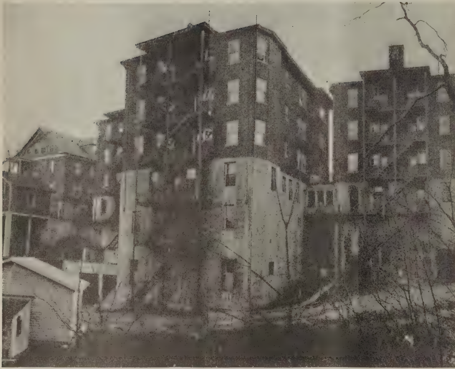
Rear view of Forest Glen Apartments, showing the $25,000 reinforced concrete wall
