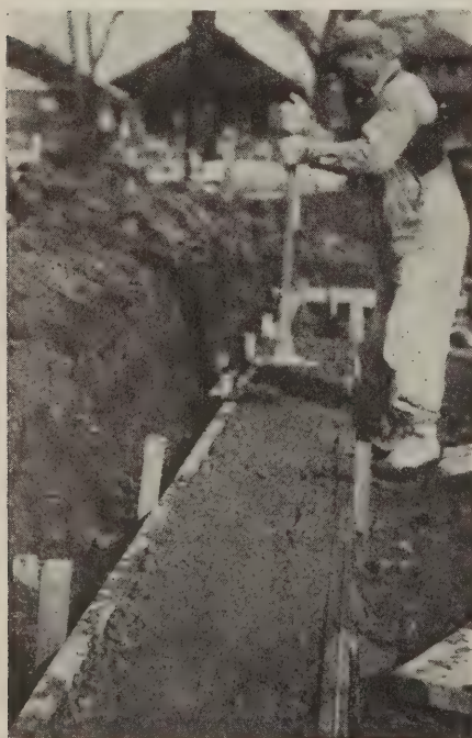
Fig. 2—Placing footing 15 in. in width for 8-in. foundation wall of concrete block
