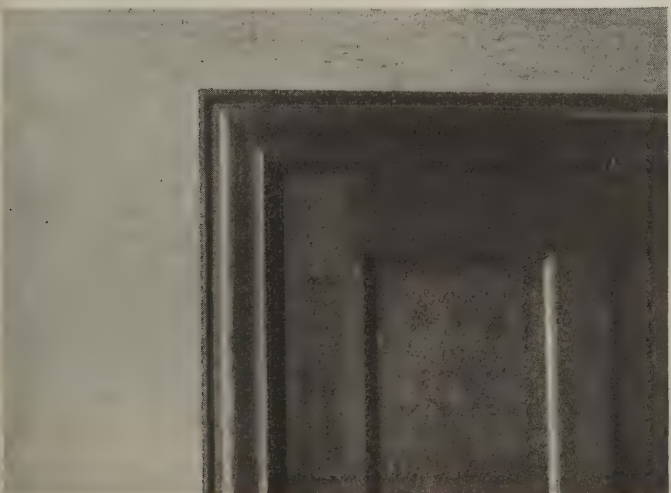
Detail of the trim used downstairs. It is finished with Early English Stain, very dark, and rubbed to a dull finish. Note the excellent workmanship on the mitred joint
