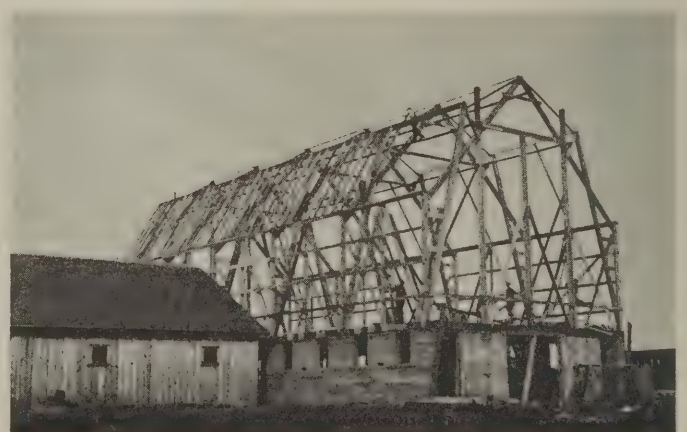
Bents all erected and all ties and struts placed
