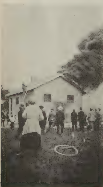
Fire test of gypsum stucco house with wood supported members
