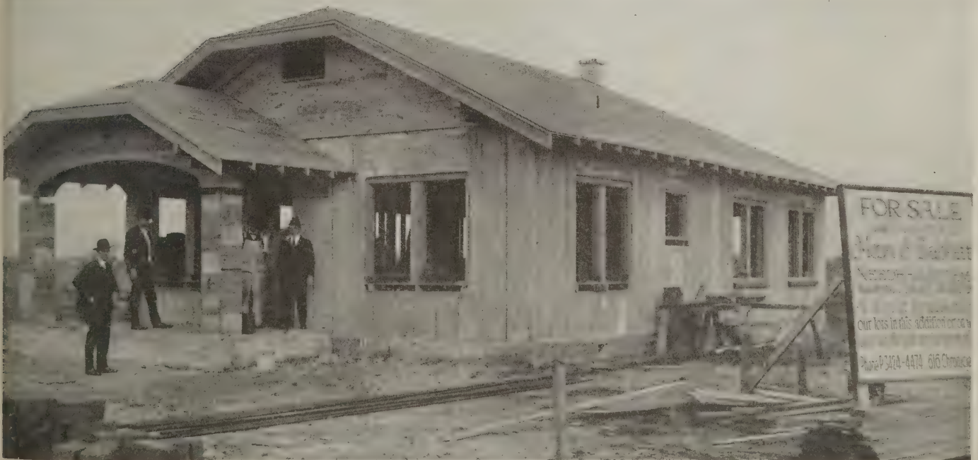
Bungalow roofed and ready for stucco finish
