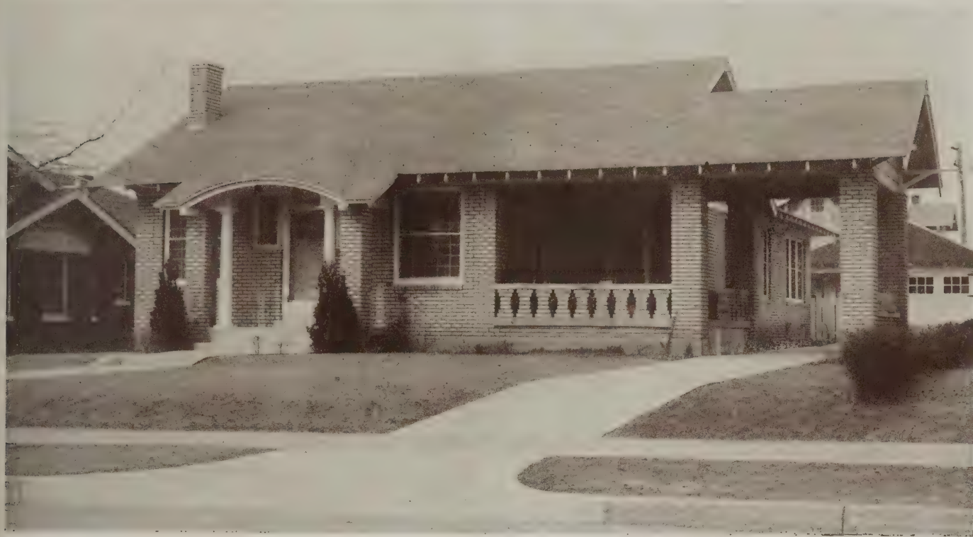
Bungalow in Munger Place. A. R. Eckert, designer and builder, Dallas, Texas
