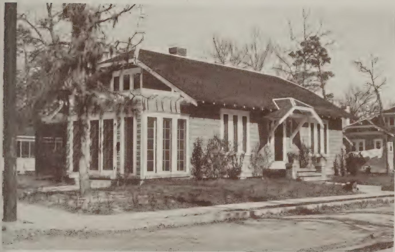
Bungalow. Bell Construction Co., Houston, Tex. See additional views and plan as House No. 2, page 29
