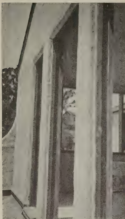
Fig. 12—The scratch coat in place
