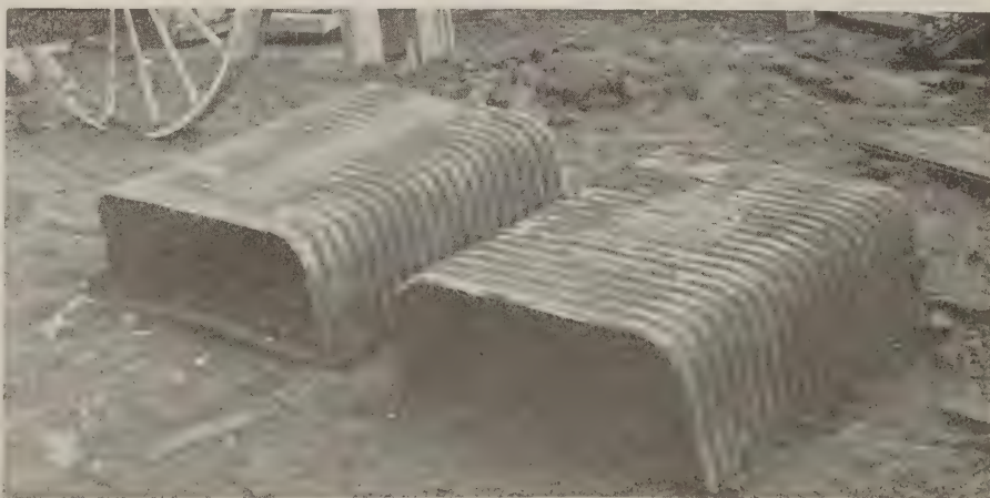
Steel "dome" forms for floor construction of God's Bible School
