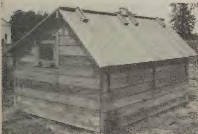
Fig. 2—Combination roof hog house with the doors and windows closed for winter time. The side walls are made as nearly wind proof as possible
