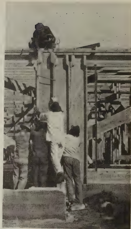
Placing concrete uprights in position
