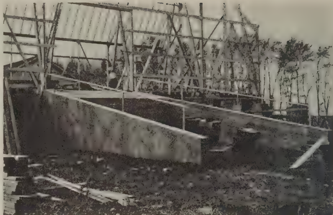
Main entrance to barn floor showing concrete retaining walls for fill and back of wet-feed vault
