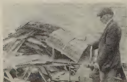
The bundle completed and the screws pressing the shingles together so that bands may be nailed to cross pieces
