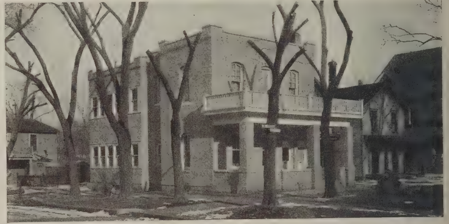
Completed job—Old brick dwelling becomes modern two-apartment house
