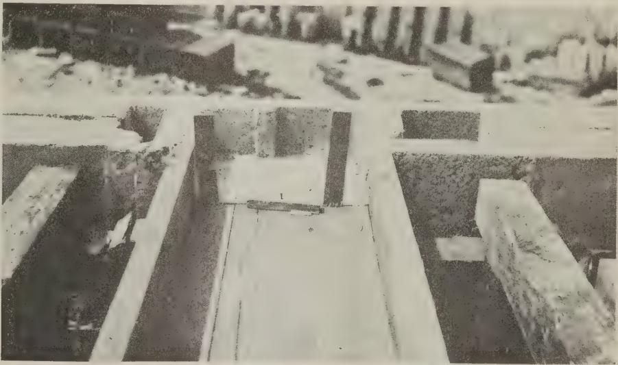
Fig. 28—Forms for concrete floor beam, showing recess left in block wall to receive the beam
