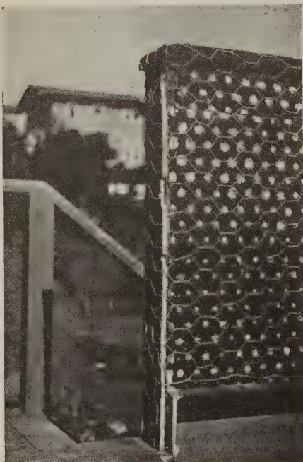
Fig. 8—Button lath, reinforcing and flashing
