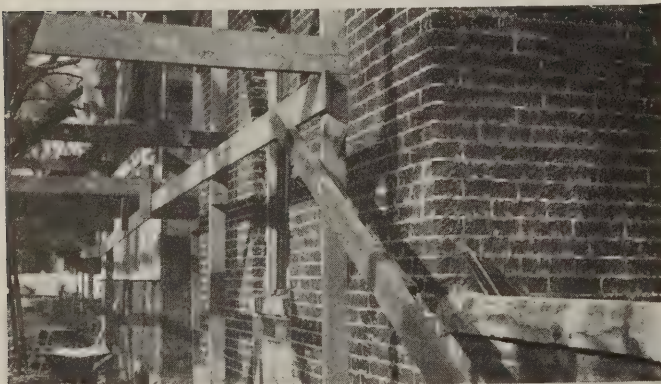
Brickwork prepared to receive the stucco surface
