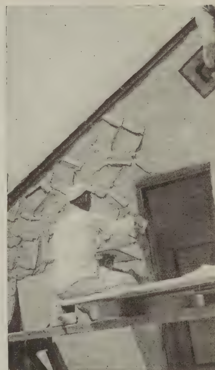
Fig. 15—Applying the "jazzy" effect of Mission texture. Edges have to be smoothed off
