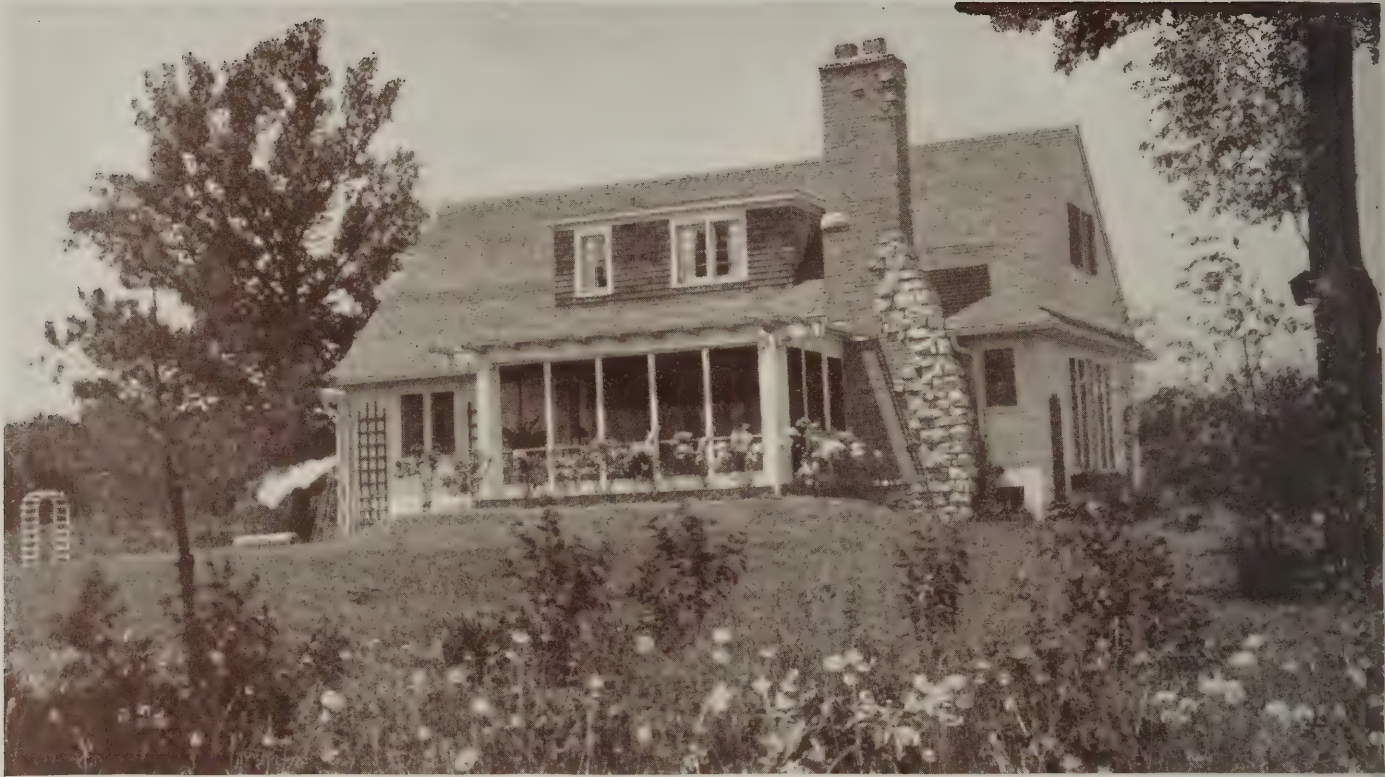
An unusual location and treatment of the chimney—matters that should be handled with care. A distinct suggestion of the colonial is seen in this bungalow
