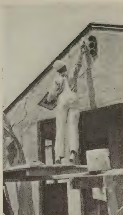
Fig. 14—Applying the finish coat
