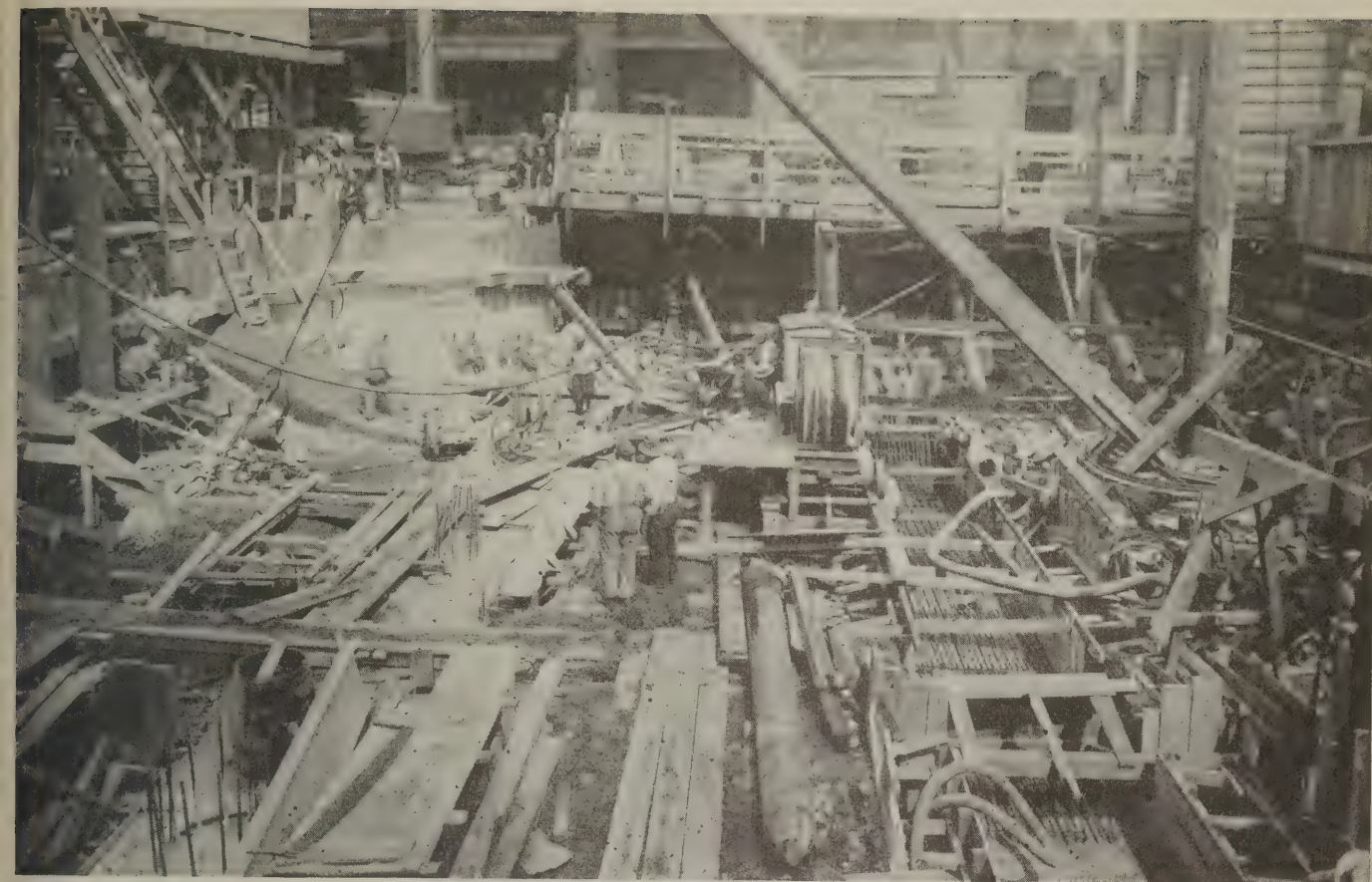
Basement, showing the method of jacking down the pre-test piles
