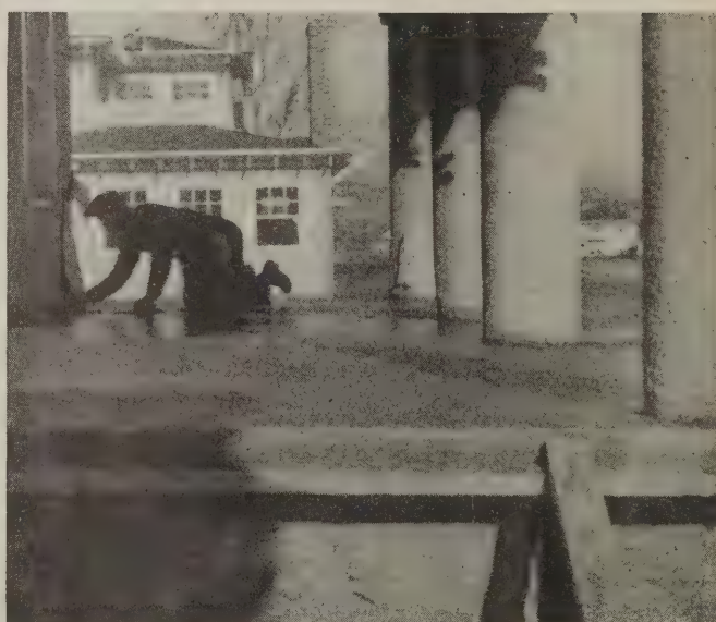
Finishing a concrete porch floor
