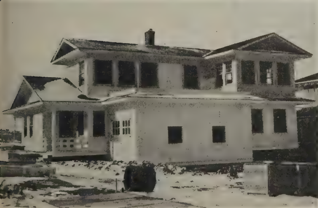
Back and side view of 5731 Oak street
