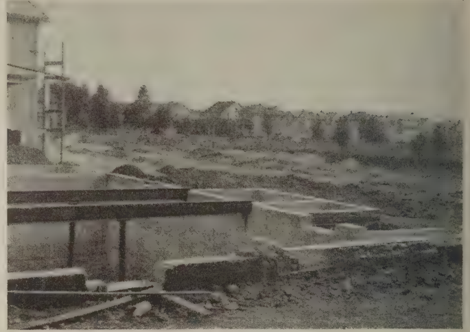
Steel beams and steel posts support the houses themselves. These steel members cost only $28 more per house than wooden beams and posts would have cost, and they make an effective "talking point"
