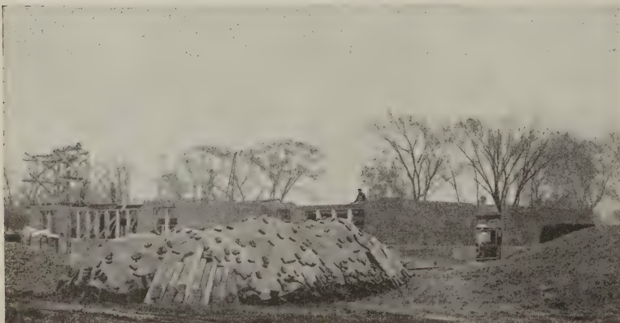
Winter construction. Face brick protected from frosty weather by tarpaulins
