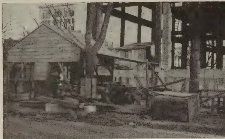
Gasoline engine driven saw mill for building form sections
