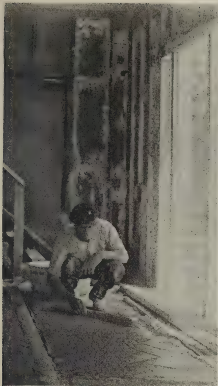
Fig. 1—Evening-off an Insulex pour. Note the slabs in the wall studdings
