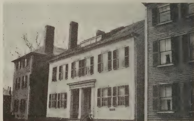
An old double house. The front is covered with wide, matched boards
