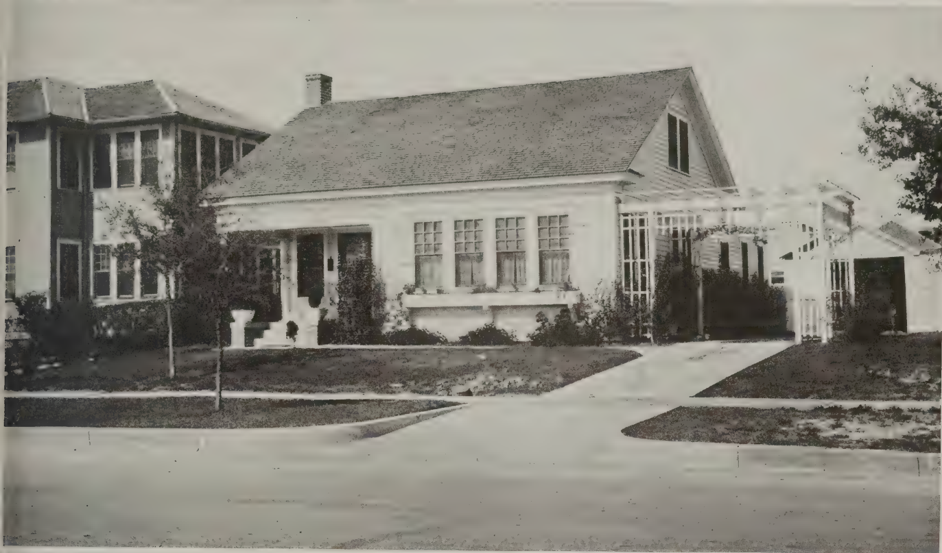
Attractive story-and-a-half house in Houston, Texas. Small but "homey" looking—due probably in some degree to the shrubbery. Wood shingled roof
