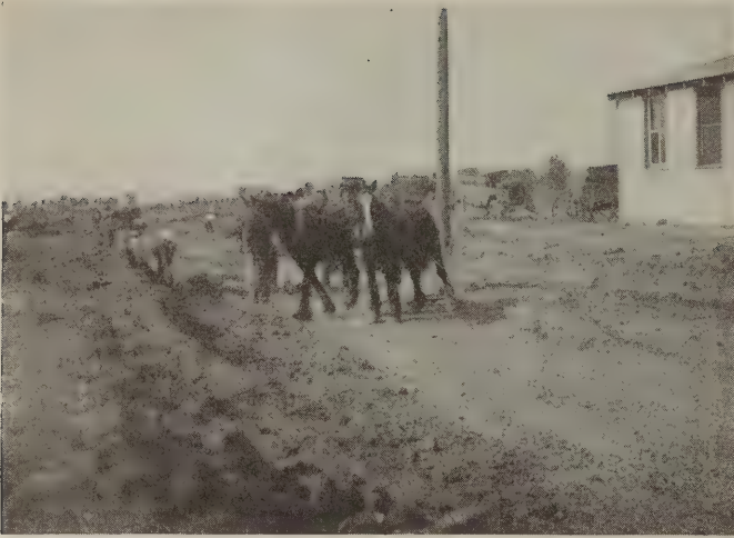
The development of the Jones property in the Fair Oaks section meant the paving of streets and alleys as well as the building of houses. Sewers and gas and water pipes had to be laid, too
