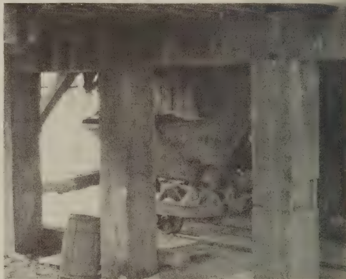
Type of car used to charge concrete mixer
