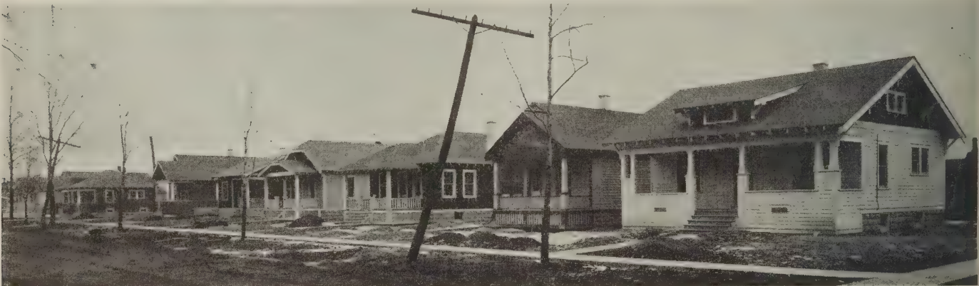
Row of one-story cottages built in 1921 by Lockport Homes Co.
