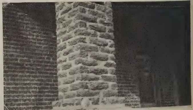
Detail of old brick post chopped with hatchet to make stucco bond
