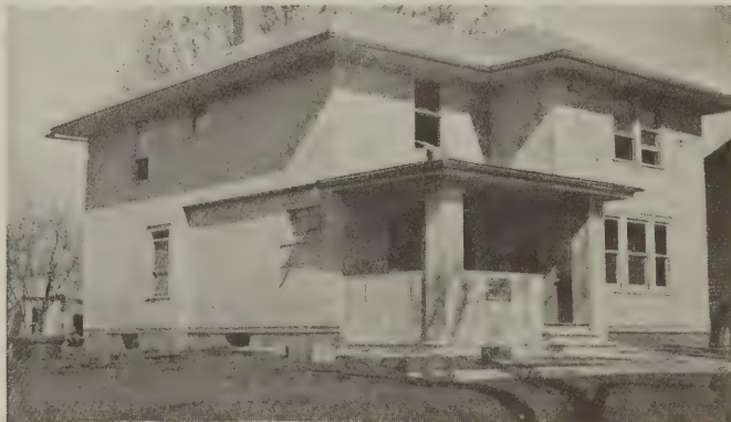
After remodeling, May 1, 1921
