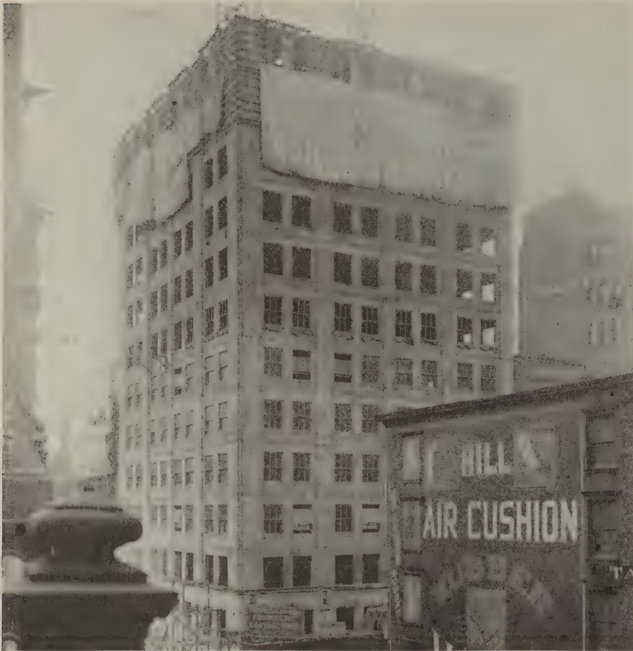
The building had reached the fourteenth story. Note the method of protecting the concrete from freezing. Also that the lower floors have already been glazed, making it possible to advance the interior finish along with the structural construction
