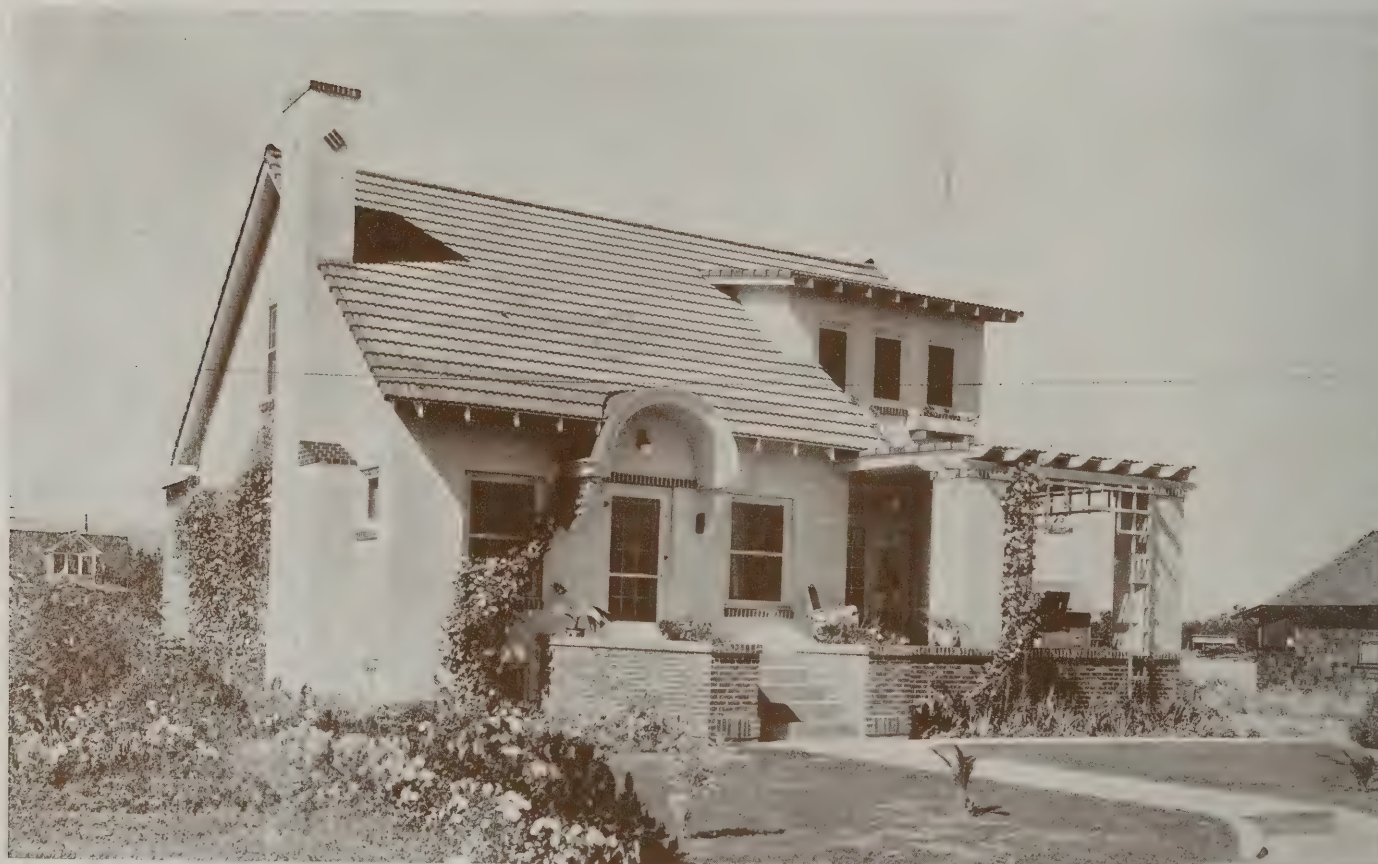
House built by Medford Construction Co., Medford, Ore., from plan 1175-E of the Hollow Tile Association
