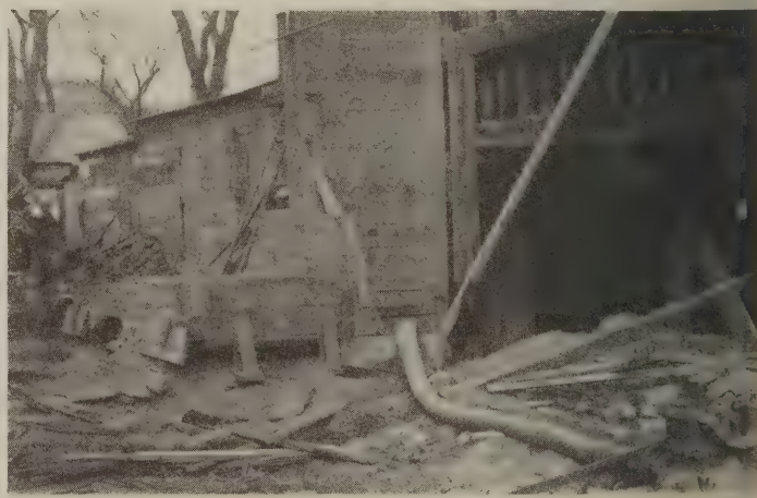
Another view of receiving hopper for aggregates showing pump for drainage of elevator boot. Cement stock house at the left
