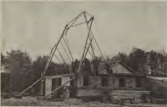
Raising the first bent
