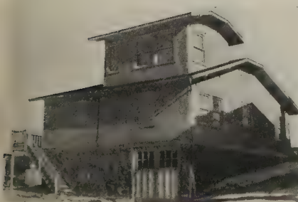
Back view of 5706 Locust street
