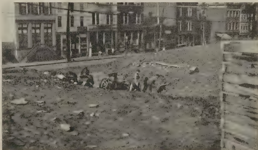
Starting excavation for combined store and bungalow at Bowman Terrace
