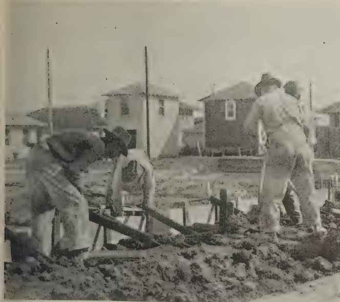
Concrete foundations introduced in Houston. No cellars
