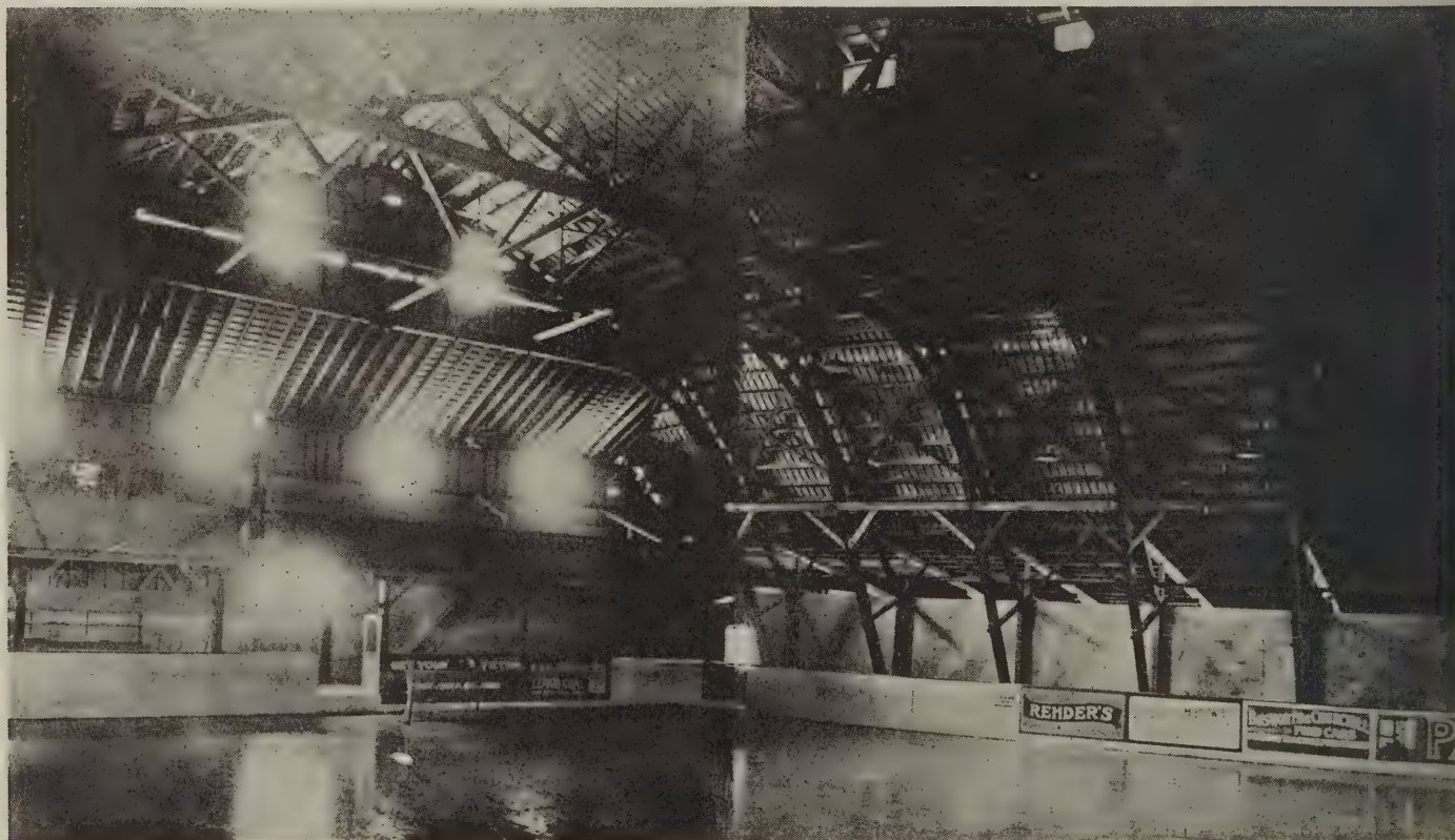
Corner of arena at Paris, Ont., showing truss arrangement
