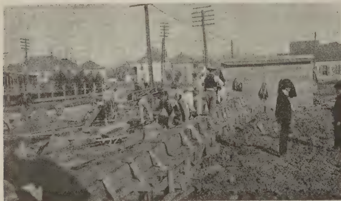
Placing the concrete foundations for Green & Green Bottling Works
