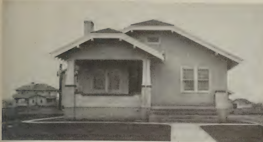
Front view of hollow-tile bungalow
