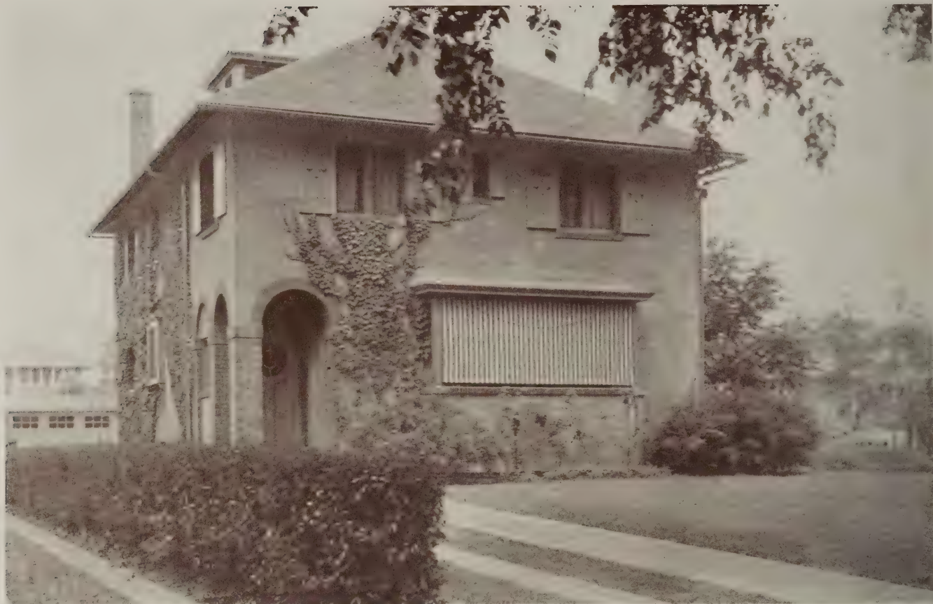
No. 15—A well proportioned square house with attractive details. A "close-up" of the entrance appears on page 41. The use of brick in the porch and for the window sills is good. The stucco is gray and the blinds are painted a pea green
