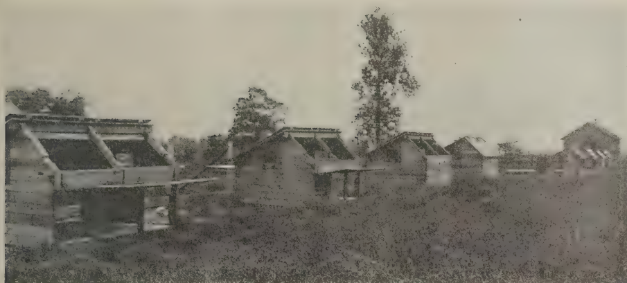
Fig. 1—Combination roof hog houses with the windows and doors open for summer time. The side walls serve as sun shades for summer
