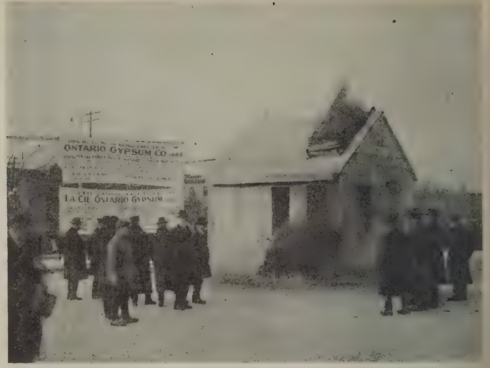
Another view of the house in process of construction and a fire-test in public to show the incombustible character of the materials
