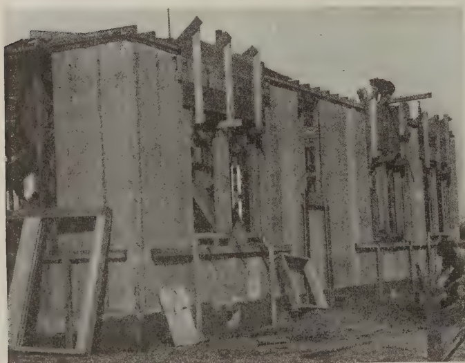
Forms in place for concrete. Lintels over window frames
