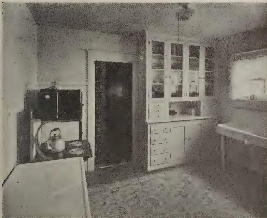
Trim is all finished in white enamel. Doors, 1¾-in. one-panel, are birch, finished in dark mahogany. Sink has double drainboard, all white porcelain. Cooler door can be seen on main shelf of cupboard, right-hand side. Clothes chute door over table on left-hand side
