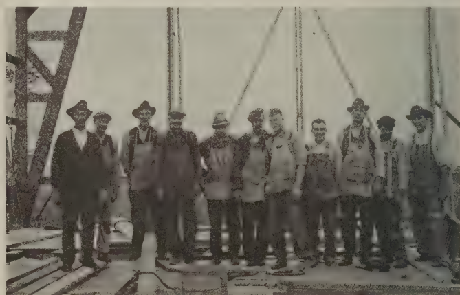
John Schifferle and his barn construction crew
