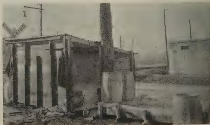
Covered curing bin for lime putty
