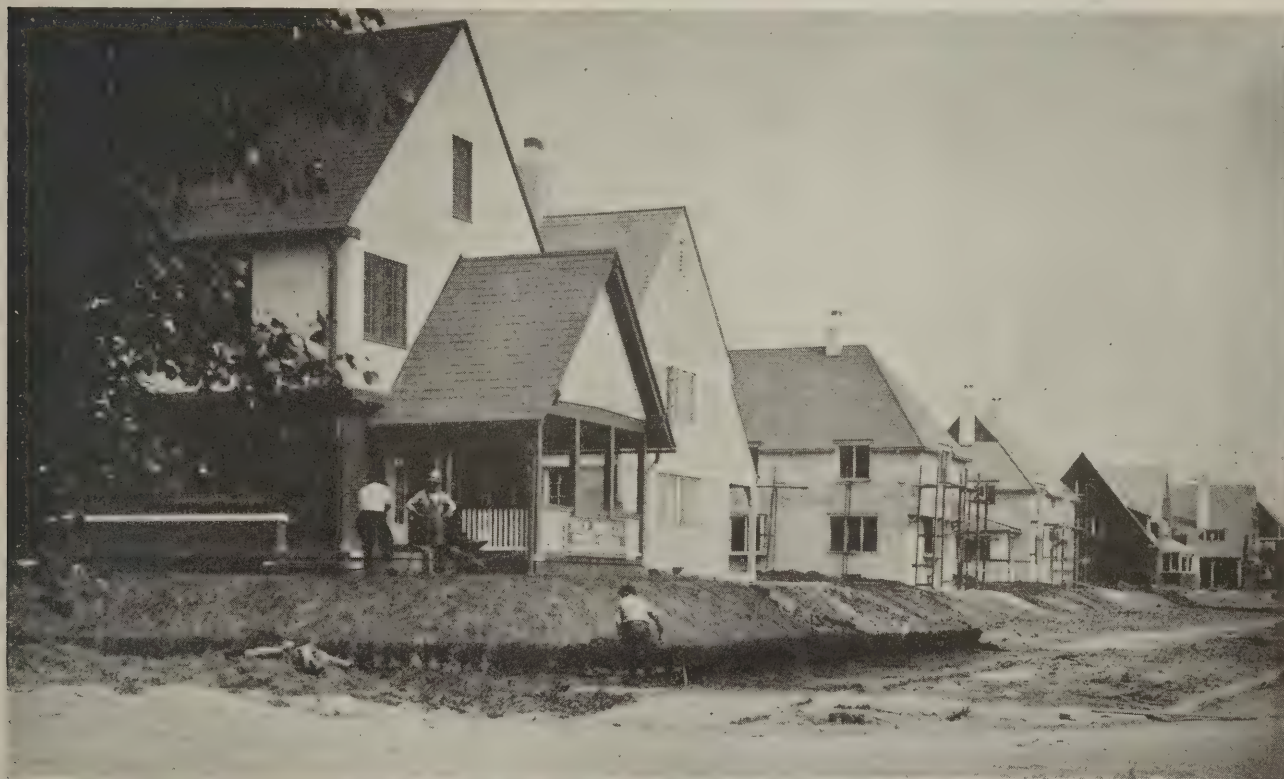
The twelve houses now under construction. Seven are visible in the picture, but foundations for five more are in between the houses shown beyond the first two. Seven will be "Stonekote" stucco, four stucco and brick veneer, and one—the center house—all brick veneer. All are of English design, some with half timbers. The houses do not line up in a straight line in front, but sweep back in a graceful curve from each end; thus each commands a view up and down the street and, with the terracing and shrubs in, will present a pleasing appearance as a group. Other houses to be built on other streets will be of the Colonial type
