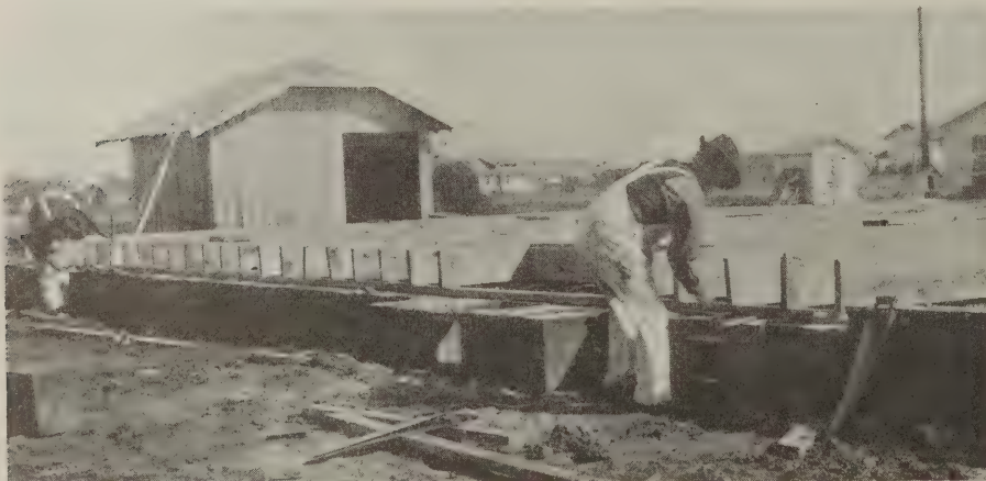
Extra wide foundation walls to receive concrete uprights
