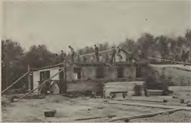
Trusses laid out on barn floor preliminary to raising
