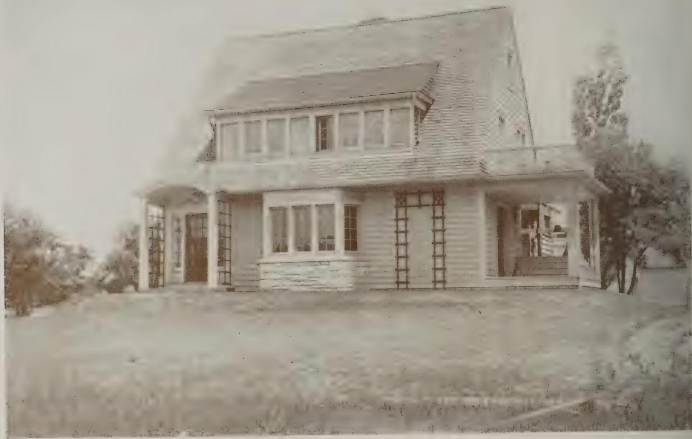
No. 15—This house and the one below are similar in plan. The proportions of the dormers are good and the treatment of the roof in both cases excellent
