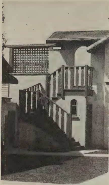
Detail of stairway to the roof of the garage, with tool storage underneath
