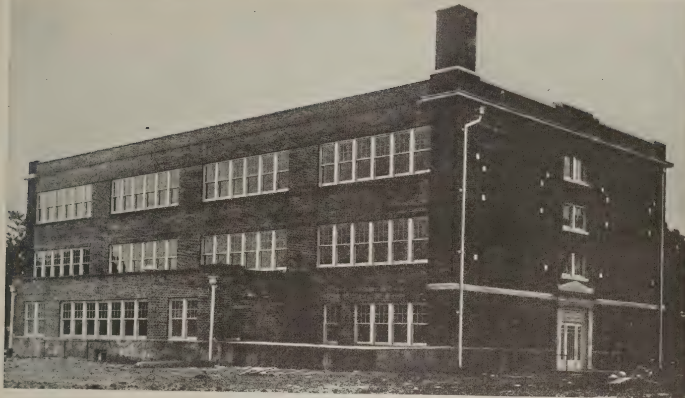
Rear elevation of Brookfield school building
