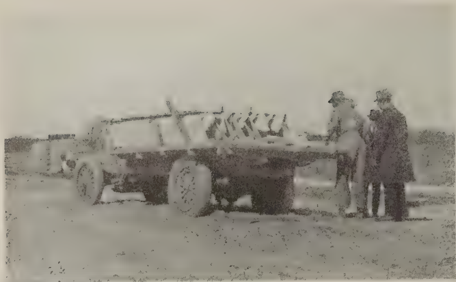
Concrete channel members handled like lumber
