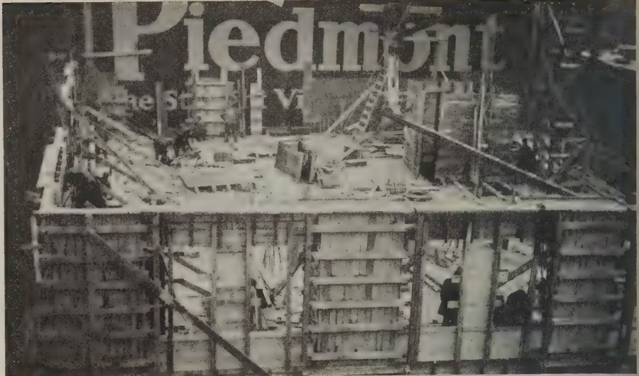
The entire curtain wall, lintels, mullions and columns from floor to floor were poured at one time
