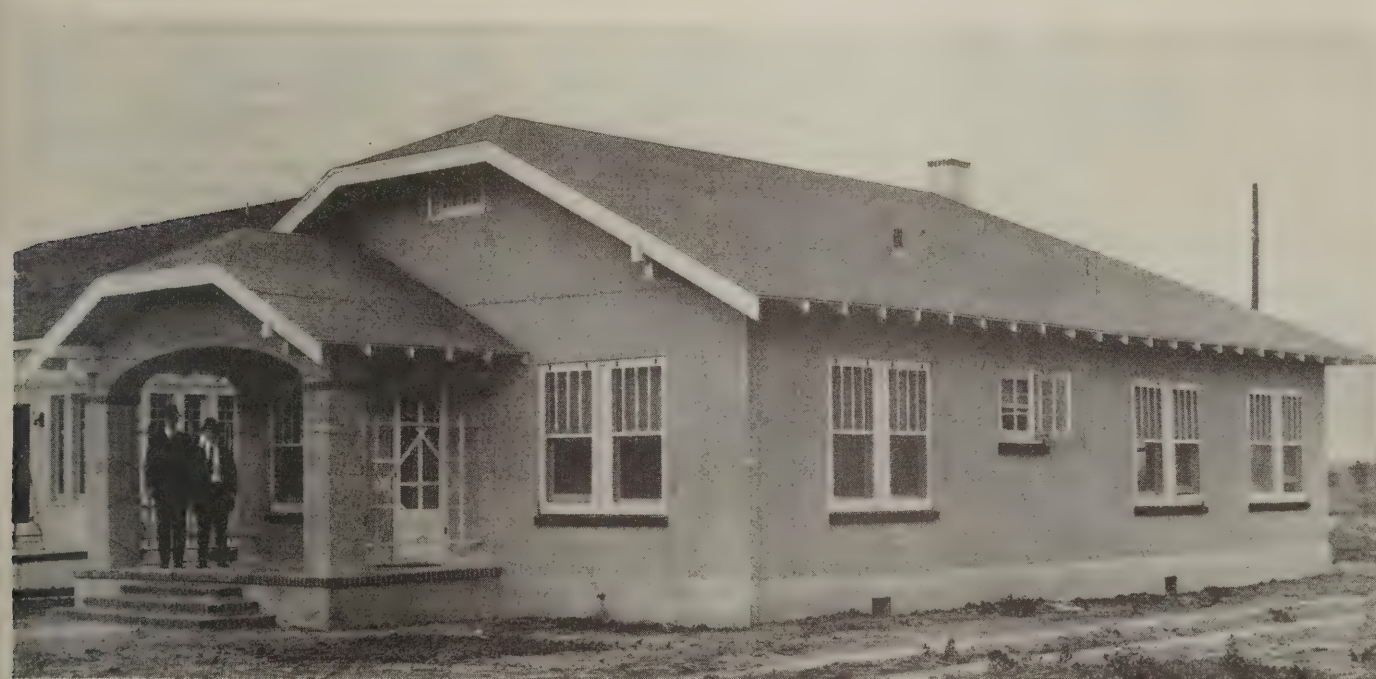
Bungalow complete and ready to move into
