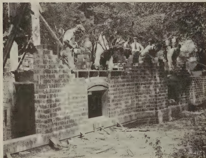
Ideal wall house under way
