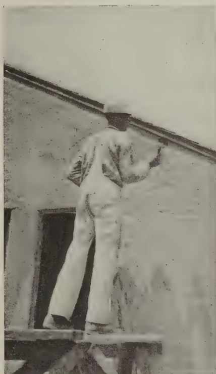
Fig. 13—Dampening down the scratch coat
