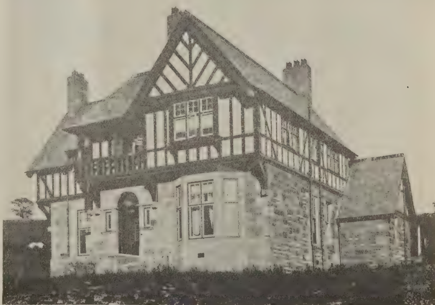
Timber framed and stucco wall of an upper story
