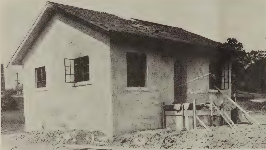
Gypsum stucco house with wood supporting members practically intact after the fire test
