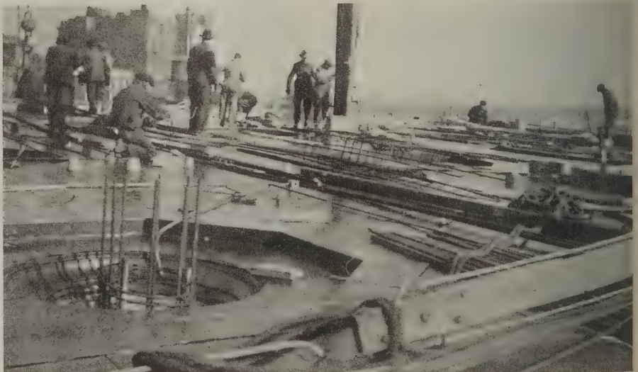
Showing steel form for column
