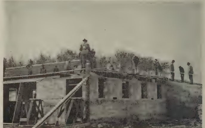
Braced corner post for holding end truss
