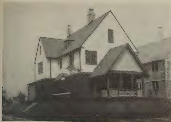
The corner house, entirely completed, with terracing done and shrubs and trees set out. The design is distinctly English, with its steep roof projecting only about eight inches at the eaves and finished only by a rake mould on the gables
