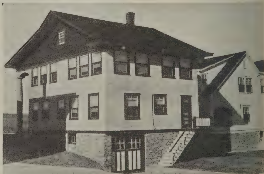
Back and side view of 5711 Oak street
