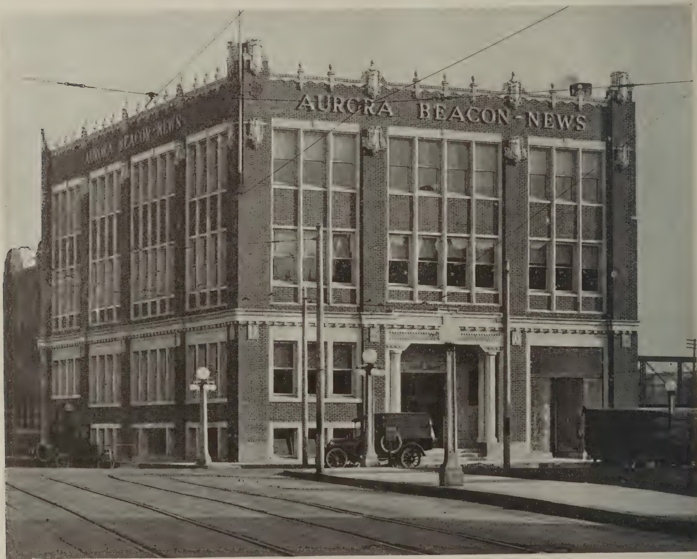
"Beacon-News" newspaper plant in Aurora, Ill., designed by Zimmerman, Saxe and Zimmerman, architects, Chicago
