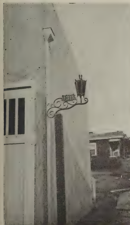
Fig. 11—Wrought-iron lantern and bracket in place, with numbering of upper apartment. Entrance stair at side rear
