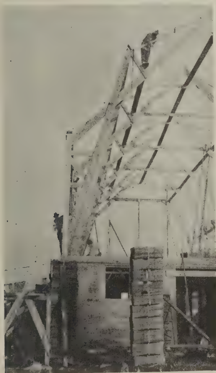
Bundles of shingles made into columns to support end bent before raising
