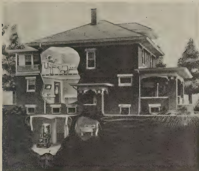
The illustration at the left shows a shallow well or cistern system, pumping to a lift of 25 feet. The illustration to the right shows a deep well system pumping to a lift of 100 feet below pump. Fort Wayne Engineering and Manufacturing Co., Fort Wayne, Ind.
