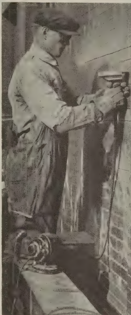
Cutting out mortar between masonry joints by machine
