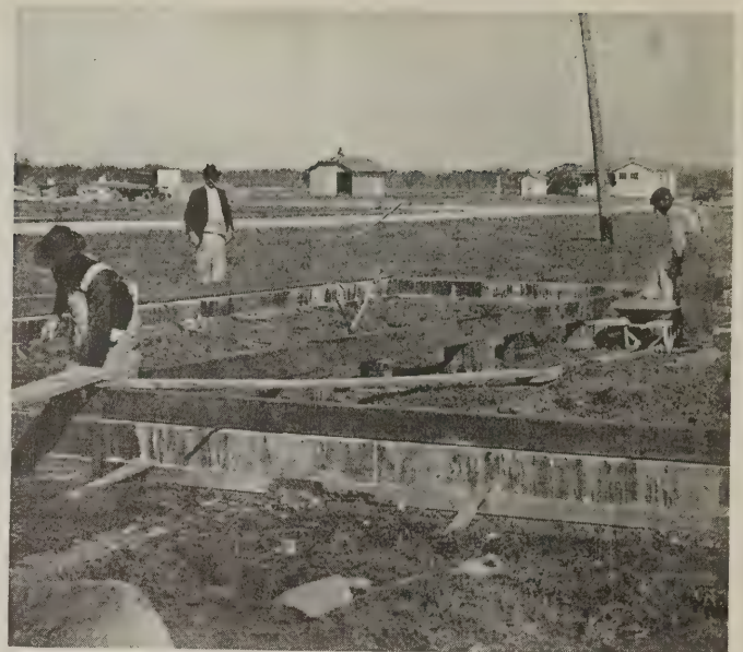
4 x 6 sills; 6x8 girders
