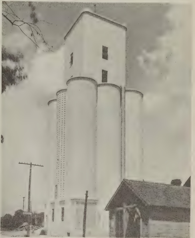
Fig. 2—Concrete elevator and ear corn storage at Pesotum, Ill., designed by Holbrook, Warren and Andrew, engineers, Decatur, Ill. The capacity of the elevator is 45,000 bushels of small grain and 3,000 bushels of corn on the ear
