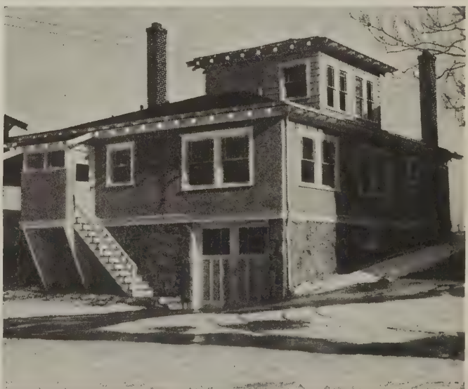
Back view of 5718 Locust street
