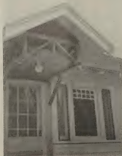
Showing method of bridging used in porch hood
