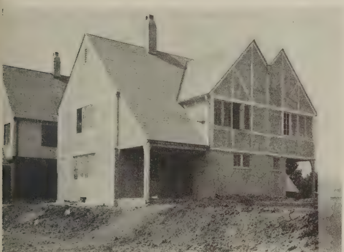
The second house from the corner, built of "Stonekote" stucco in a buff tint over metal lath. The half-timbers will be painted a dark brown to contrast
