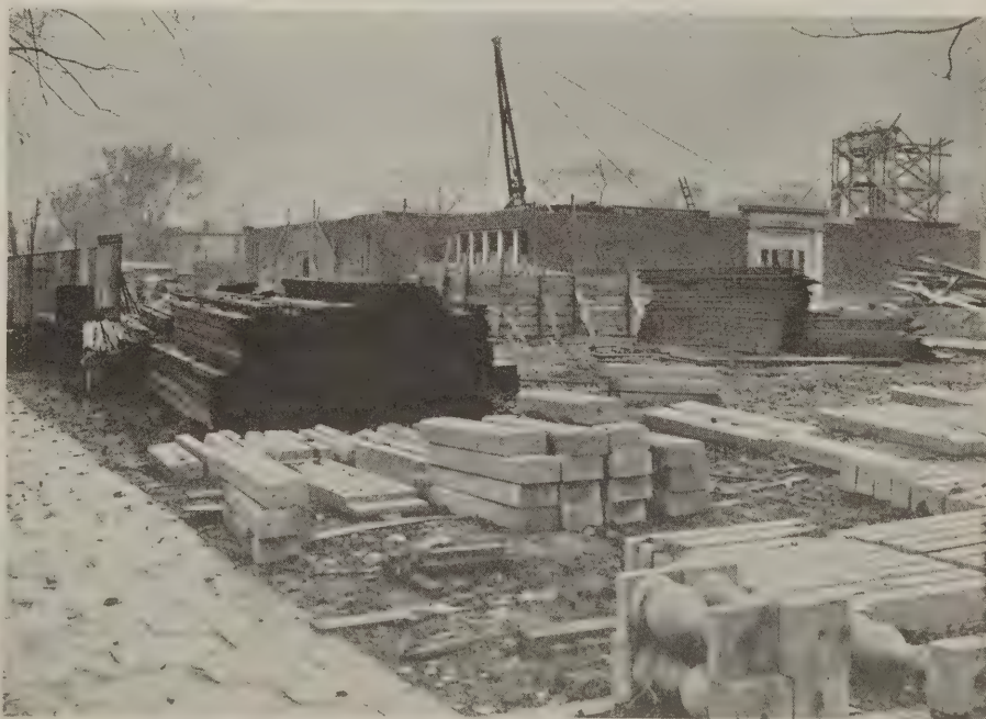
Winter construction. Note the orderliness of material layout
