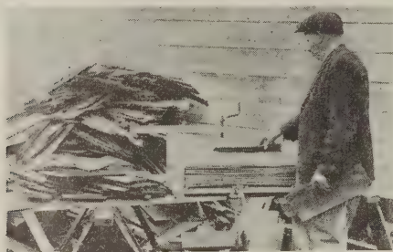
Assembling the shingles in baler
