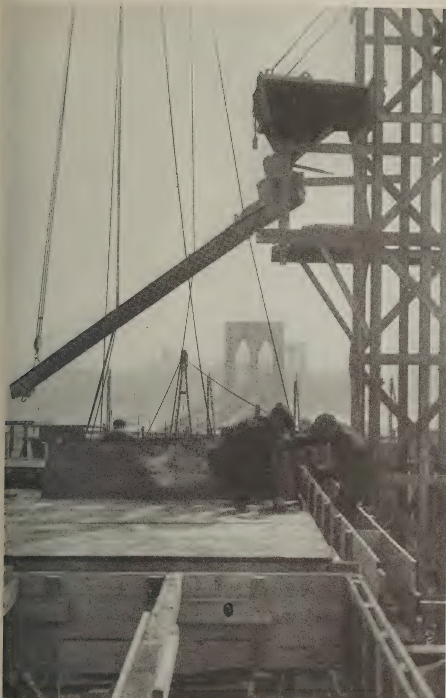
Laying down plates of steel floor forms. Copyright International
