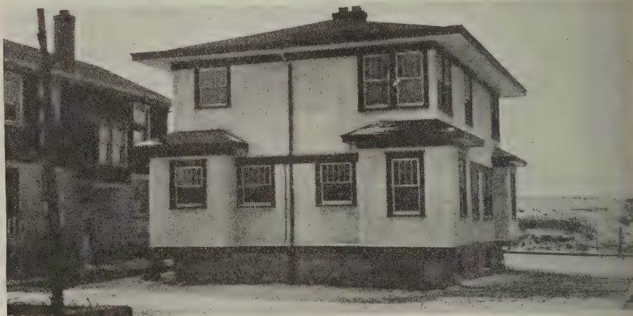
Side and back view of 5701 Oak street
