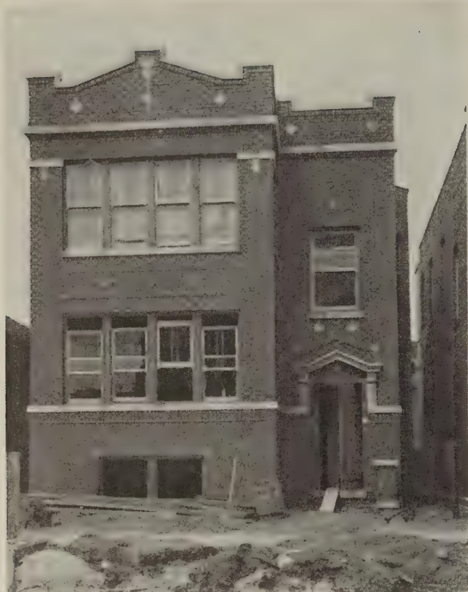
Typical two-flat building just completed
