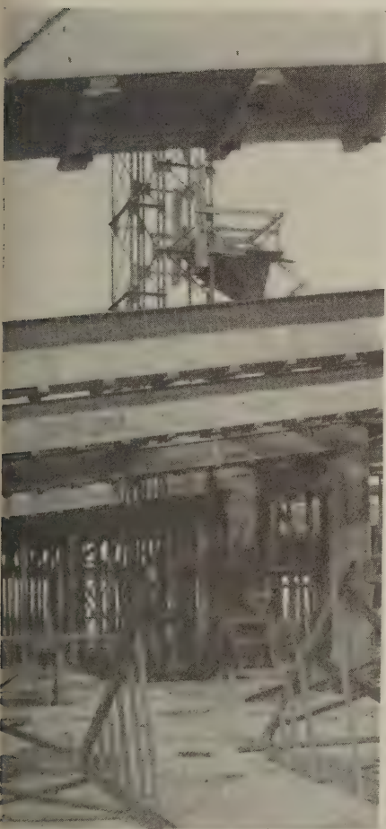
Top of concrete elevator shaft and lower hoppers for receiving the skipload of mix
