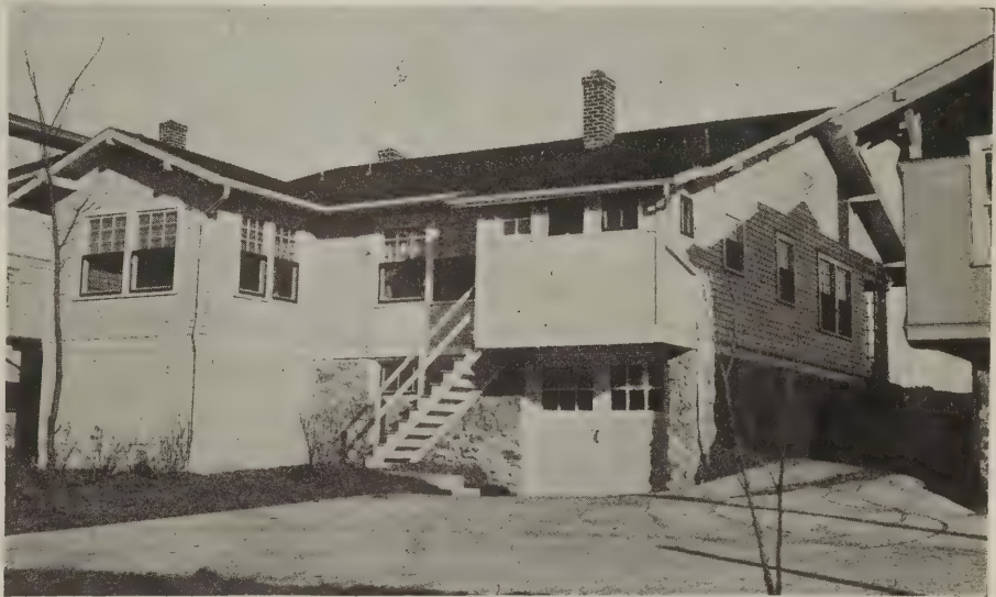
Back view of 5714 Locust street
