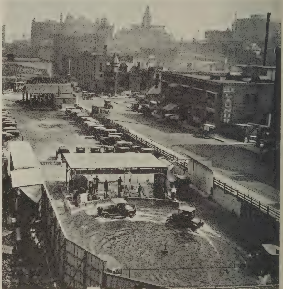
Automobile wash bowl, St. Paul, Minn. A new type of structure for concrete contractors to build
