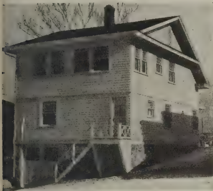
Back view of 5728 Locust street
