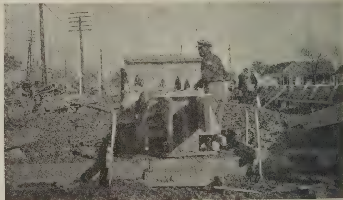
Use of 2-in. floor joists for concrete forms
