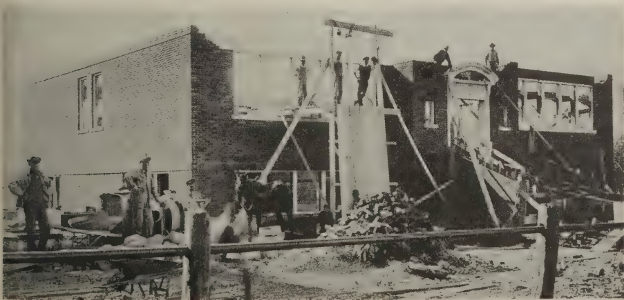
Progress photograph, November 2, 1921—Front
