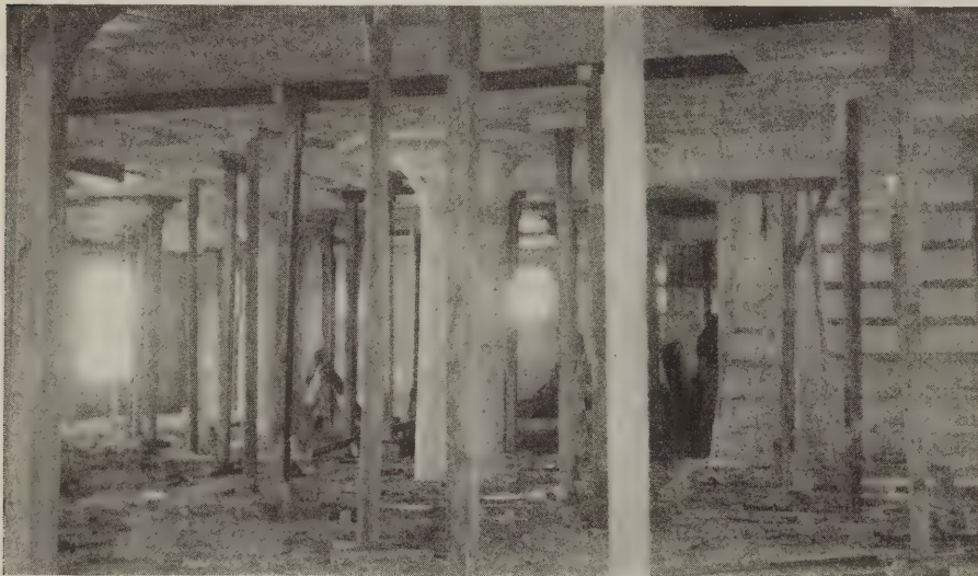
Shows method of shoring, which made it possible to strip the greater part of the shores under floor slab and still leave sufficient form work undisturbed to carry slab with absolute safety, when the steel forms and shoring were needed for upper floors and the concrete had not set sufficiently to be left unsupported
