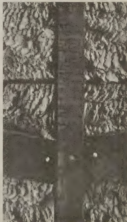
Back of metal lath between studs before back plastering
