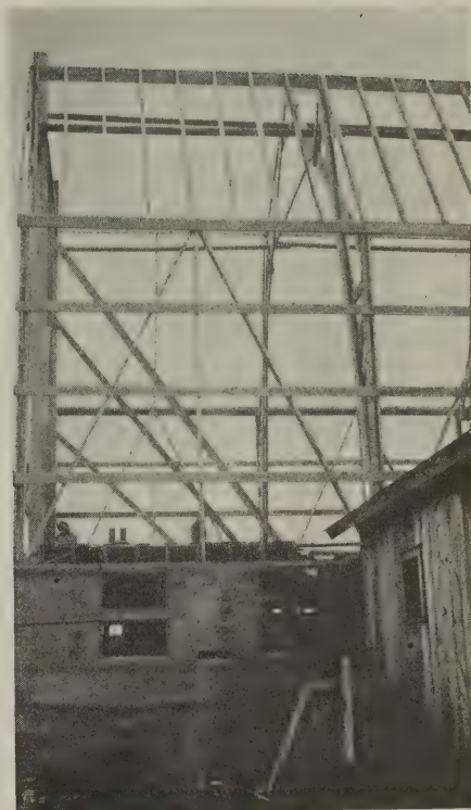
Framing and rafters complete
