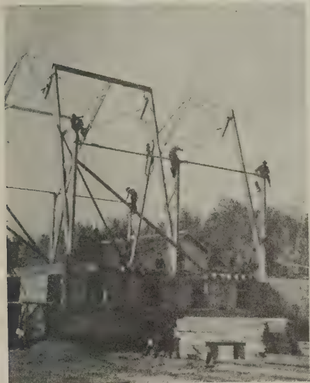
Placing longitudinal struts and ties
