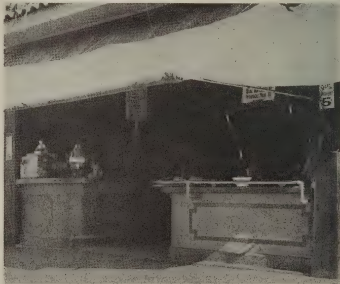
This is one-coat work troweled on rough framework
