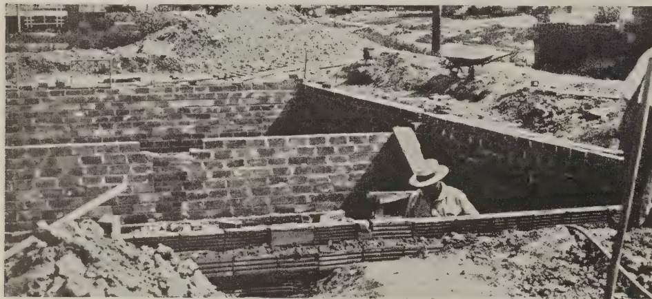
Cleveland house foundation made of hollow clay tile
