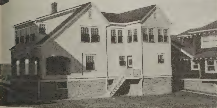
Side and back view of 5709 Oak street
