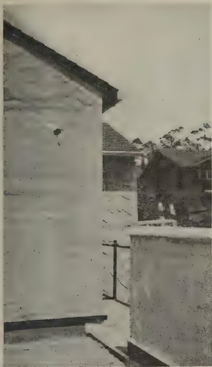
Fig. 10—Unenclosed rear upstairs hall from deck of garage
