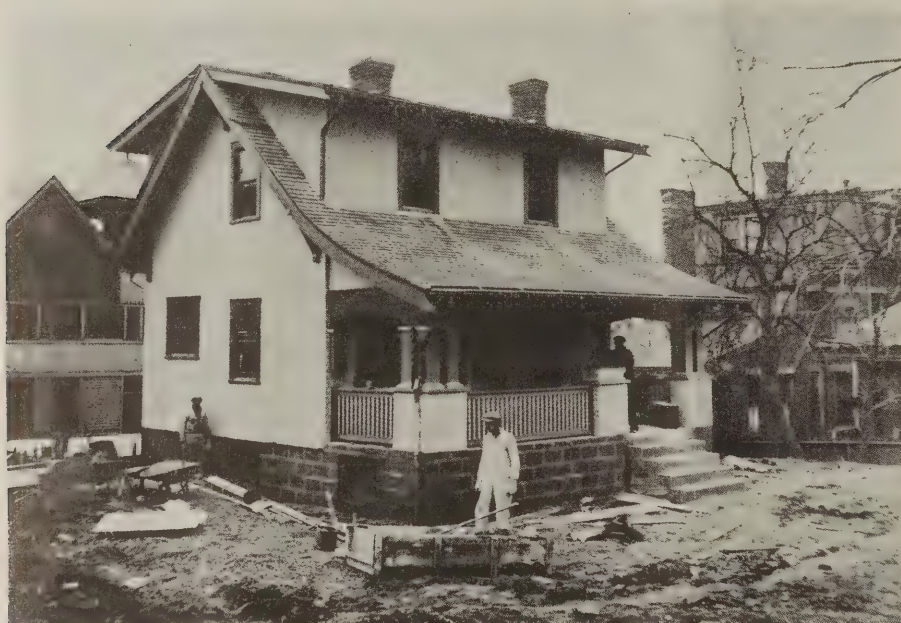
The $4500 Joseph Phillips' house near completion
