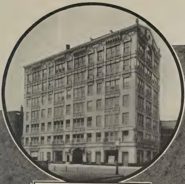
Studio Building, Cass and Superior Sts., Chicago CELOTEX used for Roof insulation
