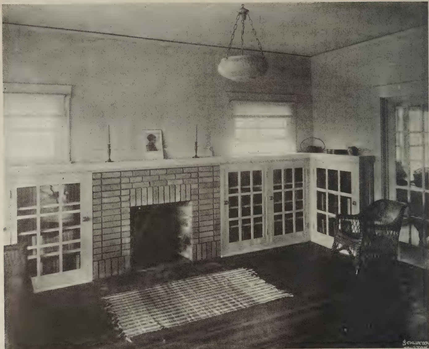
Interior of living room of concrete bungalow
