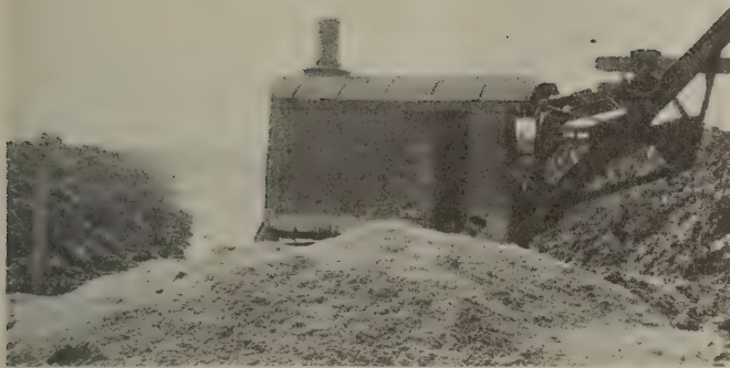
Fig. 7—Excavator scooping out for basements
