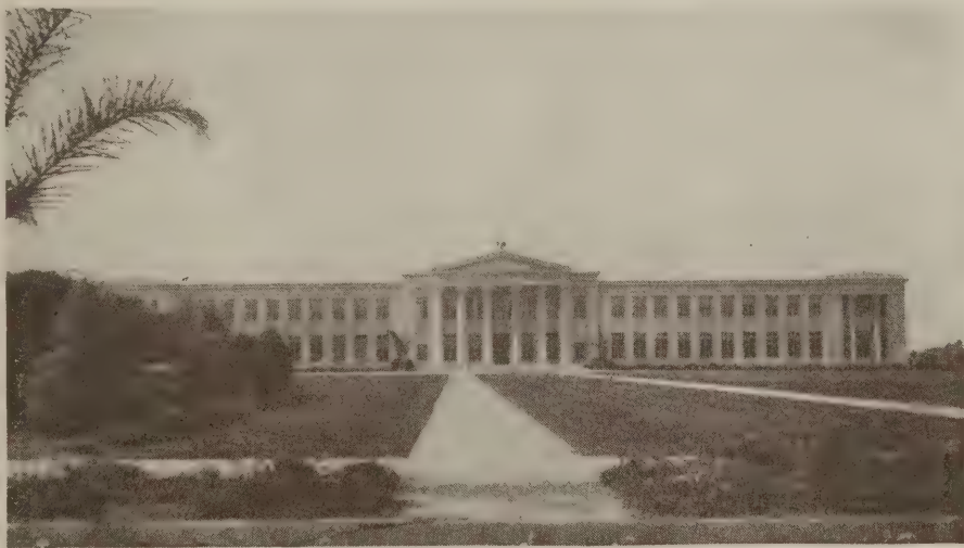
The buildings and grounds are interesting at every viewpoint
