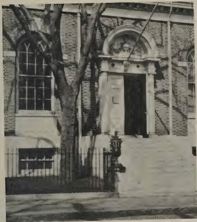
Plate 1—Entrance to the library at Swampscott, Mass. Kelly & Graves, architects. A well designed piece of stonework, beautifully detailed
