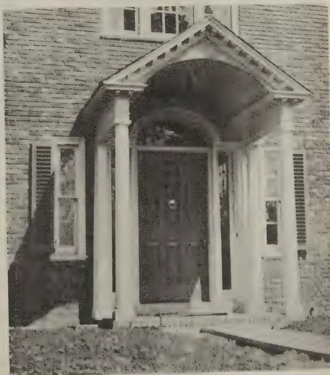
Plate 4—A well designed colonial entrance that will be improved by the planting. The soffit is of stucco and the floor is of brick
