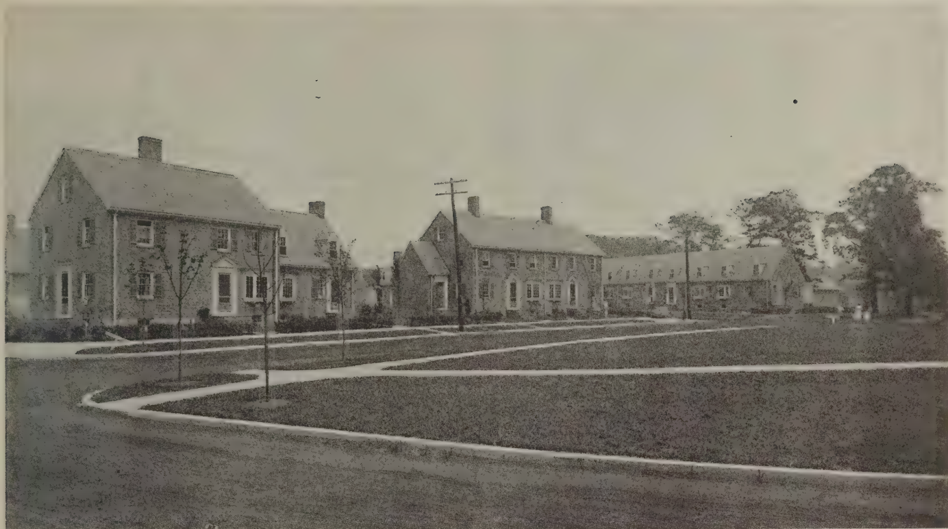
Plate 16—At the left a K-8-10 and 11 group. Center, two H-6 houses. Distance, a row of K-11 houses. Crane Tract
