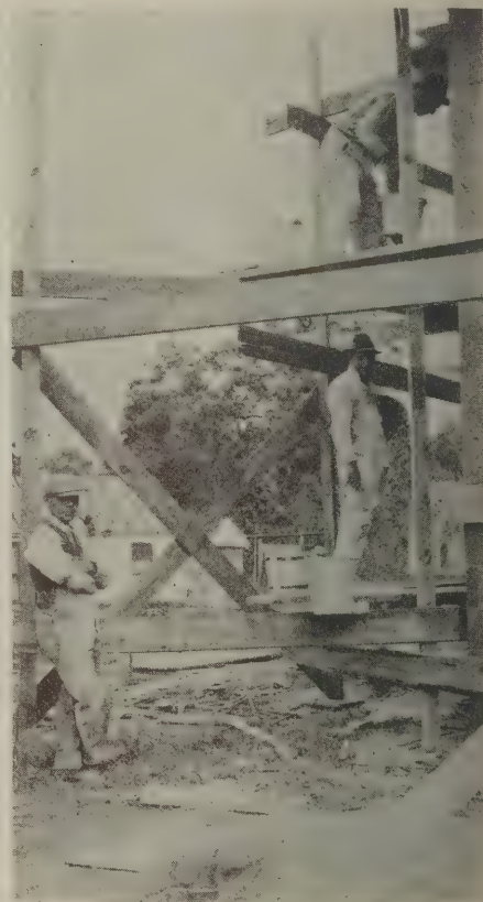
Plate 3—A three-deck plasterer's scaffold showing the diagonal support at the corner.
