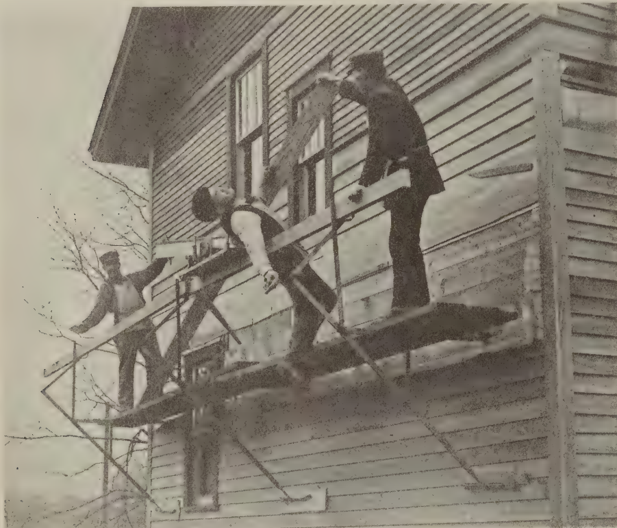
Plate 1—An ingenious scaffold support made of steel and providing a support for a 2 by 4 guard rail.
