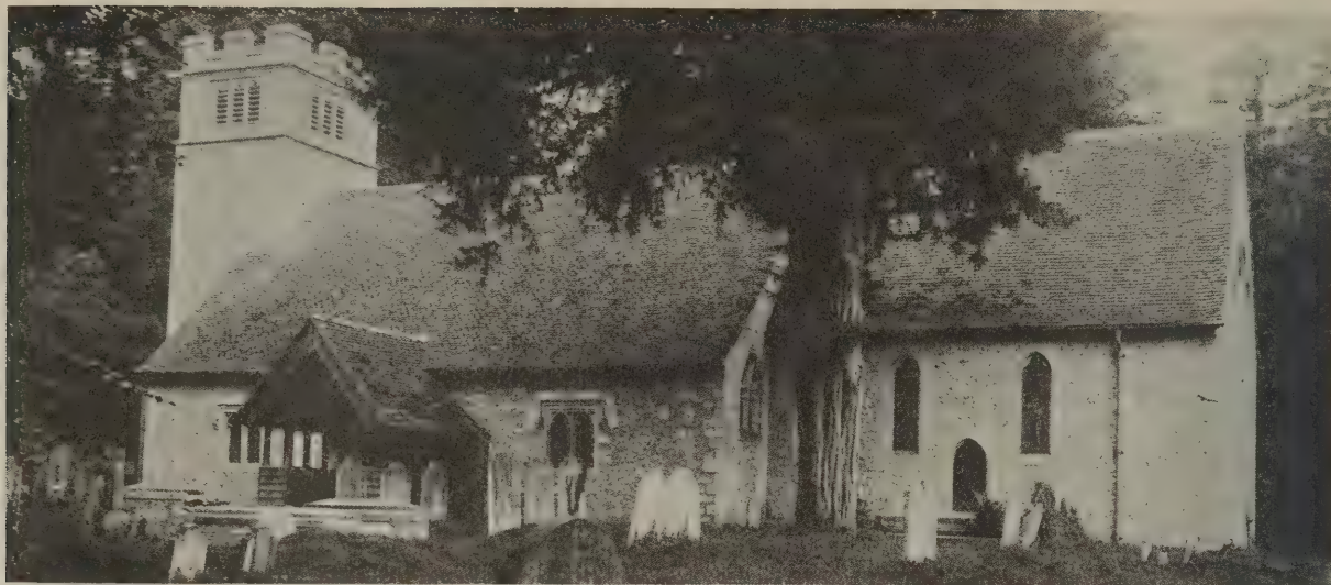
A village church built of random rubble with stone dressings at the openings
