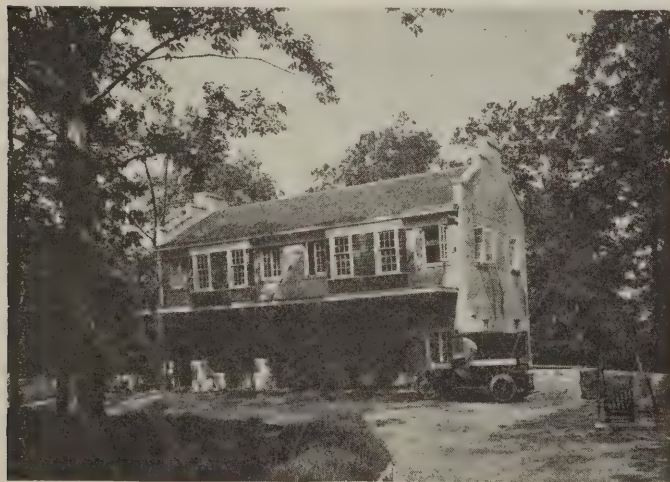
Plate 1—A garage for a fleet of delivery autos. Chauffeurs' quarters in second story
