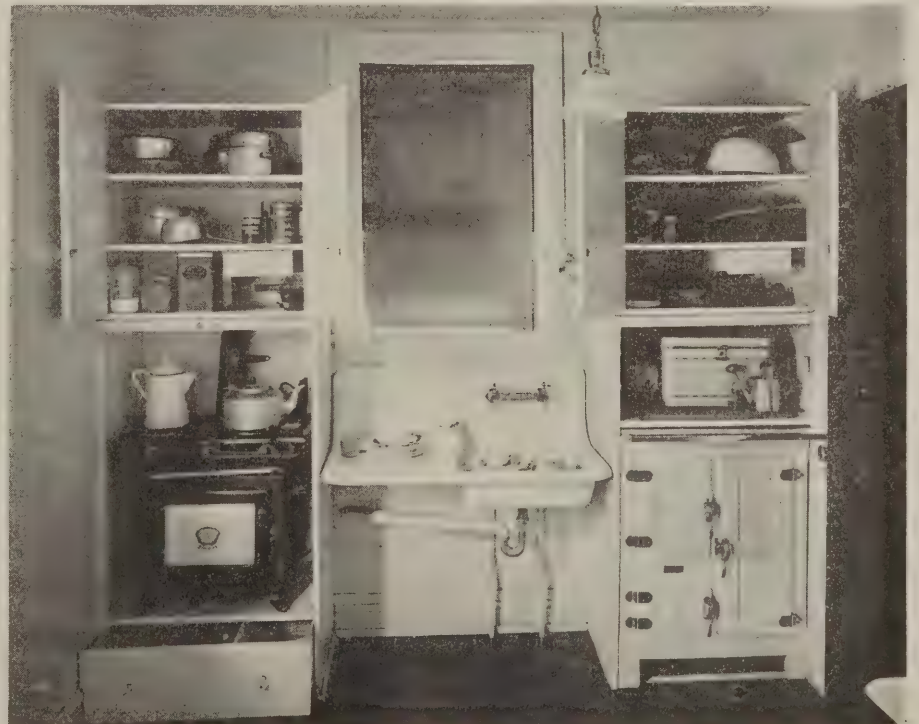
Plate 2—One of the steel buffet kitchens that proved to be space savers. Note the numerous shelves, the drawers, sliding work board, and the grouping of stove, sink and refrigerator
