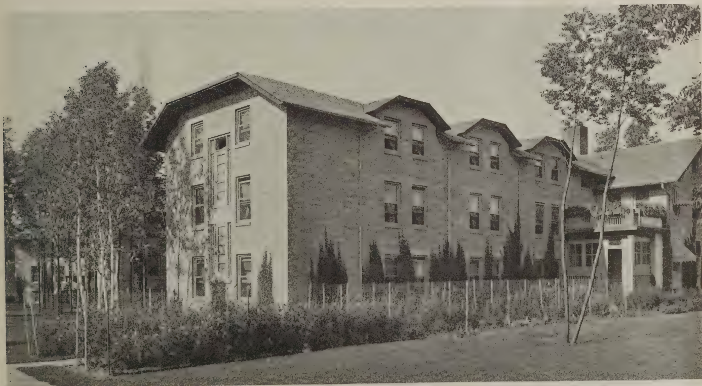
Figure 8. The boarding house at Morgan Park is known as the Nenovan Club. It is an attractive building of concrete block having 12 bedrooms on each floor, large reading, recreation and dining rooms, equipped in the most modern fashion throughout
