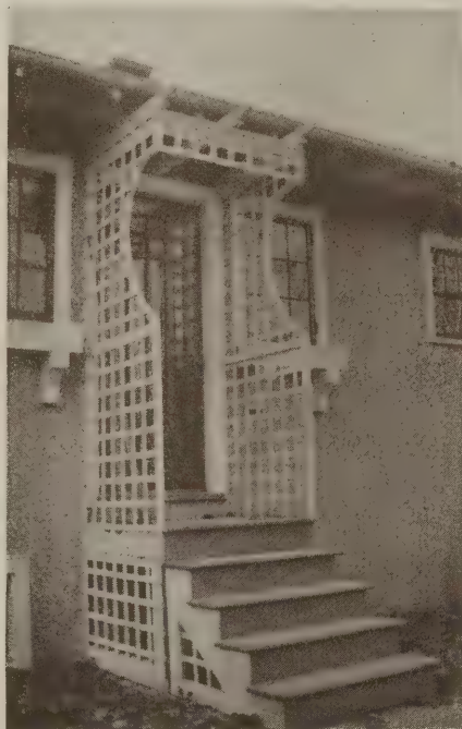
Plate 3—This house is on a corner lot and the rear entrance is directly off the side street. In such cases a decorative treatment is almost compulsory
