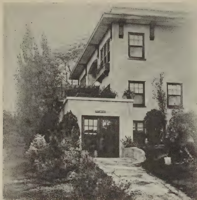
This garage, entered from a rear alley, is directly joined to the house, its roof comprising a side pergola and terrace. The doors are of glass. It is located in Kansas City, Mo.
