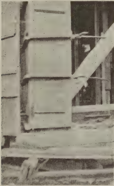
Plate 1—Metal clamps in place around column form
