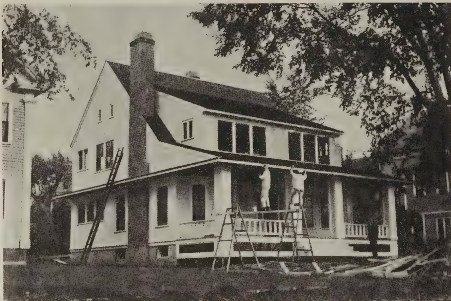
Fig. 1—Construction photograph made before the planting and sodding were complete
