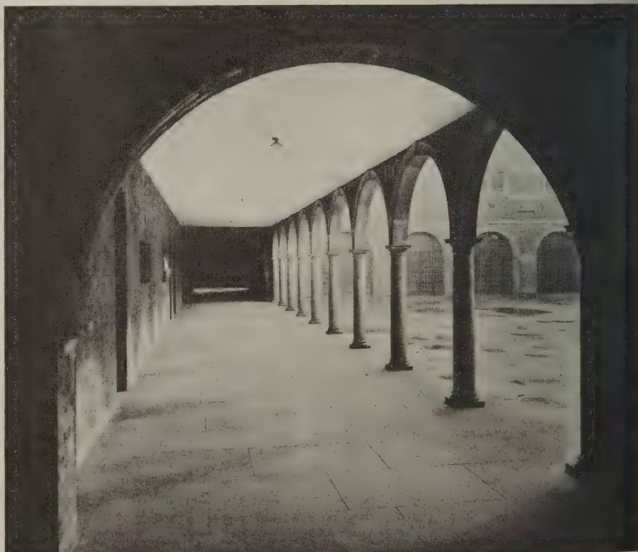
Covered passage at the side of quad, Stockport Grammar School. Showing monolithic stone columns with semicircular stone arch fitted on the spandrels with brickwork
