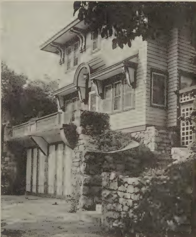
Facing a picturesque canyon in Kansas City, Mo., and approached by a winding road or hillside street, this house has a pair of garages built directly under the front entrance as a feature of the basement. A sort of balcony over the garages forms the front porch of the house
