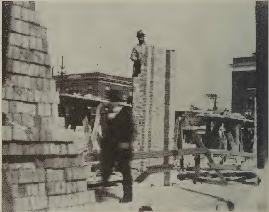
This barrier keeps pedestrians out of the danger zone
