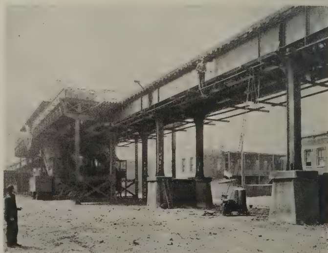
Painting structural iron, tanks and stacks with the air-confined jet is speedy, economical and cleanly
