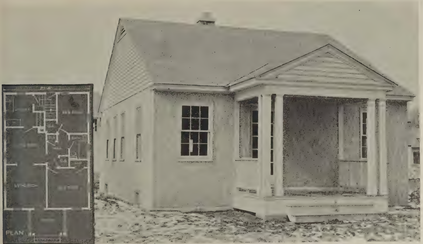
Fig. 2—Clapboards effectively used in the main gable and the porch pediment
