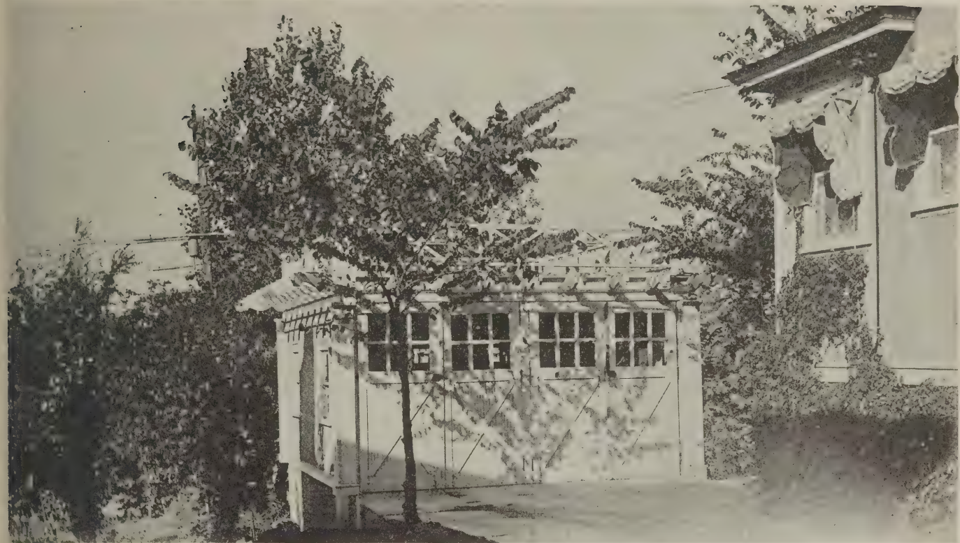
An attractive two-car garage of a Kansas City, Mo., home. The flat roof is used as a children's play porch, reached by a stairway on one side
