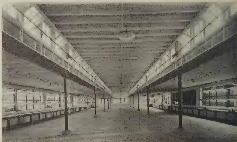
An assembly plant built on the "daylight factory" principle
