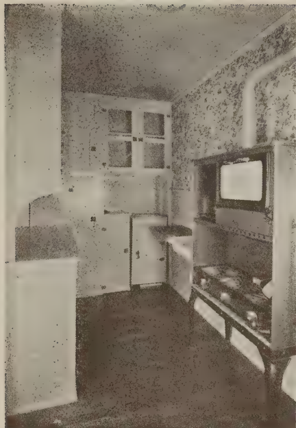
Plate 4—One end of the kitchenette. Reference to the plan will show that some changes were made during construction.
