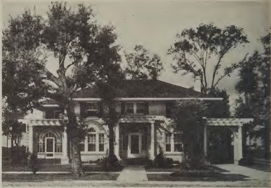
Plate 5—This house suggests the Italian order and is built of stucco on hollow tile
