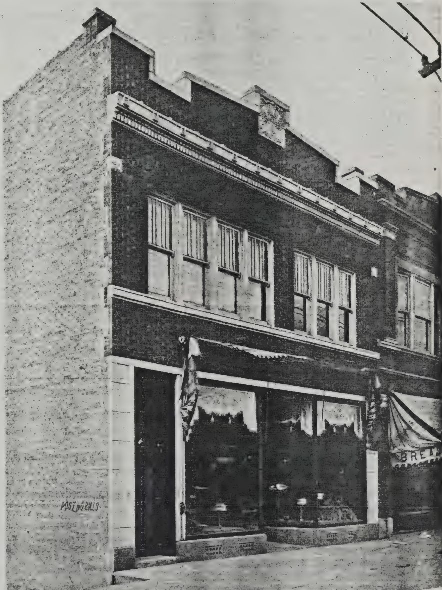
A well proportioned combination of brickwork, terra cotta and plate glass will bring an out of date front right up to the minute
