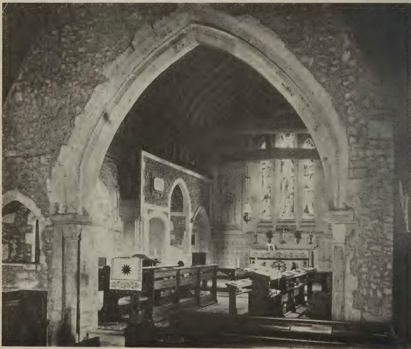
Rubble wall with stone dressings and Gothic arch
