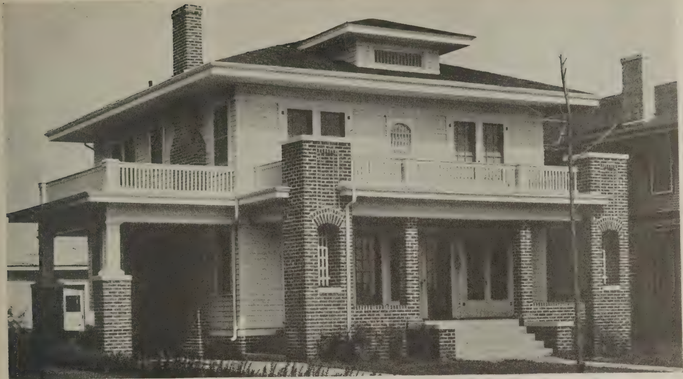
Wood siding and brick piers
