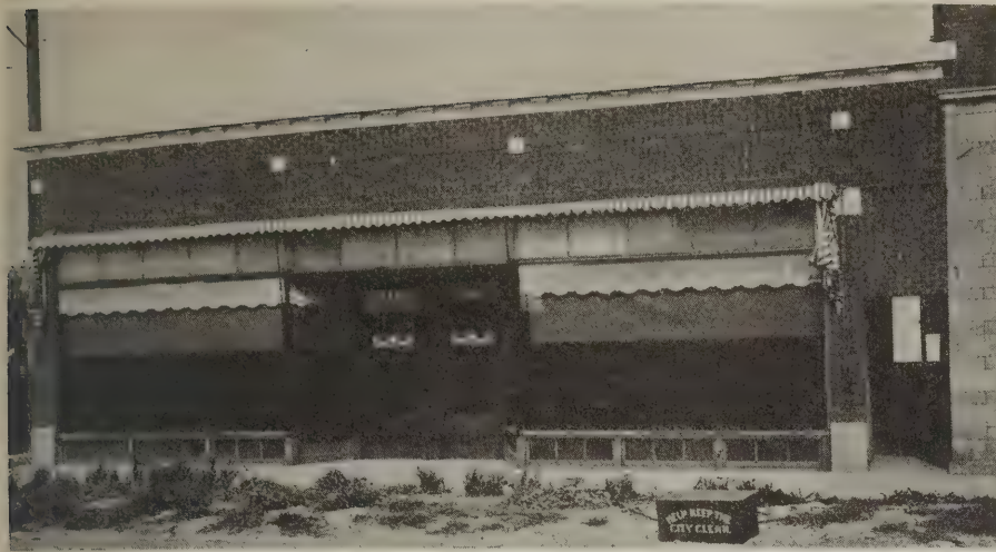
Plate 3—A one-story building of brick with terra cotta trimmings. A large variety of "stock" patterns are carried by the manufacturers, thus offering economy and quick delivery
