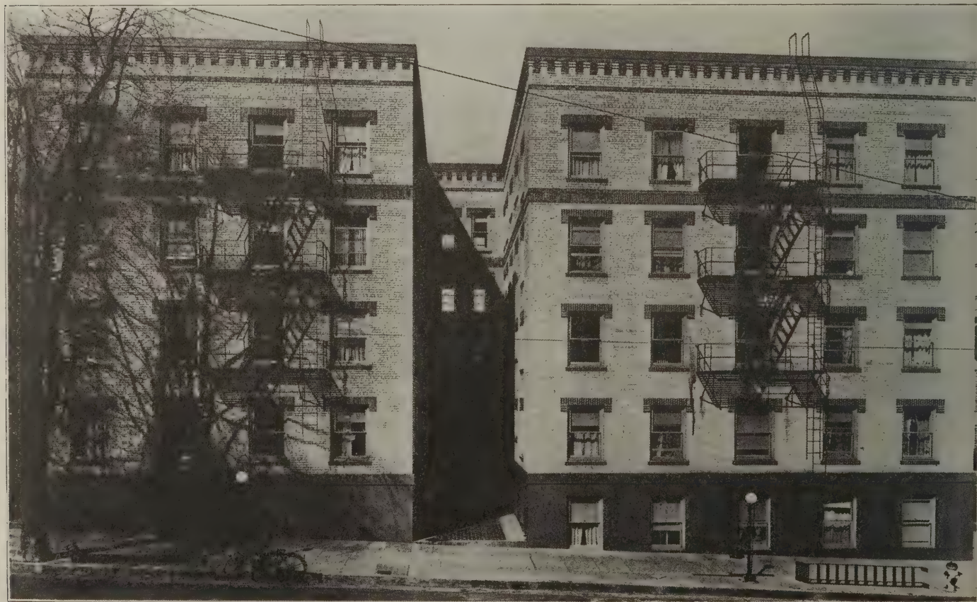
Apartment building at Portland, Ore., with ordinary cement face brick, buff colored
