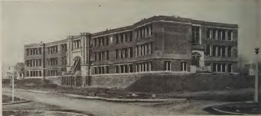
Plate 4—Many of the modern schools are built of hollow tile faced with brick and have combination hollow tile and concrete floors
