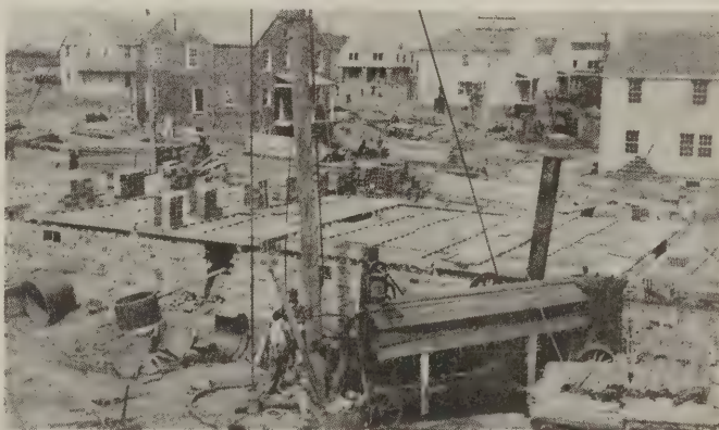
Plate 2—Lumber, hollow tile and lath piled in an orderly manner on a large housing development
