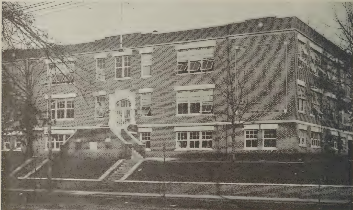
School at Sheffield, Alabama. B. B. Burnham, Architect; P. E. Bostic, Builder
