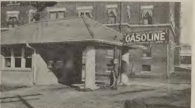
Plate 8—A filling station of stucco on hollow tile
