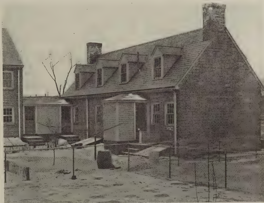
Plate 13—Rear view of two K-11 houses joined to a group of K-8-9 and 10 houses, Crane Tract
