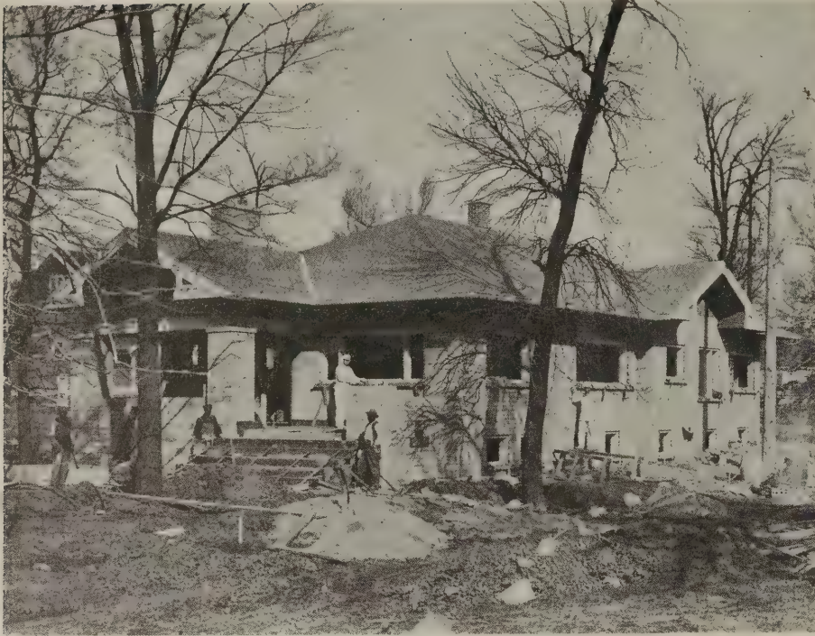
Concrete and tile walls ready to receive stucco coats
