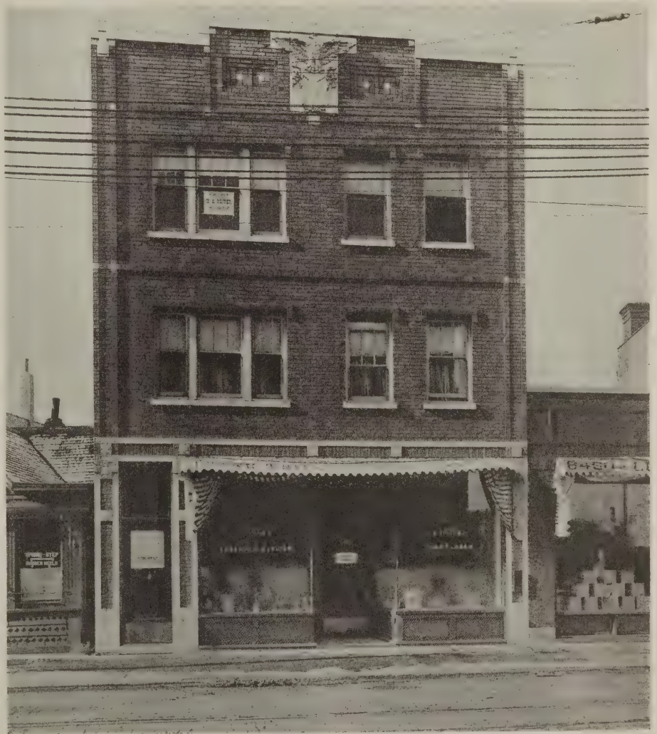
Plate 4—Another combination store and apartment building. The walls are of tapestry brick with terra cotta trimmings. The piers appear "skinny" and timber added to their width would be an improvement
