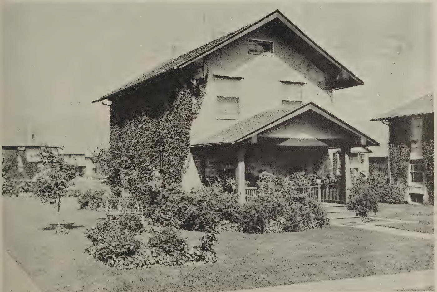
Figure 2. Concrete block residence, the home of a Morgan Park steel worker, which rents for $5 per room per month. The floors, as well as the walls, are of concrete, the former of monolithic construction. In later buildings enclosed porches of concrete block were used in place of open wooden porches like the one shown in the picture
