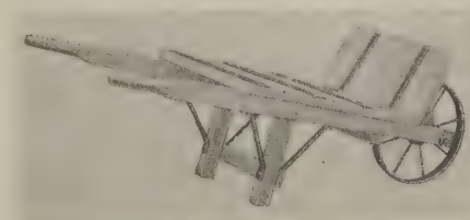
Fig. 3—Stone or mason's barrow
