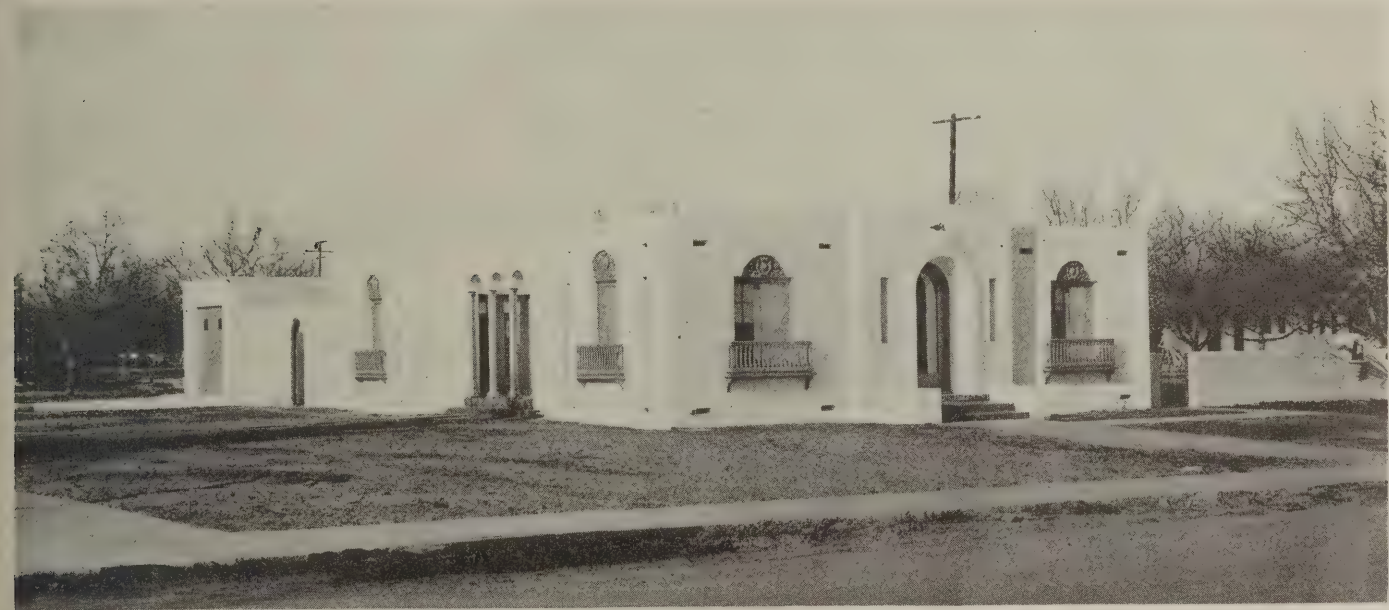
Fig. 4—The completed building of modernized adobe
