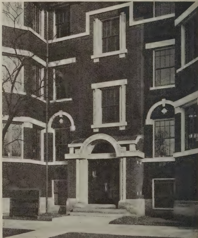
Plate 4—Another apartment house entrance. There are too many different kinds of detailing around the windows
