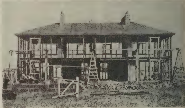
The illustration at the left shows workmen erecting the steel frame of a house; the right illustration shows the same house with roof and window frames
