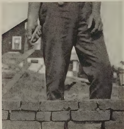
Fig. 1—Correct way of holding trowel. Note handle between thumb and forefinger. Fingers loose
