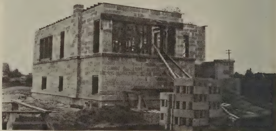
Fig. 2. General view of bungalow under construction. The block are quick to lay because of the stucco covering, requiring only plain flush joints
