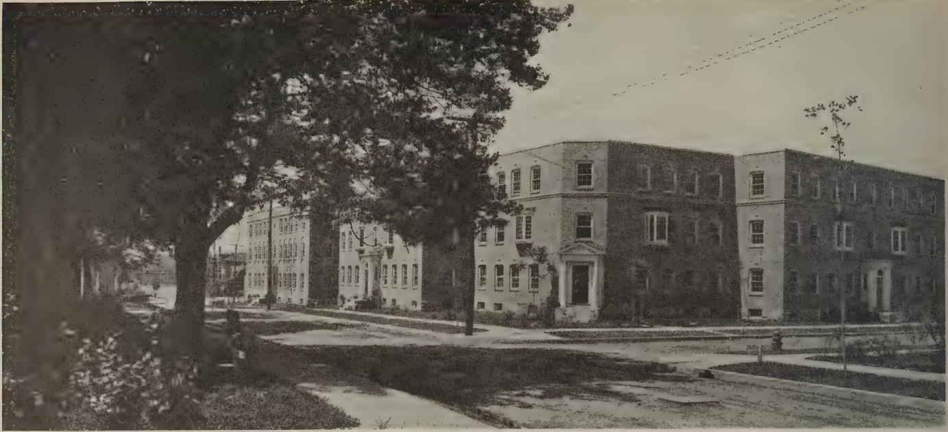
Fig. 1—(a) One corner of the "Black Rock" Apartment House development
