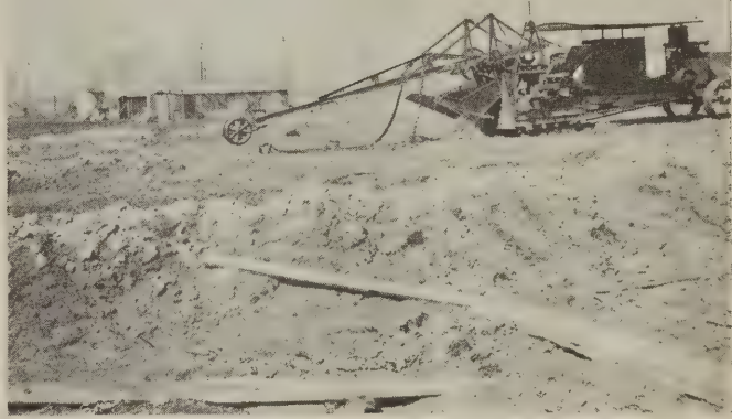
Fig. 10—Trench and ditch excavator
