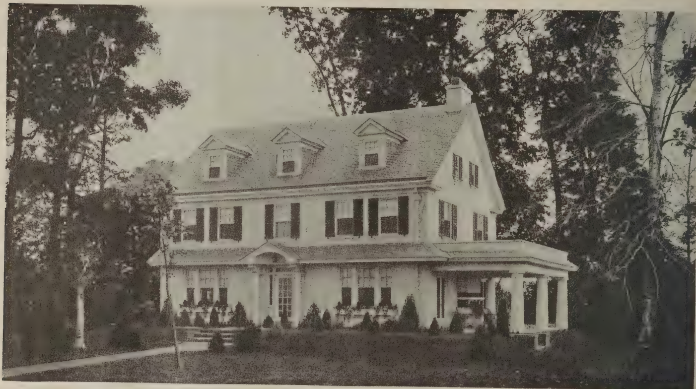
Fig. 3—Stucco house with wood trim and slate roof. Chas. T. Schermerhorn, Architect
