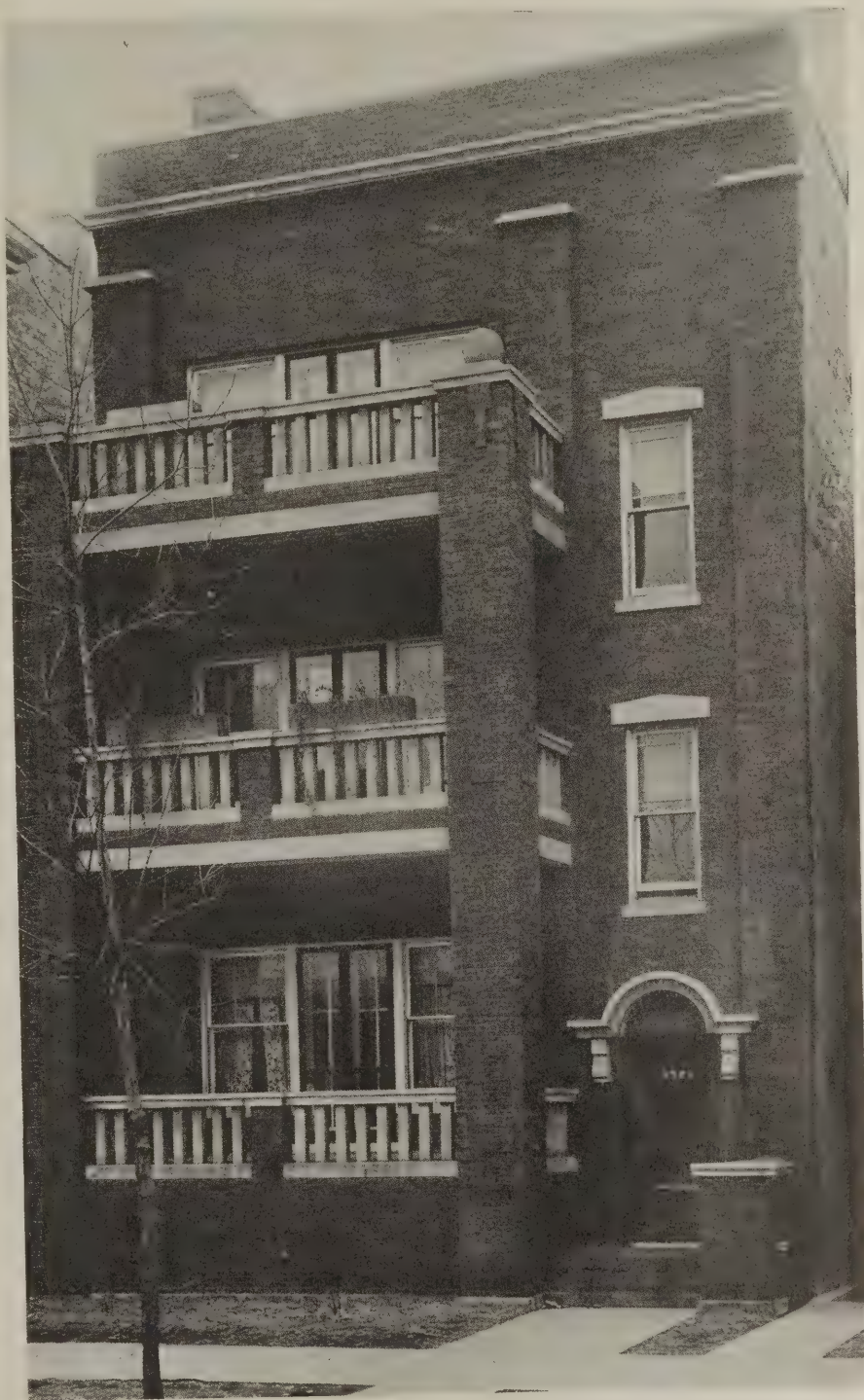
Rough-texture brick with a minimum amount of Bedford stone trimmings. These brick are "random-run" with five shades of red, mixed, laid with a close, tooled joint in natural-colored mortar. This is probably the cheapest type of brick front that is at the same time, attractive
