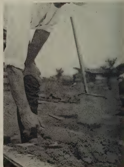
Fig. 3—Correct position in lifting mortar from board. Note position of thumb on top of trowel
