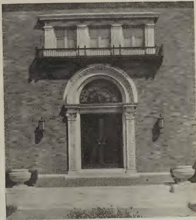
Plate 2—Entrance to a Kansas City, Mo., residence, Keene & Simpson, architects. An Italian Renaissance type in terra cotta combined with ornamental ironwork
