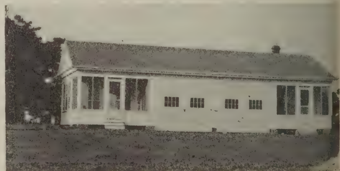
Plate 3—The servants' quarters and the garage are combined under a single roof
