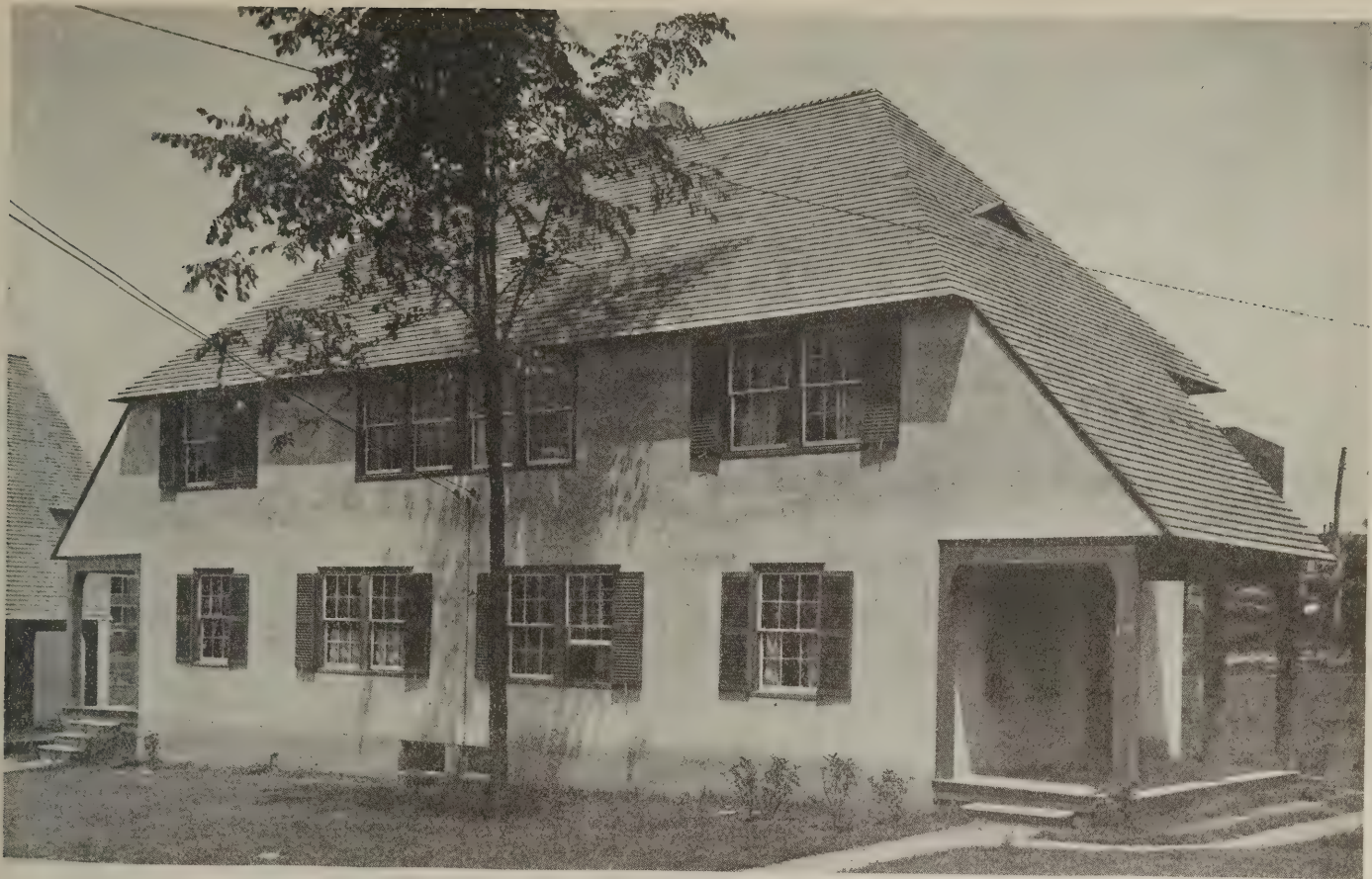
Fig. 2—Two-family, six-room houses at Waterbury. Murphy & Dana, architects
