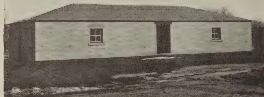
Concrete block potato, salt and flour warehouse at Detroit, Minn.
