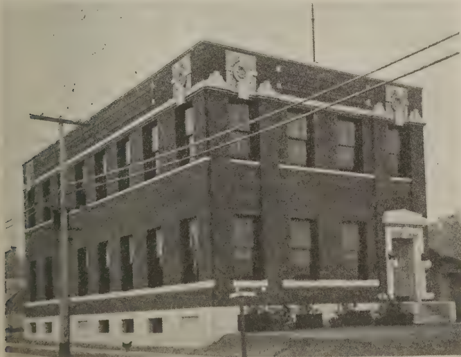
Plate 2—Branch telephone exchange, Dallas, Texas
