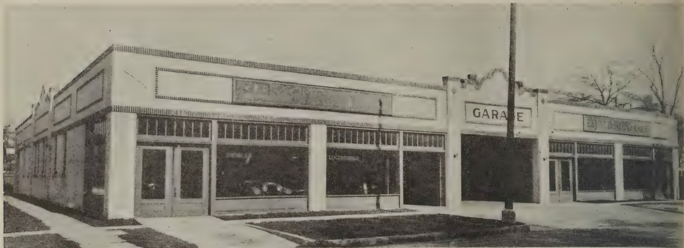
Plate 2—Stucco on brick with brick trimmings. The brick copings might give trouble in a severe climate
