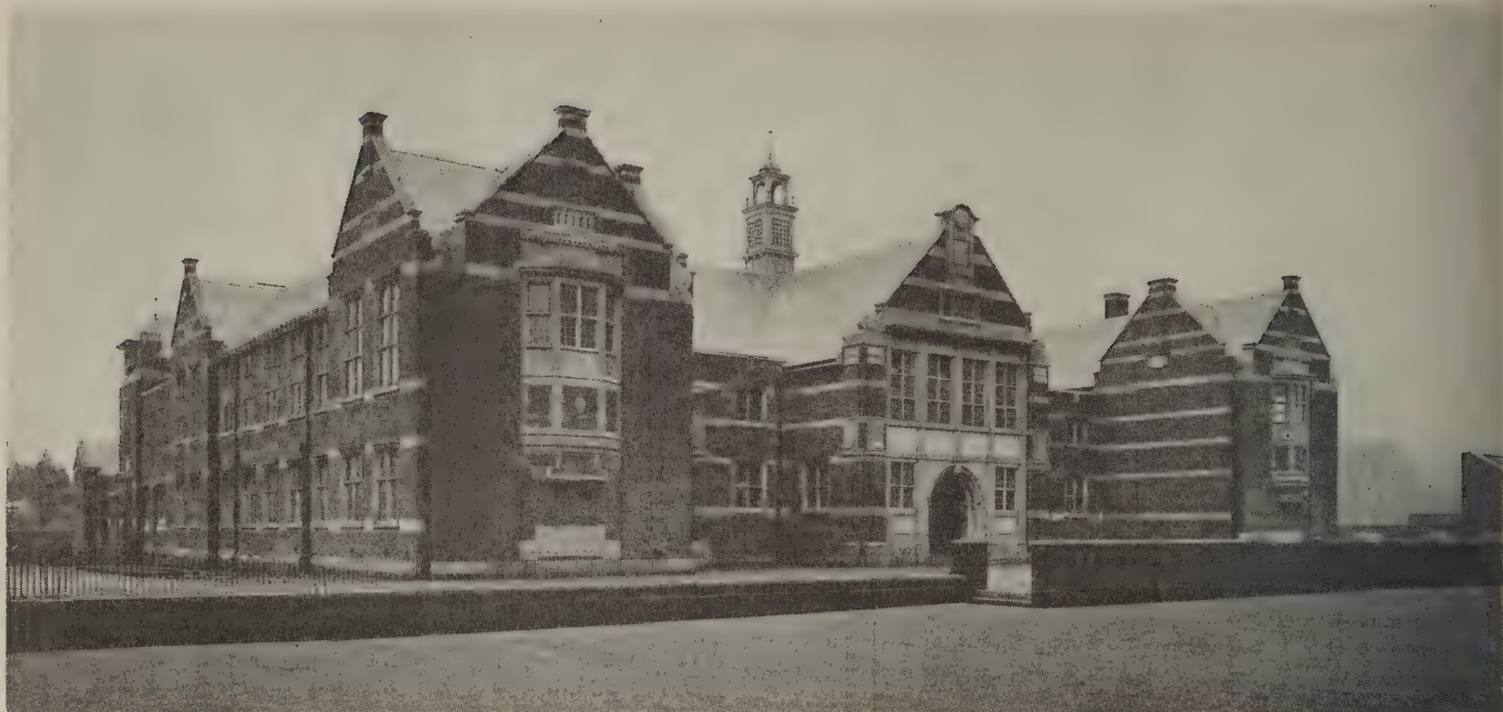
Grammar School, Stockport, England. General view of building showing how stone courses and trimmings may be laid to enhance the appearance of the brickwork
