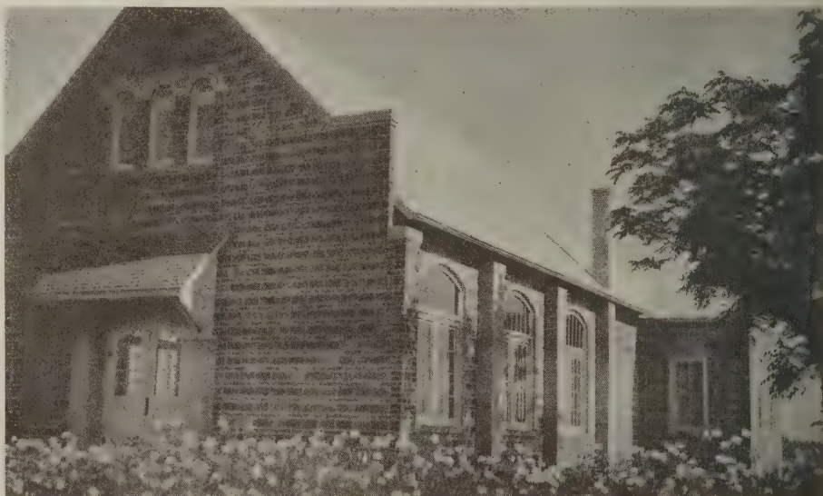
Hollow tile chapel at Luling, Texas
