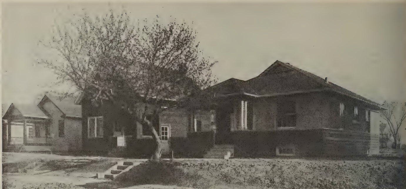
Plate 2—House C 1. A bungalow with a combination of stucco and clapboards on the walls
