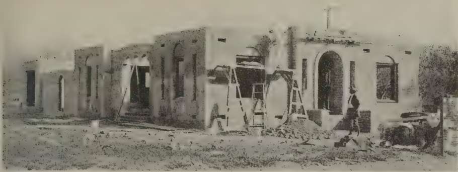
Fig. 3—The adobe wall completed and receiving the rough coat of cement stucco
