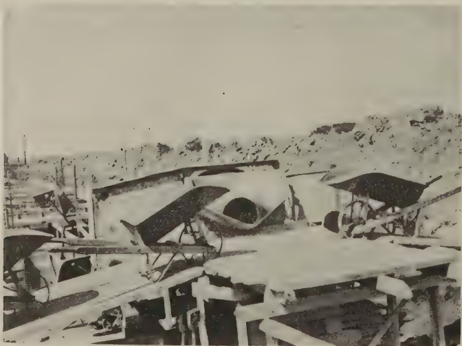
Fig. 5—Another mixer "on the job"
