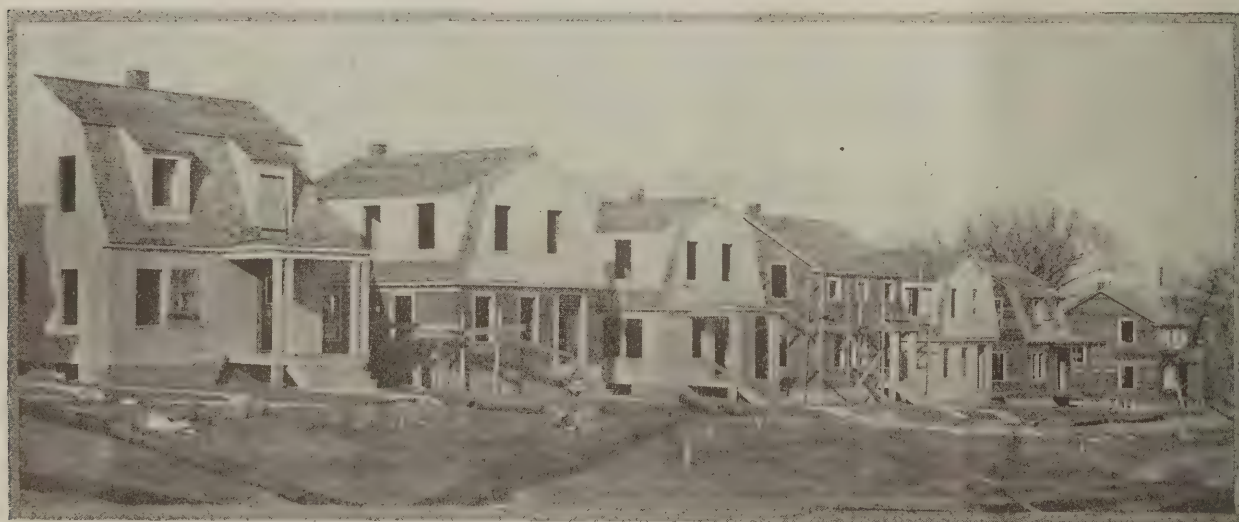
APPEARANCE OF THE HOUSES IN THE ROW Photographed during construction
