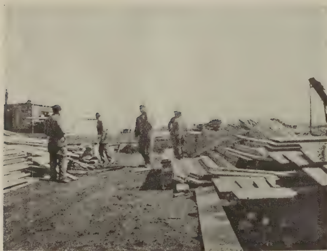
Fig. 3—Another power saw-rig in operation
