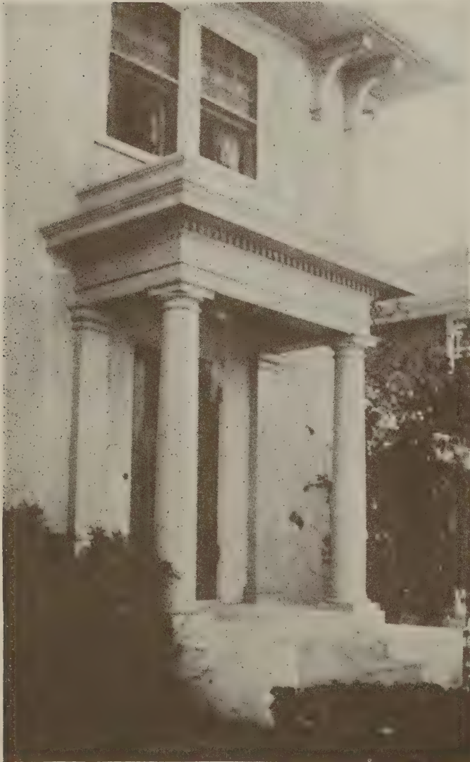
Plate 1—A simple Colonial entrance just a trifle wide for its height. A flower-box built into the top would be effective
