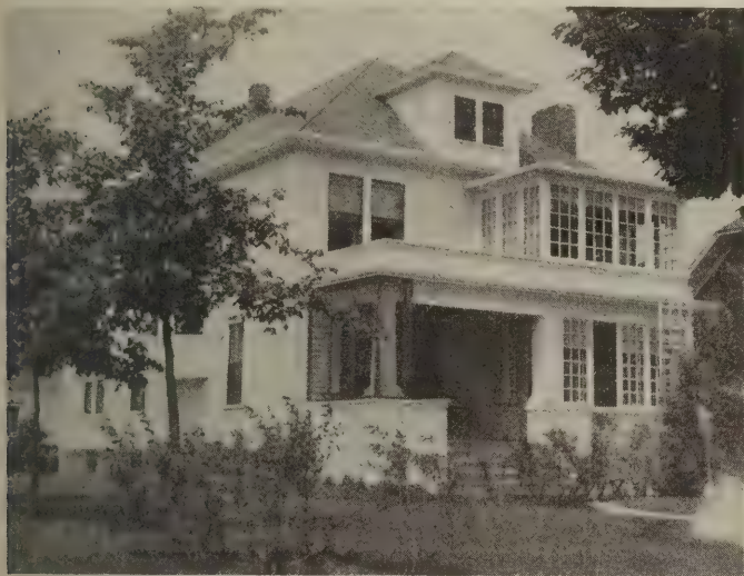
Plate 1—A remodeling job in which an old-fashioned porch is turned into a sleeping porch above and a living porch below
