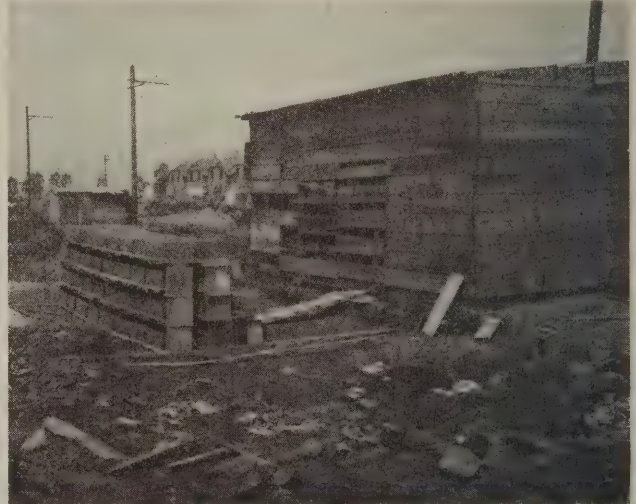
Fig. 2—Rings in curing process
