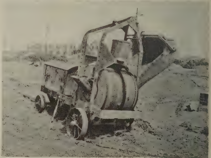
Fig. 4—Concrete mixer on the move
