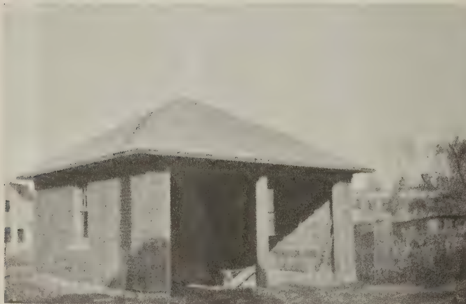
Plate 4—Garage at Davenport, Iowa
