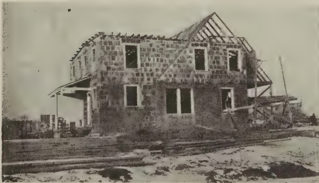
Brick-faced tile and ordinary tile—the latter ready for stucco
