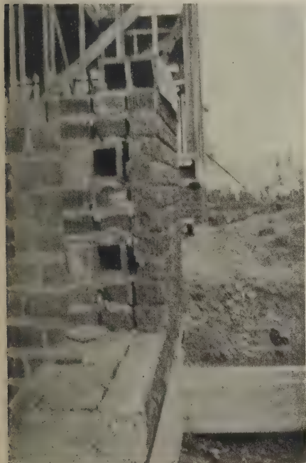
Plate 5—In this example short courses of tile were filled out with brickwork
