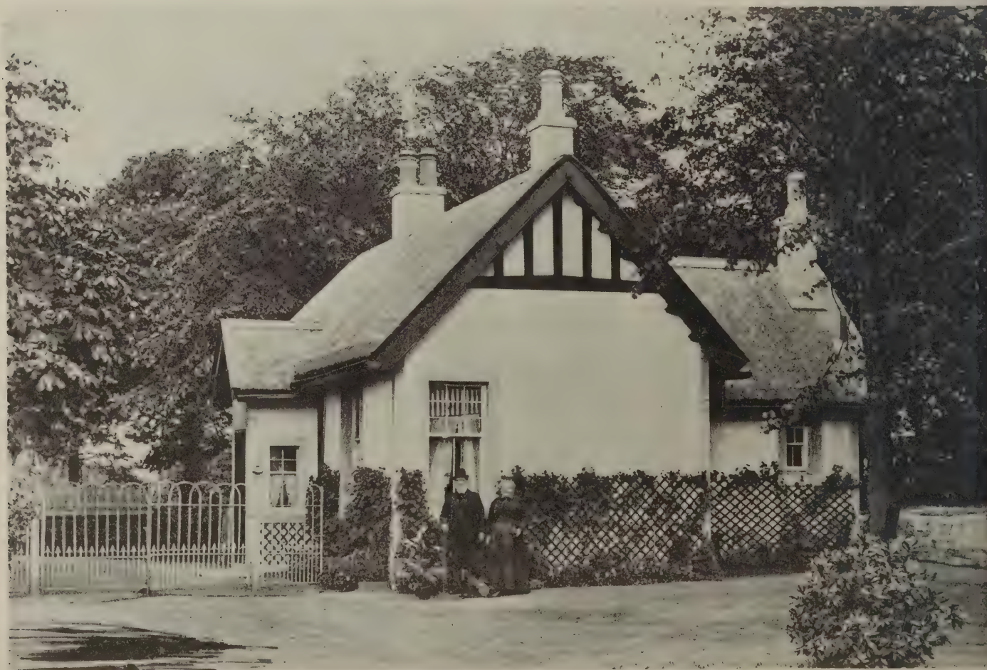
Fig. 5—Gate lodge showing gable end of thatched roof
