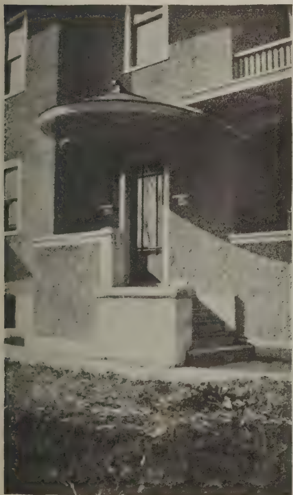
Plate 4—A semi-circular hood supported on stucco brackets forms this unusual entrance.
