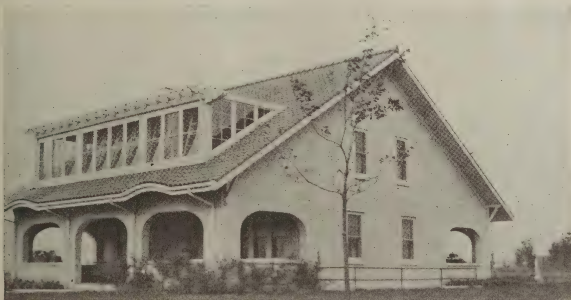
Plate 3—A sleeping porch built into a roof. Note the pergola effect of the pattern-sawed rafter ends
