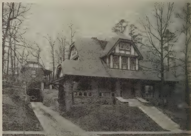
Plate 2—A garage dug into a hillside. Servants' quarters in the second story
