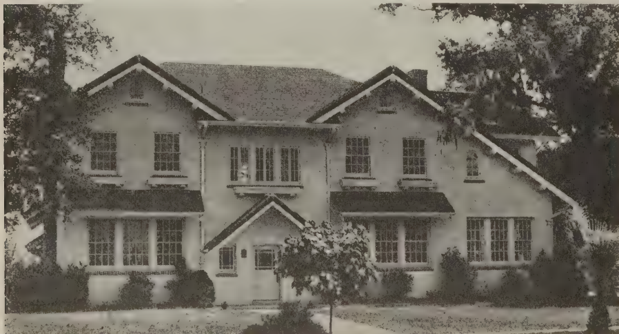
Plate 3—Stucco on hollow tile. Note the red brick window sills
