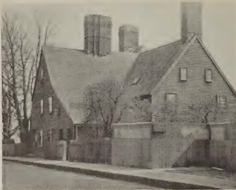
Plate 2—The chimneys of Hawthorne's "House of the Seven Gables," built about 1669. The chimney in the gable is comparatively modern
