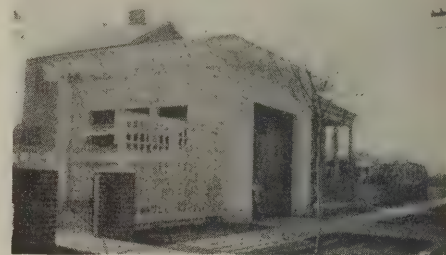
Fig. 8—Garage at New Orleans, La.
