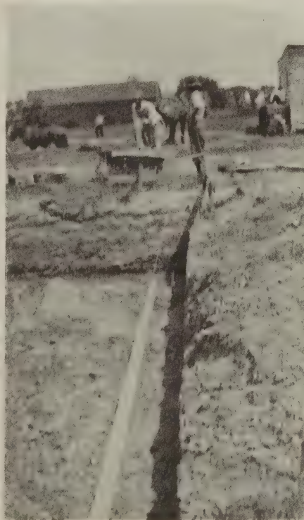
A two-by-four laid alongside of a footing trench forms a good working edge for leveling off concrete
