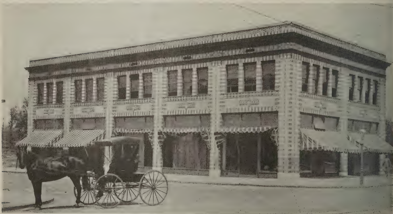
Plate 3—A "close-up" of the building shown at the right in Plate 2
