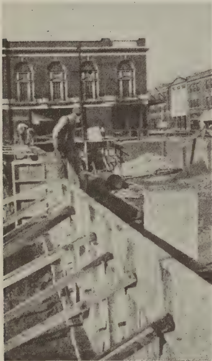
Plate 1—Wooden unit forms used for putting in a foundation for a store building
