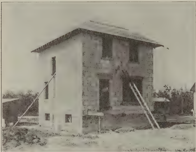
Gypsum-block house under construction
