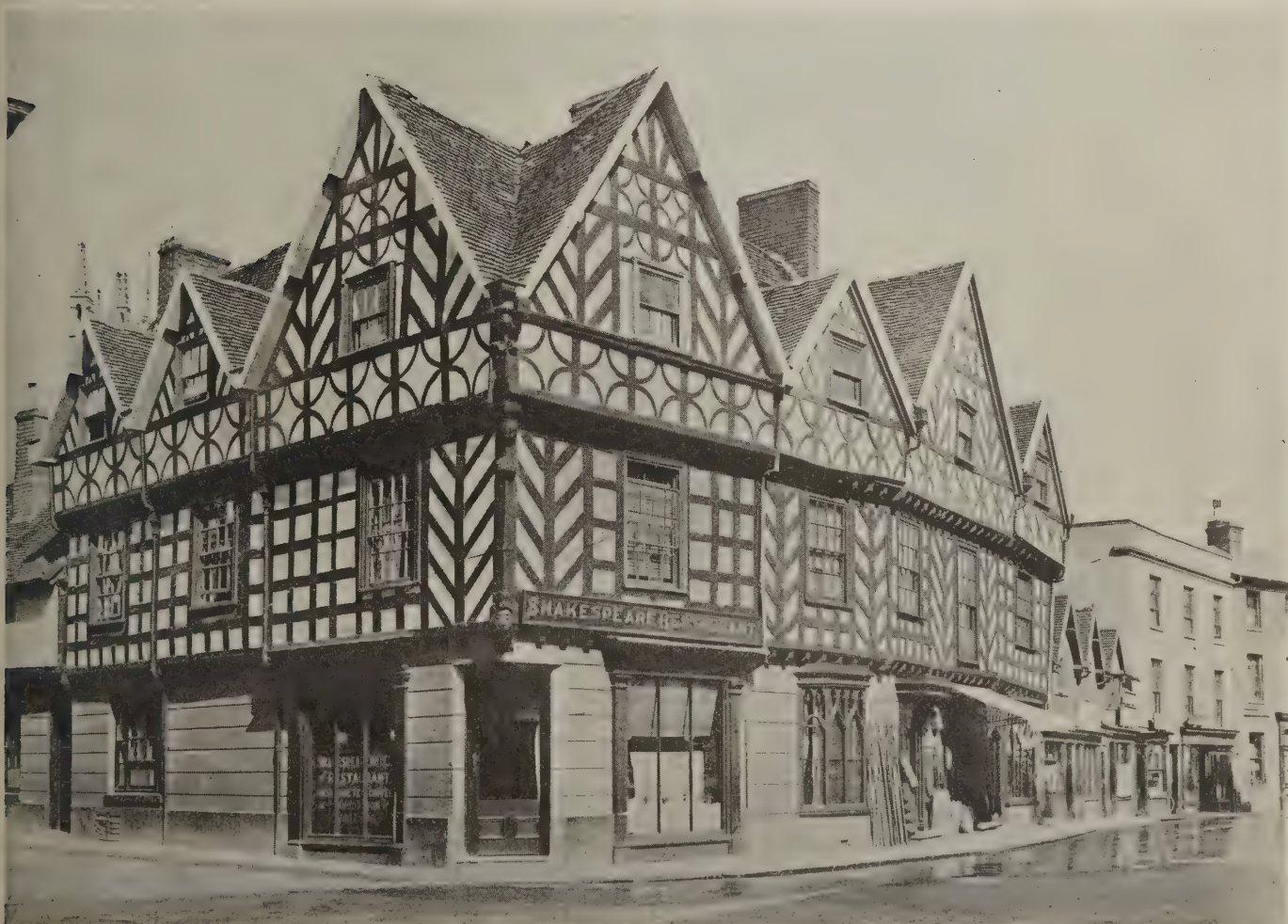
Fig. 6—The cement and timber gables of town architecture
