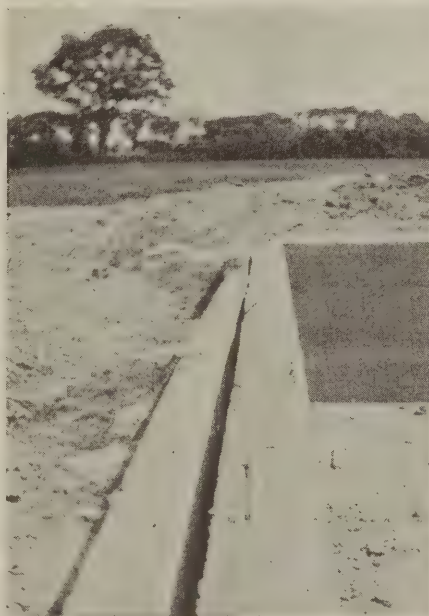
Plate 2—Anchor bolts in place ready to receive the wooden sill
