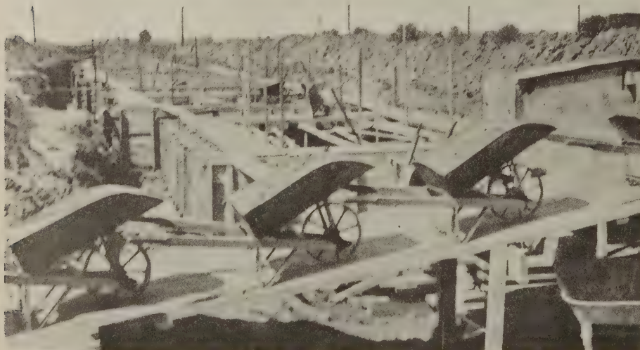
Fig. 9—New style charging barrow
