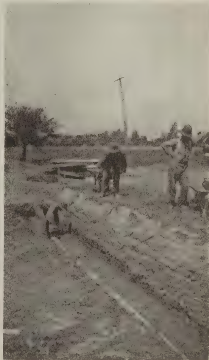
A two-by-four laid alongside of a footing trench forms a good working edge for leveling off concrete
