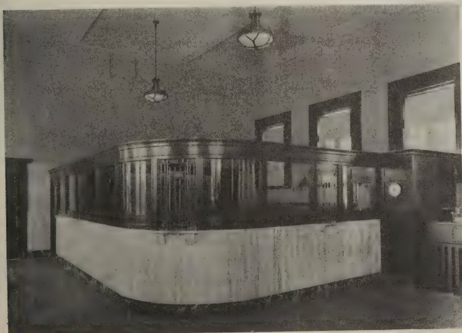
Plate 2—The interior of the Phoenix Bank showing the banking screen
