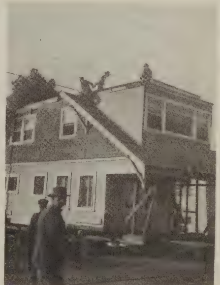
Work is continued while moving
