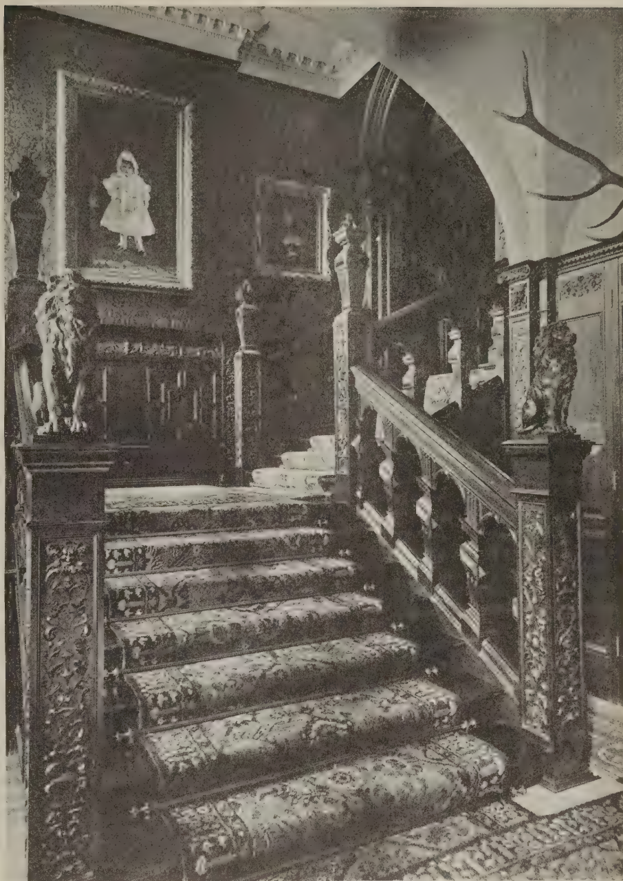
Fig. 2—Bottom of flight of an open newel stair, showing molded and carved newel posts and with square and raking balusters supporting the handrail
