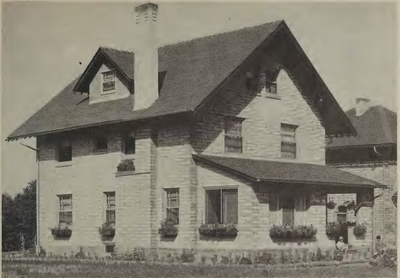
Figure 5. Nine room dwelling house of concrete block veneer and frame construction. The wall material is a cast block. Foundations are of monolithic construction. The roof is covered with red cement shingles
