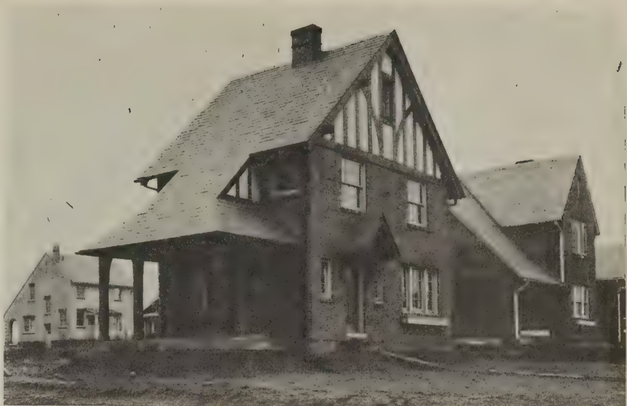
Plate 2—The wall of the house in the foreground is laid with a special hollow tile made with a brick face. The other houses are of stucco on hollow tile
