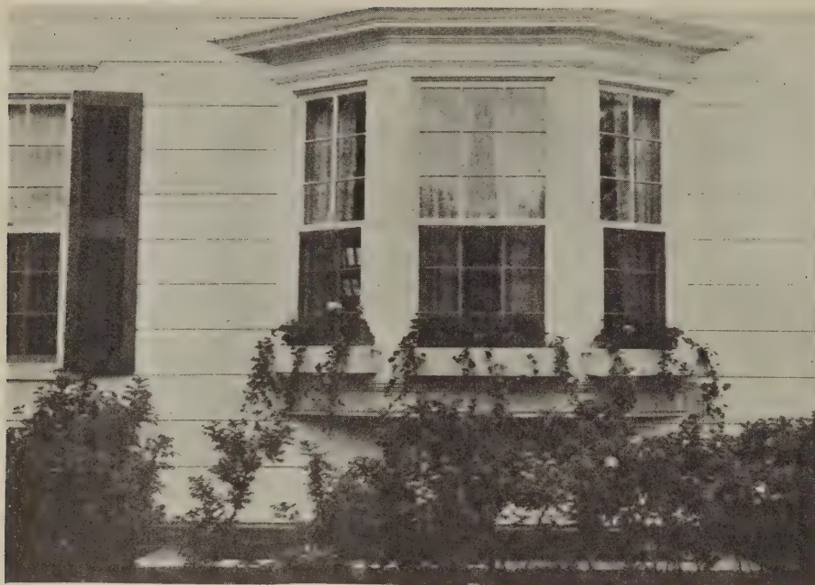
Inexpensive exterior details: drop siding with "stock" casings around the windows
