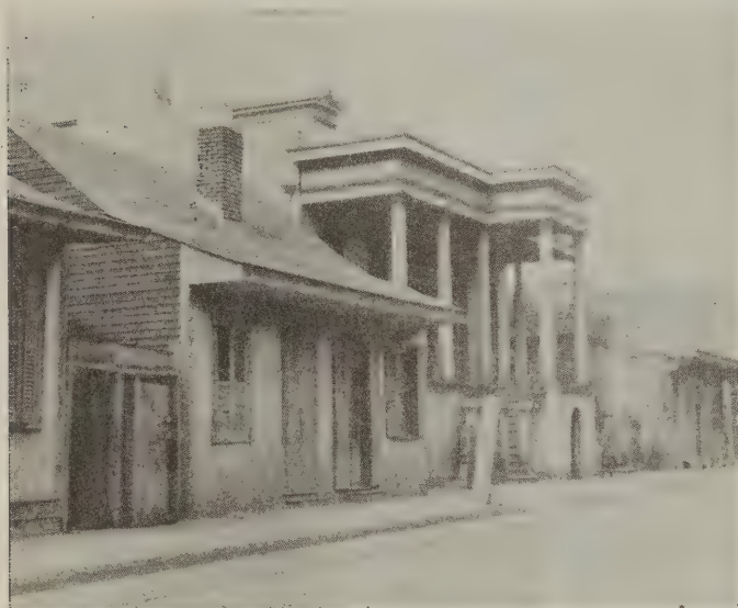
Plate 1—Old stucco walls in New Orleans
