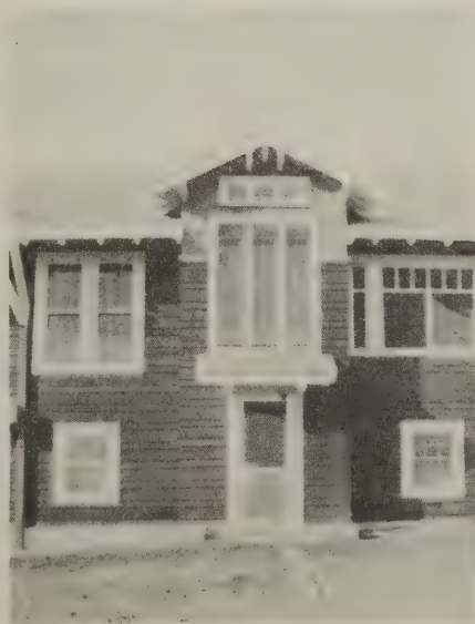
Plate 3—Detail of one of the entrances
