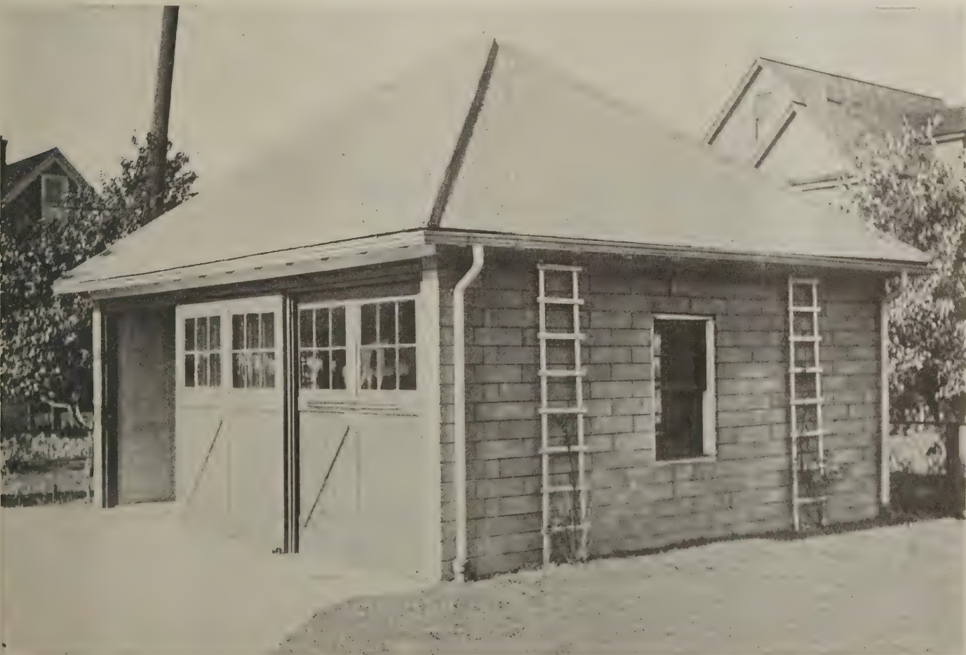
Plate 1—Attractive two-compartment garage of plain face concrete block, interior plastered directly on block
