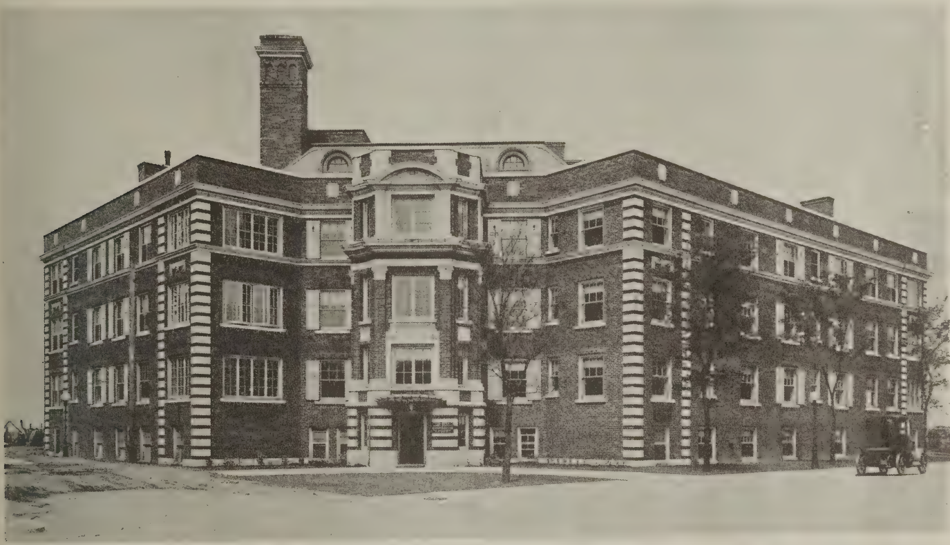
"Texture" face brick was used in this large apartment building, with architectural terra-cotta trimmings. The latter is white-glazed and the appearance of the building is fresh and attractive
