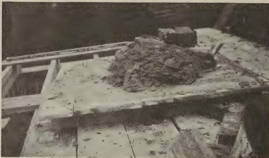
Tidy mortar board and scaffold
