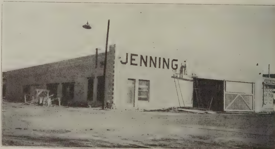
Warehouse at Douglas, Ariz., built of hollow gypsum blocks
