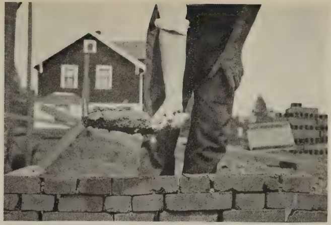
Fig. 5—Incorrect. Thumb should be on top of trowel
