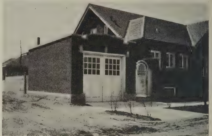
Plate 3—Garage at Chicago, Ill.
