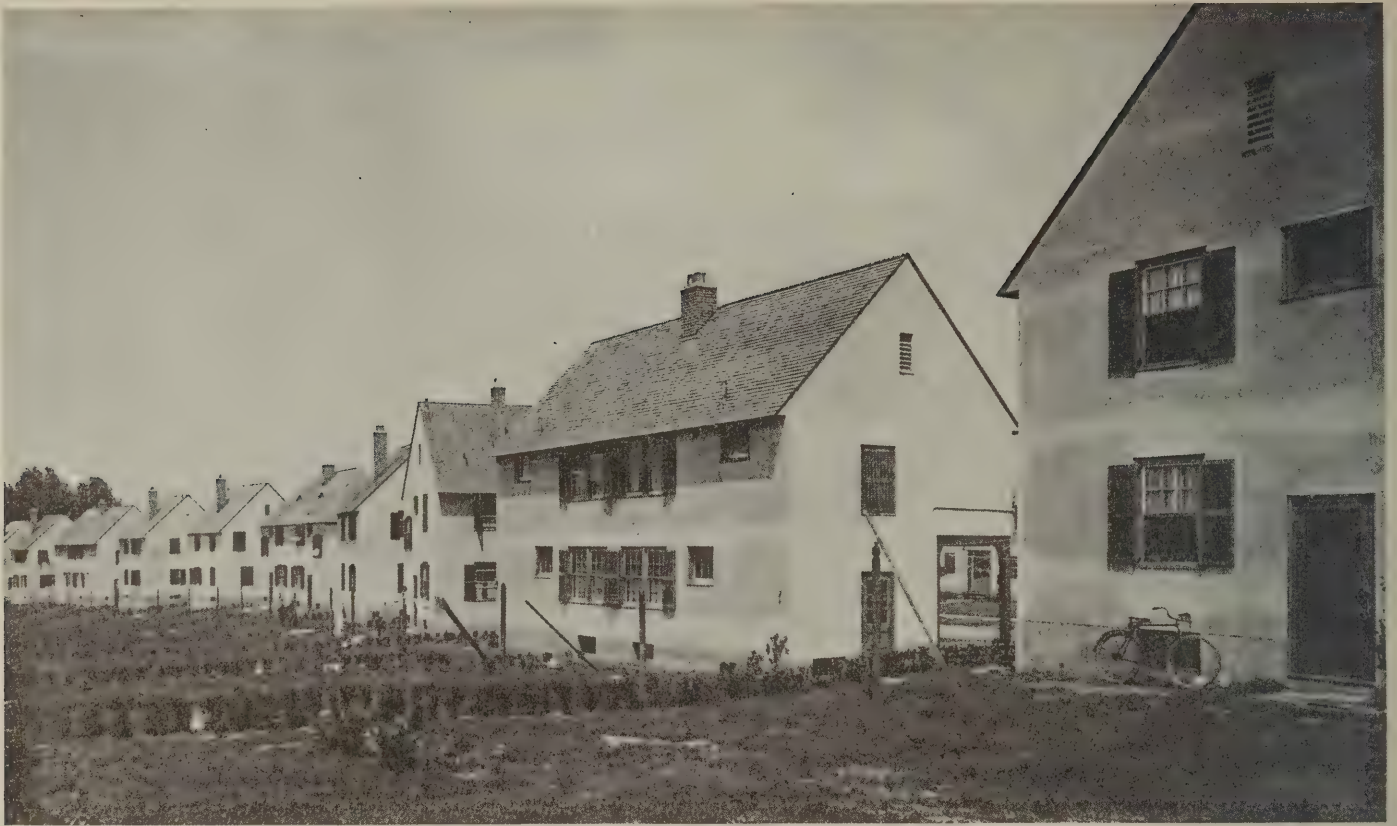
Fig. 5—Rear view of some of the houses at Waterbury. Murphy & Dana, architects
