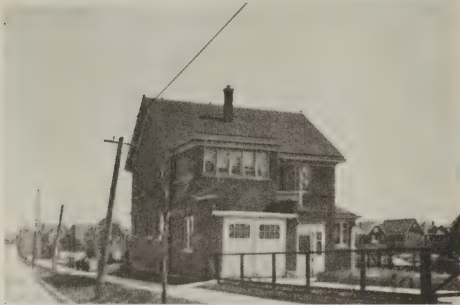
Plate 2—Garage and house at Milwaukee, Wis.
