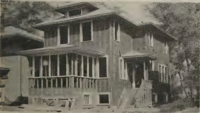
Plate 7—Ready for its stucco "skin"
