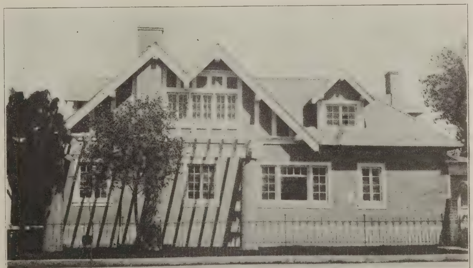
House at Douglas, Ariz., built of hollow gypsum blocks and surfaced with gypsum stucco
