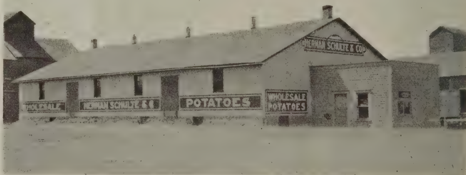
Clay brick potato warehouse at Hawley, Minn.
