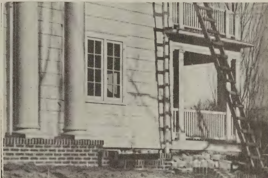
Plate 2—In some sections field stones instead of the brick specified, might be used for facing the foundation; the difference in cost to be used in cancelling an "extra" for facing the foundation; the difference in cost to be used in cancelling an "extra"
