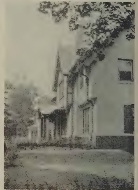
Plate 2—Stucco is used on large as well as small houses
