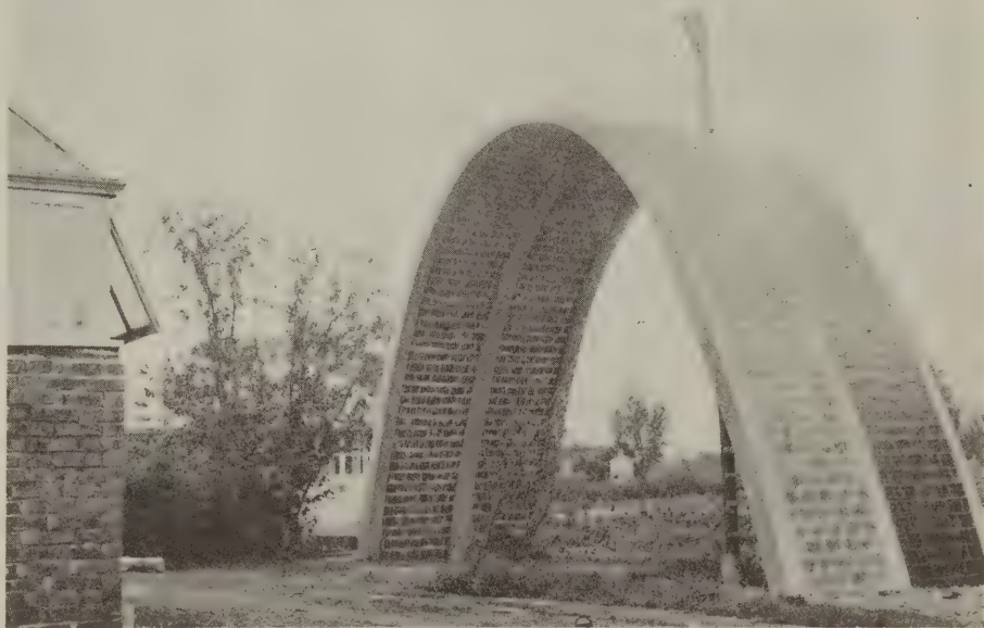
Arch demonstrating an economical form of construction for farm machinery sheds
