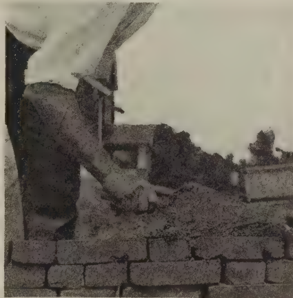
Fig. 6—Correct. Beginning to spread mortar. Notice fingers commencing to loosen as weight leaves the trowel
