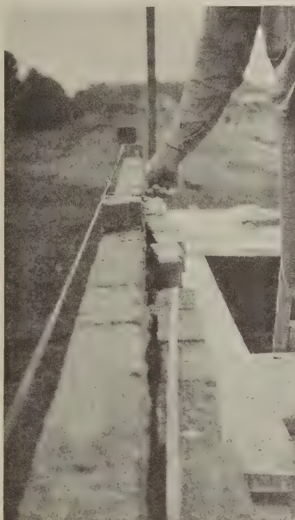
Placing a "trig"
