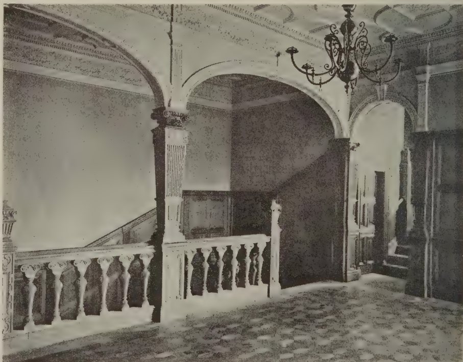
Fig. 1—Top landing of an open newel stair, showing the newel post panelled and carved, and with volute top balusters
