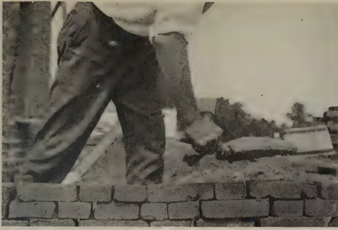
Fig. 4—Correct. Bricklayer ready to spread mortar on wall
