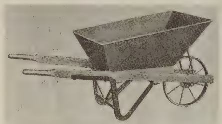
Fig. 8—Self-measuring concrete barrow
