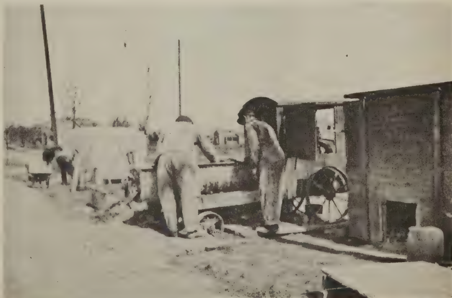
Mixing mortar with a concrete mixer
