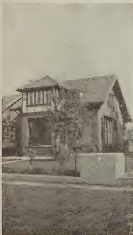
Plate 5—A sleeping porch over a rear porch. Stucco and half-timber is well suited to details of this nature
