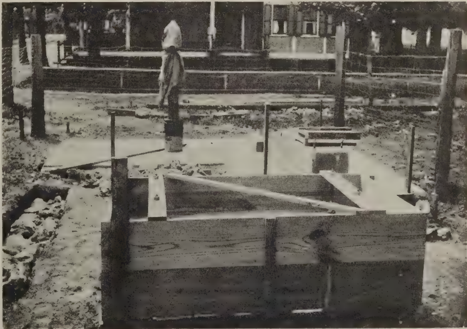
Fig. 2—Completed forms for simple machinery base with template and engine bolts in place, ready for the concrete
