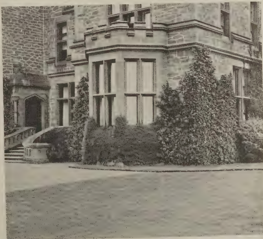
The walls on this house are built of polygonal rubble with stone dressings at the opening and corners
