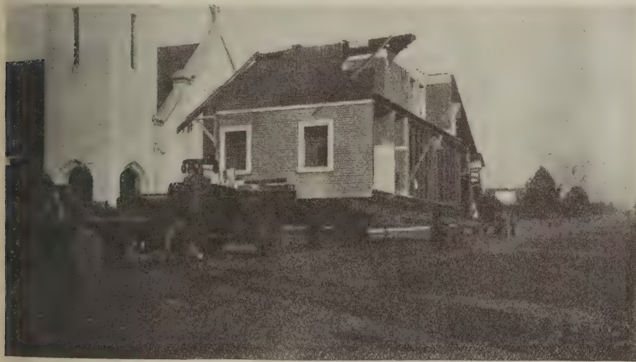
Moving houses with motor trucks
