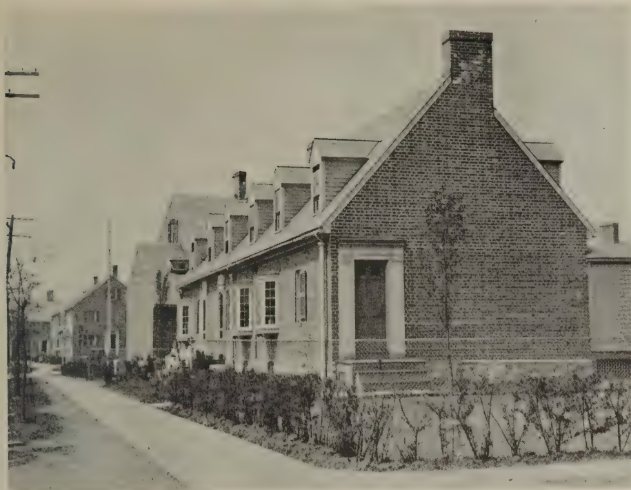
Plate 12—A row of three K-8 houses. Crane Tract
