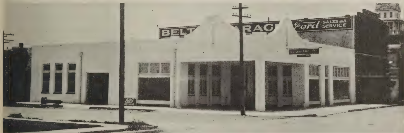
Plate 2—A public garage at Belton, Texas. A simple treatment that could be improved by a more careful study of the openings at the corner
