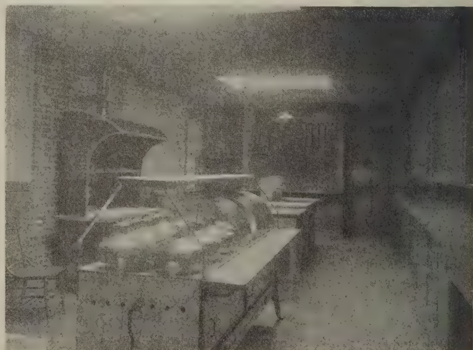
Fig. 5—The kitchen is up-to-date in its arrangement and equipment
