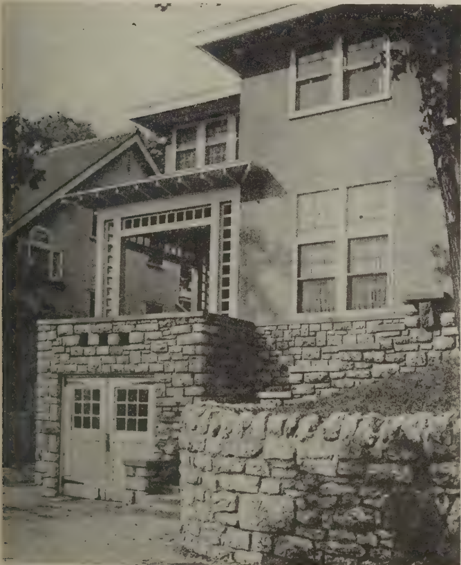
This house being situated on a hillside, the garage is in the rear and a part of the basement, and reached from a rear alley. The garage and basement walls and foundation are of stone. Directly over the garage is a rear porch, and over the porch is a glassed-in sleeping porch. Located in Kansas City, Mo.
