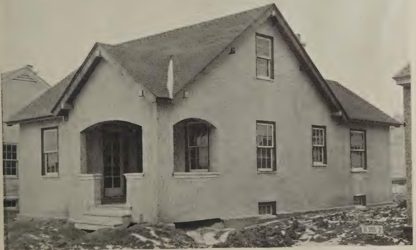
Fig. 7—Many of the bungalows have large attics
