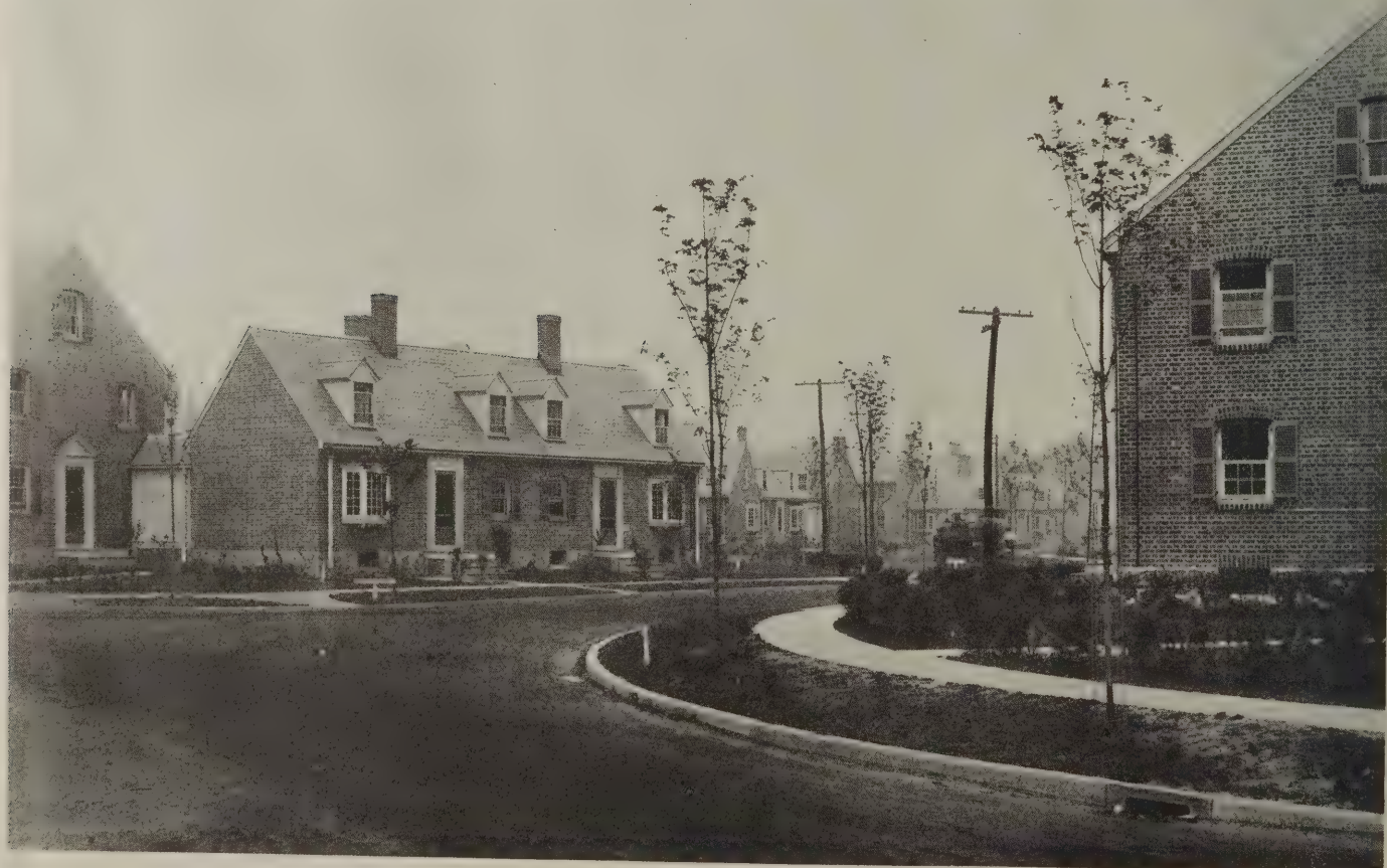
Plate 15—At the left two K-12 houses joined to a K-8-9 and 10 group. Crane Tract
