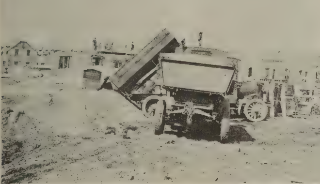
Fig. 9—Trucks unloading sand and gravel for concrete
