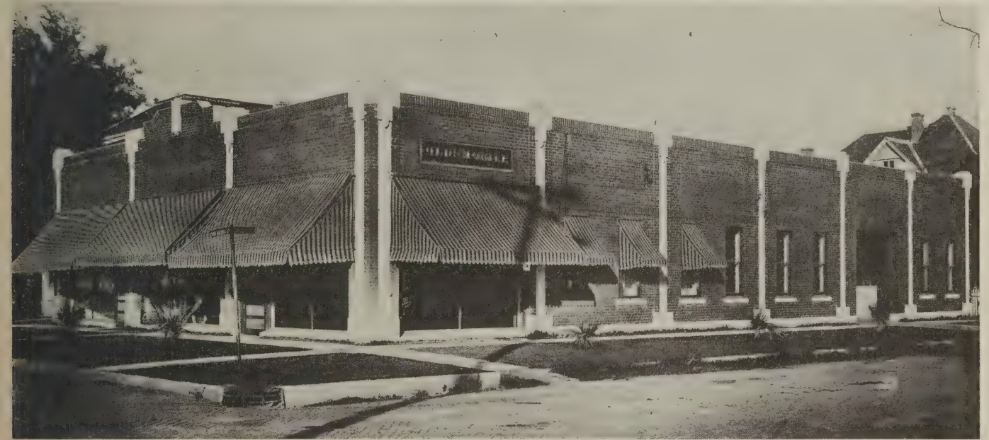
Plate 1—Brick walls with cement stone trimmings. Note the show windows which extend almost to the floor level
