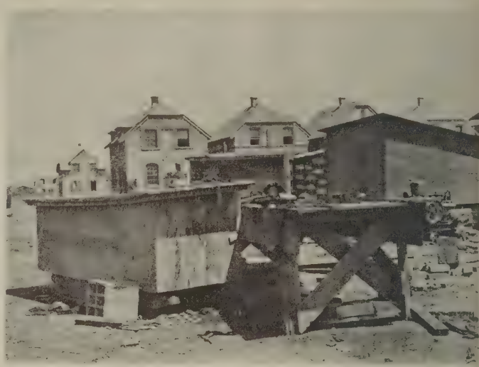
Fig. 2—Portable machine for bending reinforcing rods, conduit, pipe, etc. Power pump in background
