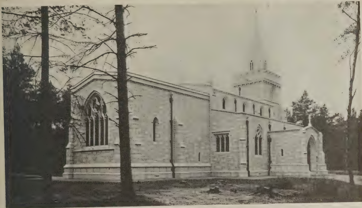
Granite church showing irregular coursed or snecked rubble
