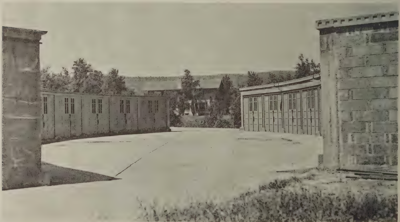
Figure 3. Circular community garage of concrete block, built like a round house. It occupies a small almost circular plat of ground, surrounded by a high class residence district. The structure will be entirely concealed by landscaping, making the whole space occupied by the garage appear from the residences like a beautifully wooded knoll
