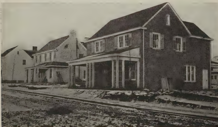
Plate 3—All of these houses have hollow tile walls. They are variously finished with brick veneer, plain stucco and half timber
