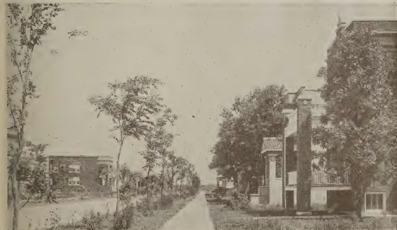
Plate 2—A subdivision showing two-flat buildings which, in this instance, were sold as fast as they could be built. The best way to operate is to build first on alternate lots, and then improve the vacant lots between. Johnson and Tyden, Builders
