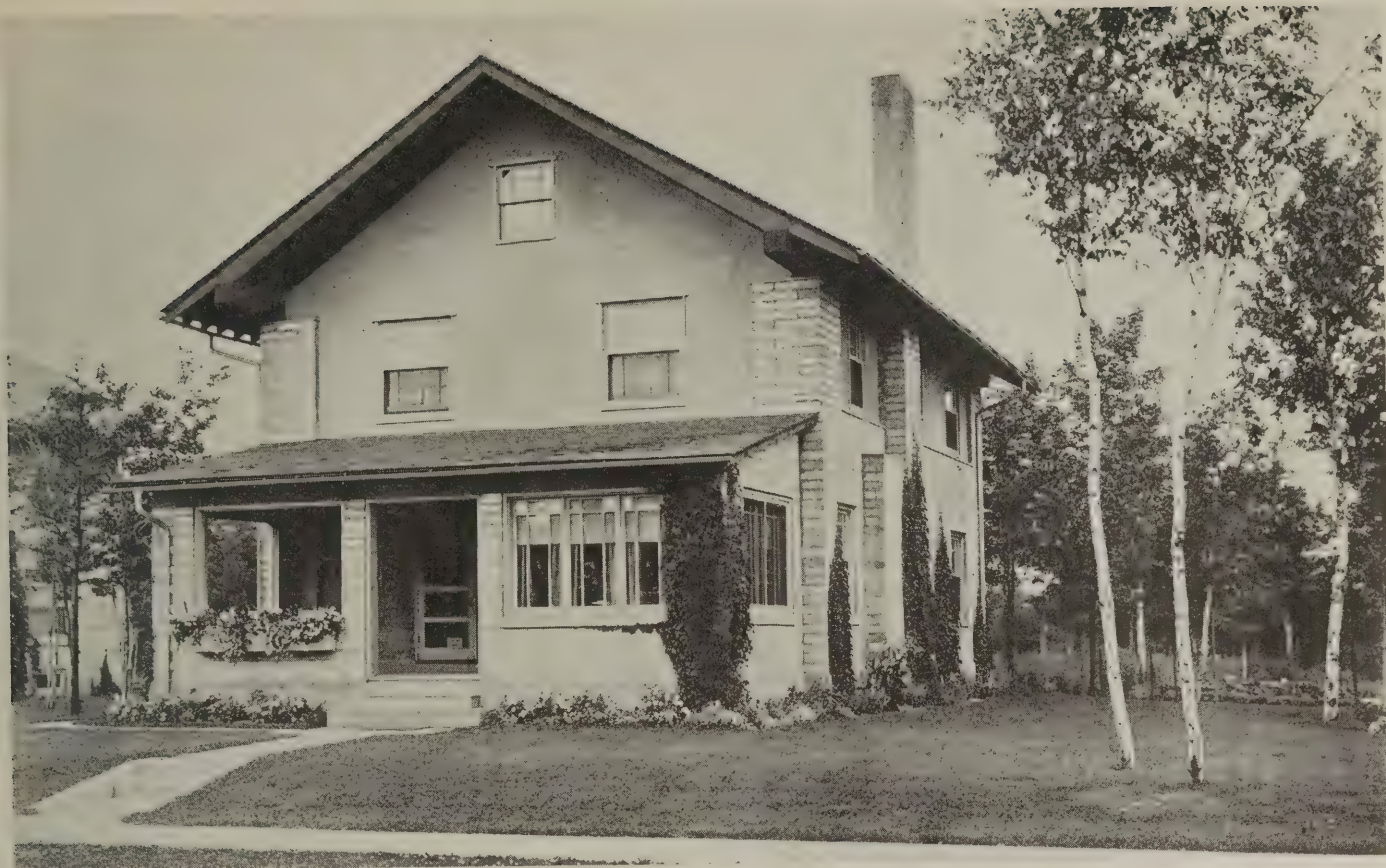
Figure 7. A type of wood frame house in the Morgan Park group, surfaced with concrete veneer block and portland cement stucco. The floor plan of this building is quite similar to that shown in Figure 6, with the exception that no rooms have been finished off on the third floor, since the roof is somewhat too low for good ceiling height
