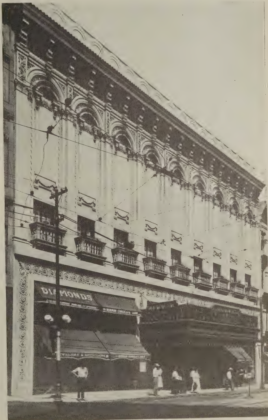
Plate 1—Newman Theatre, Kansas City, Mo., A. J. Drake, architect. A very attractive design in terra cotta. The absence of a large sign disfiguring the front is commendable
