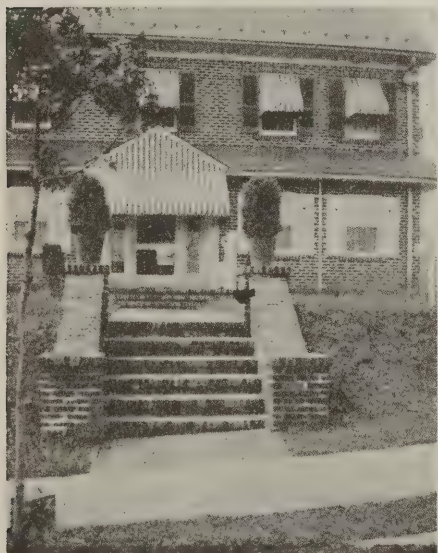
Plate 5—The upper portion of entrance awning is flat against the gable, while the lower portion is hooded
