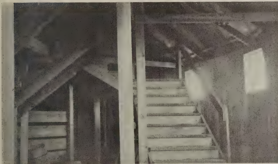
Fig. 3—Rear stairway to pavilion seats
