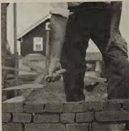
Fig. 2—Incorrect. Note "stranglehold" on trowel. Fingers and thumb tight and rigid
