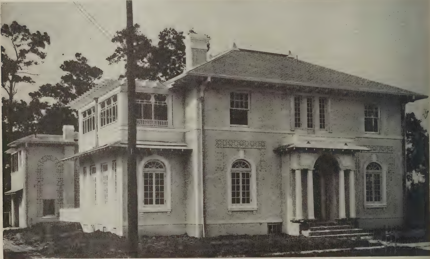
Plate 1—The unfinished entrance and uncompleted grading and planting detract considerably from the appearance of the house
