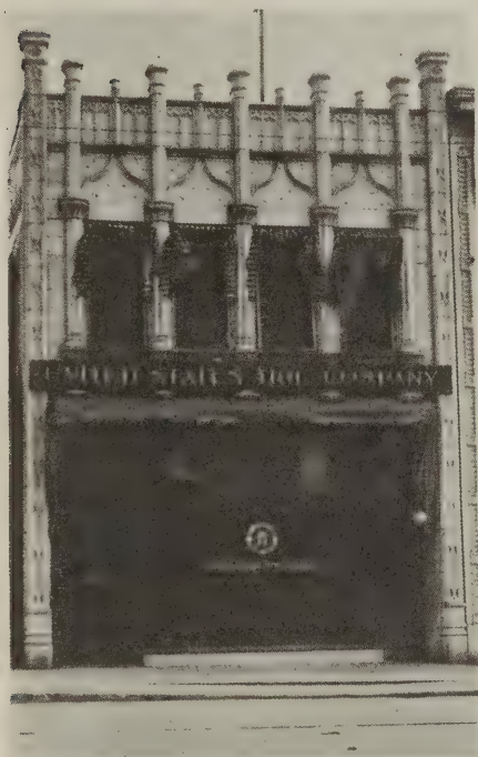
Plate 5—Store and office building, Oklahoma City, Okla.
