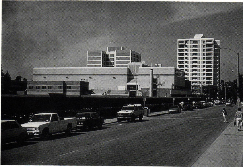
5. Recreational athletics building and dormitories, University of Southern California, 1993.
