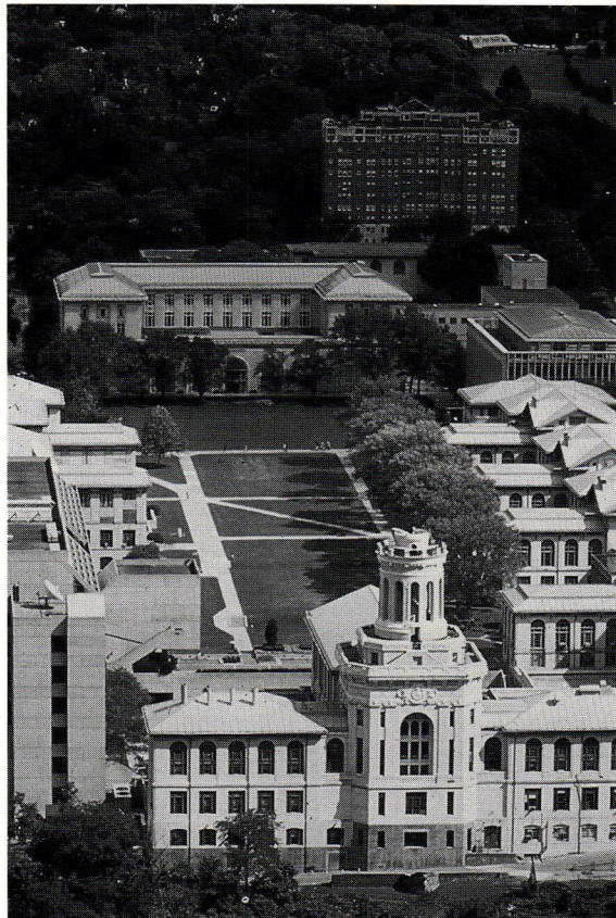
11. Aerial View of Hornbostel Mall, Carnegie Mellon University.
