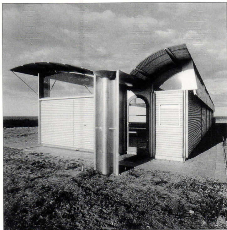
Fig. 13. Moruya House. Rain water—which is collected in huge cisterns underneath the building—is the only water supply in much of Australia.
