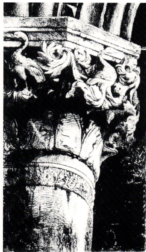
Fig. 4. Artistic expression in the play of light and shade in Venetian Gothic architecture, from The Seven Lamps of Architecture .
