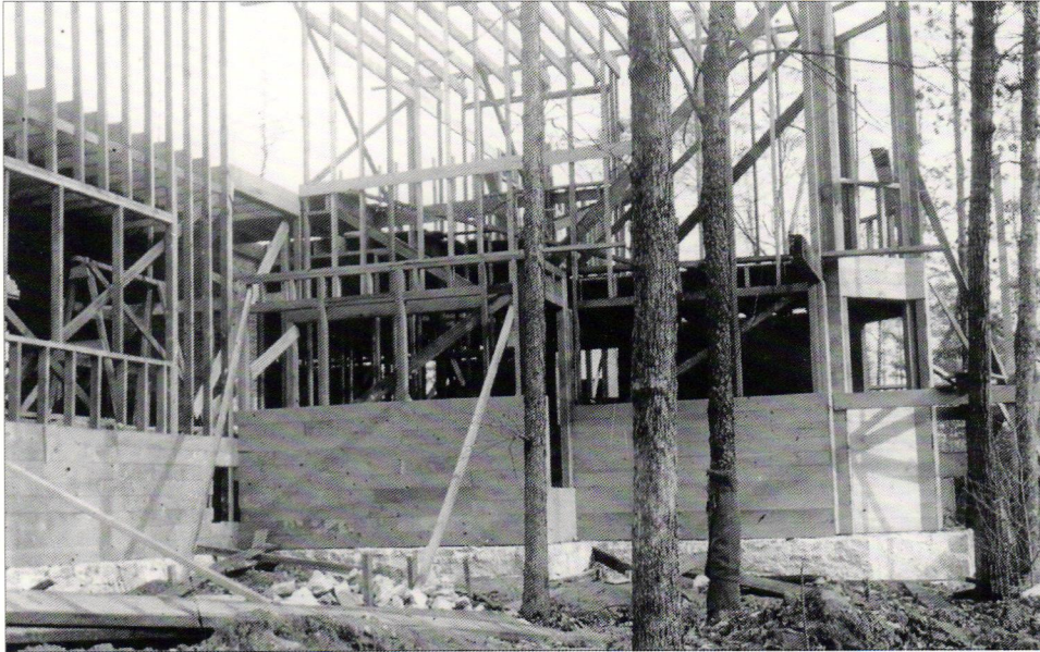
Fig. 6. Construction photograph of the Willits house balloon frame.
