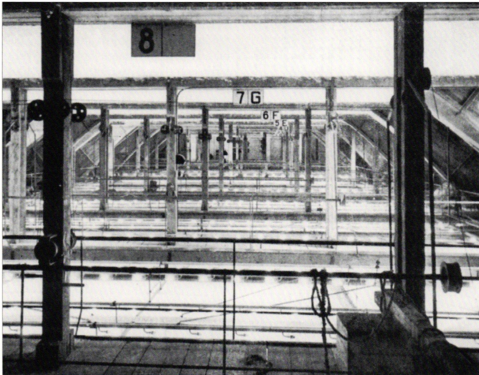
Fig. 8. View of large auditorium ceiling showing lighting system, Jaques-Dalcroze Institute of Rhythmic Gymnastics.
