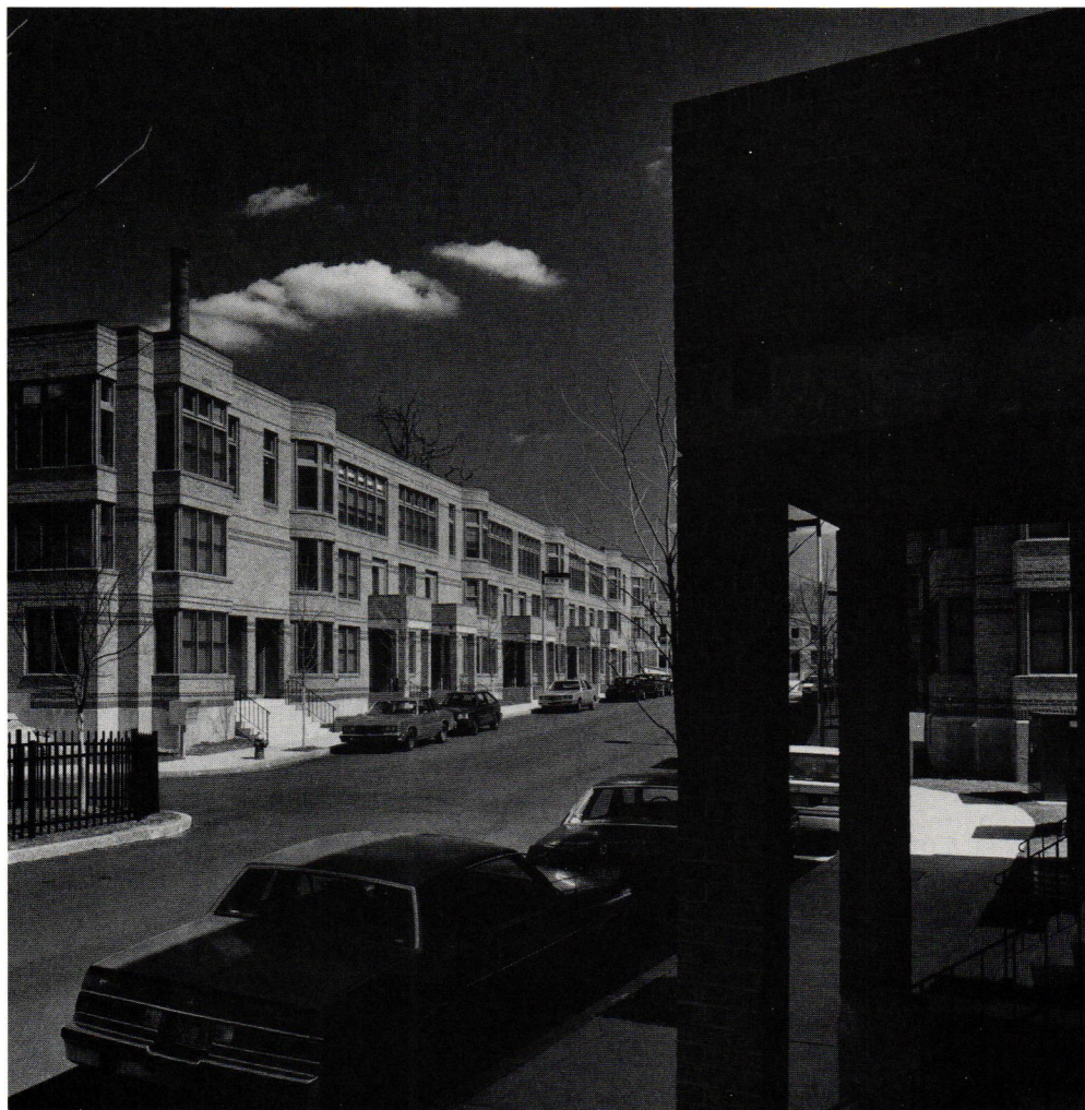
Mission Hill homes were sponsored by the Bricklayers and Laborers Non-Profit Housing Company. © 1990 Steve Rosenthal
