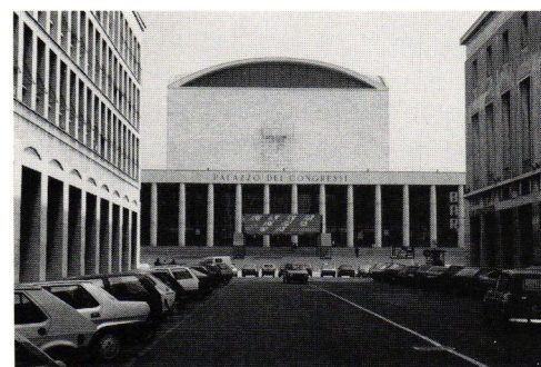
Ill. 10 EUR, Palazzo dei Congressi. Adalberto Libera, architect, 1938. View from viale della Civiltà del Lavoro. The giant portico screens a vast glass wall articulated by reticulated vertical mullions. The central cube is topped by a cross vault with glazed lunettes.
