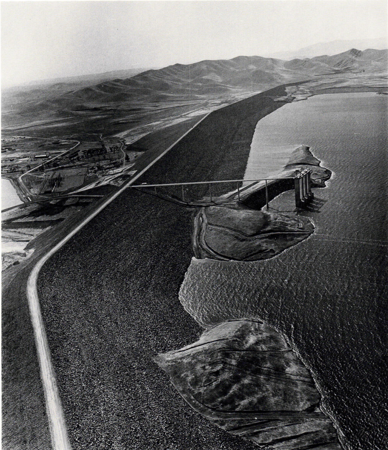
37 California Aqueduct, San Luis Reservoir, aqueduct water storage.
