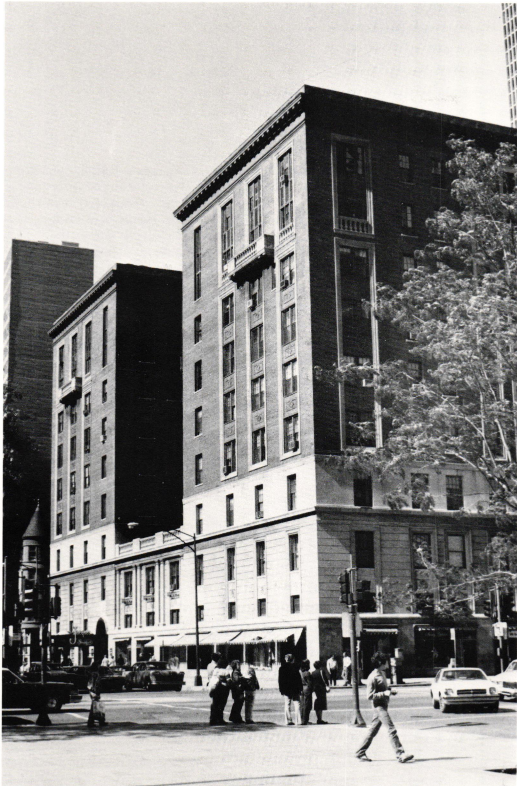
9 900 North Michigan Avenue, Chicago. Jarvis Hunt, 1925-26. View of south facade from John Hancock Tower plaza.
