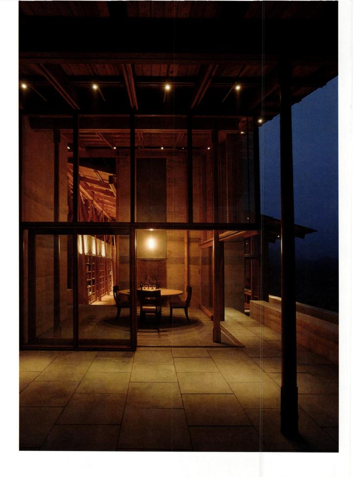
as concrete. The walls are three feet wide at the base and narrow to twenty-six inches at the top. As they rise, alternating dark and light striations are evident, an apparent haphazard result of the rammed earth process. But they're not haphazard at all. "The striations are deliberate—I drew them that way, on occasion going to the forms and marking them up," Cutler says.
