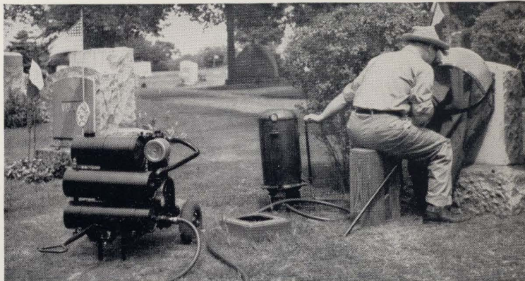
This compact and economical Lindsay Sandblast Outfit will cut average inscription letters in less than two minutes each.
