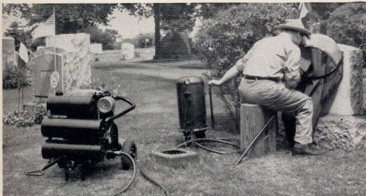
This compact and economical Lindsay Sandblast Outfit will cut average inscription letters in less than two minutes each.
