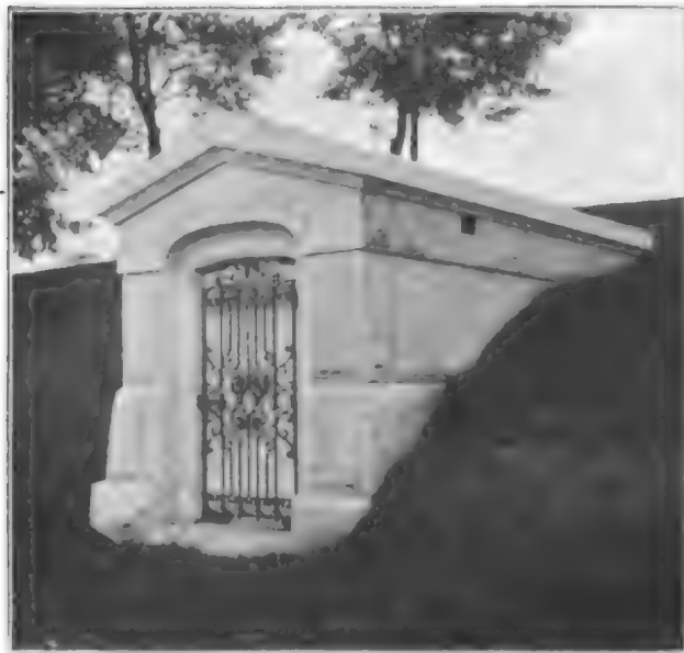
BRAYNER MAUSOLEUM, HARLEIGH CEMETERY, CAMDEN, N. J. HARRISON GRANITE CO., NEW YORK, CONTRACTORS.
