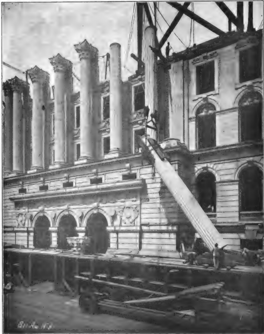
LIFTING A 40-TON COLUMN TO POSITION ON THE NEW HALL OF RECORDS, NEW YORK
