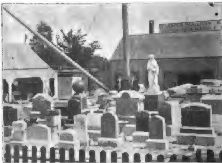
PARTIAL VIEW OF PLANT OF JNO. B. SULLIVAN & SON, TAUNTON, MASS.
