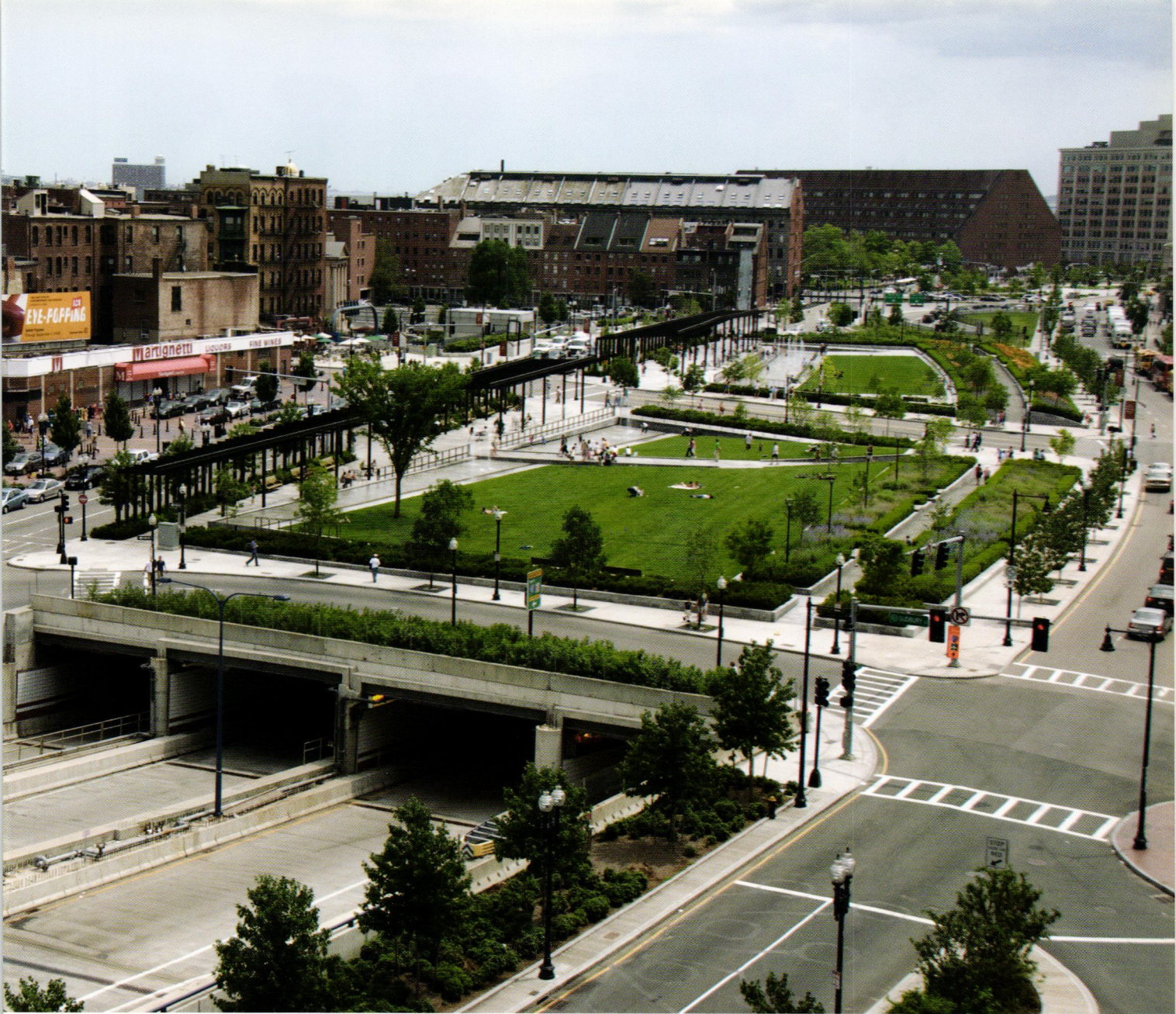
View of Greenway and northern entrance to the Central Artery Tunnel
