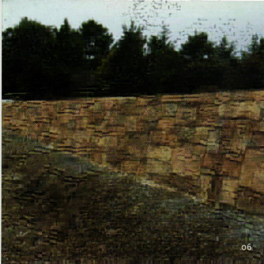
CalTrans Stacked Stone Texture on Concrete Barrier Type 60, 2003
