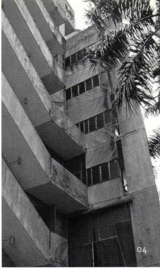
Exterior fire escape on east side of building, Ongard Satabhandhu's Building 9
