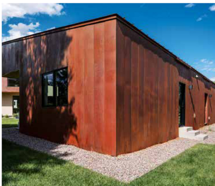
The Land+Shelter studio volume, wrapped in Corten steel, makes an exterior statement that visually differentiates it from the family home. The materials were chosen to play off the colors of the Roaring Fork Valley's natural geology.
