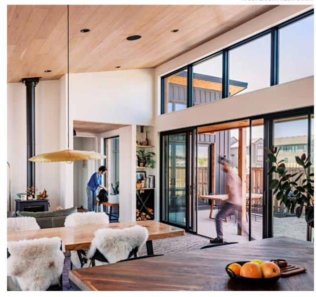
shadow boxes fit around each of the window units, creating depth and horizontal movement.
