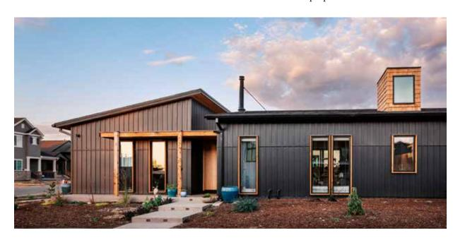
UNUM Collaborative's three-mass plan called for separate volumes for the living quarters, sleeping quarters, and garage, all connected by a series of breezeways and bridges. The low angle of the shed roof was placed at street side and opens toward the center courtyard. The vertical cedar-shake dormers serve as architectural portals that signify a sense of place within the home.
