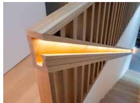
The stair rail detailing is Meridian 105 architect Daniel Lipscomb's design, and was executed by a woodworker on site. The rail is made of two solid wood pieces and includes a carved-out, LED-lit channel for the hand to follow. LEFT: A piece from artist Éric Nado's Typewriter Guns series, in which the artist meticulously sculpts objects out of recycled typewriter parts as a commentary on gun culture, is installed at the end of the upstairs hallway.
