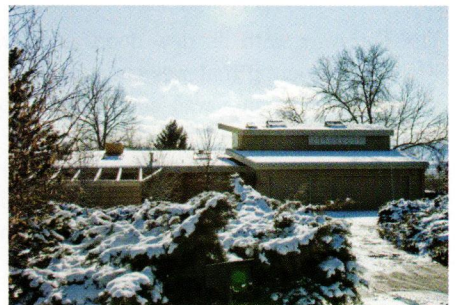
ABOVE TOP: The house during construction. The roofing of the existing carport to the left was removed, leaving beams to form a trellis over an entry court.
