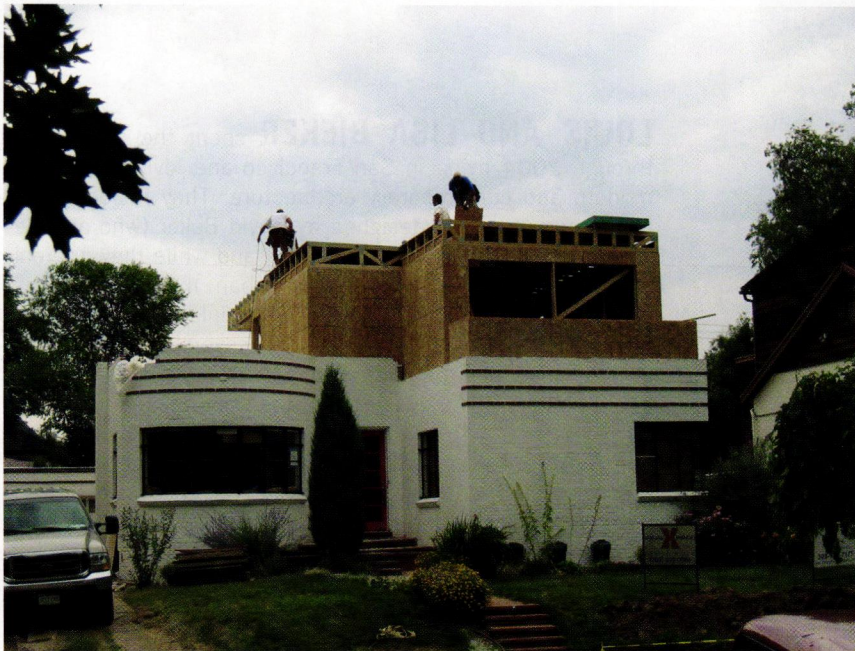
Above: Workers fitting the framing, sheathing and subfloor of the second-story addition together like puzzle pieces. Right: Louis and Lisa did all of the interior design work themselves. Louis recalls mentally arranging furniture before the couple purchased the home.
