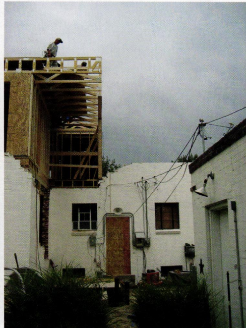
Above: Workers fitting the framing, sheathing and subfloor of the second-story addition together like puzzle pieces. Right: Louis and Lisa did all of the interior design work themselves. Louis recalls mentally arranging furniture before the couple purchased the home.
