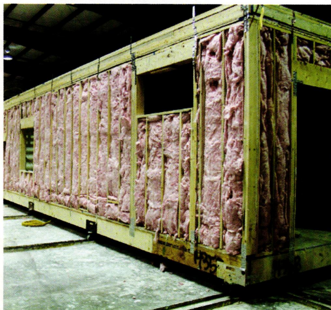
Right : The house being craned into place. Below : The house being assembled at the factory.
