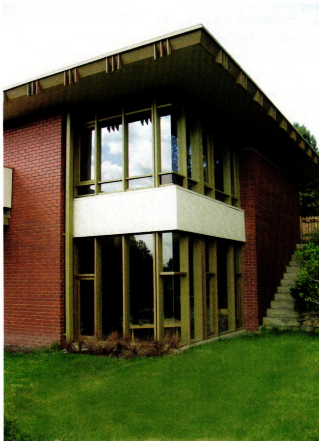
Above right: Built-in closets in the master bedroom. Above: A view from the front yard highlights the mitered glass corners and roof details.
