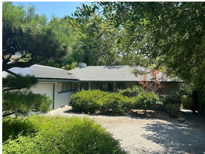
The 1941 Holmes House, Altadena, designed by Whitney Smith .
