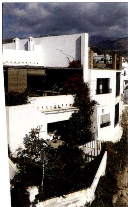
The three terraces protrude out over the cliff ▽ and help to give the town its whitewashed, cubistic image.
