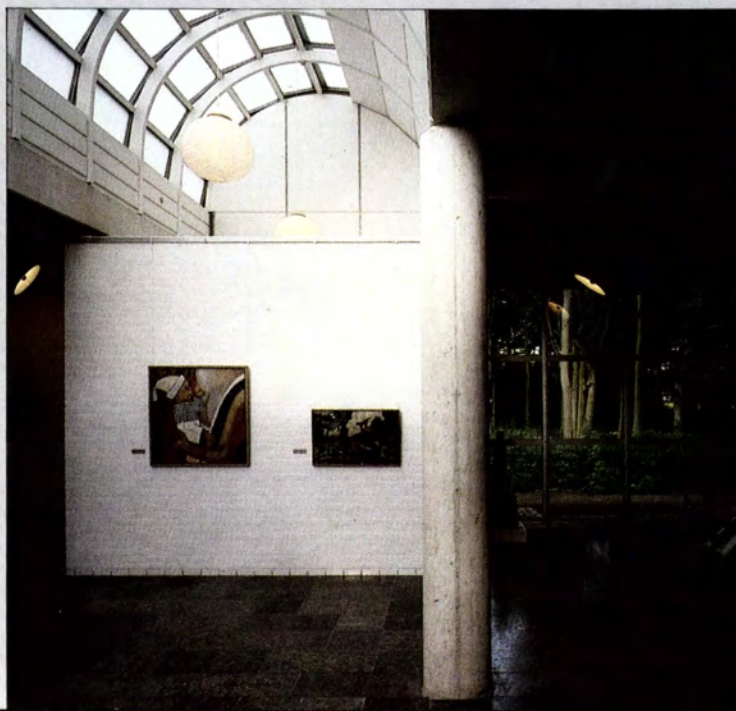
The artificial lighting is supplied by partially shaded lamps directed at the paintings. Lighting tracks between the ceiling elements allow flexible positioning of lighting fixtures.
