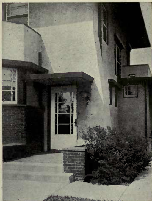
Effective use of brick with stucco to enrich the entrance
