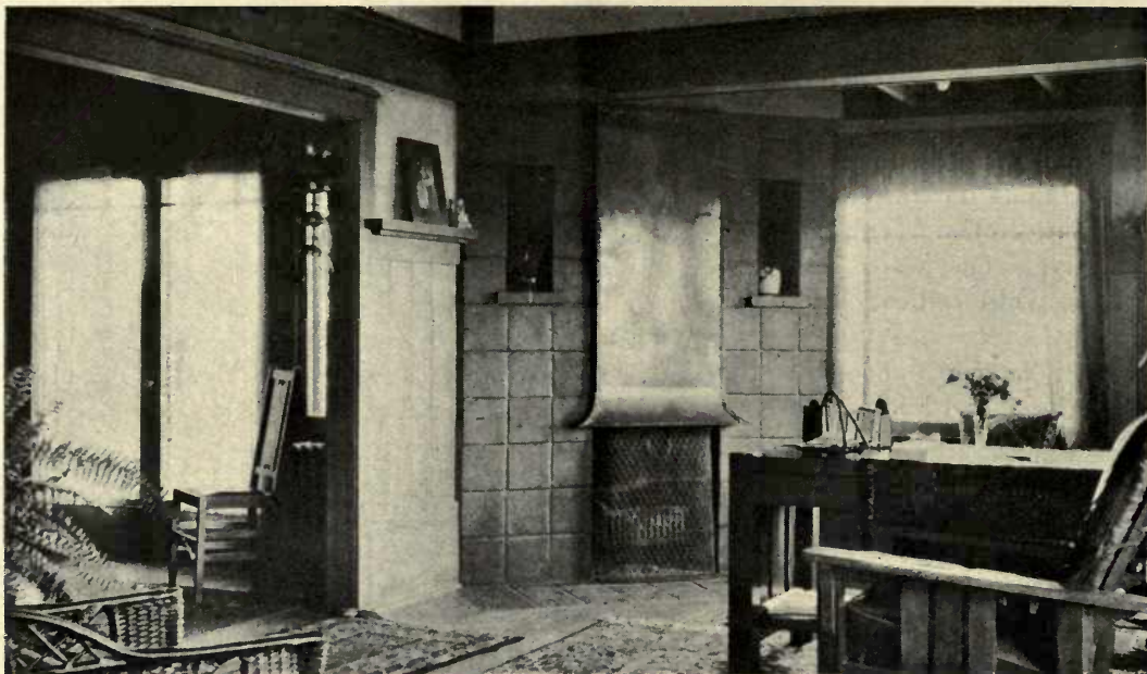
The living room fireplace built of tile and hooded with copper.
