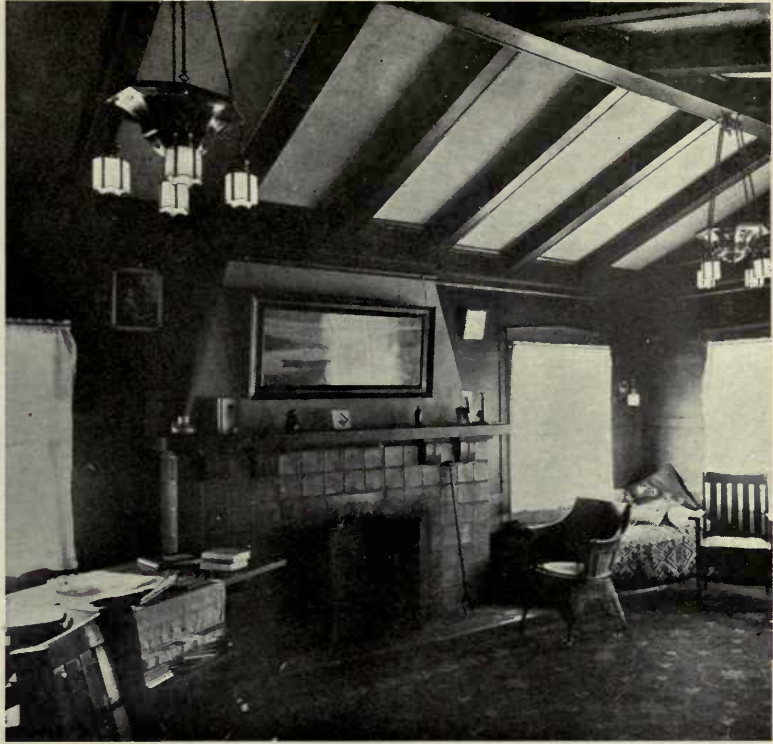
A. L. DuPuy, Architect. The ceiling is plastered between the exposed rafters.
