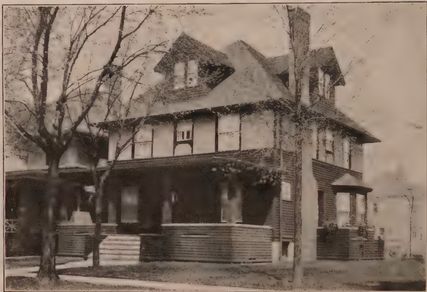
Frame and Plaster.
