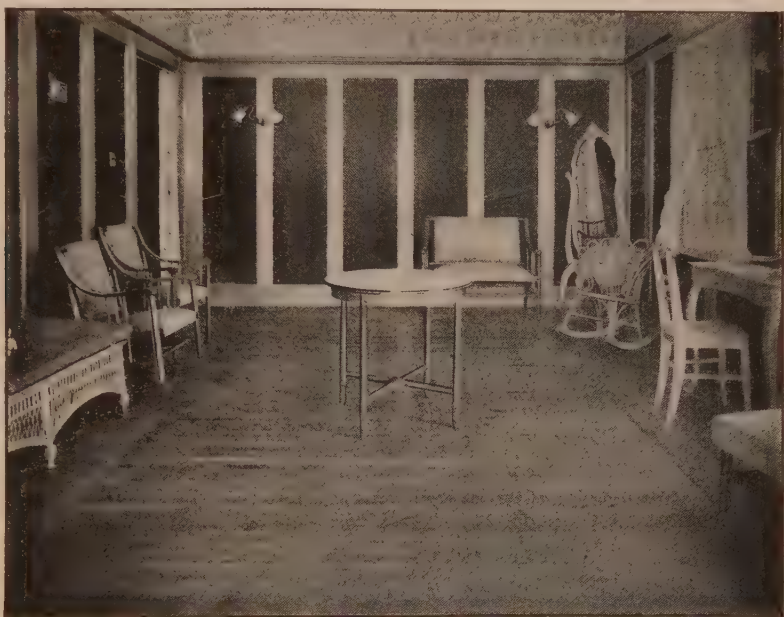
The Maple Floor in the Ladies' Rest Room.
