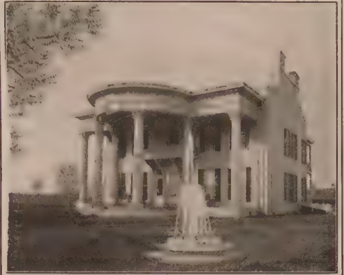
Residence of E. L. Atkins, Paducah, Ky., Supplied by Kewanee Water System
