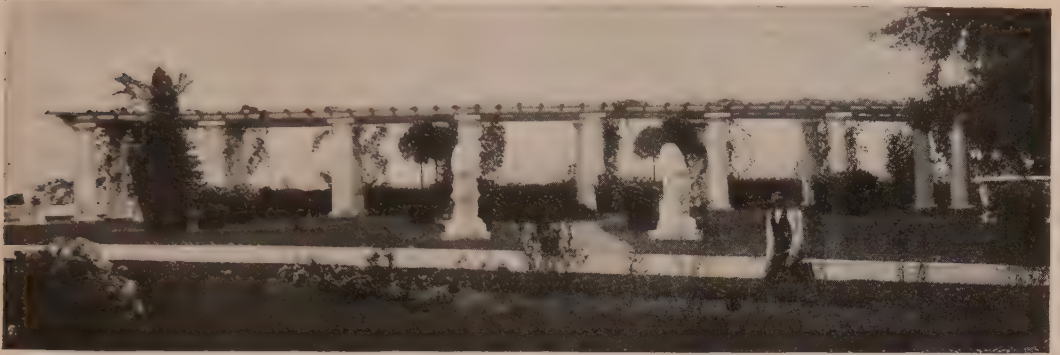
THE PERGOLA, WITH SIXTEEN DORIC COLUMNS
