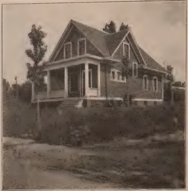
"THE COMPLETED HOUSE."
