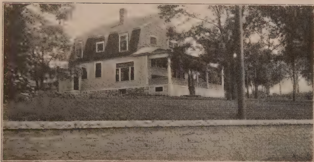
"A COLONIAL COTTAGE HOME."
