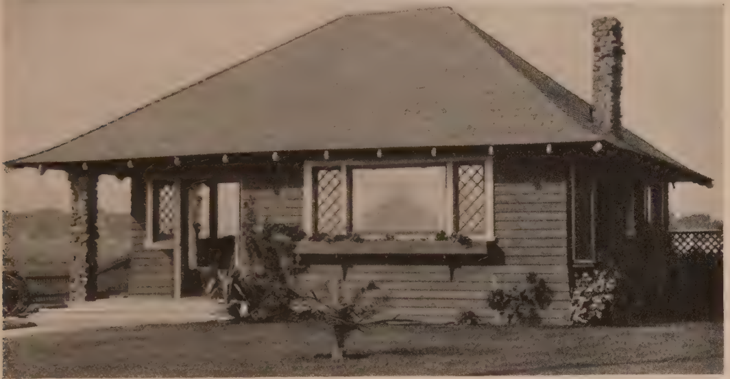
"CHIMNEY AND PORCH COLUMNS OF COBBLE STONE."
