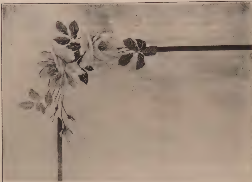
"CEILING FOR A DAINTY PARLOR."
