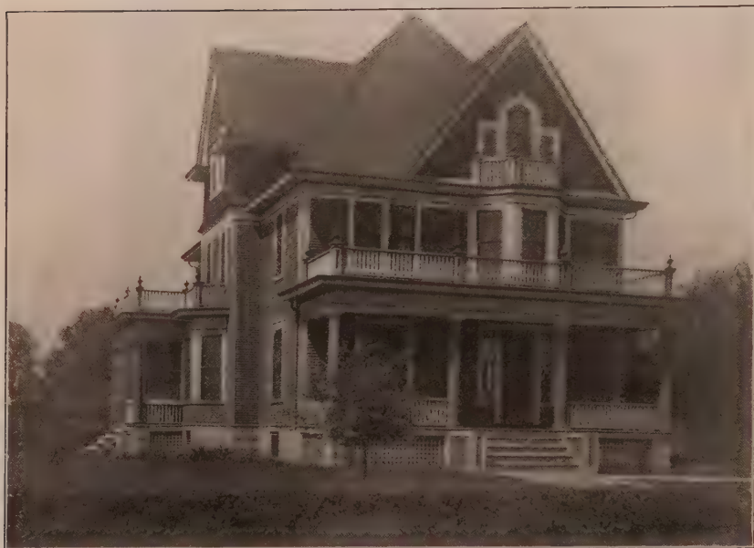
"THE COMPLETED HOUSE."
