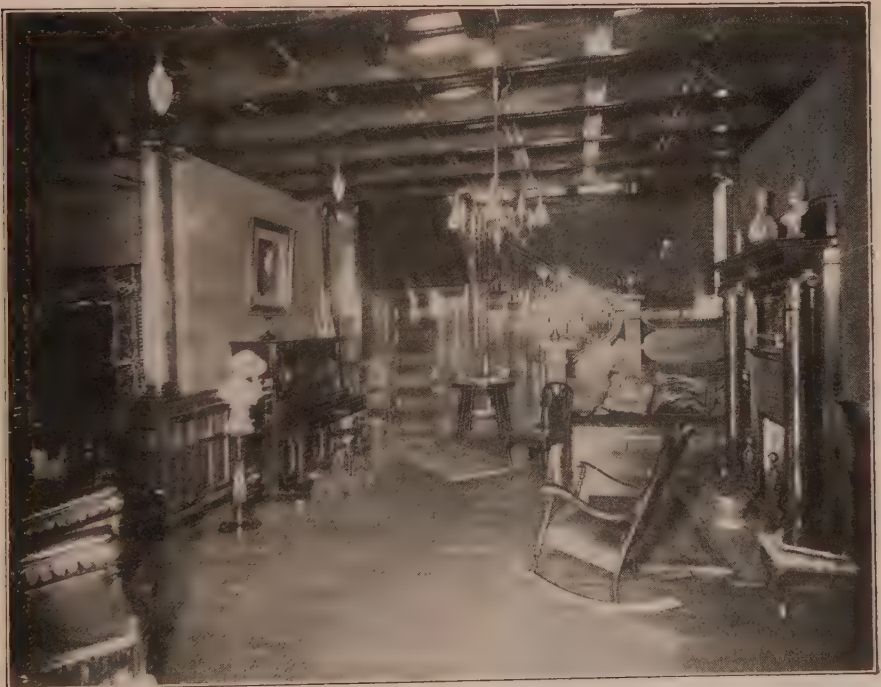
STAIRCASE HALL IN DESIGN A 124.
